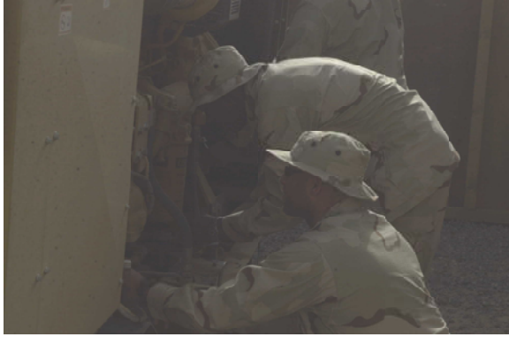
Left: Seabees repair a generator at Camp Whitehorse, An Nasiriyah.
