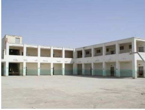
Left: Courtyard view of the Fatah School during renovation.
