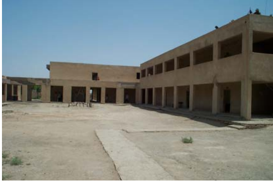
Left: View of the El Qura school courtyard before work began.
