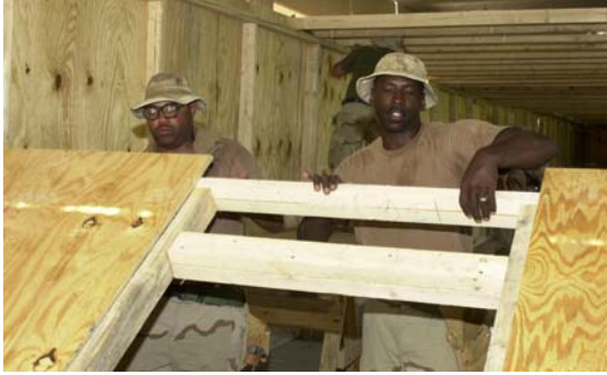
Left: Builders in the process of putting up a wall.
