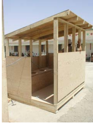
Left: A four-hole burnout constructed for the Marines.
