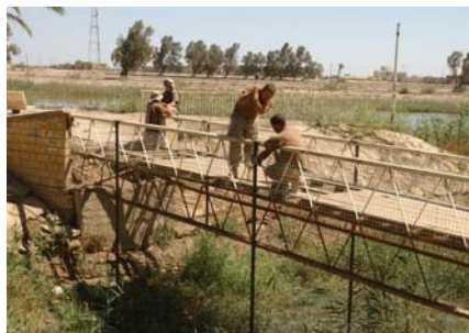
Left: NMCB SEVEN personnel replace boards in the footbridge at the park.
