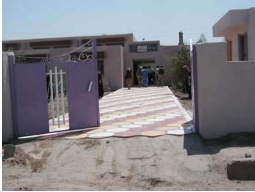
Left: Frontal view of the Al Zware School. The outer wall was rebuilt and plastered and a new gate was installed.
