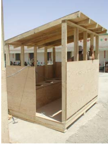
Left: A fourhole burnout built by NMCB 7 personnel.
