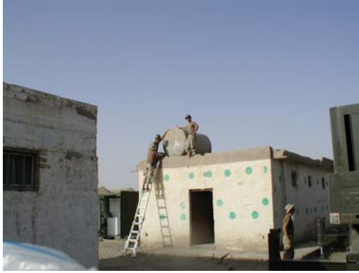
Left: Personnel from NMCB SEVEN work on the water tank.
