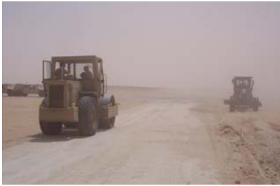
Left: Equipment Operators work on a parking apron for the Marine Cot Lot at Camp Fox, Kuwait.
