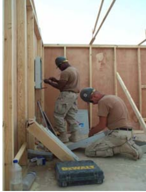
Left: Construction Electricians work to install electrical fixtures in this Seahut.
