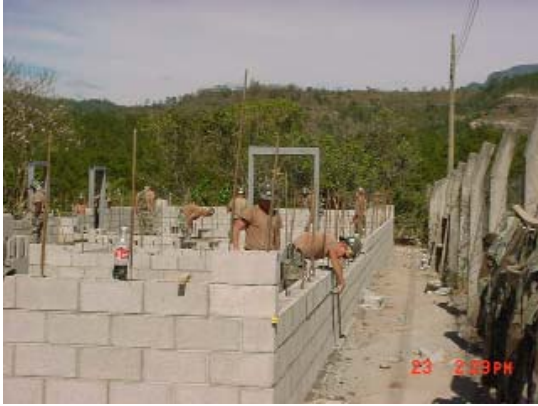
Left: Laying block and installing doorframes. Below: completed schoolhouse.
