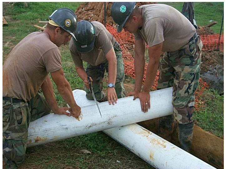
Cutting new 8-inch PVC pipe for water main.
