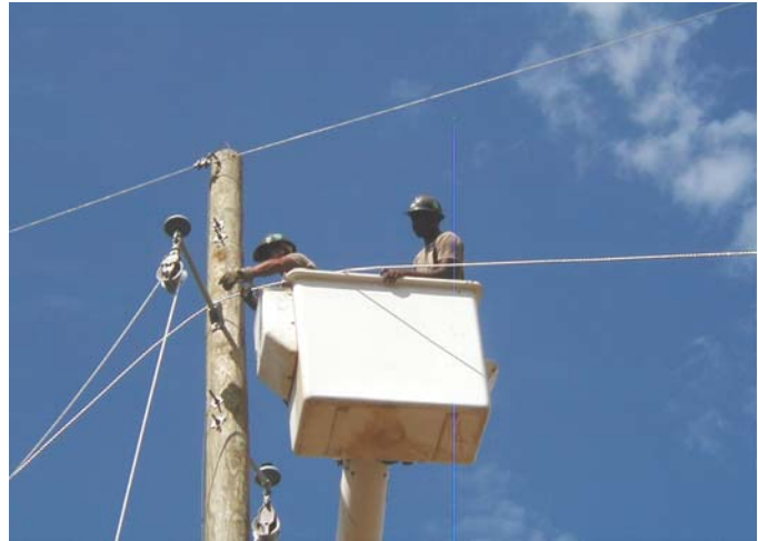
Left: The crew places one of the many power poles on top of a hill. Below: Seabees from NMCB 7 install the high voltage lines onto the stand-off brackets.
