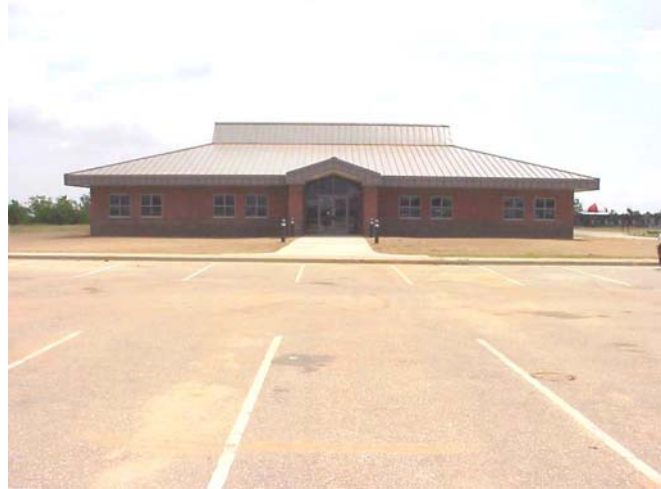
At left, erecting structural steel (October 2000). Below, completed facility (April 2001).
