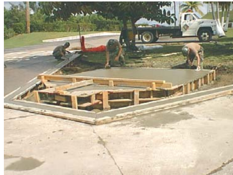
Left: Installing playground equipment, and the finished product. Above: Finishing concrete for the NAVSOUTH entrance.
