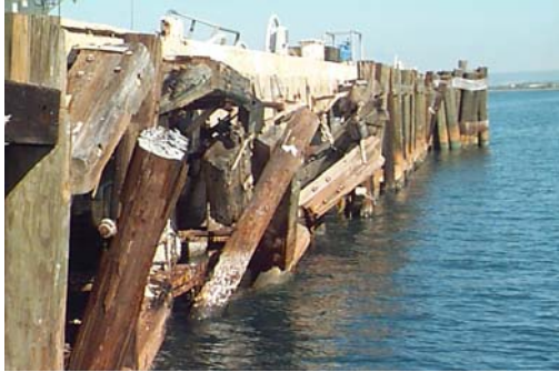
Left: Pier Victor starboard side prior to the removal of the old fender system. Below: The completed portion of the starboard fender system.
