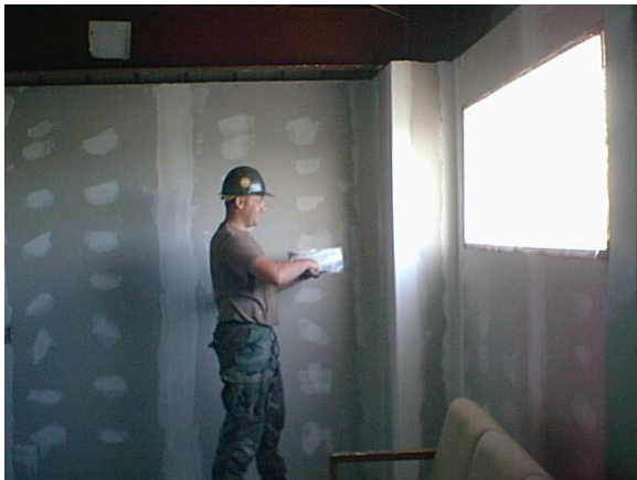
Above: Finishing drywall in Supply rehab job; Right: Augment Reserves assist in TOA Warehouse re-skin project.
