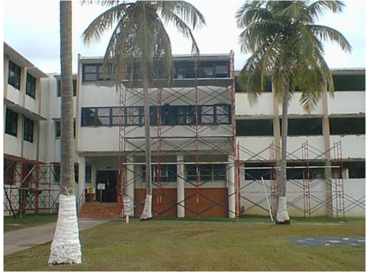
Left: Existing windows in October 2000. Below: New windows being installed (March 2001)
