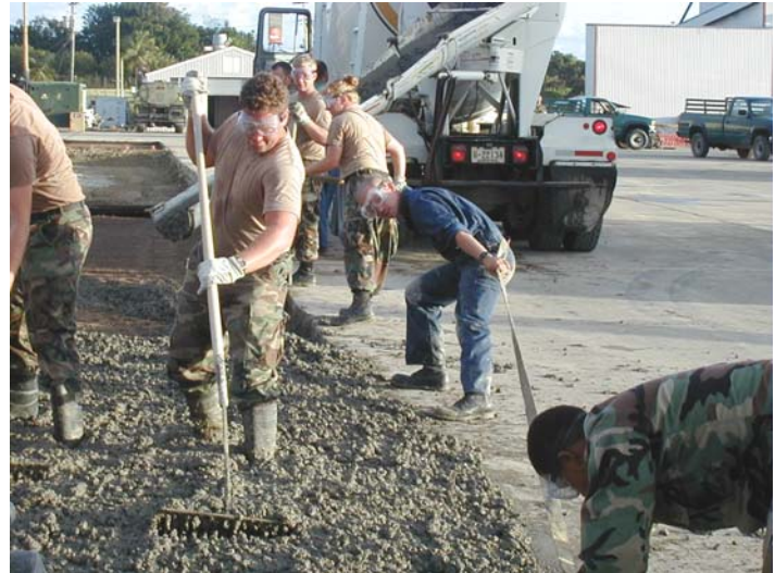
Left: Project location. Below: Concrete placement in progress.
