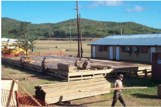
Left: Installing the plywood sub-floor. Below: Completed SEAhut.
