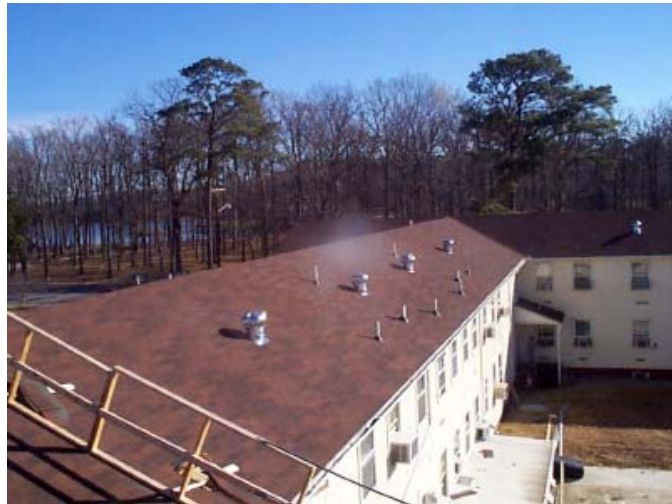
Left: Roof Replacement underway (December 2000). Below: Middle section completed (January 2001).
