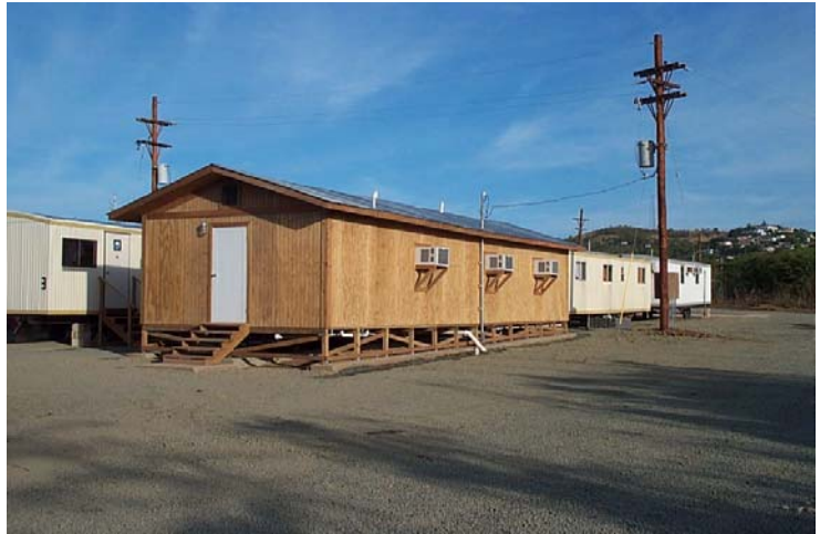
Left: Seabees from NMCB 7 clear the site that will house the POPR berthing camp. Below: The completed building shower and laundry facility.
