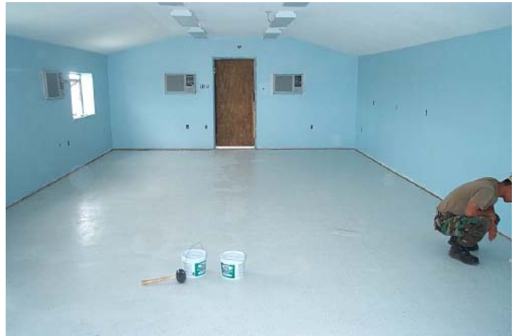
Left: Demolition phase. Below: Renovated dining area of Camp Garcia Galley.
