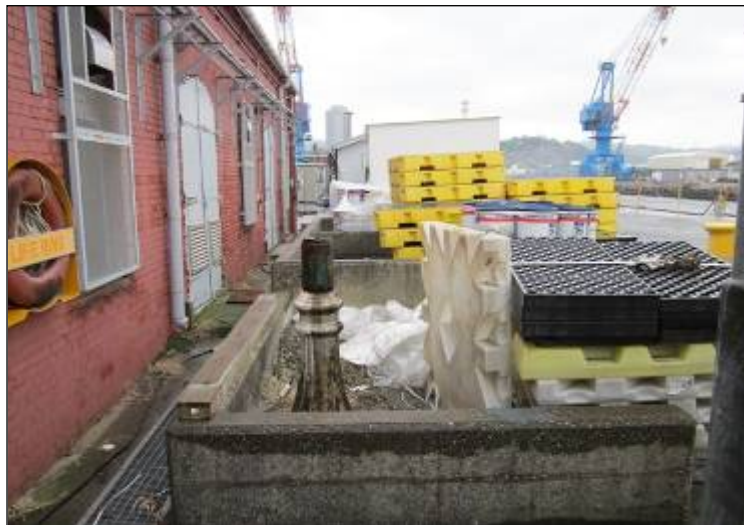
Eight concrete walls demolished for future HAZMAT lockers
