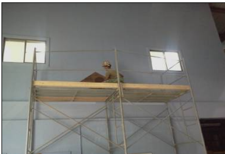
Painting wall in Alfa Shop
