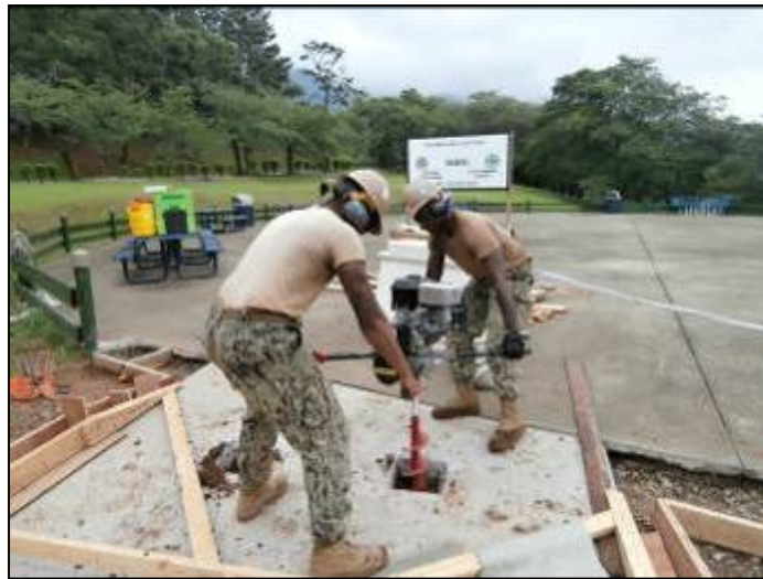
Digging holes for new bollards with the power auger
