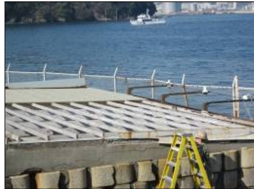
Demolishing an unstable roof
