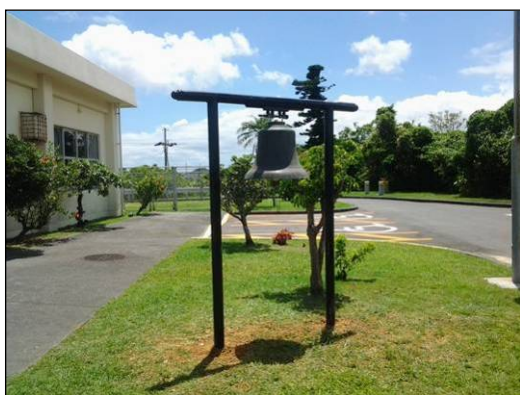
Construct frame for chapel bell
