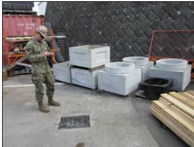
Completing inventory of materials
