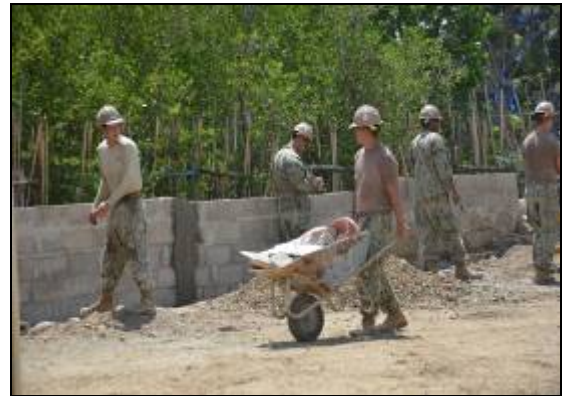
Perimeter fence at Aplaya ES
