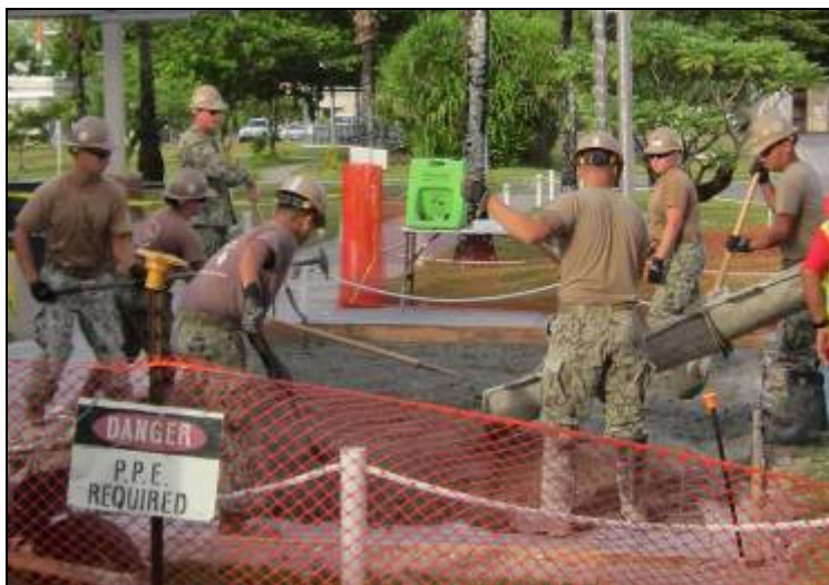
Placement of concrete bike parking pad for the island's ship store
