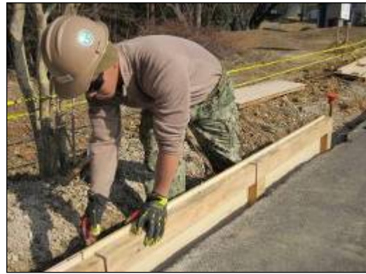
Placing new concrete sidewalks Placing forms for concrete curbs
