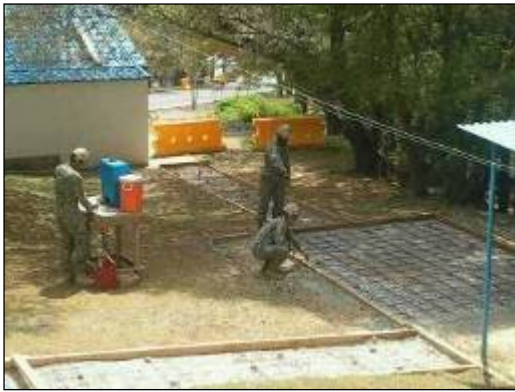
Placing new concrete sidewalks Placing forms for concrete curbs
