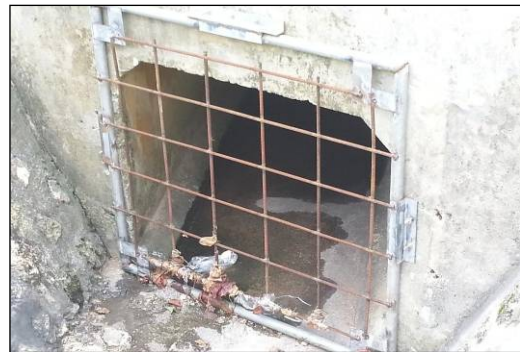
Repair Drainage Grates
