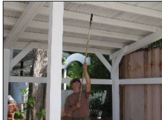
Finishing the sail storage shed
