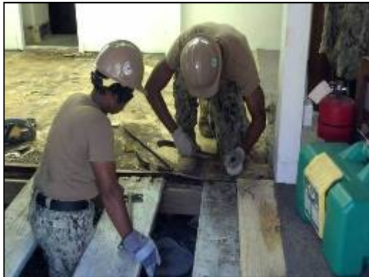
Replacement of flooring
