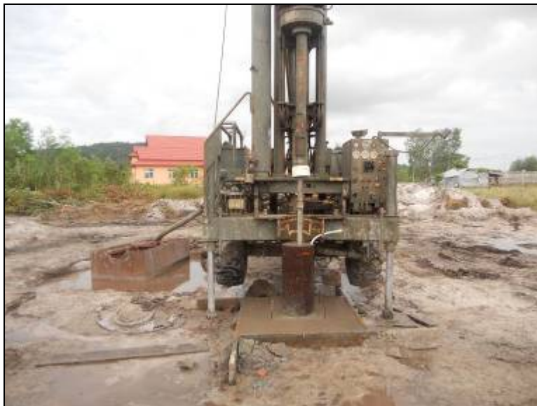
Finishing up REAM Naval Base water well project
