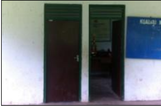
At left, the initial site conditions are pictured. Below is the completed building.
