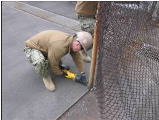
Cutting out rusted fencing
