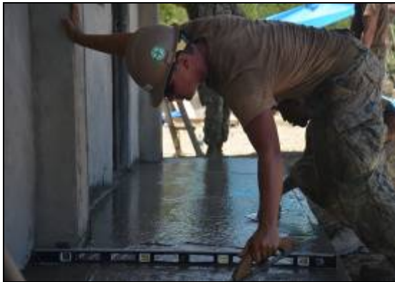
Placing sidewalk at Aplaya ES
