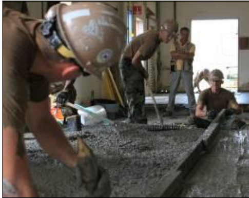
Crew places concrete pad
