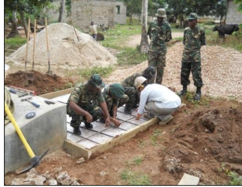
EO1 (SCW) Perez instructing TPDF members on setting rebar
