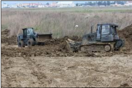
D7s push berm near airfield
