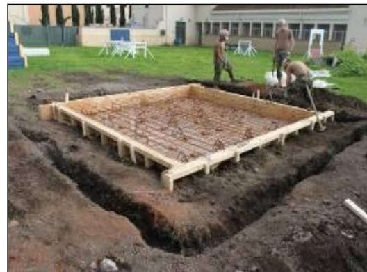
Crew examines formwork
