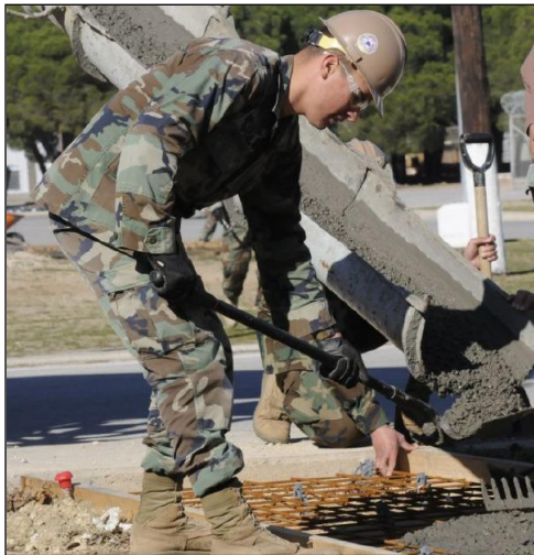
Crew prepares pad for light pole.
