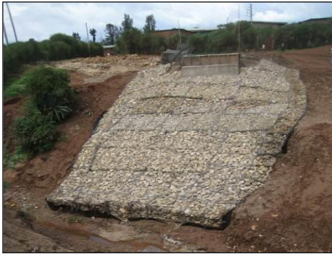
Retaining wall, to protect bridge foundation
