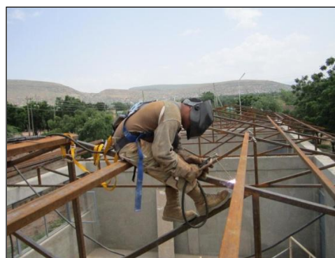
Seabee welding roof truss
