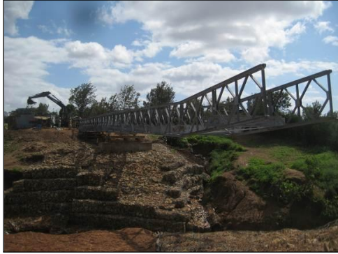
Det personnel launching bridge
