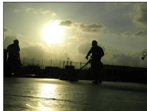
UT3 (SCW) Richardson whirley birds the LAMS II concrete slab
