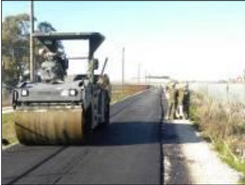
Roller compacts road at project site
