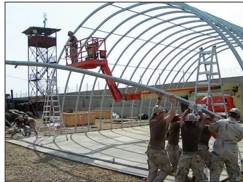
Alfa Company erects the tent for an improved maintenance shop
