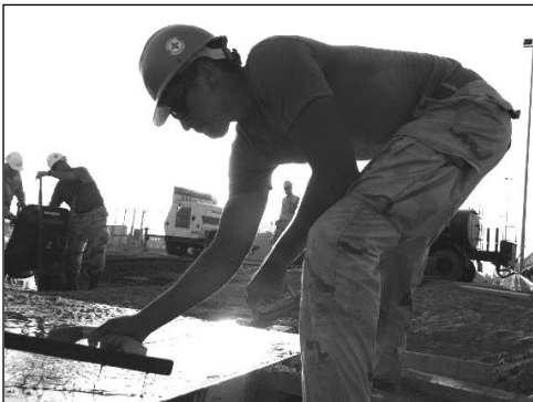
BU CN (SCW) Sanchez hand finishes the LAMS II concrete pour
