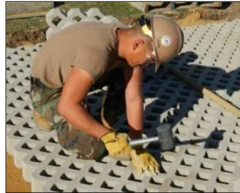
Crew places and levels paver stones
