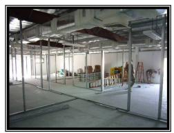
Erecting metal studs.
