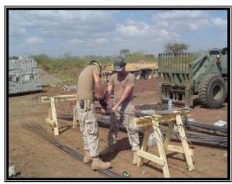
Seabees prefabricating rebar for footers.
