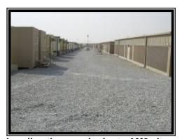
Leveling the gravel prior to AM2 placement.
