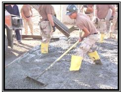
Placing concrete pad extension.
