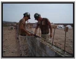
Seabee installing CMU block for wall.
