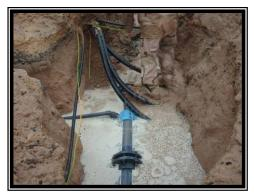
Repairing mechanical coupling.
