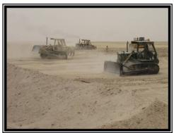
Operators create the exterior berm.
