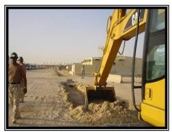
Excavating existing drainage ditch.
