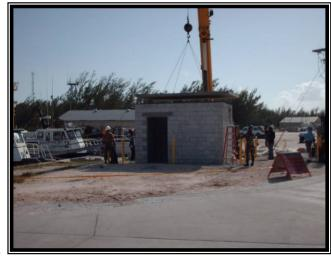
Erecting the pre-cast concrete roof in place.
