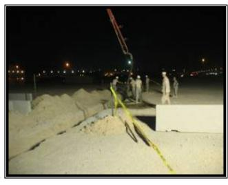
Concrete placement prior to back fill.
