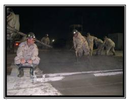
Seabee screeds placed concrete.
