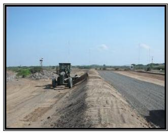
Completed v-ditch, road, and berm.
