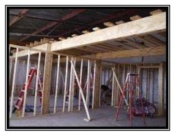
Framing of walls and joists.
