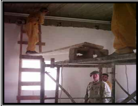
EA2 McClay observes local national contractors repairing a roof.
