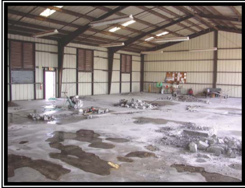
Excavation of mezzanine foundations.
