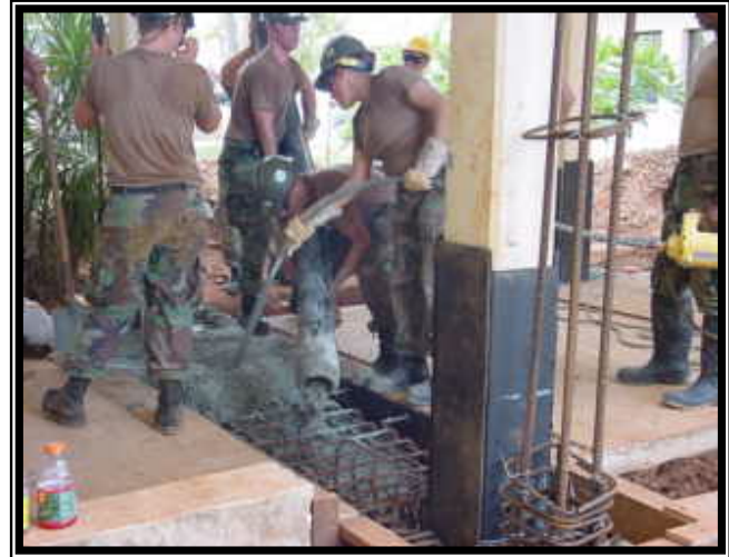
Concrete placement of grade beams.
