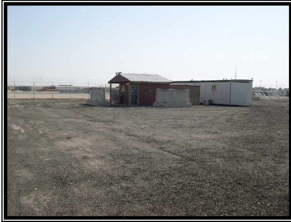
Completed asphalt milling project.
