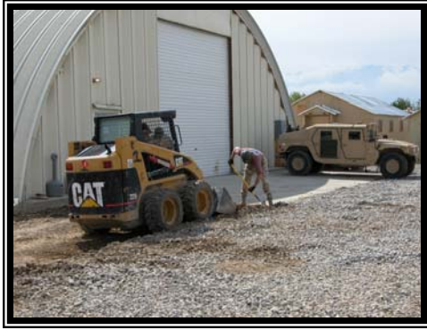
Excavation for formwork.
