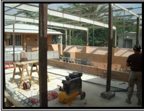
Initial stages of building addition.
