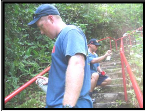
Maintenance of stair railings.
