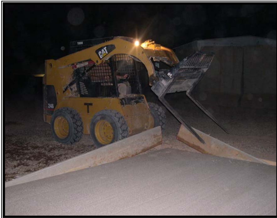
Stripping forms from a generator pad.
