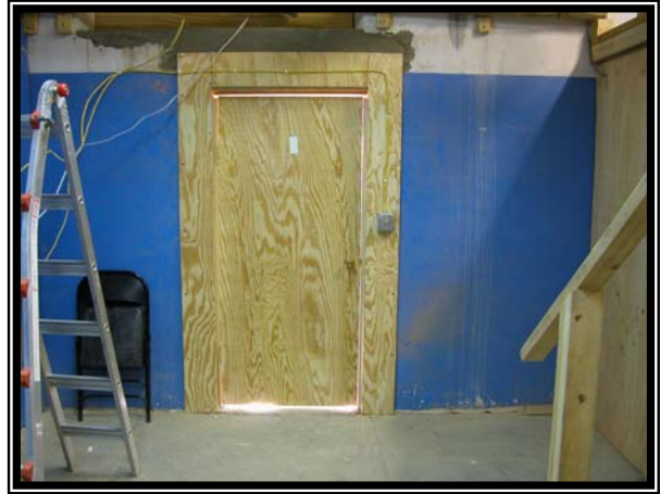
Installation of new door in concrete wall.
