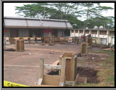
Formwork for concrete foundations.
