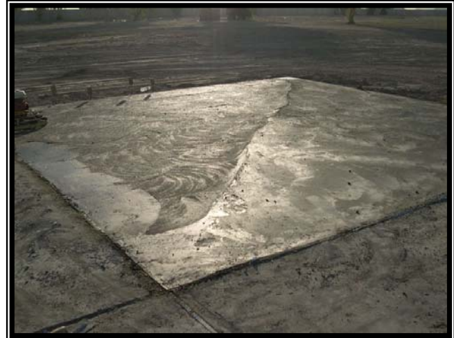
Helo pad under construction.
