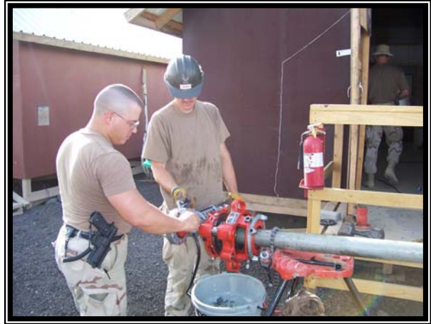
Seabees performing plumbing repairs.
