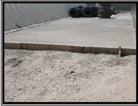
Initial concrete placement.
