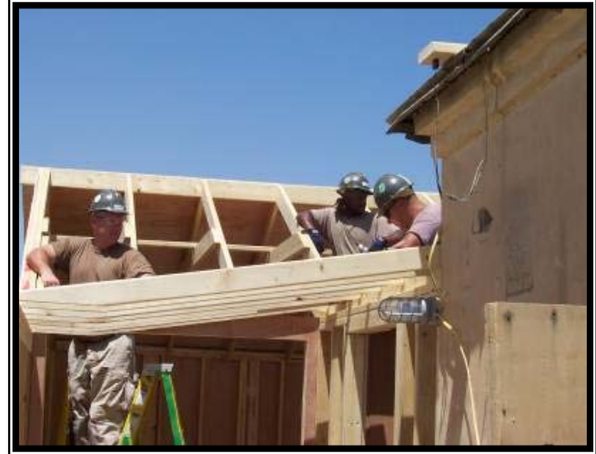
Seabees installing rafters for a building tie in.
