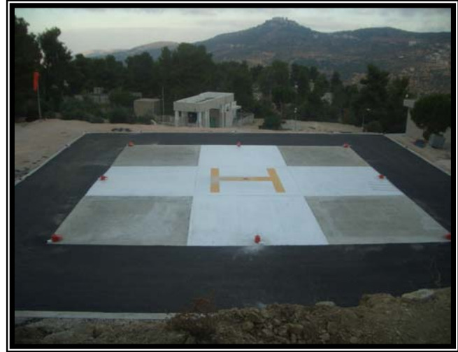
Completed helo pad.
