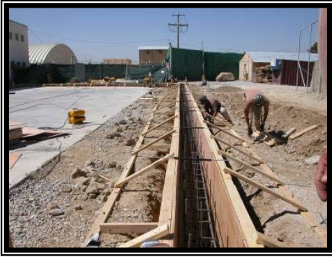
Formwork for the footer.
