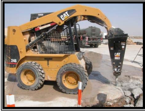
Site Work for Keyway and Footers.
