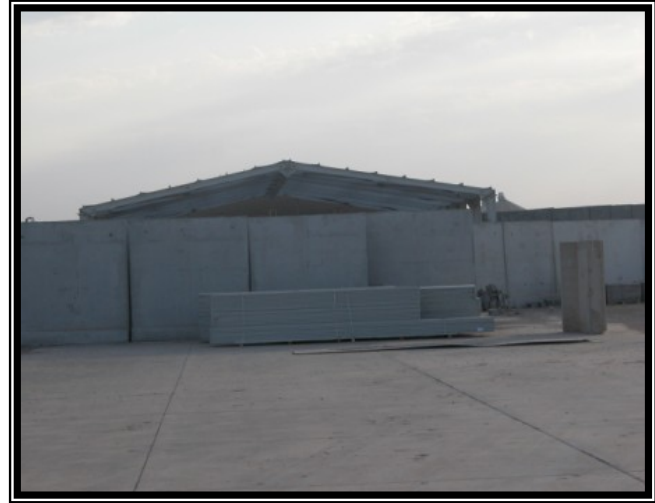
OPSEC screening of ongoing project.
