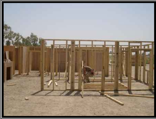
Seabees build an outdoor shoothouse.
