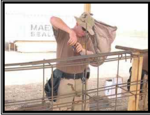
A Seabee prepares the footing.
