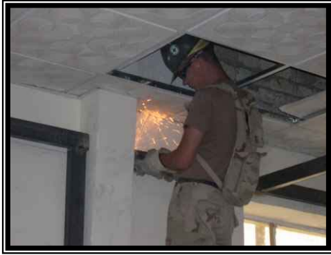
A Seabee welds the steel cage.
