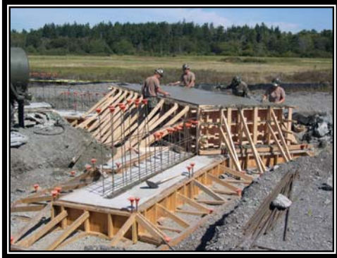
Placement of concrete for one of two abutments.
