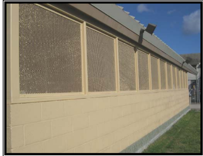
Completed kennel addition.
