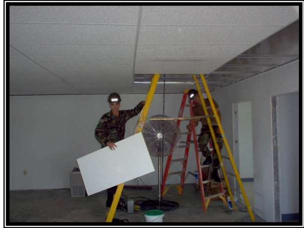
Installing ceiling tiles in new project office.
