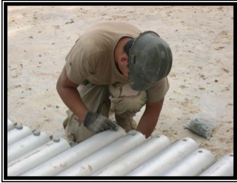
A Seabee assembles structural members.
