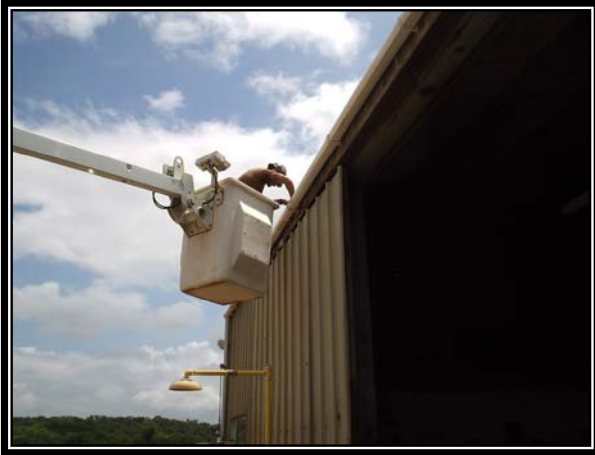
Seabee fixing rain gutter.
