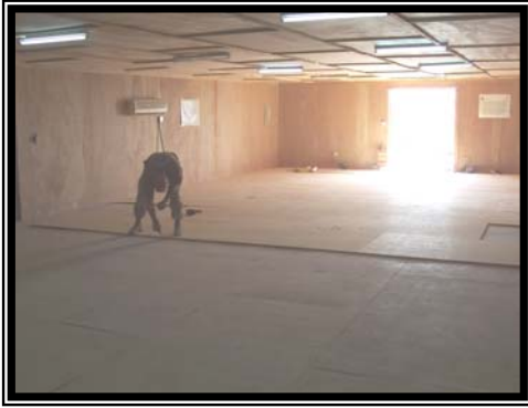
A seabee installs plywood subfloor.
