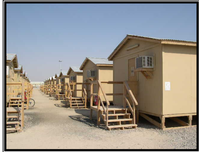
Completed SWA huts.
