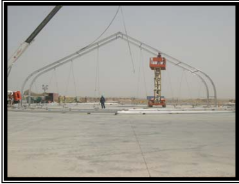
Structural steel erection.
