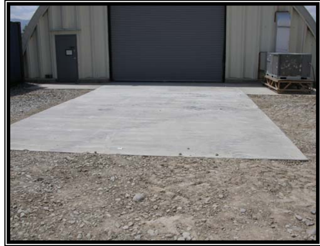
Completed concrete pad.
