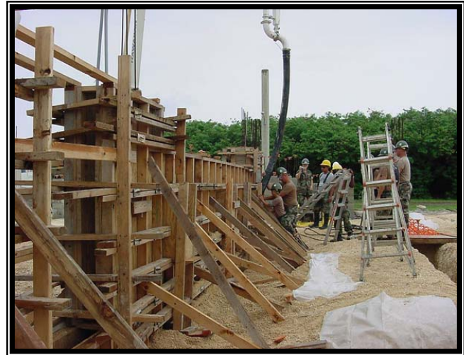
Seabees placing concrete.
