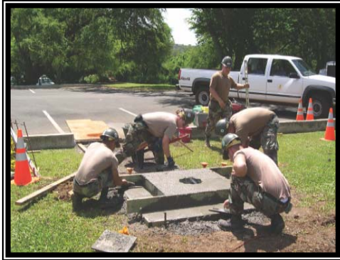
Finishing concrete for foundation.
