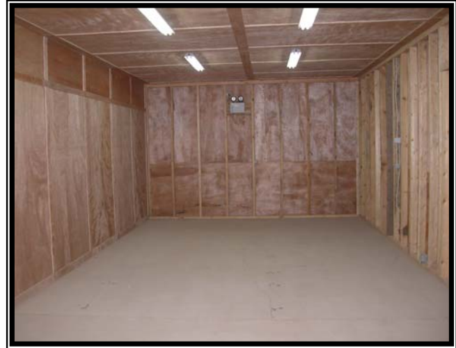
Completed storage spaces.
