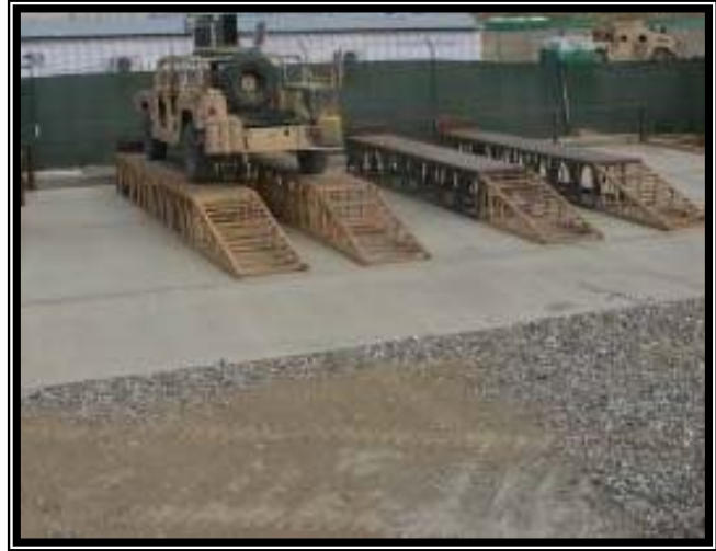
Completed wash rack.
