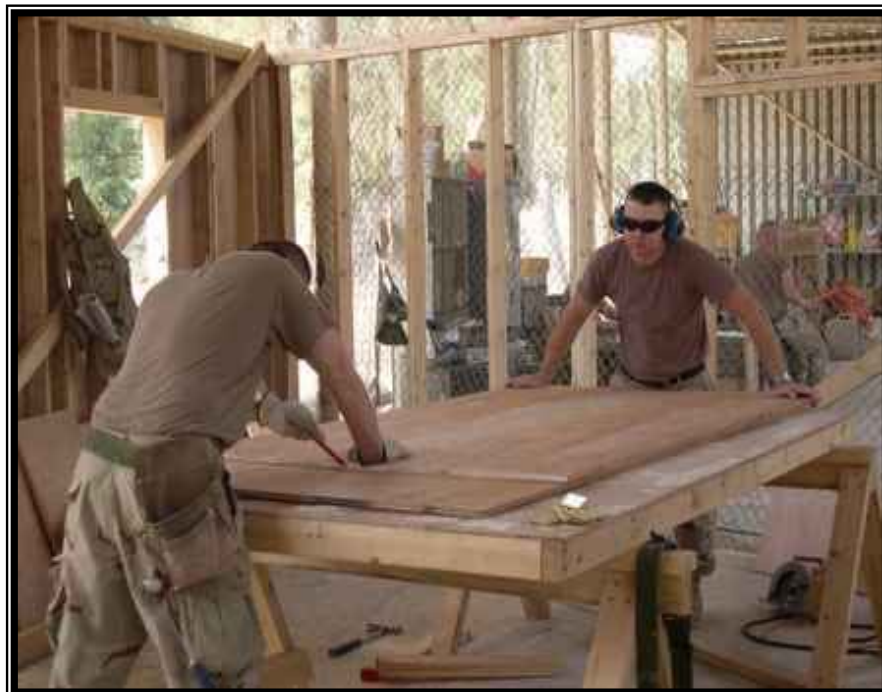
Seabees construct a new builders shop.
