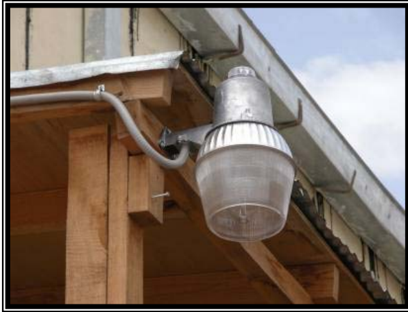
Install exterior security lighting
