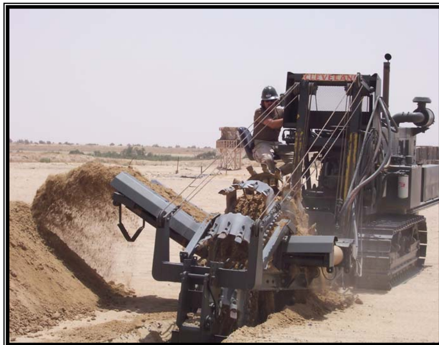
Seabee trenching the sewage lagoon.
