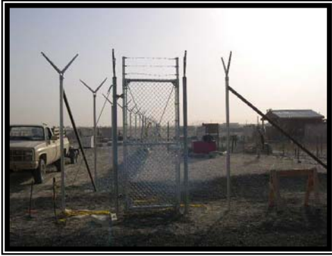
Installation of personnel gate.
