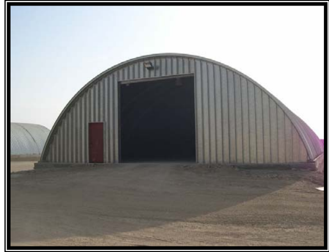
Completed K-span.
