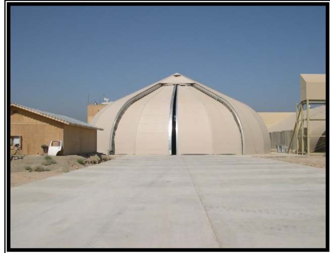
Completed hangar and taxiway ramp.
