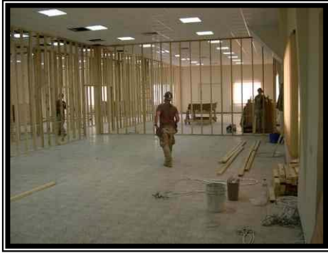
Seabees finish framing interior walls.
