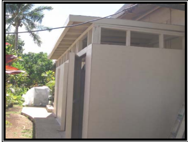
YMCA Bldg 89 shed replacement.
