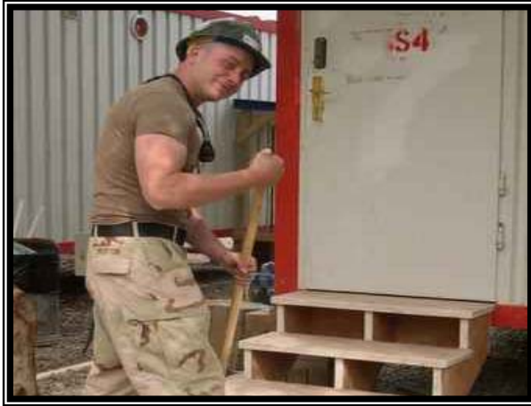
Building stairs in the trailer park.
