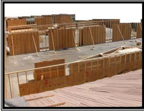
Initial framing of exterior walls.
