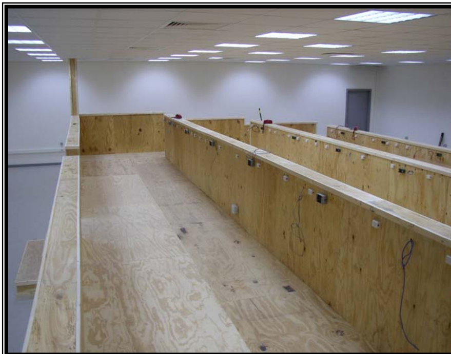
Construction of JOC platform.
