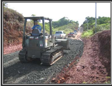
Spreading gravel.
