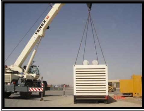
Seabees install a 1.2MW generator.
