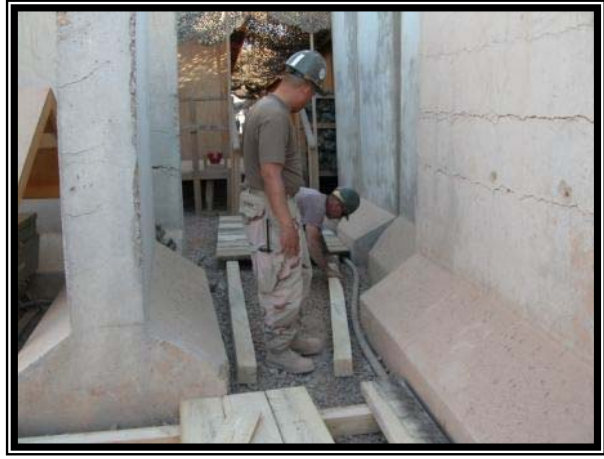
Installing a wooden walkway.
