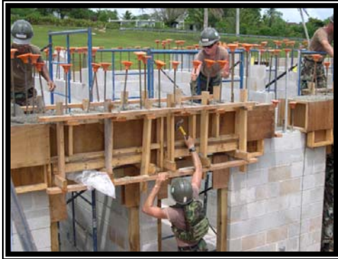
Seabees placing the concrete lintel beams.
