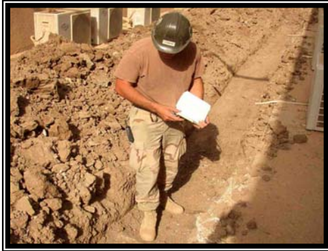
BU1 Ciman inspects sanitary sewer excavations.
