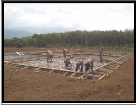
Installation of reinforcing steel.
