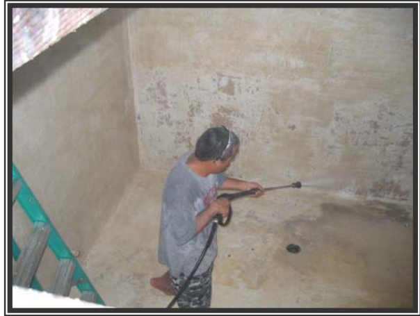
Local apprentice cleans potable water tank.
