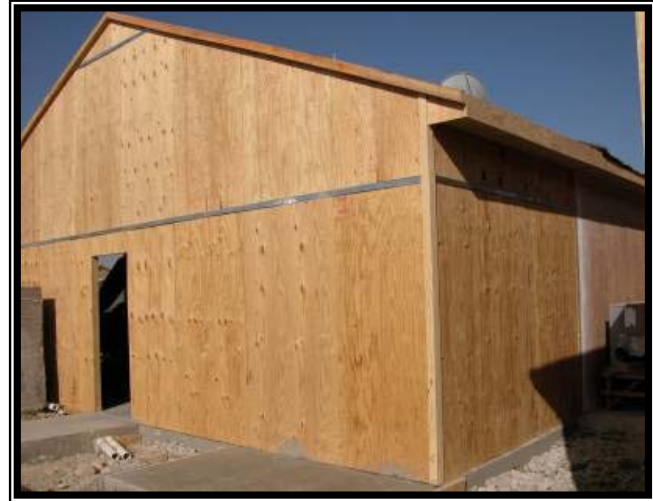
Nearly completed building.
