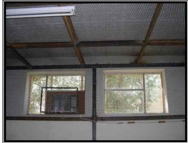
Completed steel cage for the CIF.
