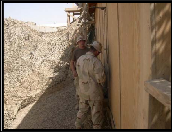
Bravo company servicing A/C units.
