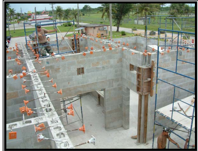
Completed CMU walls.
