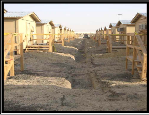
Partially backfilled trench for power lines.
