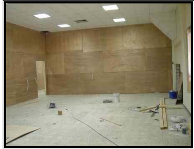
Completed wall with sheathing.
