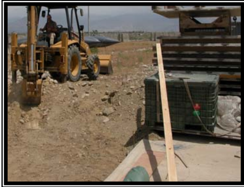
Sitework for concrete placement.
