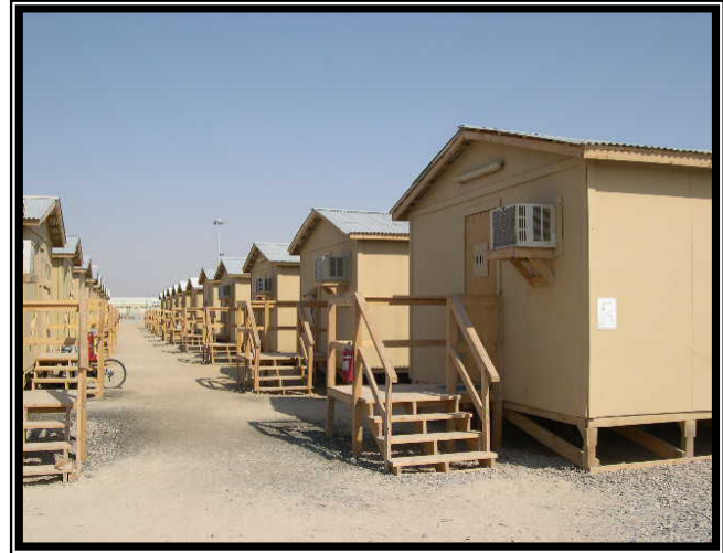
Completed SWA huts.
