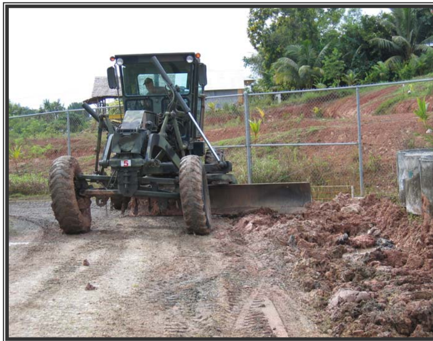
Grading V-ditch for proper camp drainage.
