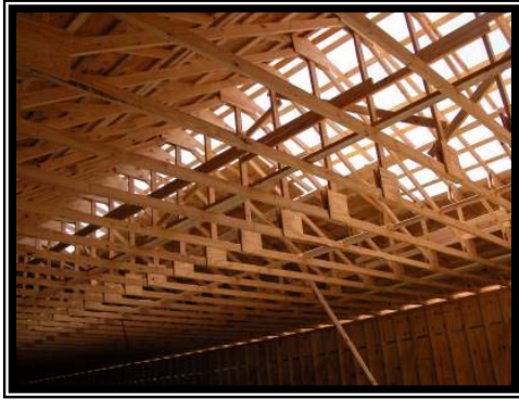
These completed roof trusses were fabricated on site.
