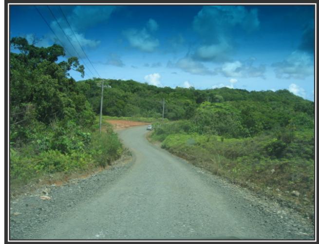
Completed section of cross island road.
