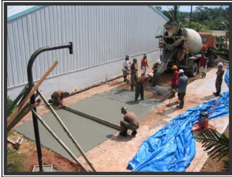
Placing 4" concrete slab.
