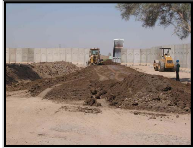
Contractor delivers fill for roadway improvement.
