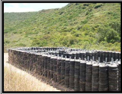
12' wall constructed of tires and sand.
