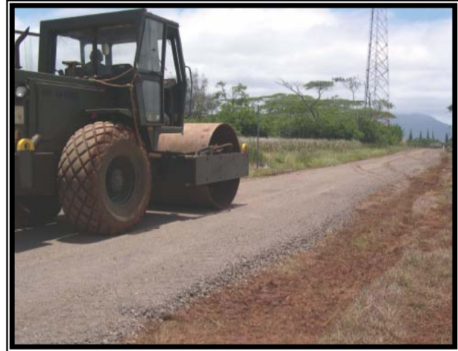
Compaction of gravel road.
