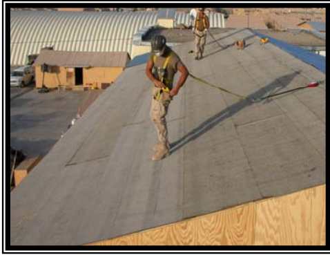
Initial installation of roll roofing.
