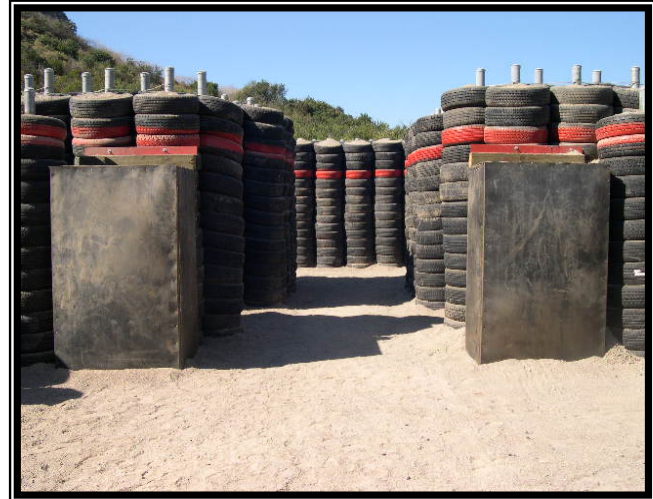
Completed interior walls of structure.
