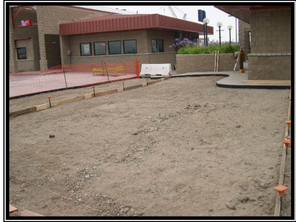
Excavation prep for sidewalk at Oasis.
