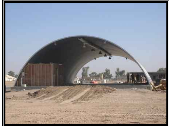
Nearly completed structure.
