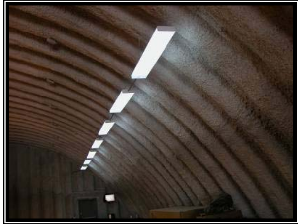
Install interior lighting for warehouse
