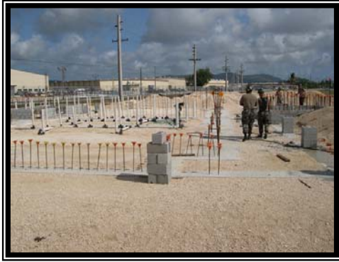
Layout of subgrade drainage piping.
