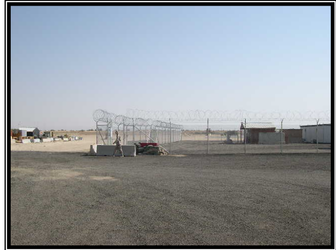
Completed security fence.
