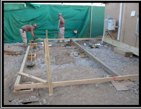
Seabees place concrete piers.
