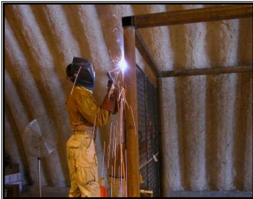
Fabrication and installation of secure storage area.
