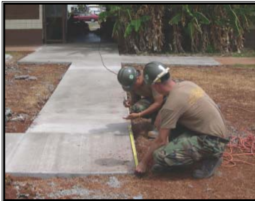
MCBH sidewalk construction.
