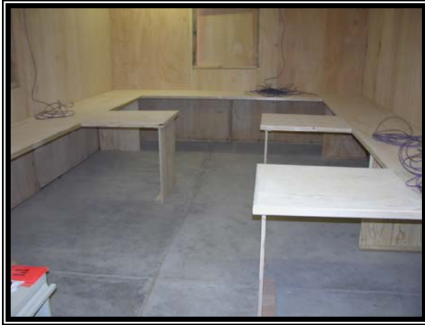
Fabrication and installation of new desks.
