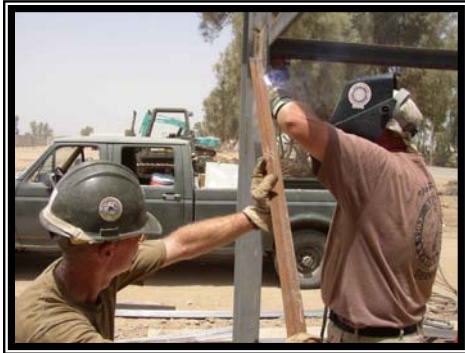
Seabees building a new ECP guard tower.
