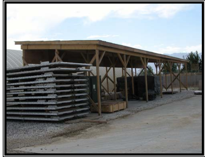
Completed pole barn.
