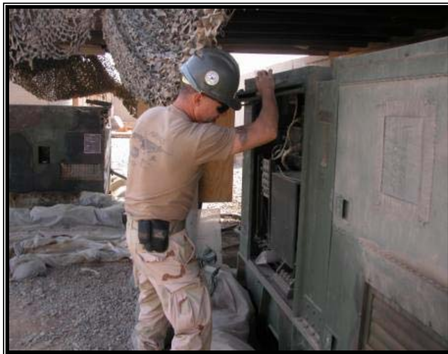
A Seabee performs preventative maintenance on a generator.
