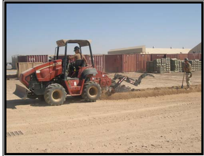
Seabees digging a trench for PVC conduit.
