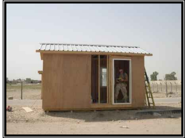
Seabees construct a guard shack.
