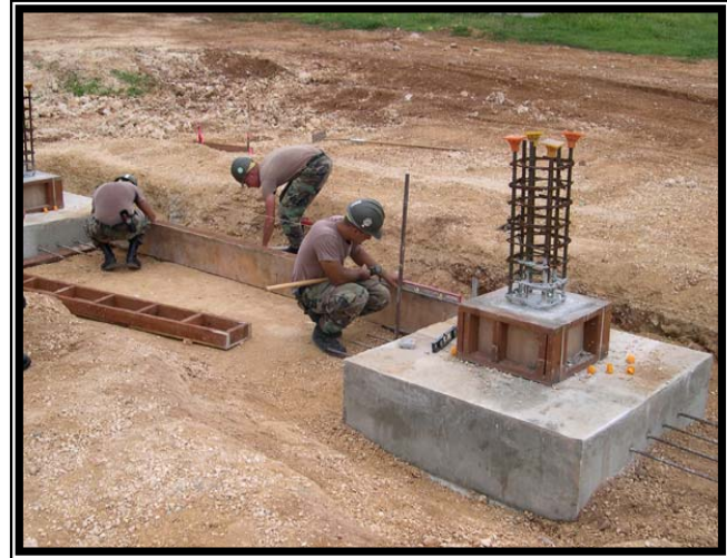
Installation of grade beam forms.
