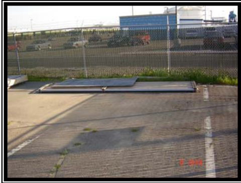
Building site prior to construction.
