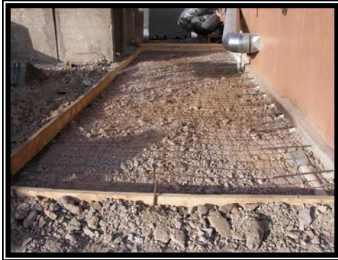
Initial concrete formwork.
