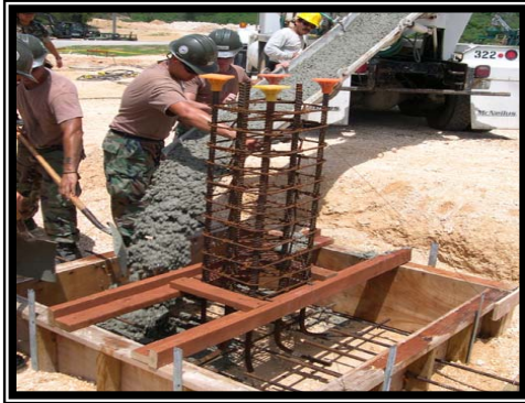
Seabees at work placing a spread footing.
