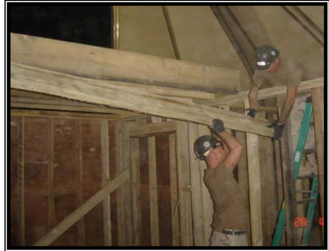
Seabees construct office space.
