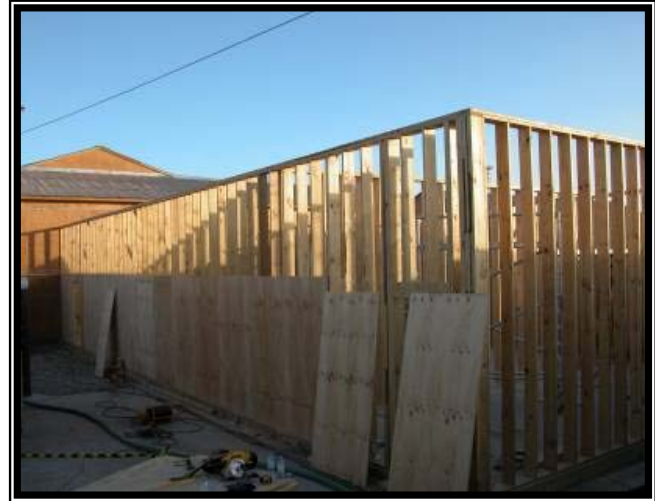
Exterior sheathing being installed.
