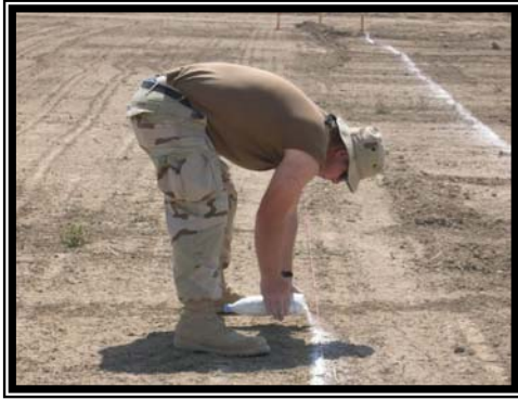
A Seabee lays out a concrete pour.
