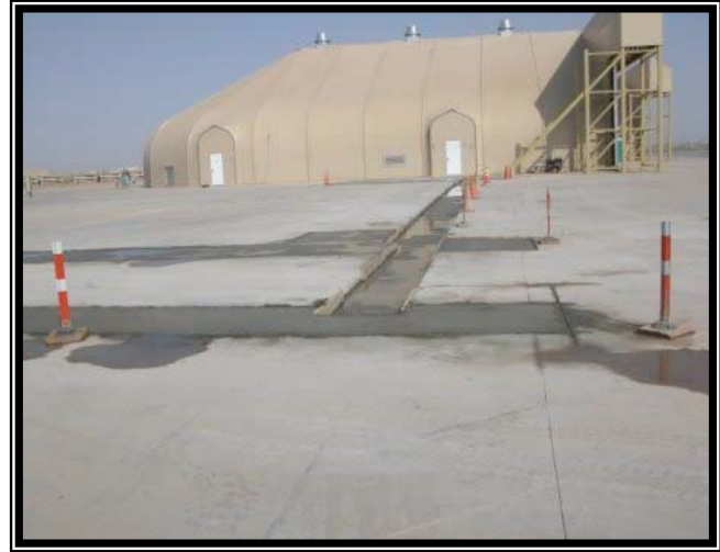
Completed Keyway and Footers.
