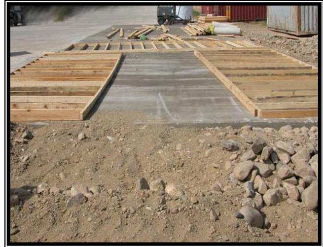
Completed concrete pad.
