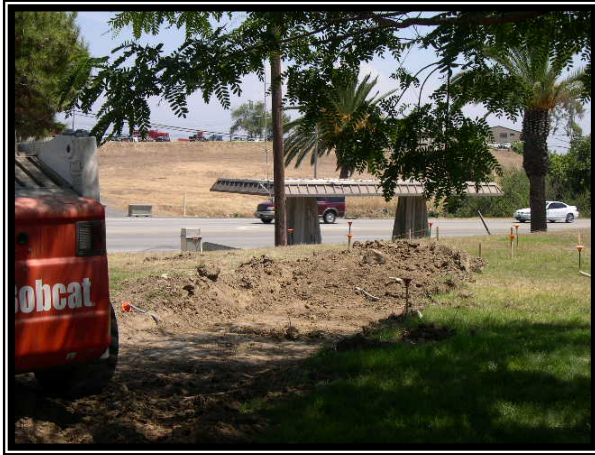
Site prep for sidewalk at childcare center.
