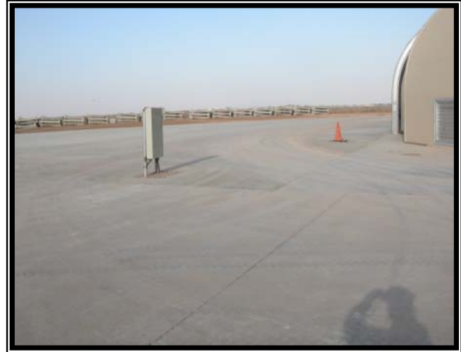
Finished concrete pad.
