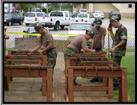
Seabees building rebar cages.
