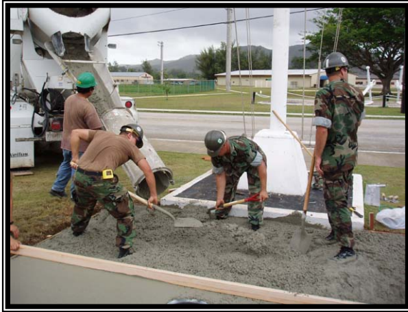
Placing concrete slab for new flagpole.
