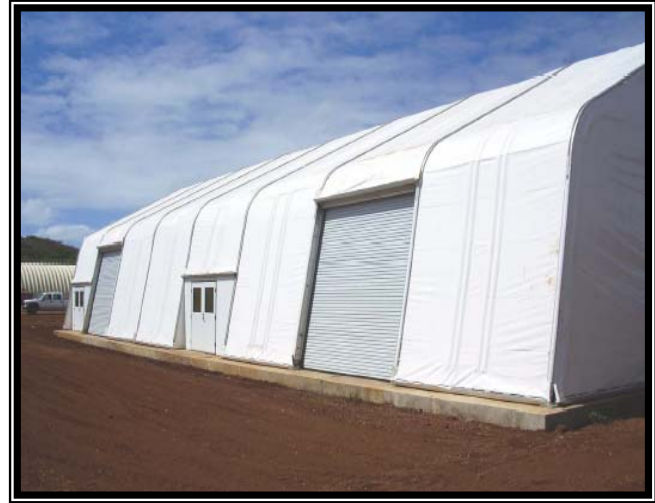
Completed Tension Fabric Structure (TFS).
