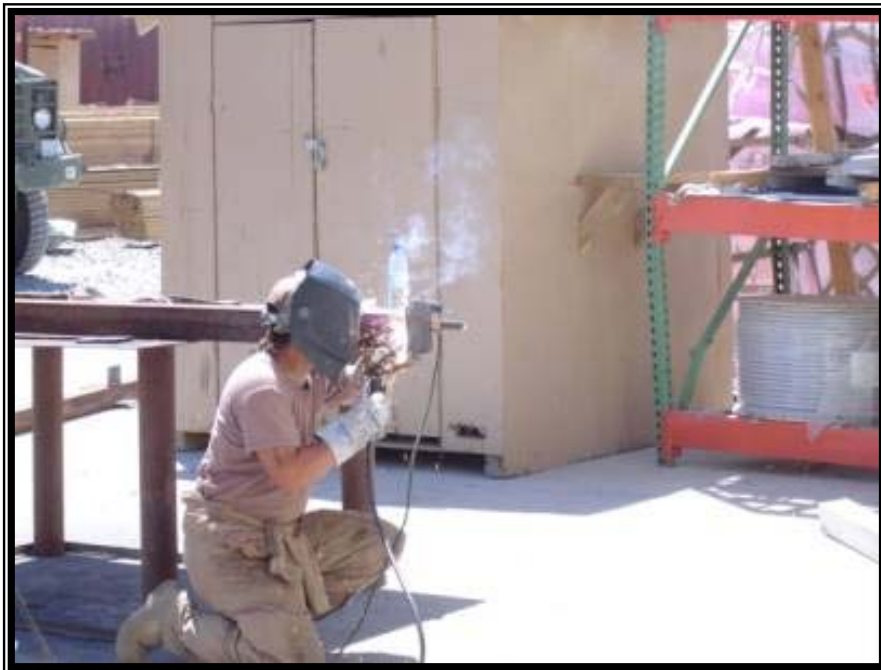
Seabee performing welding task.
