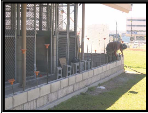
Construction of CMU wall.
