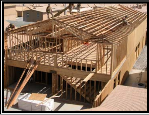
Initial rough framing.
