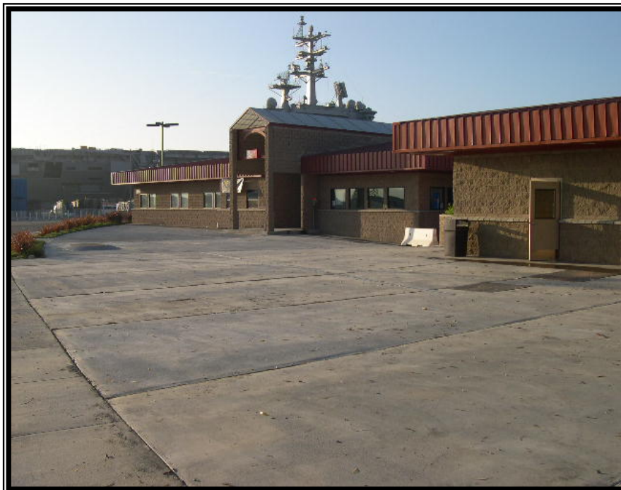
Installation of new drainage ditch and concrete..
