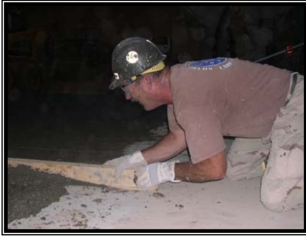
Screeding a fuel pad.
