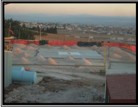
Initial site work.
