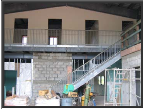
Interior of PEB.
