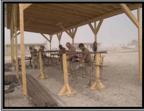
Seabees constructing footing rebar.
