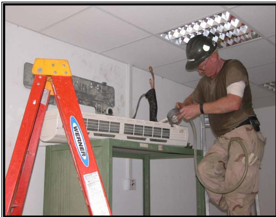
BU1 Davison replaces a faulty split A/C unit.
