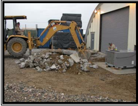
Removal of existing concrete.
