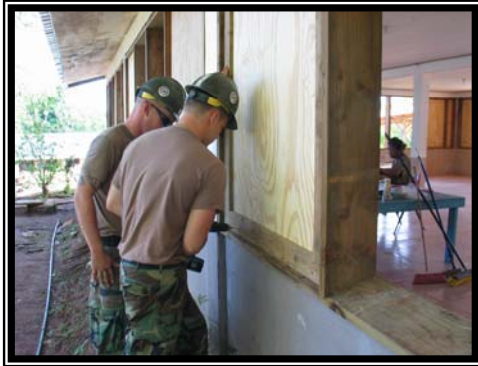
Installation of plywood dividers.
