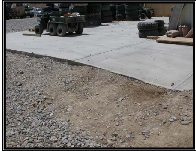
Completed concrete pad.
