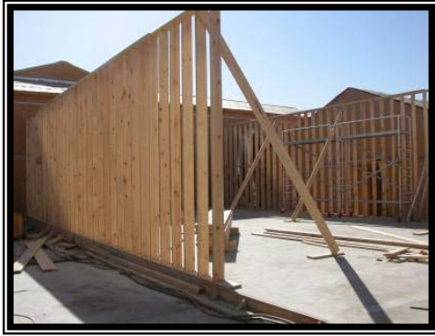
Exterior wall framing.
