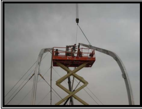
Seabees shown erecting structural steel.
