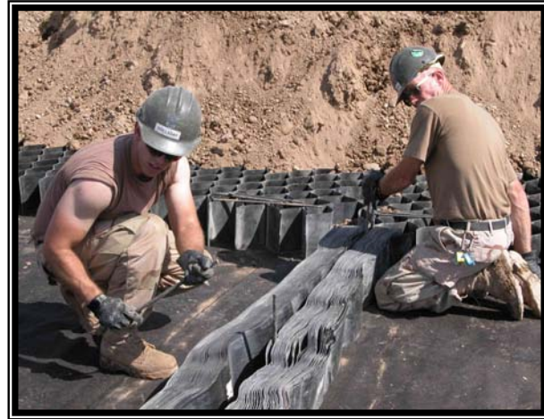
Assembling geo-textile.
