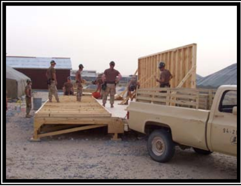
Seabees construct a SWA Hut.
