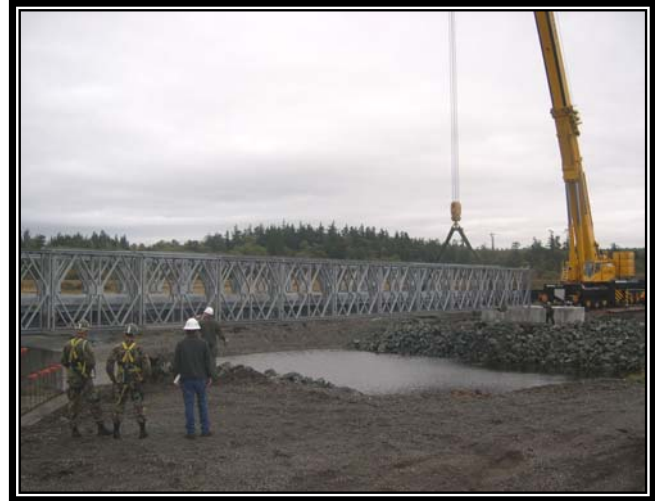
Launching of Mabey-Johnson Bridge.
