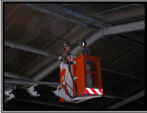
Seabees install high bay lighting.
