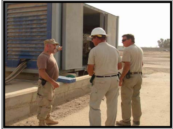
CE1 Jermyn arranges for delivery of repair parts for generators.
