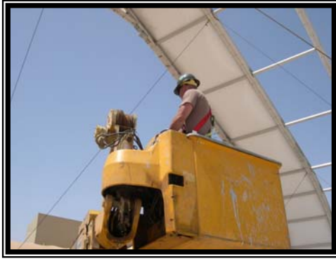
Seabees shown installing the fabric shell.
