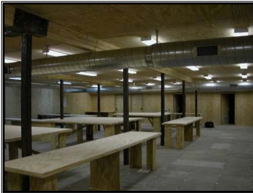
Fabrication and installation of desks and map tables.
