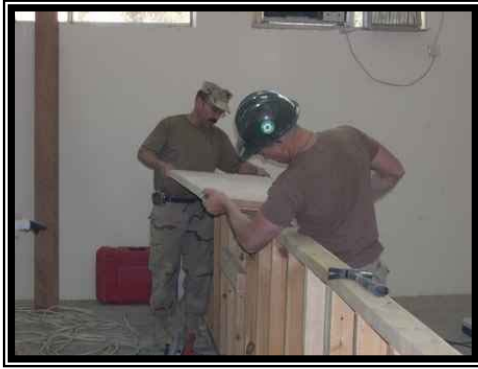
Seabees construct a counter for the issuing facility.
