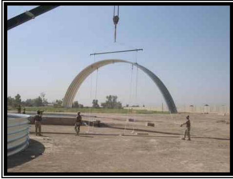
Seabees erecting steel.
