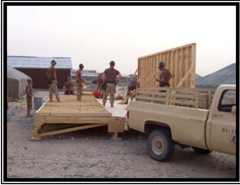
Seabees construct a SWA Hut.
