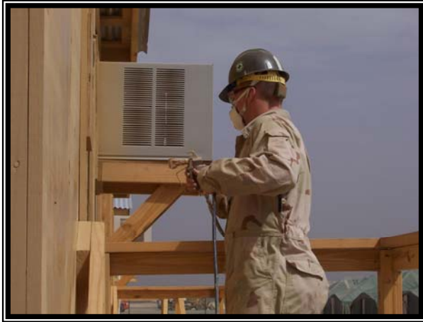
A Seabee performs building maintenance.
