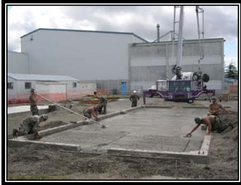
Placing the concrete slab.
