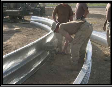
Seabees pressing steel panels.
