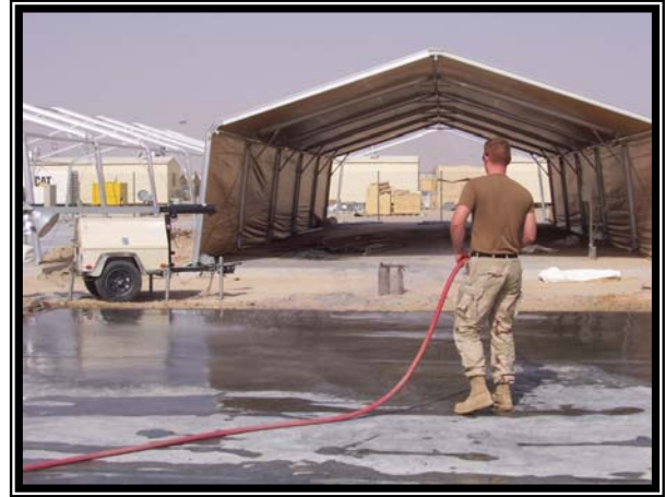
A Seabee finishes the concrete slab.
