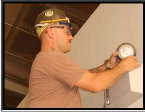
CE1 Jermyn installs emergency lighting.
