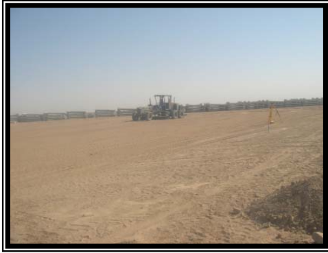
Site work in progress.
