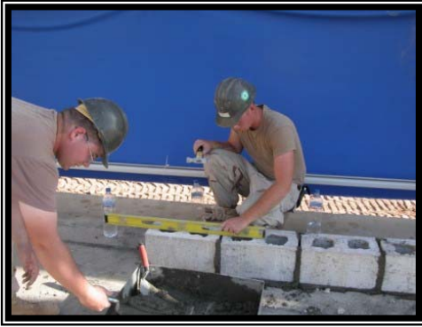
Seabees laying CMU block.
