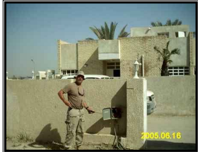
CM1 Wold tests electrical wiring.
