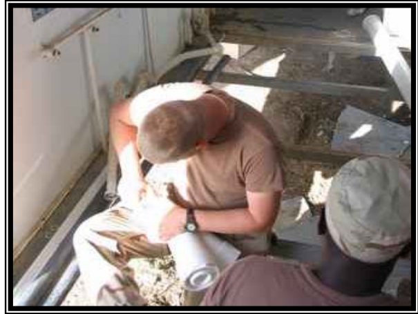
Rehabbing a shower trailer.
