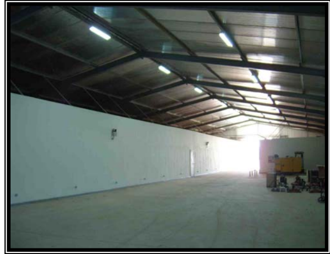
Completed Shop Spaces.
