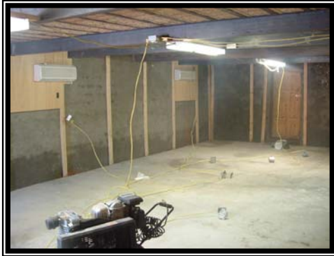
Demolition of office and berthing area.
