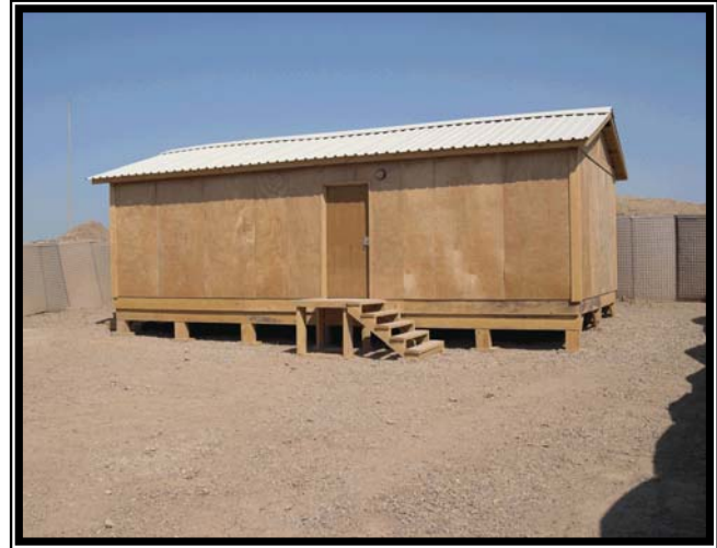
Completed SWA hut.
