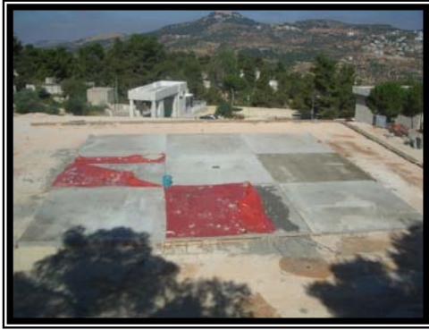
Initial concrete placement.
