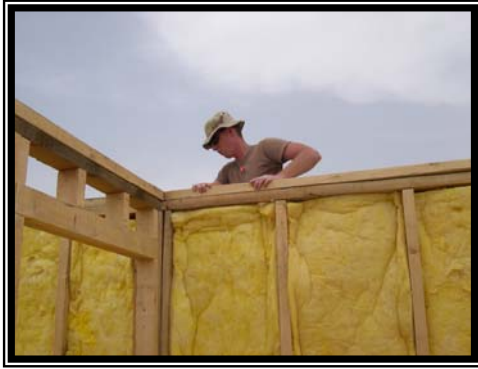
Seabees shown framing SWA hut.
