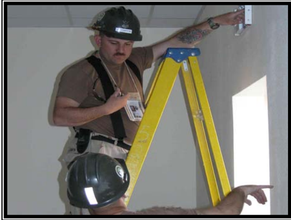
Seabees make electrical repairs.
