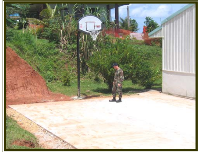
Finished basketball court.
