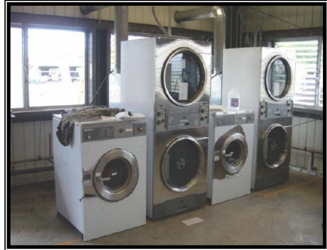
Completed appliance installation.
