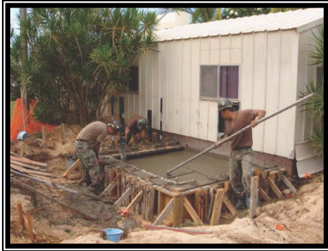
Placing concrete pad.
