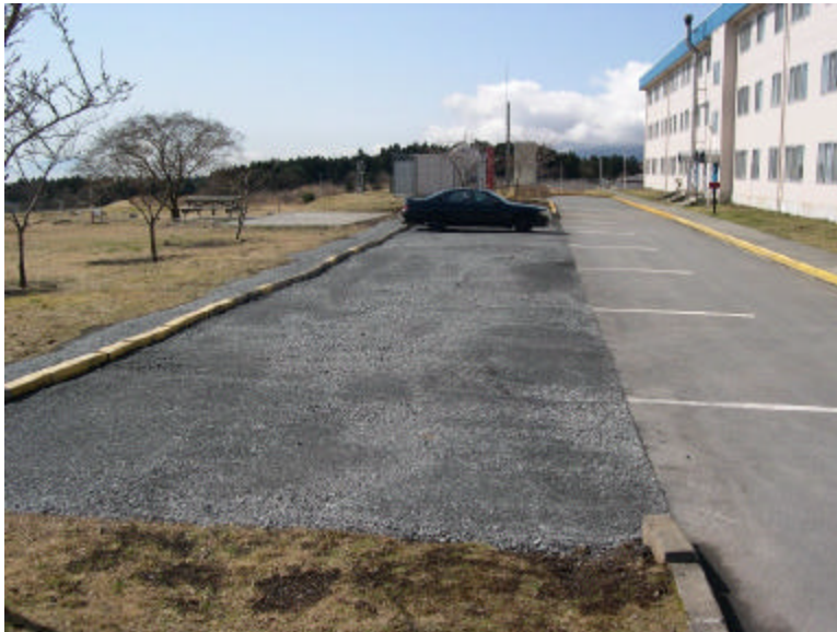
Parking lot expansion at Bldg. 450
