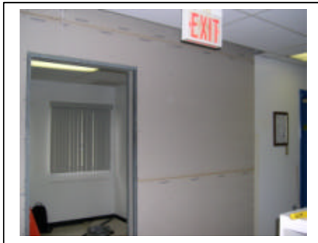
Placement of the drywall.
