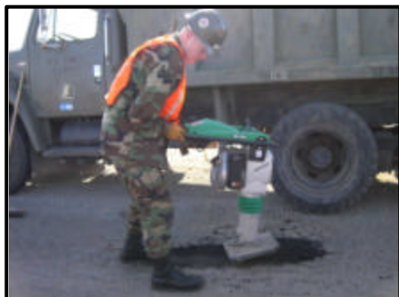
Cold Patch Ridge Road Potholes.
