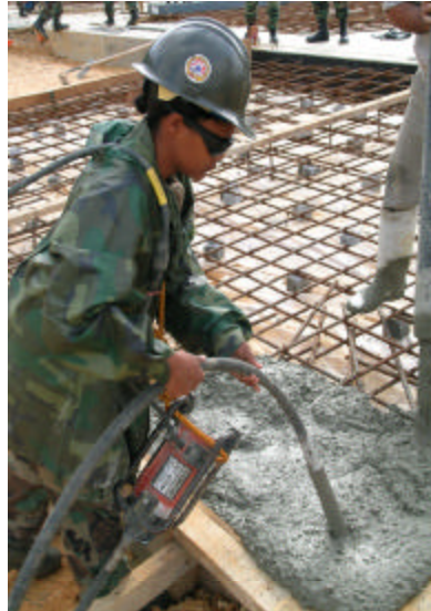
Wearing eye protection during concrete placement at SBU Project.
