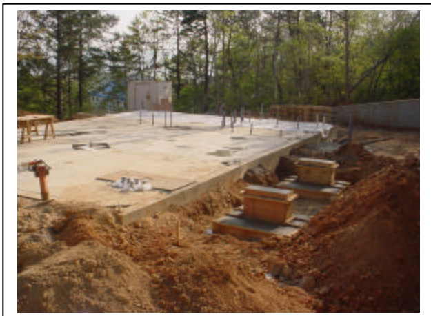
Pad prior to erection of PEB
