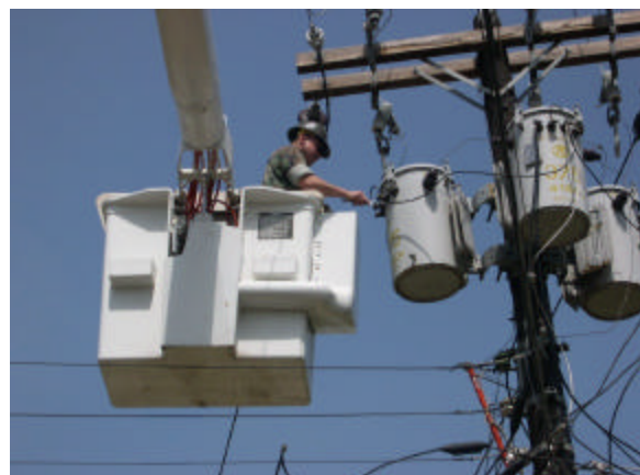
Installing new transformer bank.
