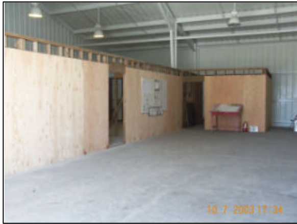
Exterior walls, sheathed in A/C grade plywood for the new NMCB Office Spaces.
