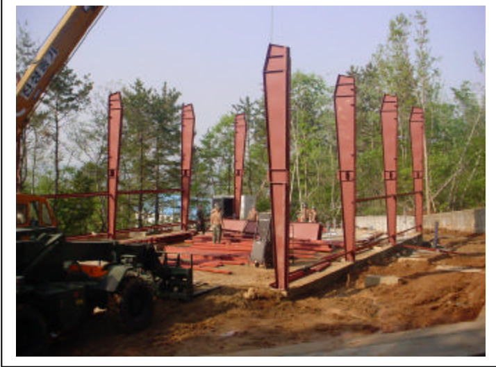
Above: Start of PEB Erection
