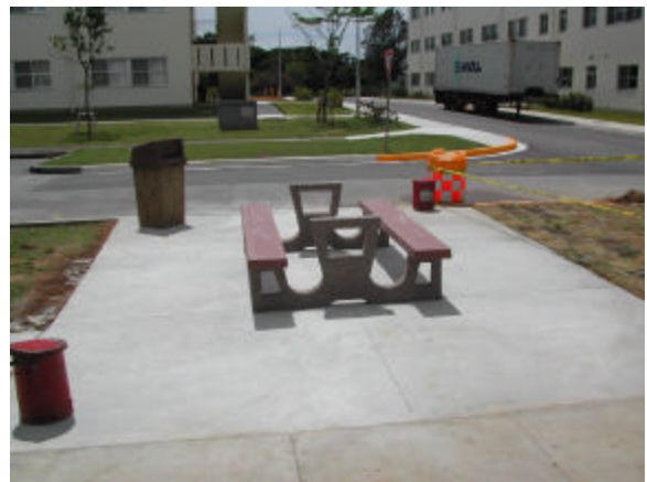
Construct Concrete Pad / Lay Sod & Install Picnic Tables, Bldg 7216
