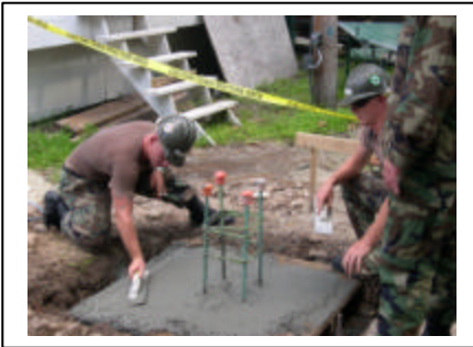
Above, the placement of the concrete footers, Right, the Finished Pavilion.
