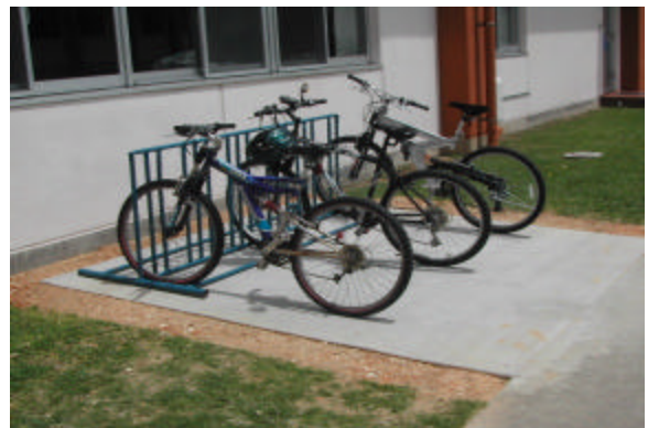
Construct Bike Rack Concrete Pad Outside Bravo & Charlie Company Spaces, Bldg 6310
