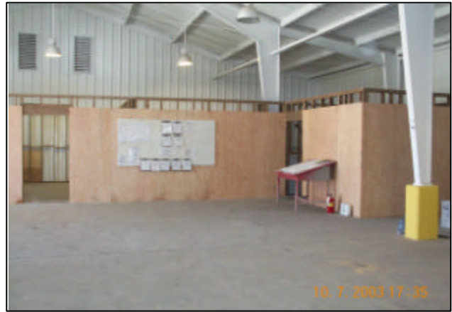
Exterior walls, sheathed in A/C grade plywood for the new NMCB Office Spaces.
