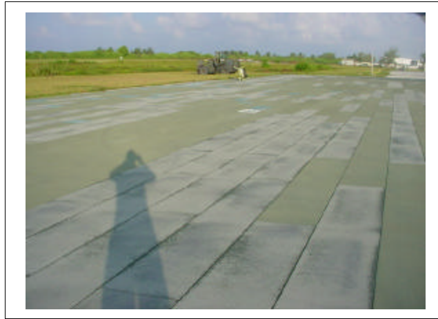
AM2 Matting Removal
