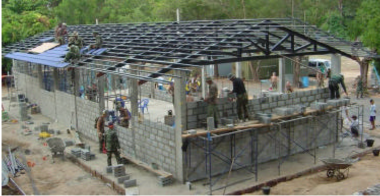
Above left, Seabees and Thais work on CMU walls and roof tile. Above right, the nearly complete building is shown.
