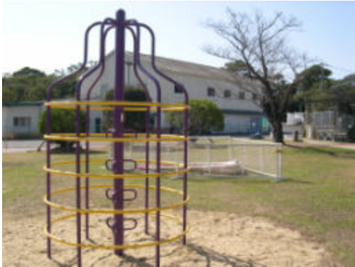
Install Playground Equipment, Nimitz Park
