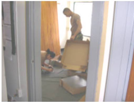
Office Suite Renovation
