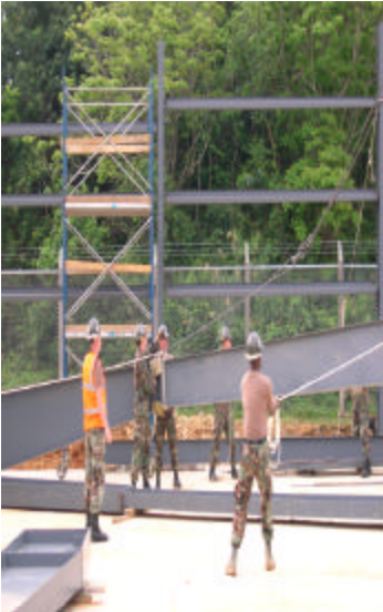
Placing structural steel in place at the Bas Barn Project.
