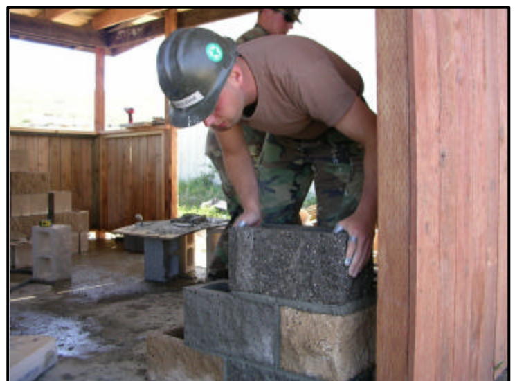
Construct Gazebo & Grill for Det Recreation Area.
