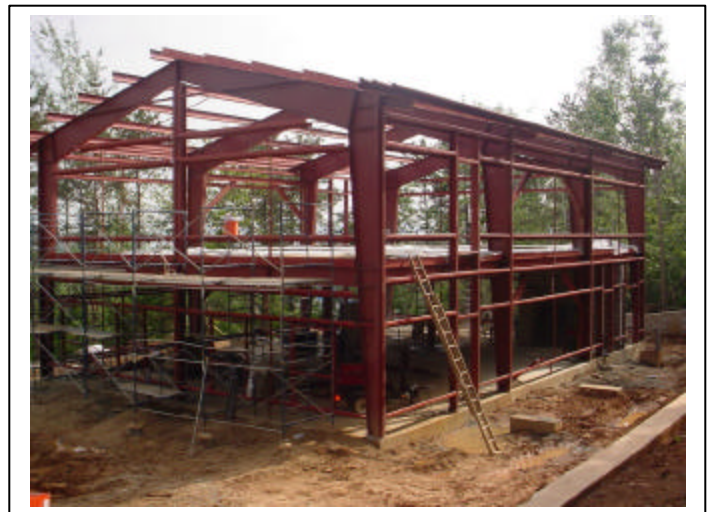
PEB with second floor decking installed
