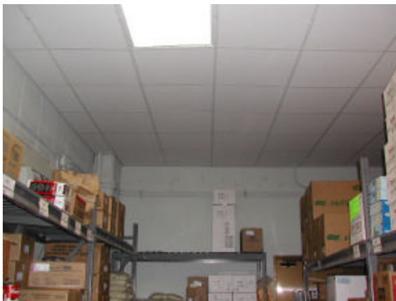
Install Drop Ceiling in Galley Dry Storage Room, Bldg 7205
