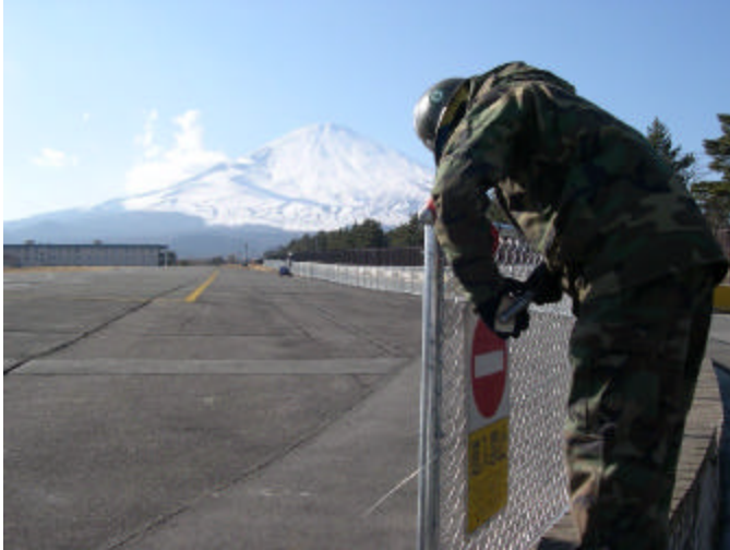
Putting the finishing touches on the flightline fence
