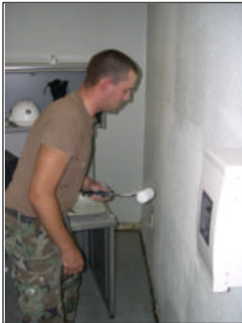
Painting interior of det spaces
