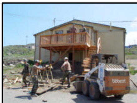
Construct Deck OIC/AOIC House.
