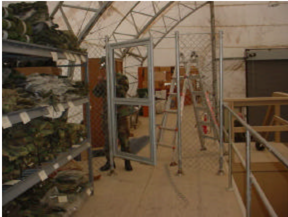
Installing security gate to military gear issue storage area.
