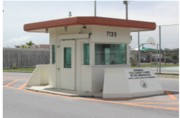
Repaint Guard Shack, Bldg 7139
