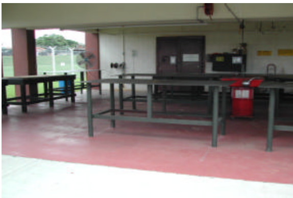
Repaint Armory Deck, Bldg 5001
