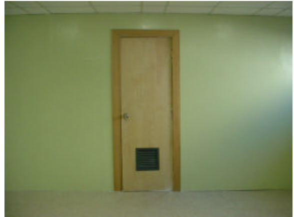
Completed MWR equipment gear issue room in Recreation Facility.
