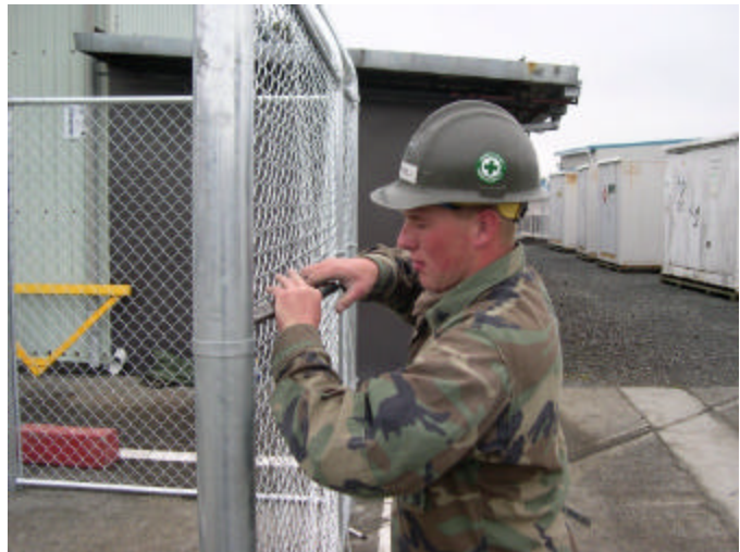
Tightening tension wire on the HAZWASTE building security fence
