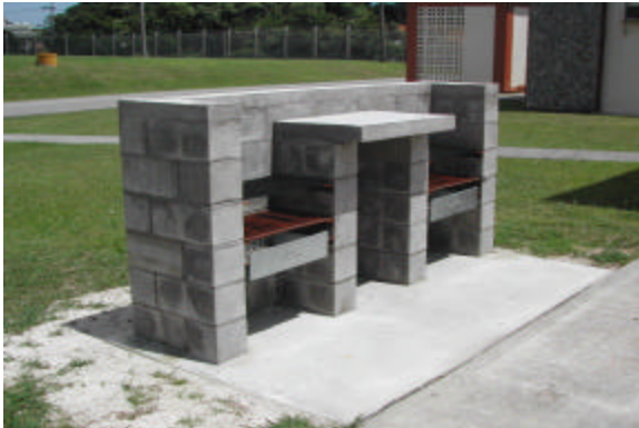
Construct BBQ Pits at Various Locations in Camp Shields
