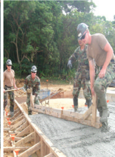
Placing concrete at SBU Facility
