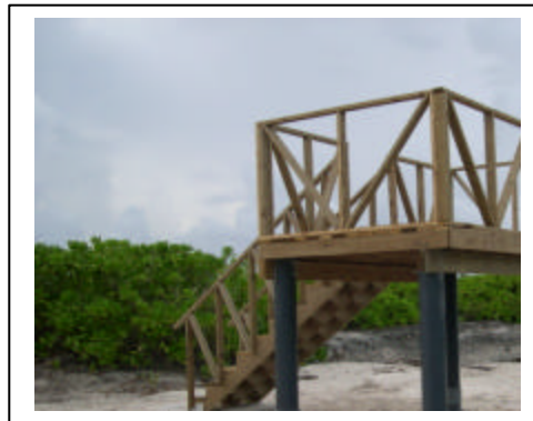
Completed Turtle Cove Platform
