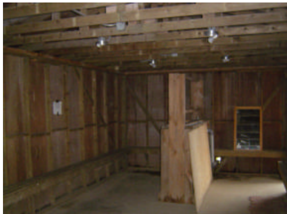
Shower Facility before renovation.
