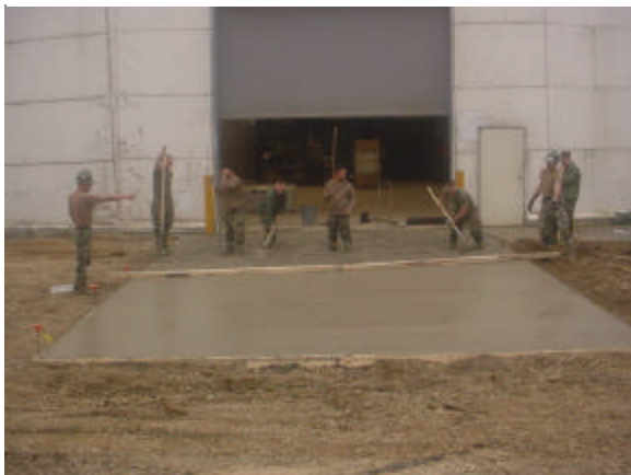
Placing concrete for parking ramp for mechanic shop.
