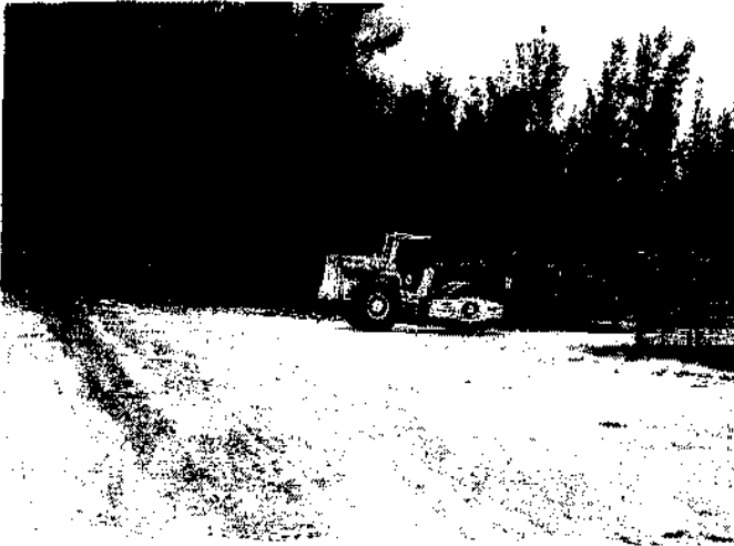
EOs of NMCB 5 repairing the entrance to Seabee compound
