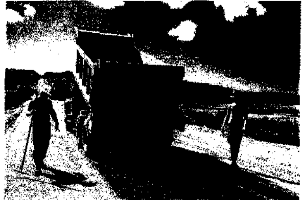
BELOW: Applying gravel on top of the emulsion compound on road surface.
