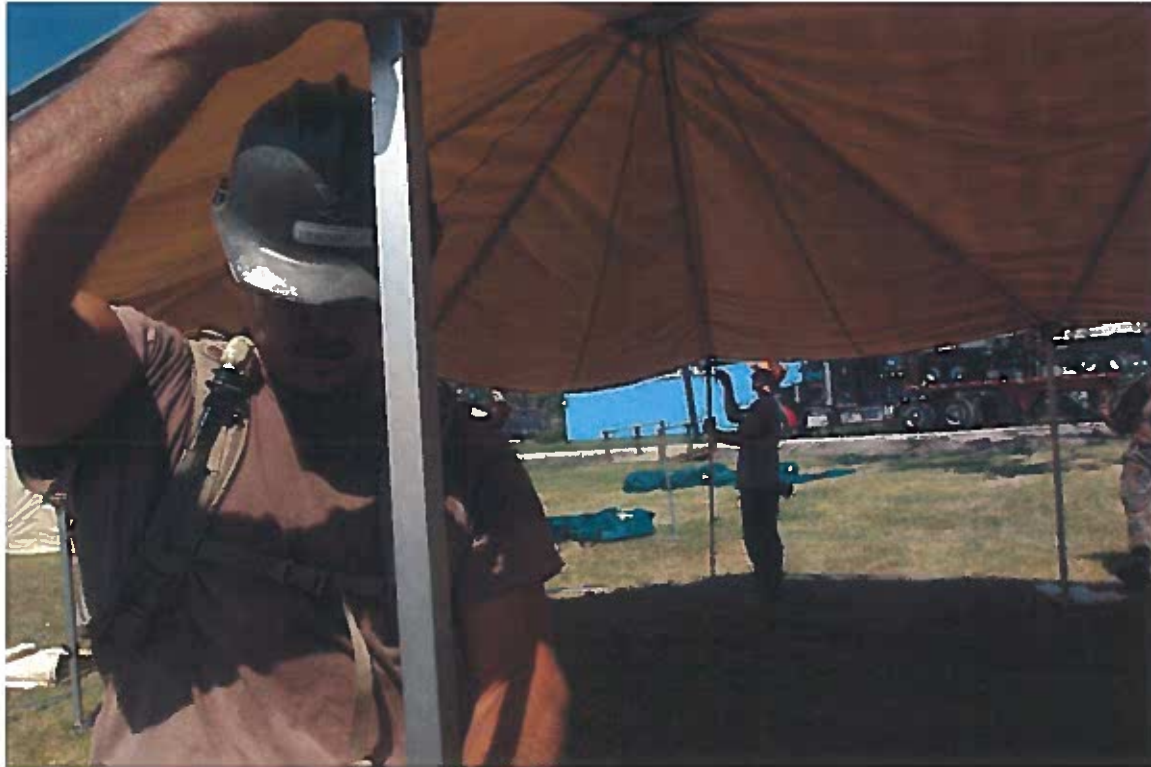
050928-N-2653P-027 Plaquemines Parish (Sept 28, 2005) - Construction Electrician 3rd Class German Carillo assigned to Naval Mobile Construction Battalion Four Zero (NMCB-40) helps assemble a tent, which is part of a larger 500 person Federal Emergency management Agency (FEMA) tent city. The camp will allow FEMA officials to move from Belle Chasse Primary School so school officials can expedite getting the school open for students. The Navy's involvement in the Hurricane Katrina humanitarian assistance operations are led by the Federal Emergency management Agency (FEMA), in conjunction with the Department of Defense. U.S. Navy photo by Journalist 1st Class James Pinsky (RELEASED)
