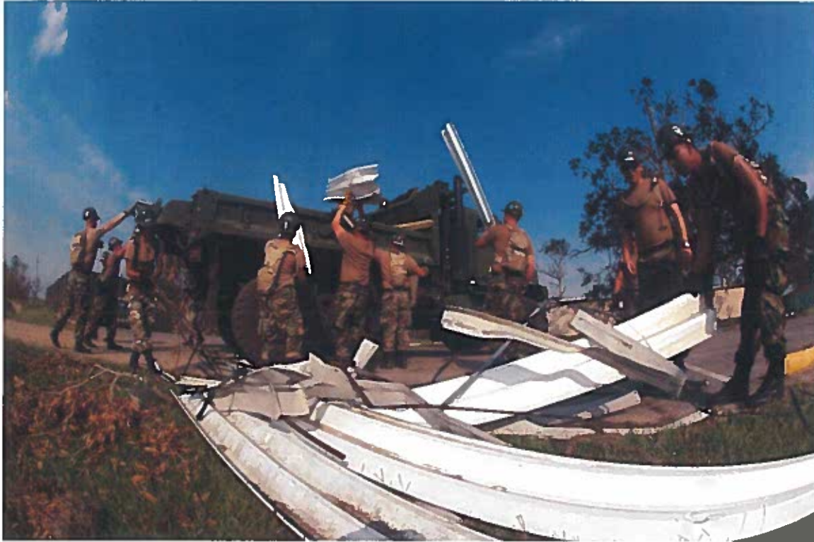
050909-N-5526M-004 New Orleans (Sept. 09, 2005) - U.S. Navy Seabee's assigned to Naval Mobile Construction Battalion Four Zero (NMCB-40) load metal Debris left behind from hurricane Katrina at Naval Air Station Joint Reserve Base New Orleans. U.S. Navy photo by Photographer's Mate 1st Class Robert McRill (RELEASED)
