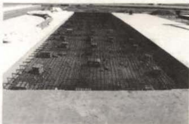
Taxiway apron project, Sigonella
