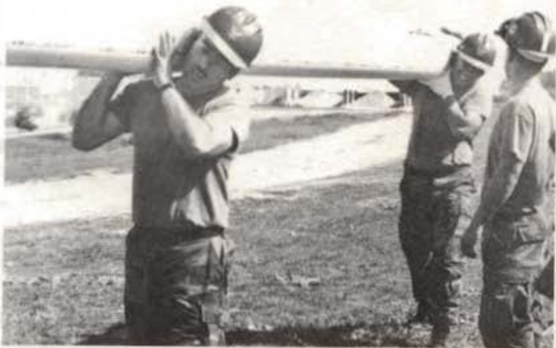
Waterline project, Rota
