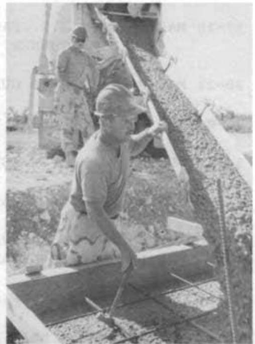
(Top left) The Alfa Company asphalt crew takes a rest at the Fleet Hospital Hardstand. (Left) Crew members pump concrete into footer forms at the Inarajan School. (Above) Concrete is placed in footers for the DTS Pre-Engineered building.
