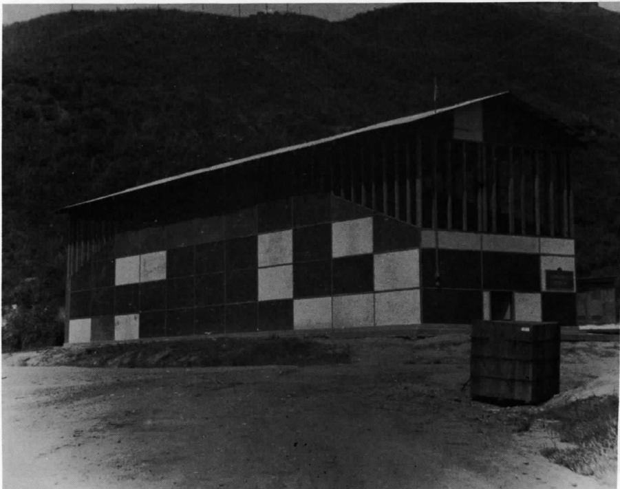
Salvaged material was used in the reconstruction of the Handball courts at Freedom Hill
