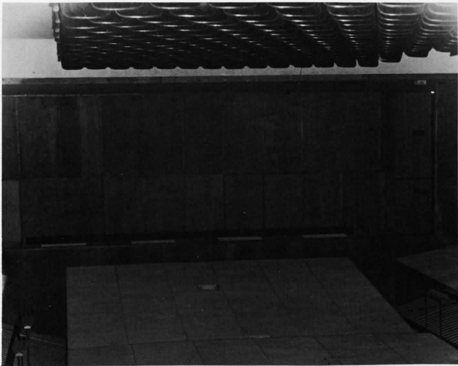
Acoustical panels were hung inside the new theater to develop desired acoustics
