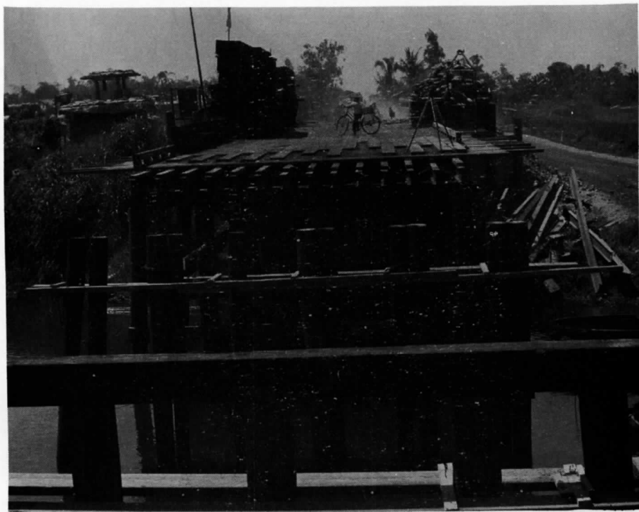
Than Quit Bridge-New piles driven, ready to receive pile cap and stringers
