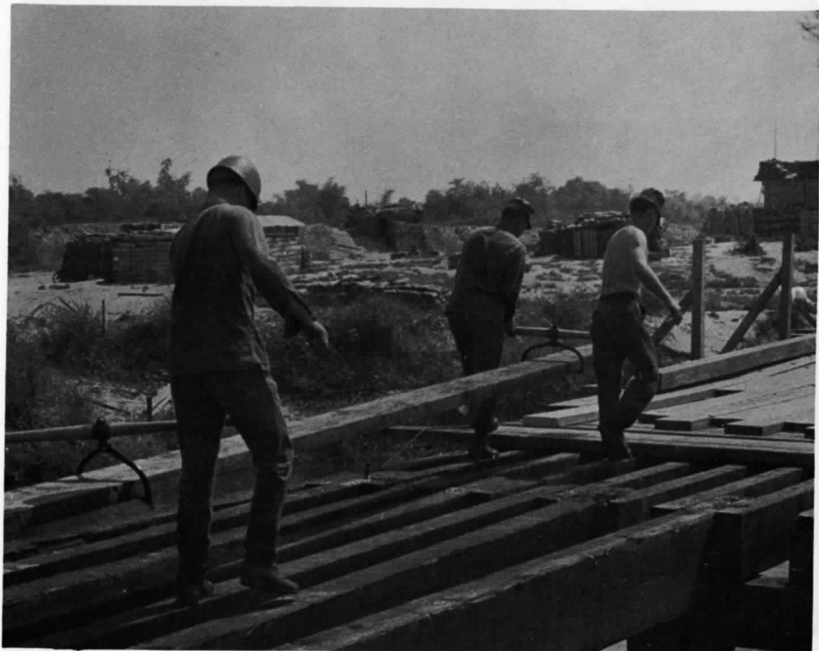
Cooper Bridge-Replacing bridge decking
