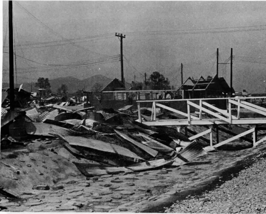
3rd MP berthing area after ASP-1 explosion
