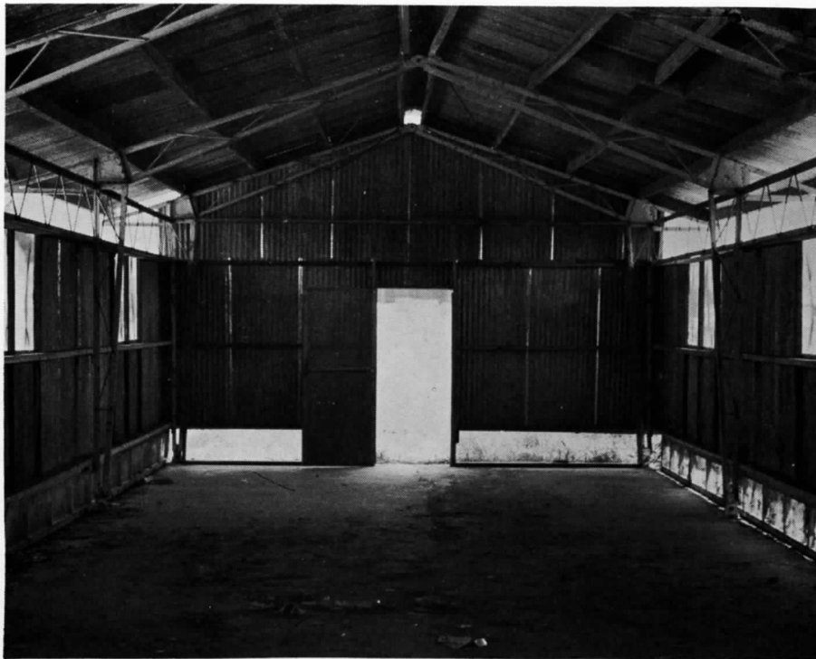
Cholon Building-A European pre-engineered building erected for Regional Forces
