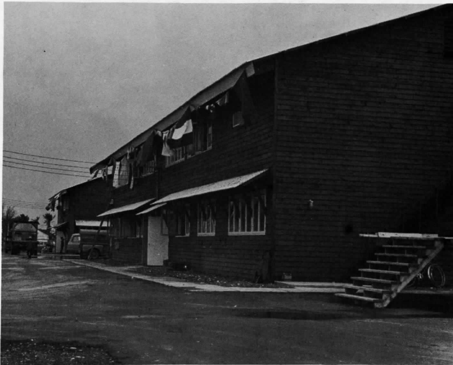
The customer began preparation for a dedication ceremony as the SEABEES put the finishing touches on the interior
