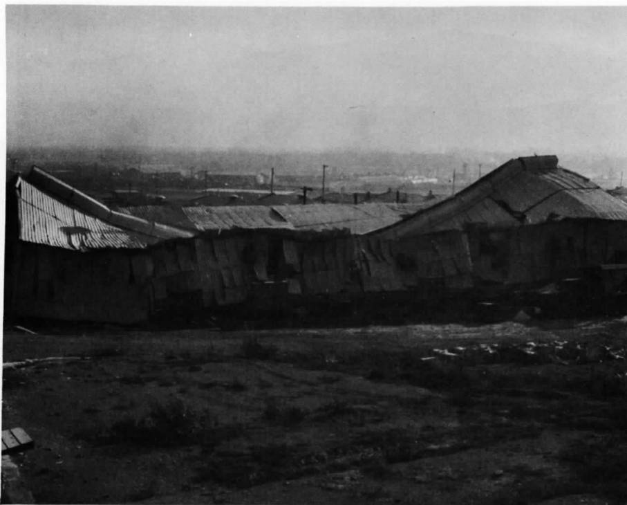
Freedom Hill theater was totally destroyed by ASP-1 explosion of April 1969
