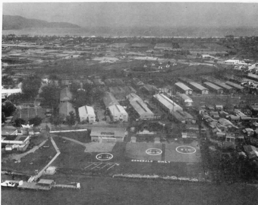
III MAF Headquarters, Camp Horn-Damage from ARVN ASP explosion was repaired by MCB FOUR
