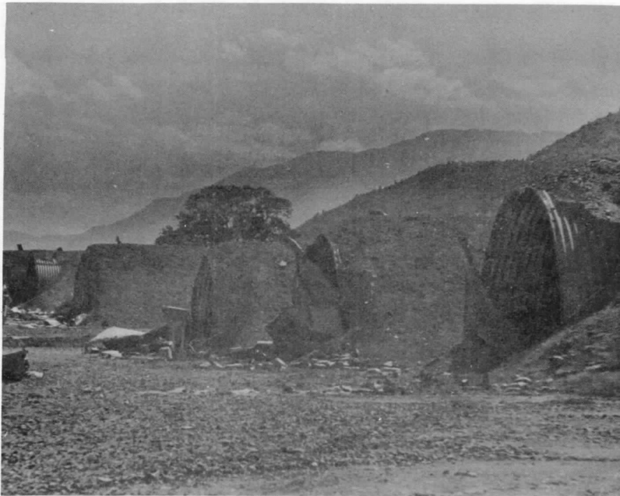
Damaged ammo storage magazines after the ASP-1 explosion
