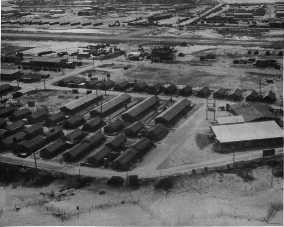
MAG-16 Expansion-Four new BOQ buildings were completed in only 3 weeks
