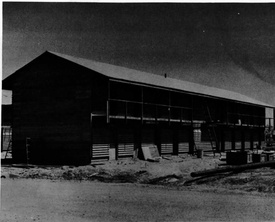
20'X108' two-story BOQ built for the U.S. Army Support Command, Danang
