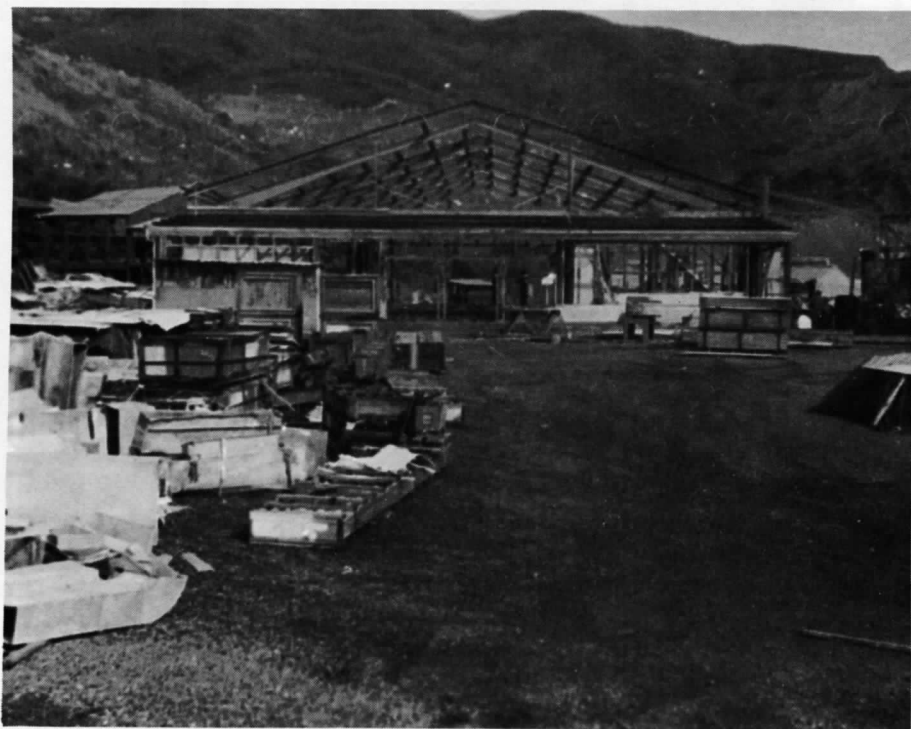
Framework is complete on the new Freedom Hill theater
