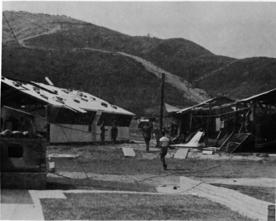
The 3rd MP Administration building (left) was established as MCB FOUR Control Center for reconstruction
