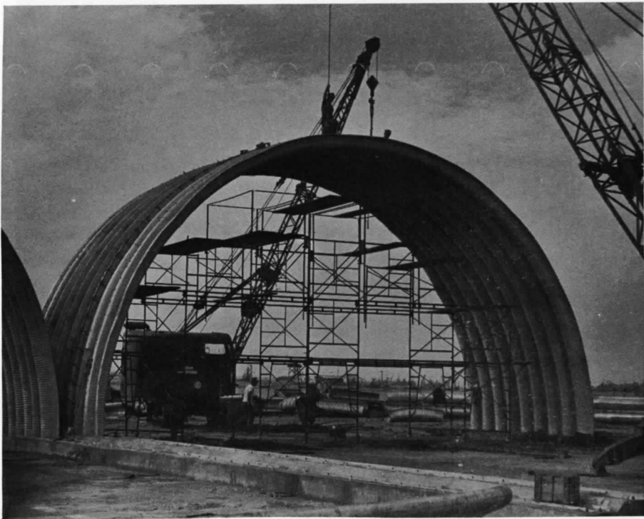
MAG-16 Aircraft Shelters-Arched ribs of "Wonder Buildings" are lowered into place
