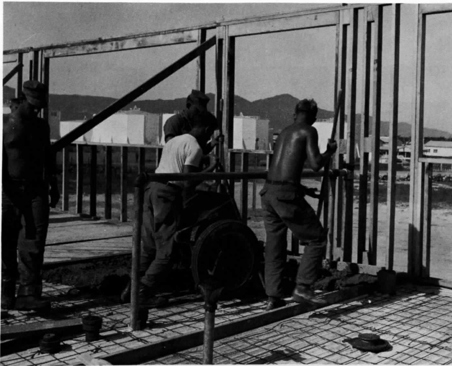
Pouring second deck in IRD building, Danang
