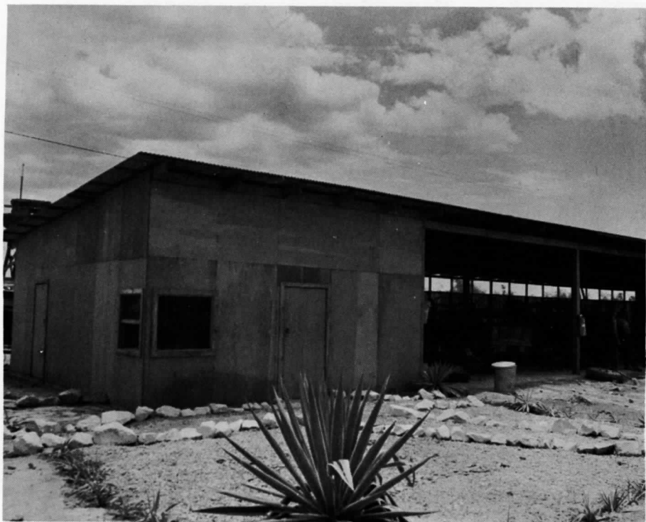
Vehicle maintenance garage - CAG II
