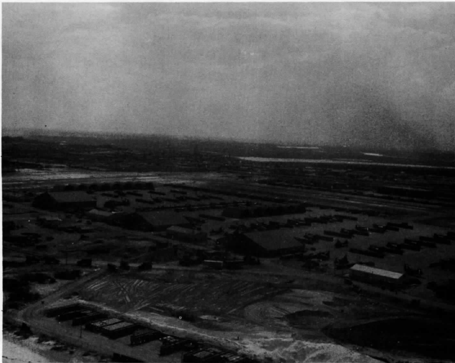
MAG-16 Aircraft Shelters-MCB FOUR's concrete batch at lower center was established to batch concrete for the "Wonder Buildings"
