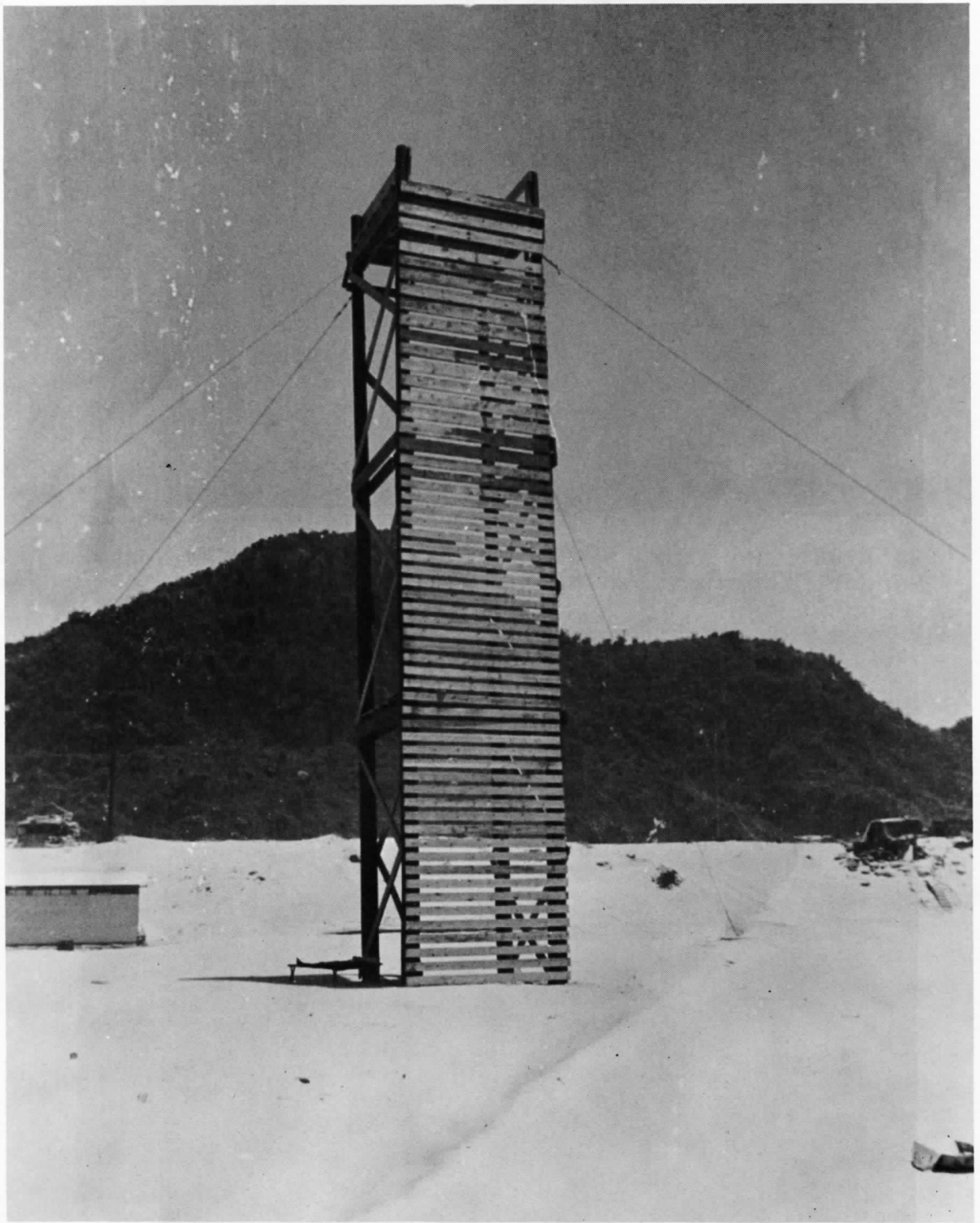
This 60 ft rappelling tower at Marble Mountain was built for the Special Forces to maintain their climbing proficiency
