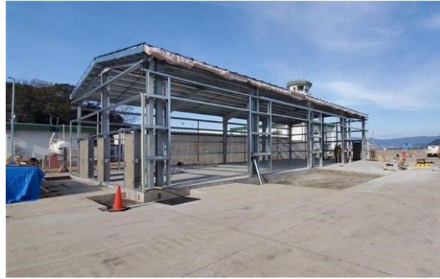
40 ft x 80 ft Storage PEB
