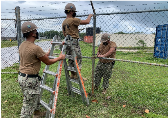
Crew securing new chain link fencing to posts at fuel farm.
