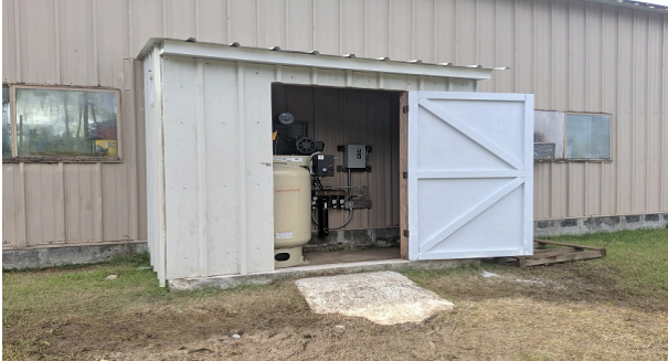
Renovated Maintenance Shed.
