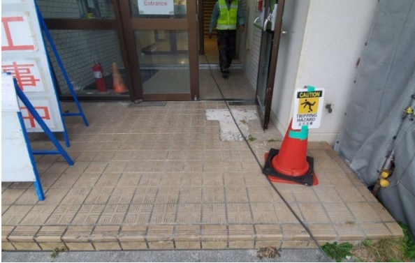
Before Project Start
