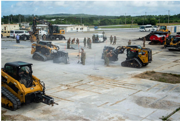
Seabees and Airman from 18 th CES conduct a joint rapid ADR exercise on Kadena Air Base in Okinawa, JP.
