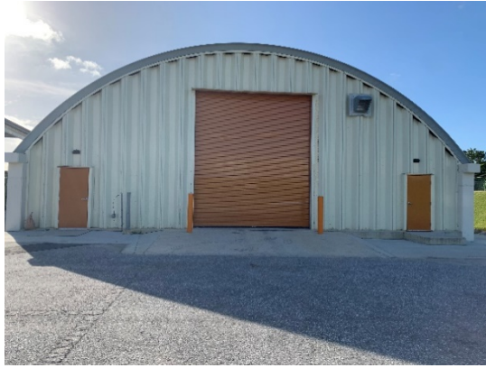
K-Span III End View (Facing West)
