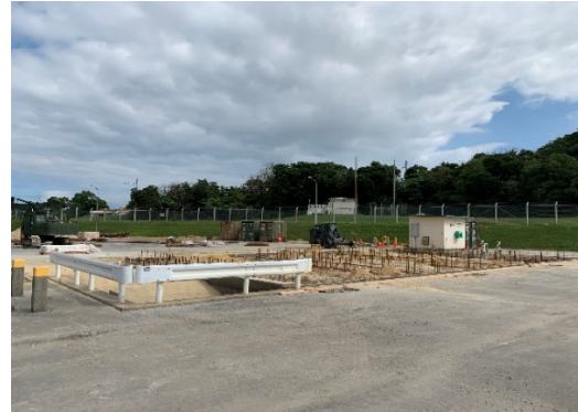
Preparation for Footer Placement
