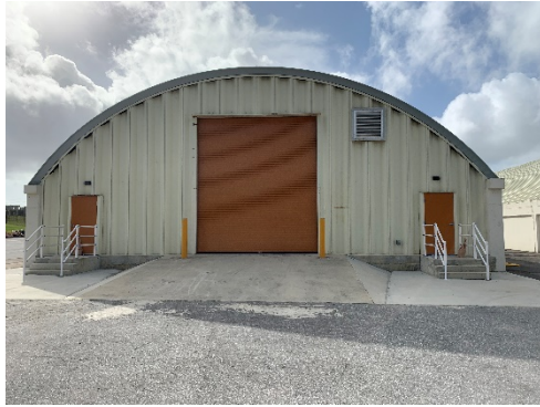
K-Span II End View (Facing South)
