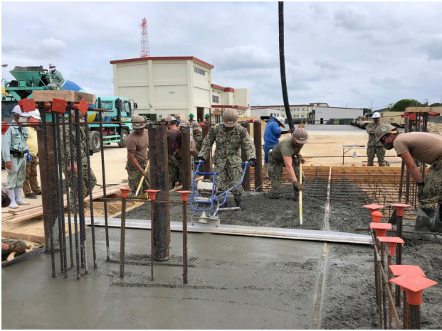
Placement of Pad 1
