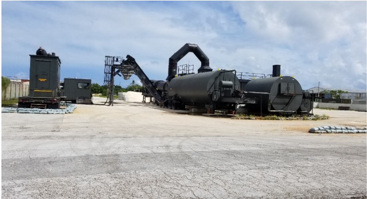
Detail Guam Seabees conduct maintenance on the Asphalt Batch Plant
