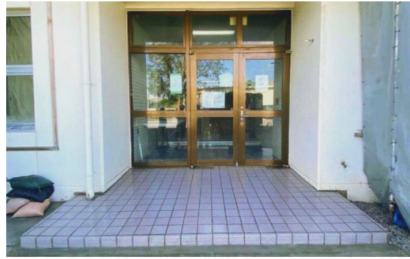
After Project Completion
