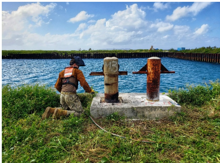
Detail Tinian Seabees complete demo of bollards in support of Tinian Harbor Project
