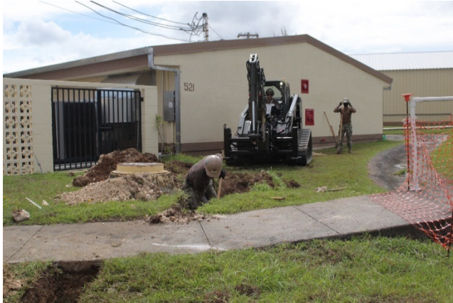
Seabees dig trench for future fiber optics ISO USO.
