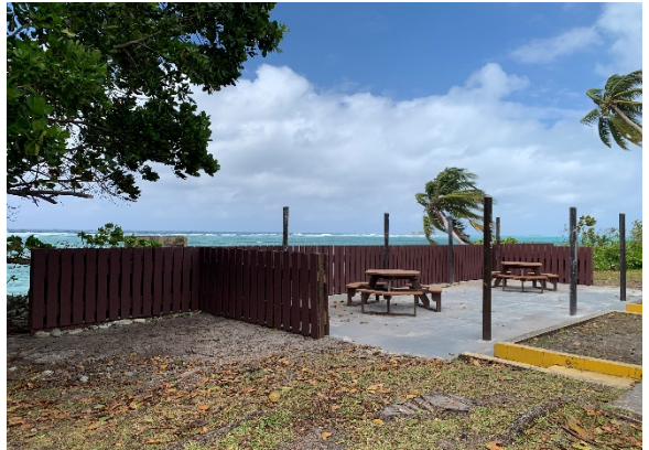
Completed MWR Liberty Center Perimeter Fence.
