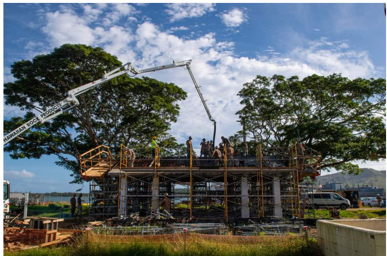
GM18-879: Seabees conduct overhead concrete placement.
