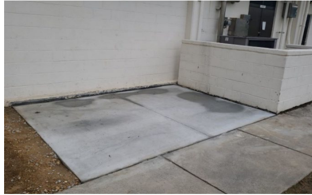
After Project Completion
