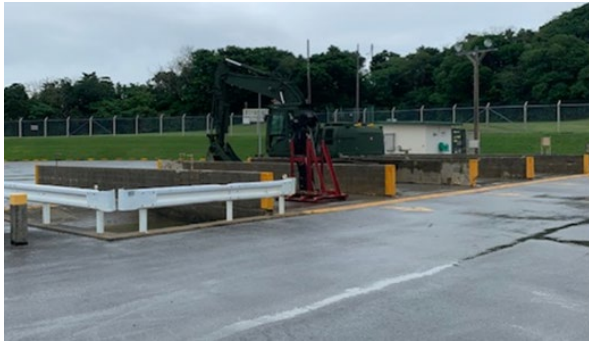
Before Project Start
