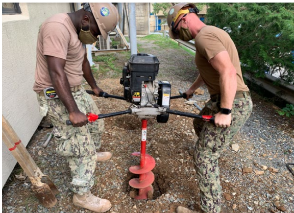
Using an auger to create holes for workout station.
