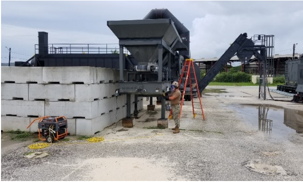
Corrosive preventative maintenance.
