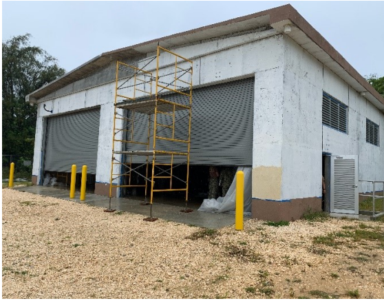
Project at Turnover
