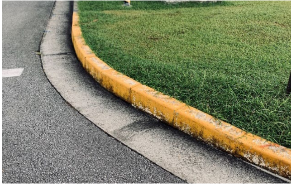
Before Project Start
