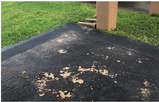
CDC playground for newly installed drains.
