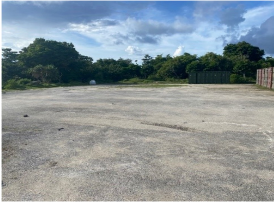
Project at Turnover
