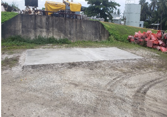
Completed concrete pad for baler machine.
