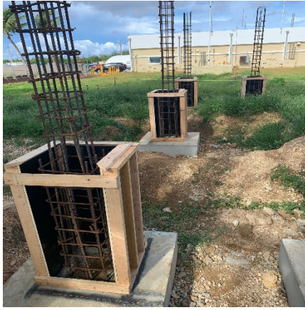
Project at Turnover
