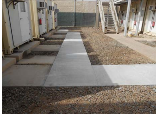
Completed Containerized Living Unit sidewalks
