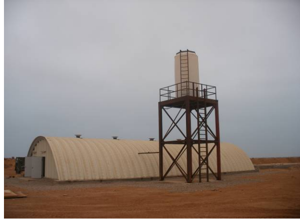
Completed K-Span with water tank
