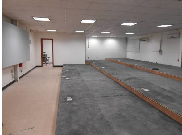
Completed SOCCE JOC floor
