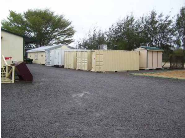
Gravel spread in lay down area
