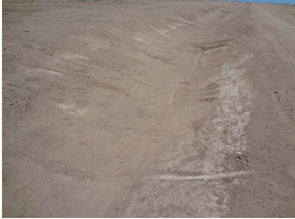
V-Ditch facing the Gulf of Aden
