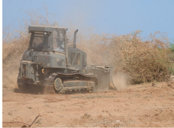
Clearing and grubbing
