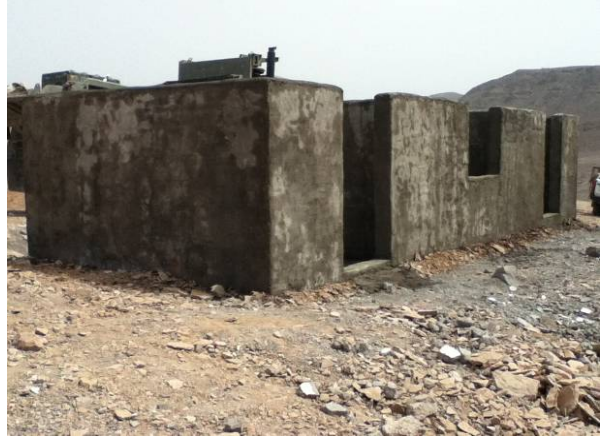
Completed shoot house
