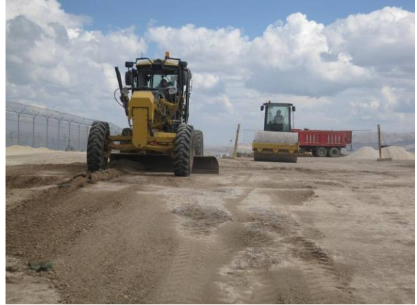
Grading temporary DFAC site
