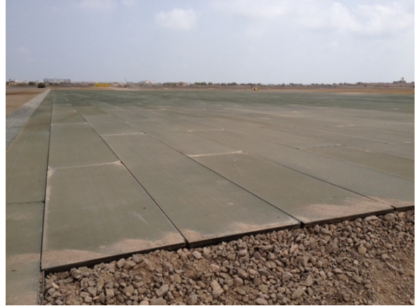
Aircraft parking apron extension
