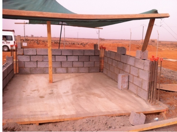
Cooking structure CMU
