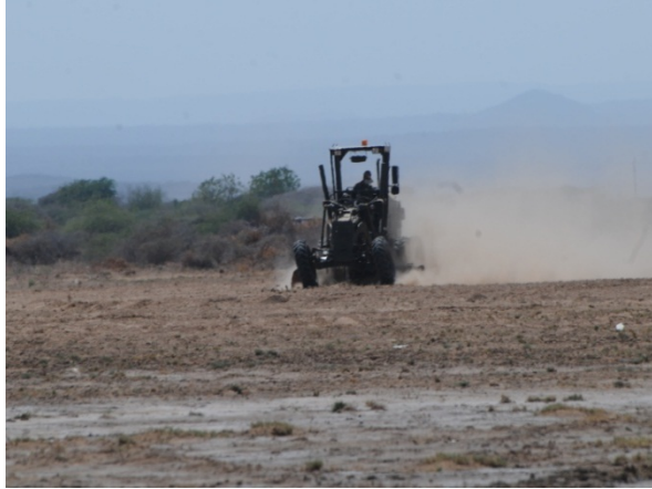
Grading the drop zone
