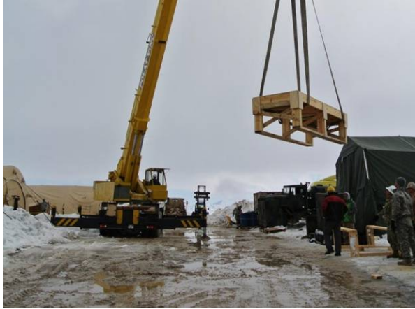
Lowering generator stand into place
