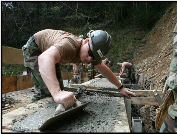
Finishing Concrete Placement for Retaining Wall
