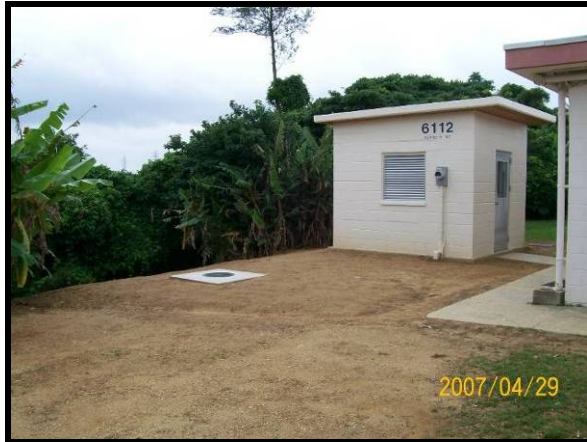
Finish Photo of Exterior
