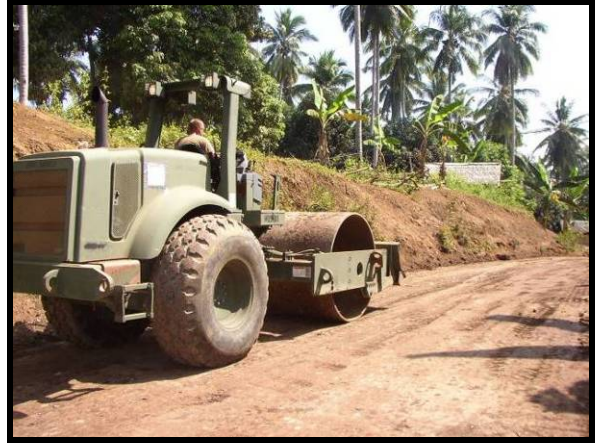
Road Nearing Completion
