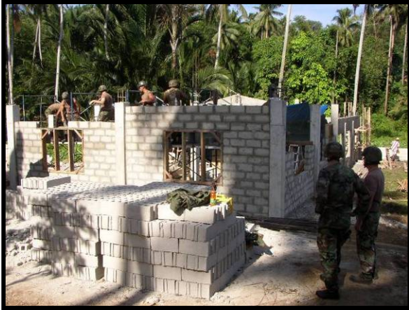
Constructing CMU Walls
