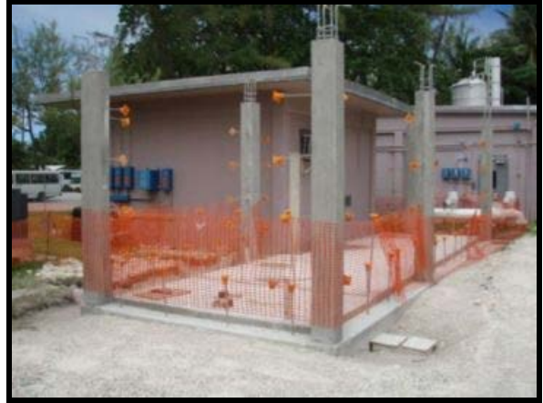
Condition at Turnover
