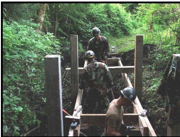
Exercise Trail Bridge Under Construction
