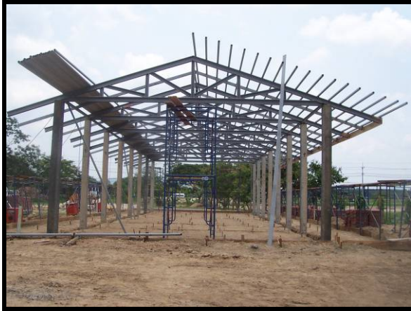
Purlins Placed for Roof
