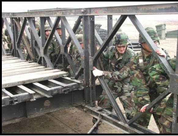
Constructing Bailey Bridge
