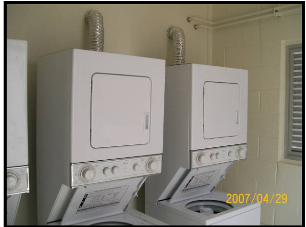
Newly Installed Washer & Dryer Units
