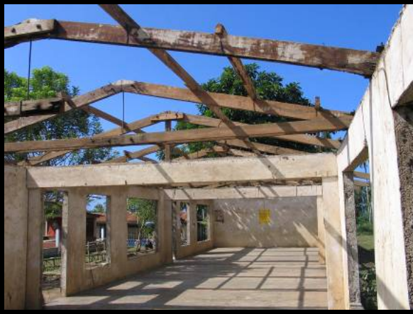
Taglibi School Prior to Construction
