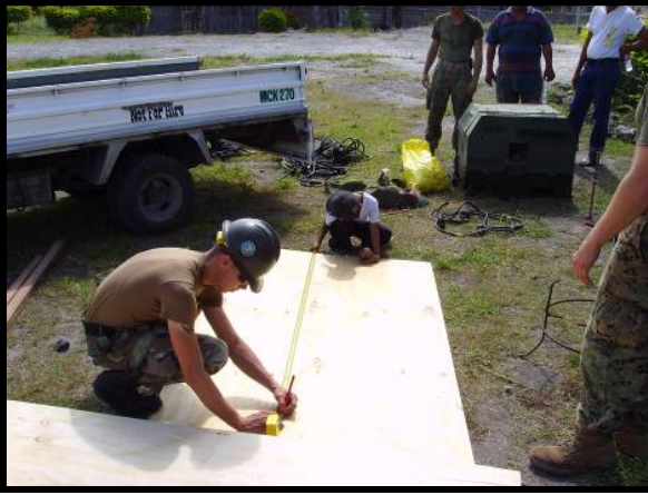
Measuring Plywood for Ceiling Repair
