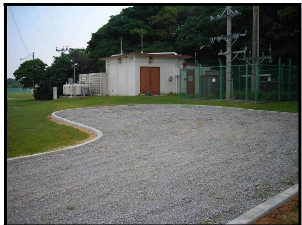
Gravel Access Road to Electrical Substation
