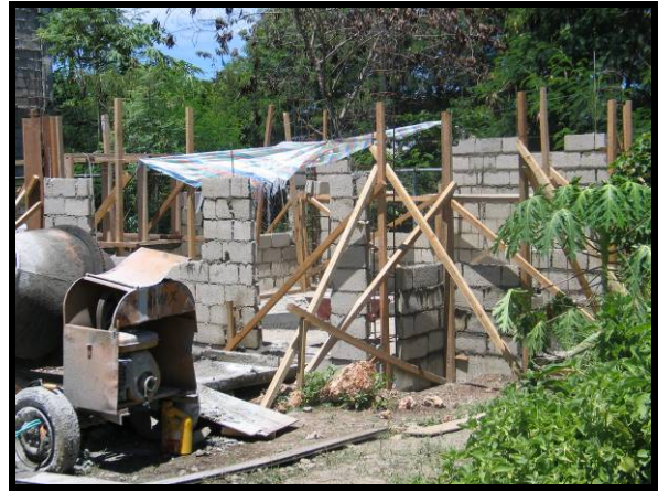
Condition at Turnover
