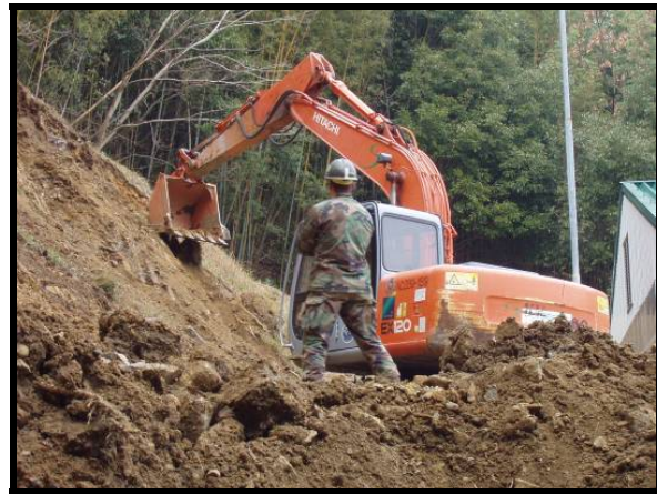
Earthwork at Sasebo's Hario Shima Ordnance Facility
