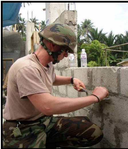
Blockwork at Bato Bato School
