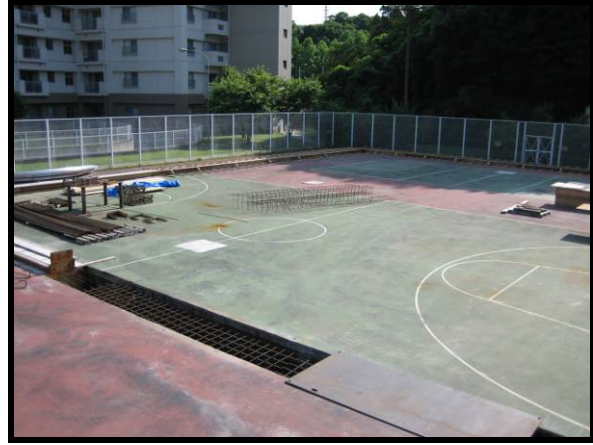
Condition at Turnover
