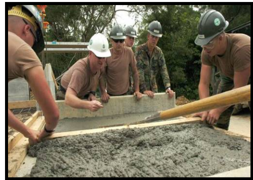
Concrete Placement OJT
