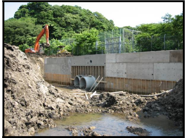
Condition at Turnover
