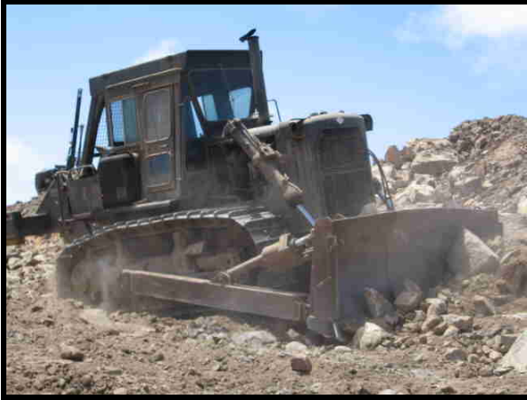
Dozer Ripping Rock at the Mid-island Quarry
