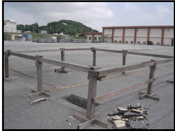
Condition at Turnover
