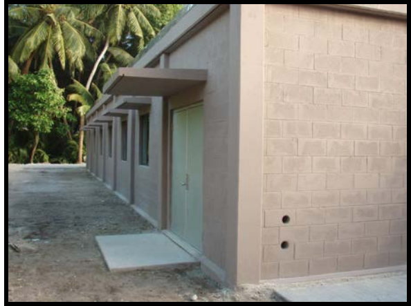
Condition at Turnover
