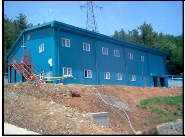
Condition at Turnover
