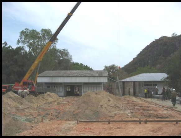
Placing First Column
