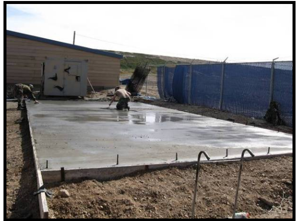
Seabees Completing the Facilities pad at MAROPS
