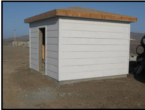
Completed Compressor Shed at MAROPS
