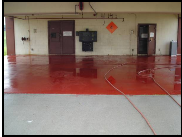
Newly Painted Floor Surface
