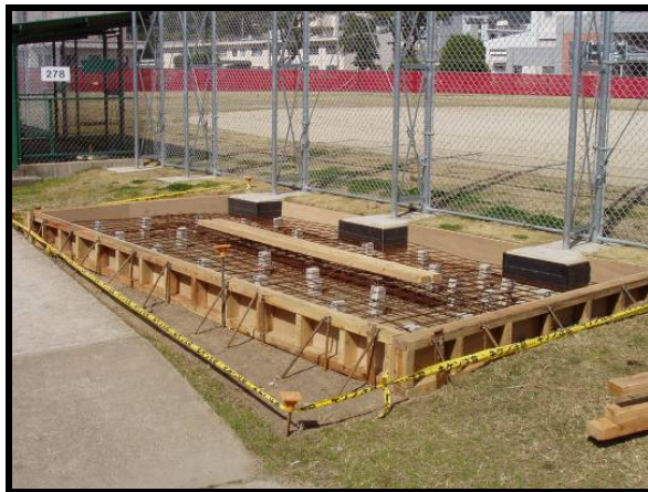
MWR Bleachers in Progress
