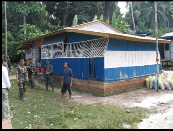
Daycare Prior to Construction
