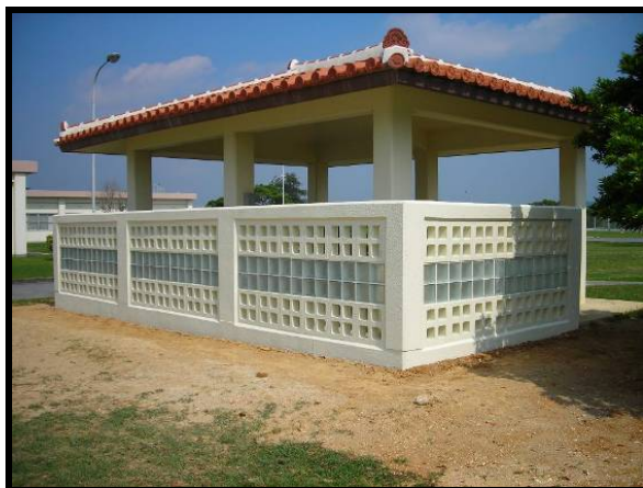
New Pavilion Wall
