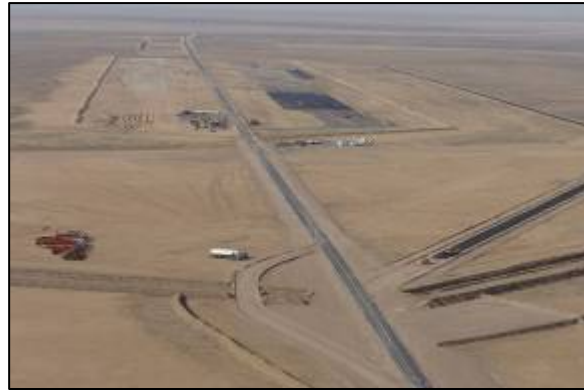
Aerial View of entire K-Crossing project site
