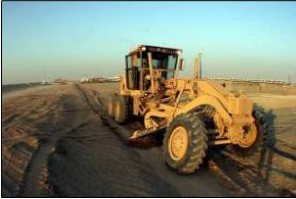
Grading along loading ramps for drainage
