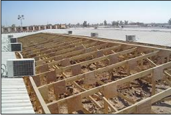
Soil used for blast protection in DFAC roof
