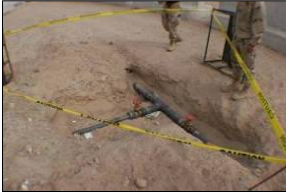
Connecting water lines
