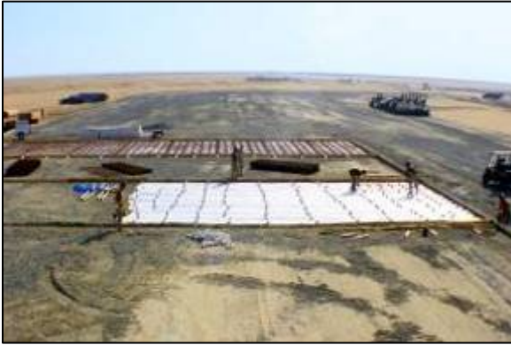
Setting forms for fueling slab
