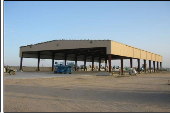
Nearly completed structure
