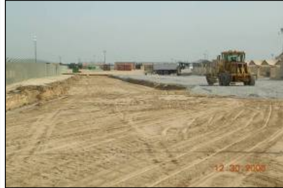
Flat bottom ditch
