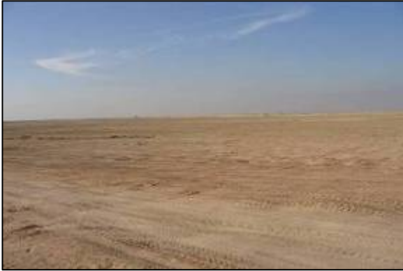
Starting site work
