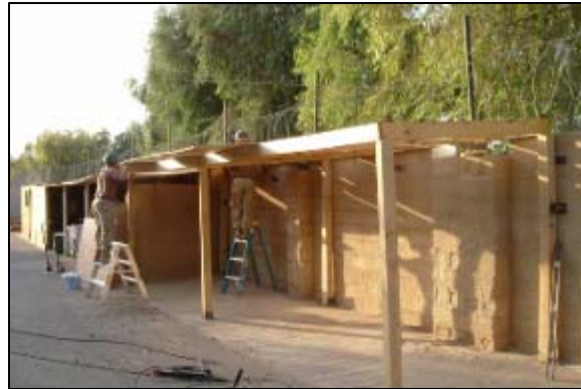
Constructing covered storage for CTR outlet
