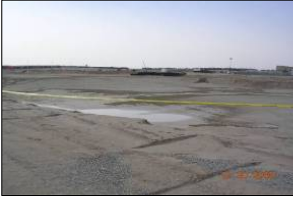
Excavated retention pond
