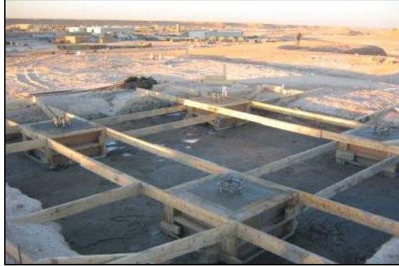
Spot Footings and slab concrete in place
