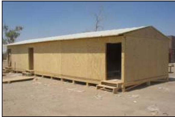
SWA Hut being Constructed for Marines
