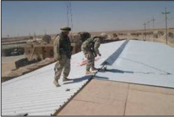
Completing Tin and Ridge Cap
