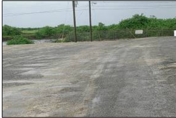
Completed laydown area
