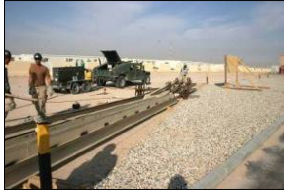
Welding gutters to central support I-Beams
