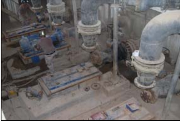
Before - Old pumps/motors removed
