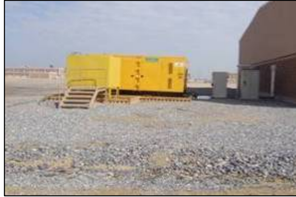
Final grade of pad
