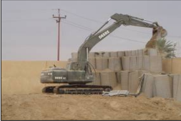
Filling protective HESCOs
