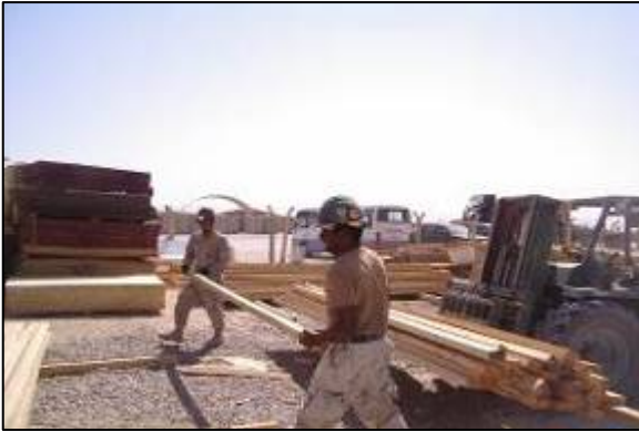
Preparing laydown yard
