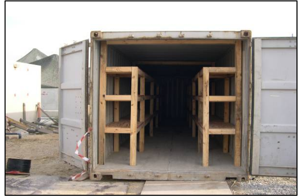
Preparing container for TOA
