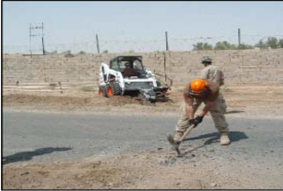
Trenching to install underground feeder cable
