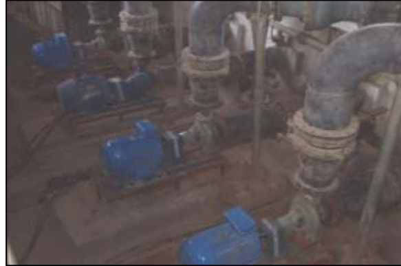
After - Replacement pumps/motors tied in
