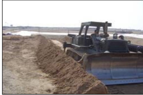
Cutting ditch for culvert
