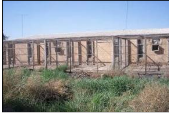
Renovating bldg for use as Seabee berthing
