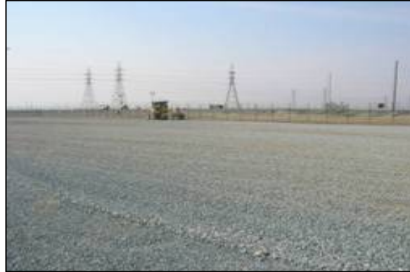
Beginning of grading phase
