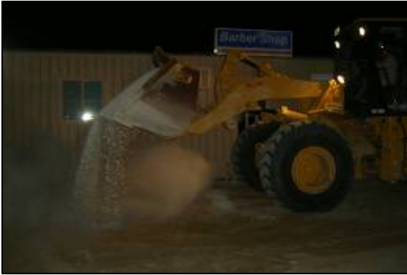
Work was performed at night for pedestrian safety reasons
