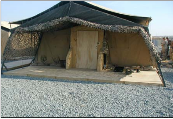
Tent build-out complete
