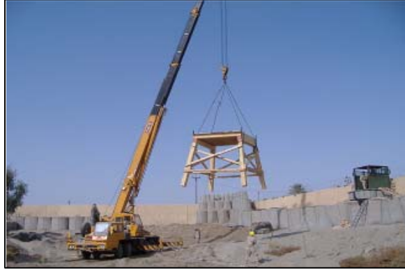
Placing the tower base
