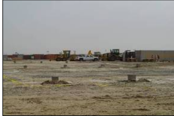
Footers in place
