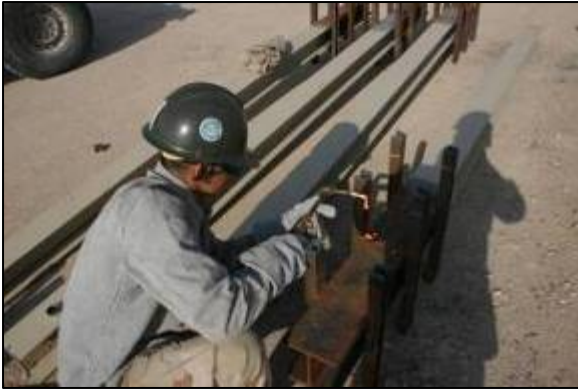
Cutting column extensions to size
