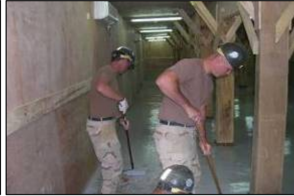
Crew applying floor sealant
