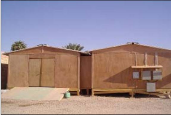
Completed SWA huts
