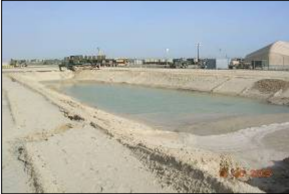
Excavated retention pond
