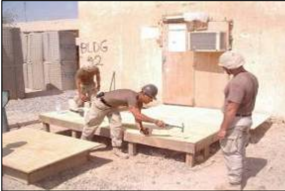
Constructing CPO mess decking
