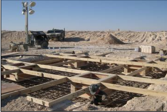
Placing rebar and formwork
