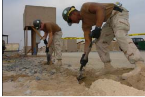
Trenching for new utilities
