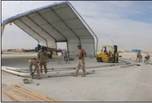
Laying out new structure
