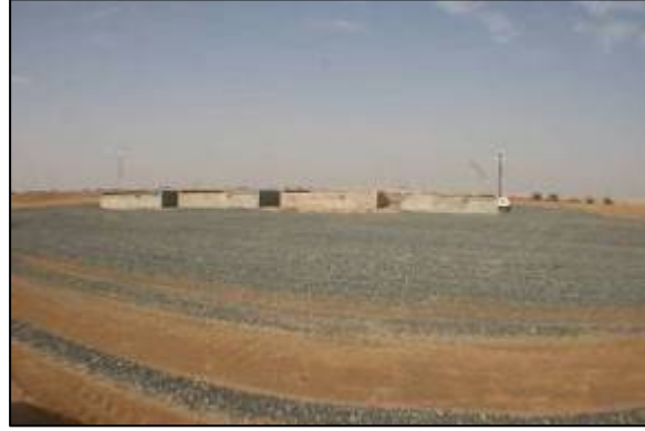
Finished grading and compacting
