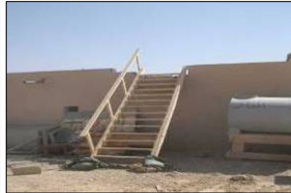
Replacement Ladder Well
