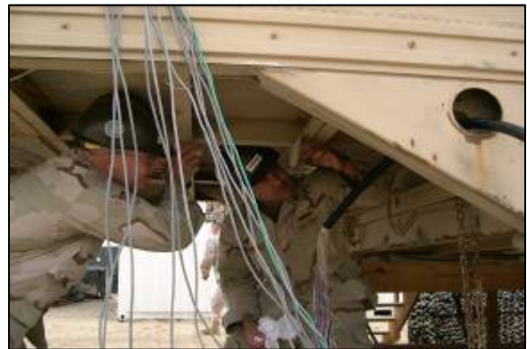
ISD Techs installing LAN Fiber
