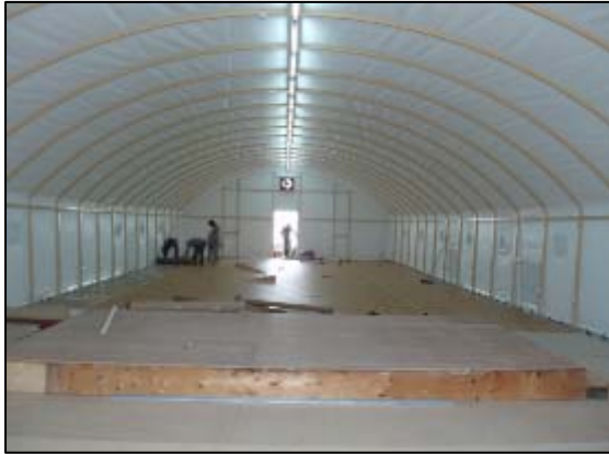
Start of work
