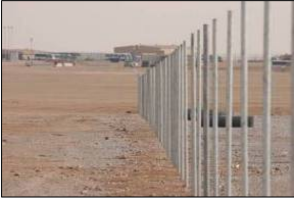
Laying out the fence post
