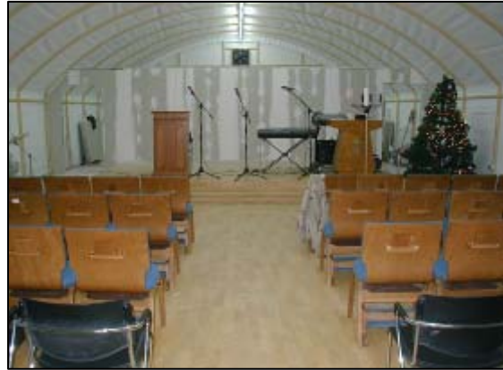
Wall completed awaiting paint
