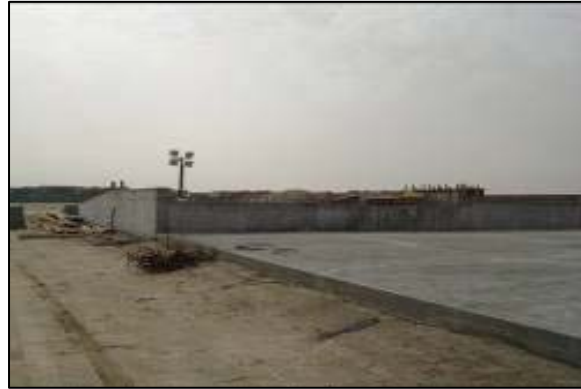
Concrete walls and apron
