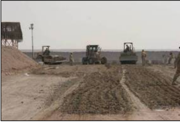
Making the first lifts
