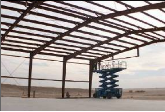
Laying out new structure
