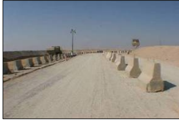
Completed entry/exit & starting track vehicle lane
