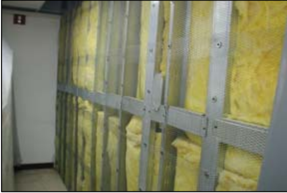
Metal studs and wire lathe
