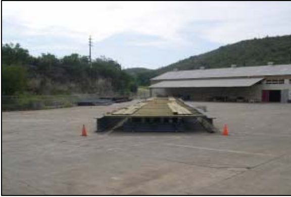
Bridge pre-assembly underway
