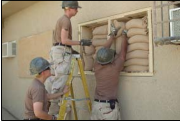
Installing blast protection Security container for BFT IZ5-100 Camp Fallujah CO Discretionary
