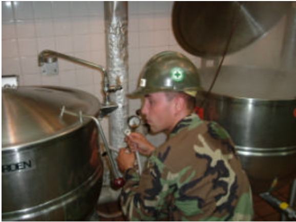
UT3 WOOD INSTALLING A WATERLINE FOR THE COPPER IN THE GALLEY.
