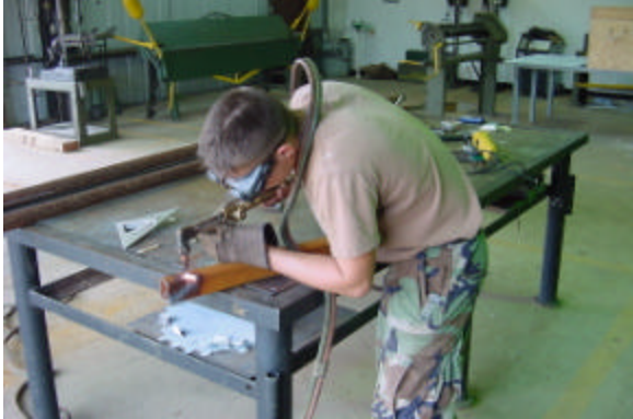
SWCN HILLEGASS FINISHING UP THE CUT ON A PIECE OF TUBE STEEL.
