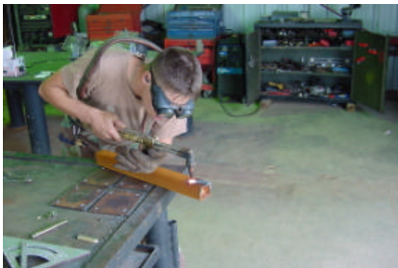
SWCN HILLEGASS CUTTING PIPE WITH TORCH FOR MCD PROJECT.
