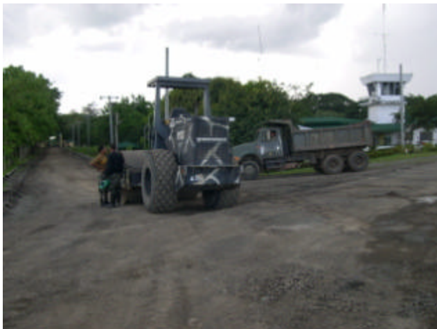
Preparing Aviation Access road for asphalt at Fort Magsaysay
