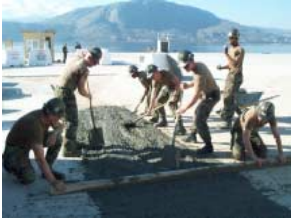
Marathi Recreation Center, Exterior Improvements
