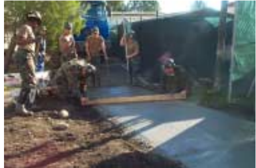
BOQ/BEQ, sidewalk construction
