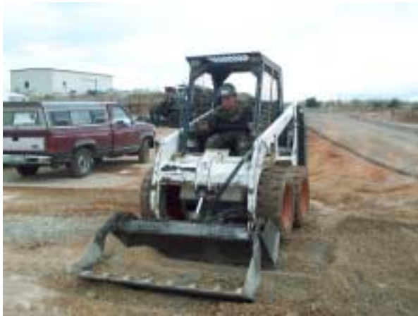
Construct Swale Behind PW
