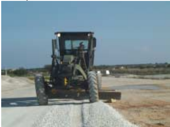
Taxiway Access Road Shoulder
