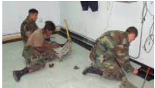
Install tile Black Stallion Supply Office
