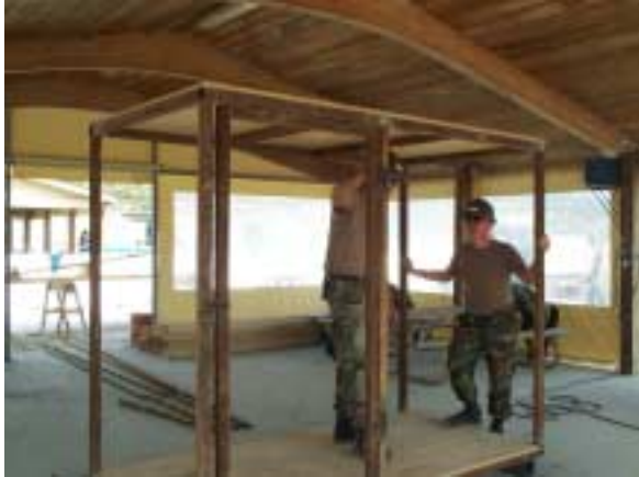
Construct EODMU 8 Drying Cage
