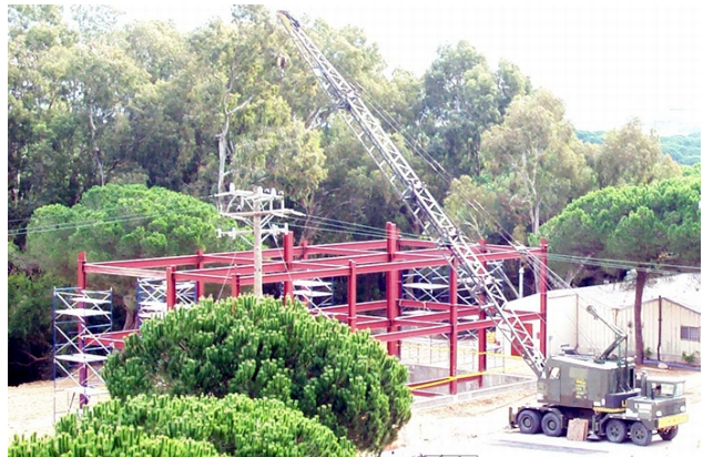
Crane Operations at Camp Mitchell Admin Facility
