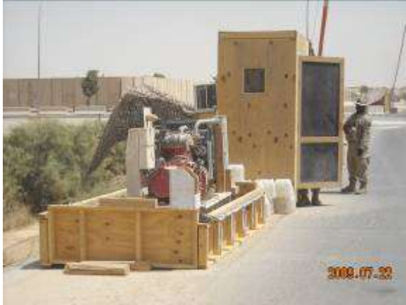
Generator and guard shack completed
