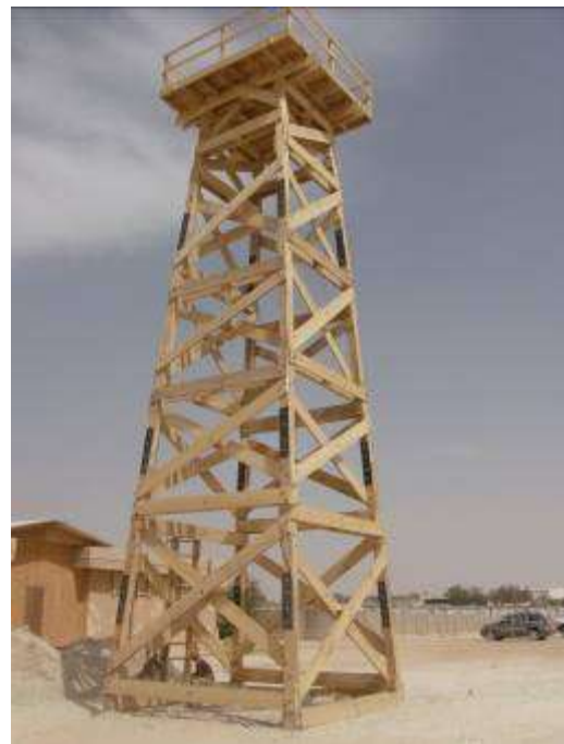
Completed tower framing
