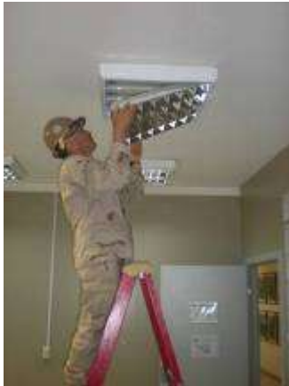
Ballasts replaced in a fluorescent fixture
