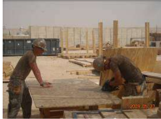
Prefab wall panel construction underway
