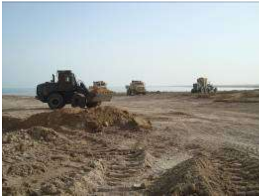
Work on turn around area continues
