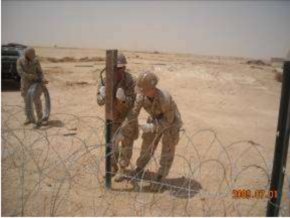
Concertina Post installation
