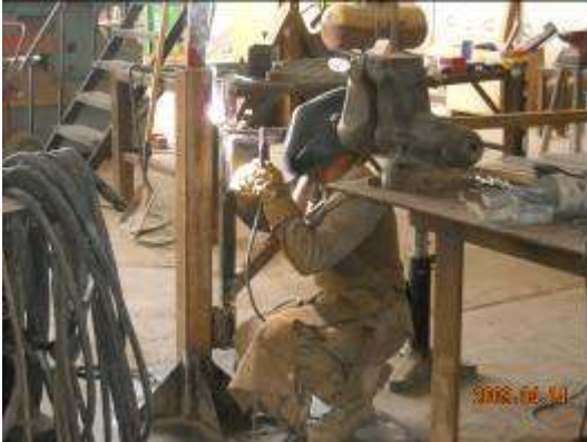
Steelworker welds gate at shop
