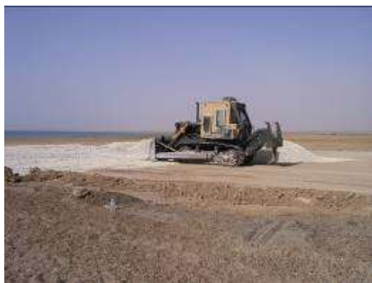
Dozer moves rock at equipment pad
