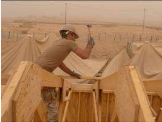
Purlin installation underway
