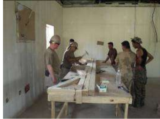
ISF learn floor truss prefab
