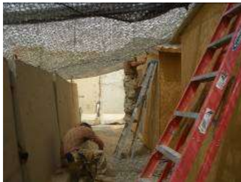
Shade netting installed
