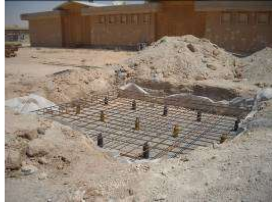
Foundation Mat constructed
