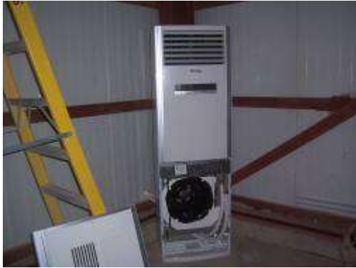
AC Unit placed
