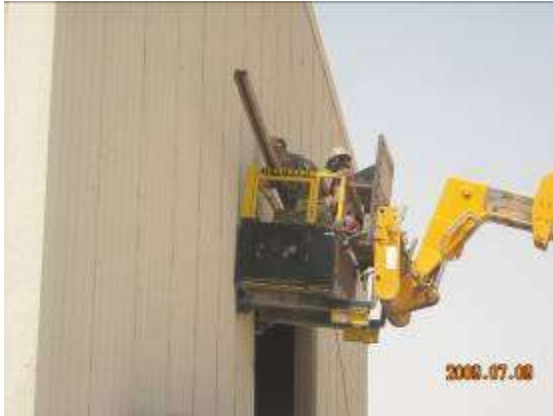
Door support rail installed
