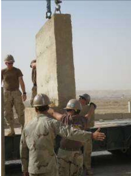
T-Wall stands unloaded
