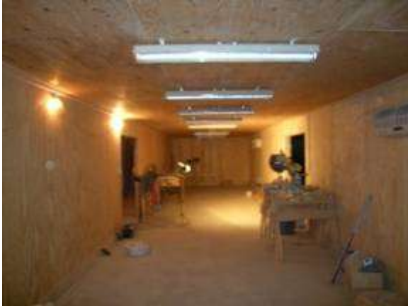
Interior of one of the Buildings
