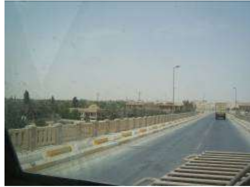
Bridge photo assessment
