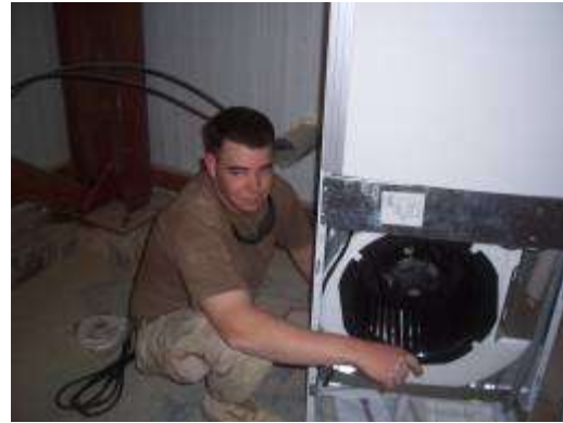
AC Unit prep underway
