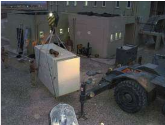
New Generator being installed
