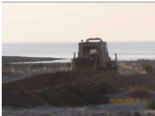
Dozer moves earth for roadway
