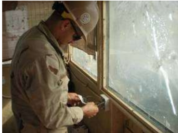
A receptacle is added
