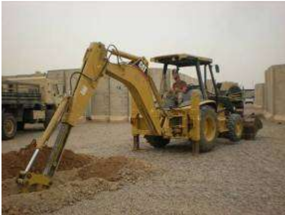
A trench is dug
