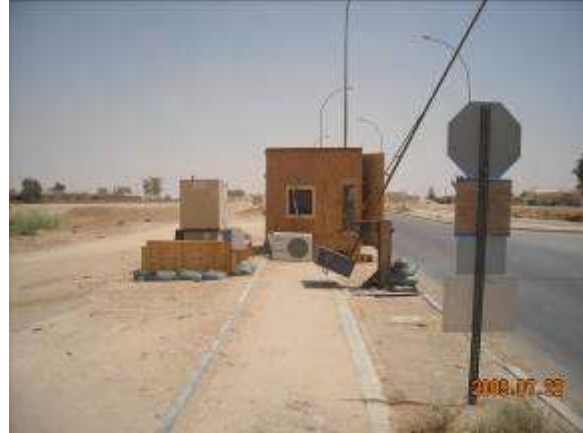
Guard shack, generator and gate
