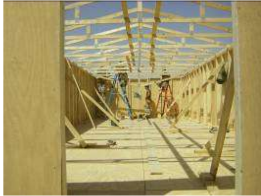
Seabees install trusses
