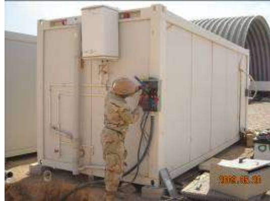
CE installs wiring at breaker panel
