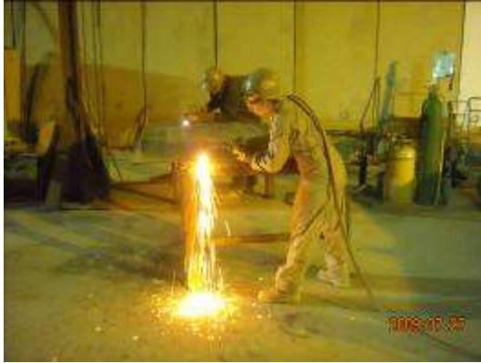
Steelworker cuts steel plates
