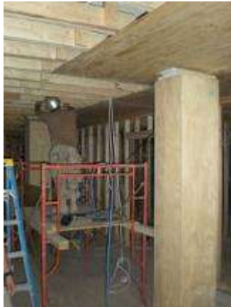
Ceiling installation on the first floor
