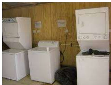
Dryer piping and power installed
