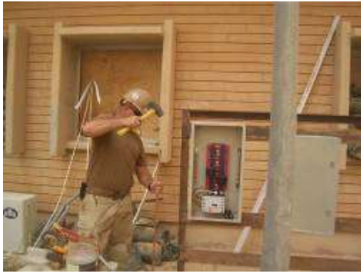
Breaker panel grounding rod install
