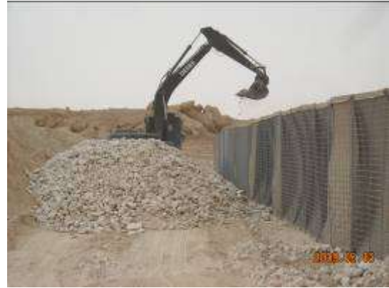
Excavator fills HESCOs with gravel
