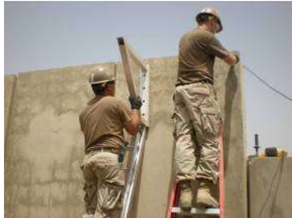
Solar lights installed across the camp
