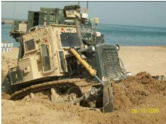
Dozer moves earth from Ramp area
