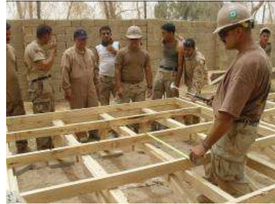
ISF view floor framing procedures
