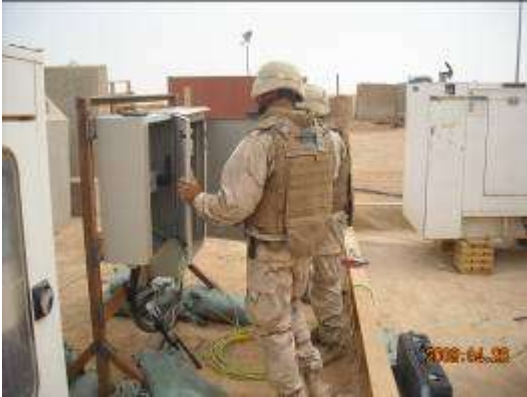
Breaker panel tie-in takes place
