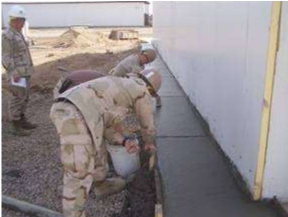
Concrete apron placed around building
