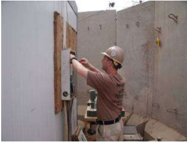
An existing panel is rewired correctly
