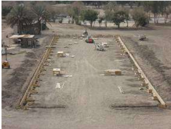
Formwork for Footers Installed
