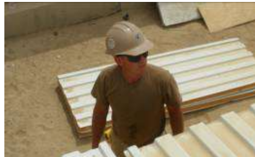
Seabee surveys the roof work
