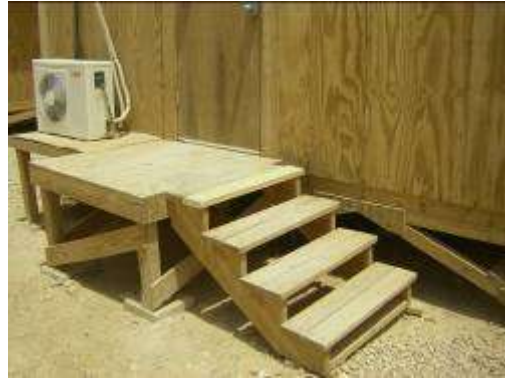
Stair and AC Unit platform
