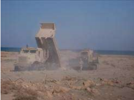
Road Construction underway
