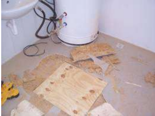
Repaired floor at water damaged area
