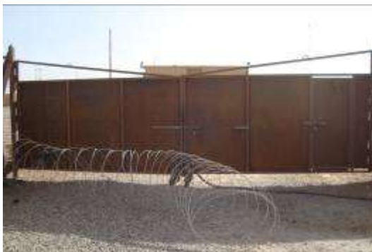
Concertina wire and Gate final install
