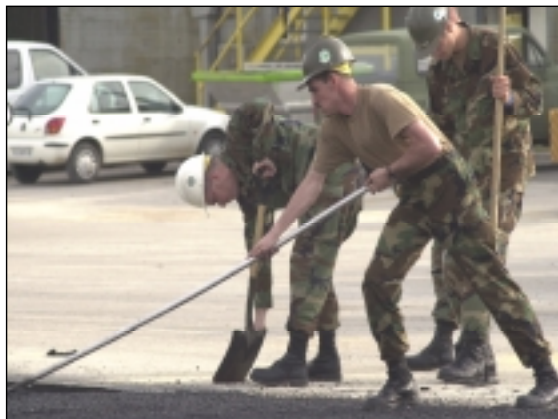
Spreading asphalt at Camp Mitchell.
