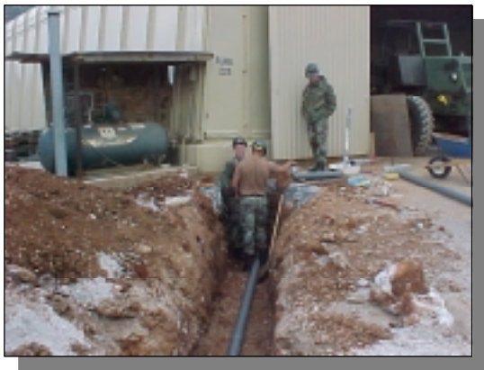
Seabees installing a sewage line for the mechanic shop head facility.
