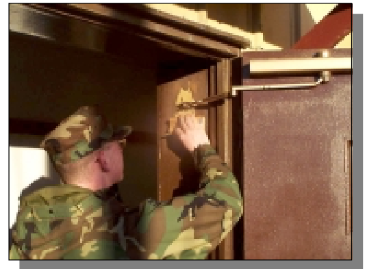
UT2 Akerman sanding repairs to door jamb.
