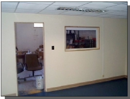
Renovated MLO Office
