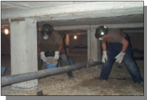
Soil removal from the galley underslab
