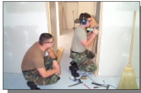
Construction of the Cyber Café
