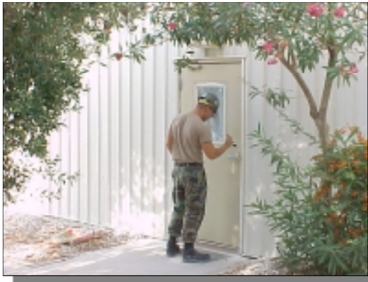
UTCN Accorsy painting Building 53.
