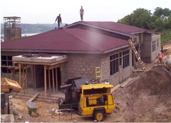
Medical/dental facility during construction.
