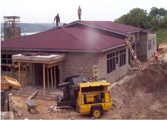
Medical/dental facility during construction.
