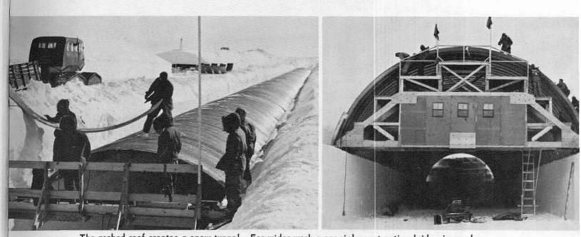
The arched roof creates a snow tunnel. For wider work a special construction bridge is used.
