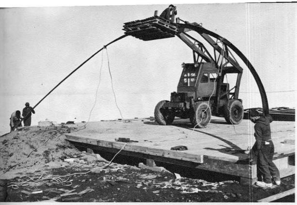
Navy CB steelworkers place a steel arch into place as they construct VX-6's hangar.
