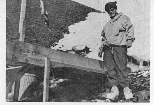
Lt Joseph A. Kelly, MC, officer in charge, standing beside newly built trough that is collecting water from a melting glacier at the rate of 30 gallons a minute.
