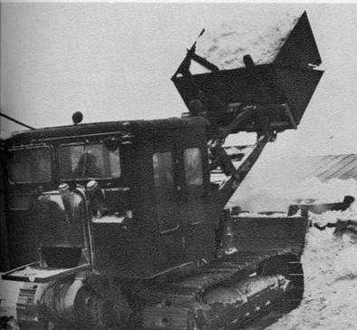
Above: At Williams Field two giant Hercules await loading of cargo for delivery to inland stations. Left: Snow for the water supply at McMurdo is hauled 24 hours a day from a nearby hillside and dumped into the melter.
