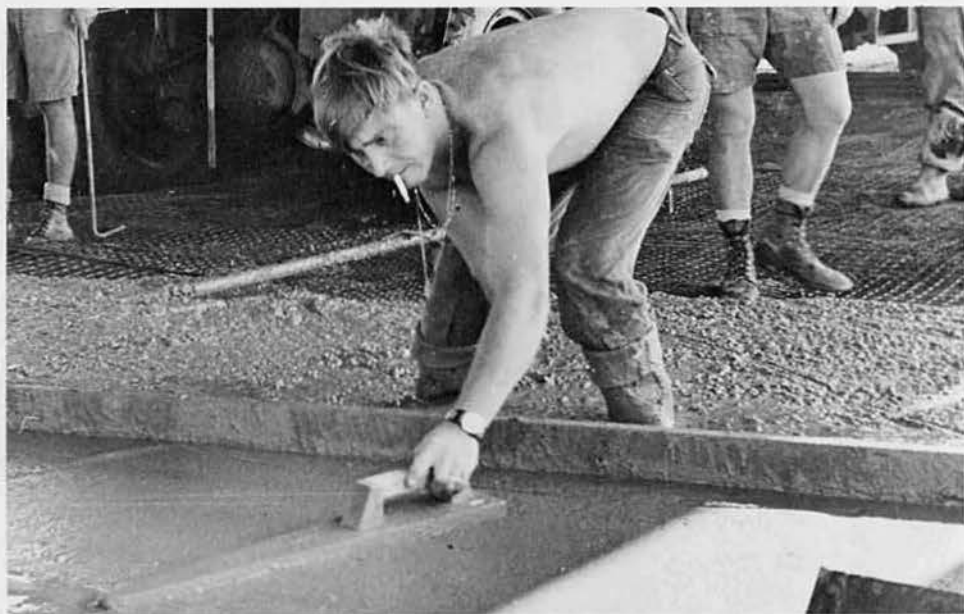
ABOVE: EA2 Bouska "floats" freshly poured cement.
