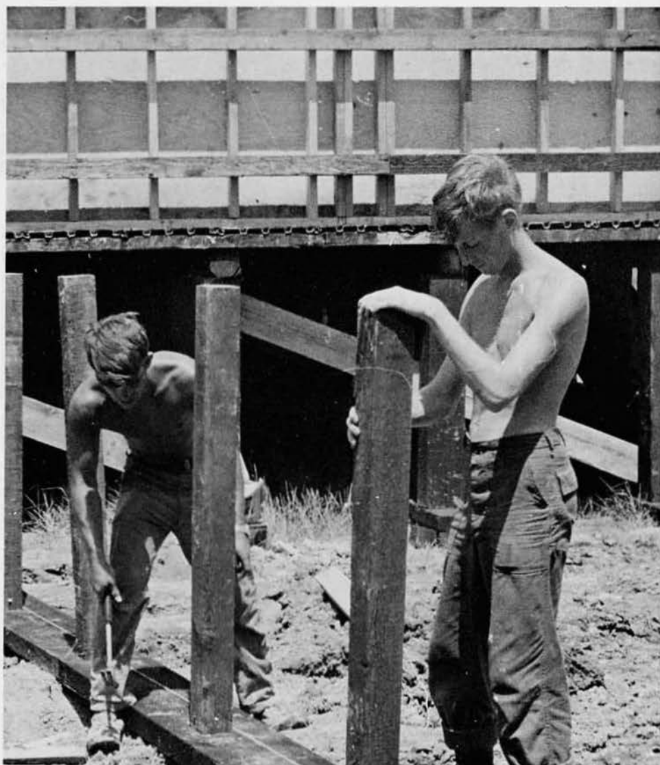
RIGHT: Building supports for various facilities and catwalks to be constructed.
