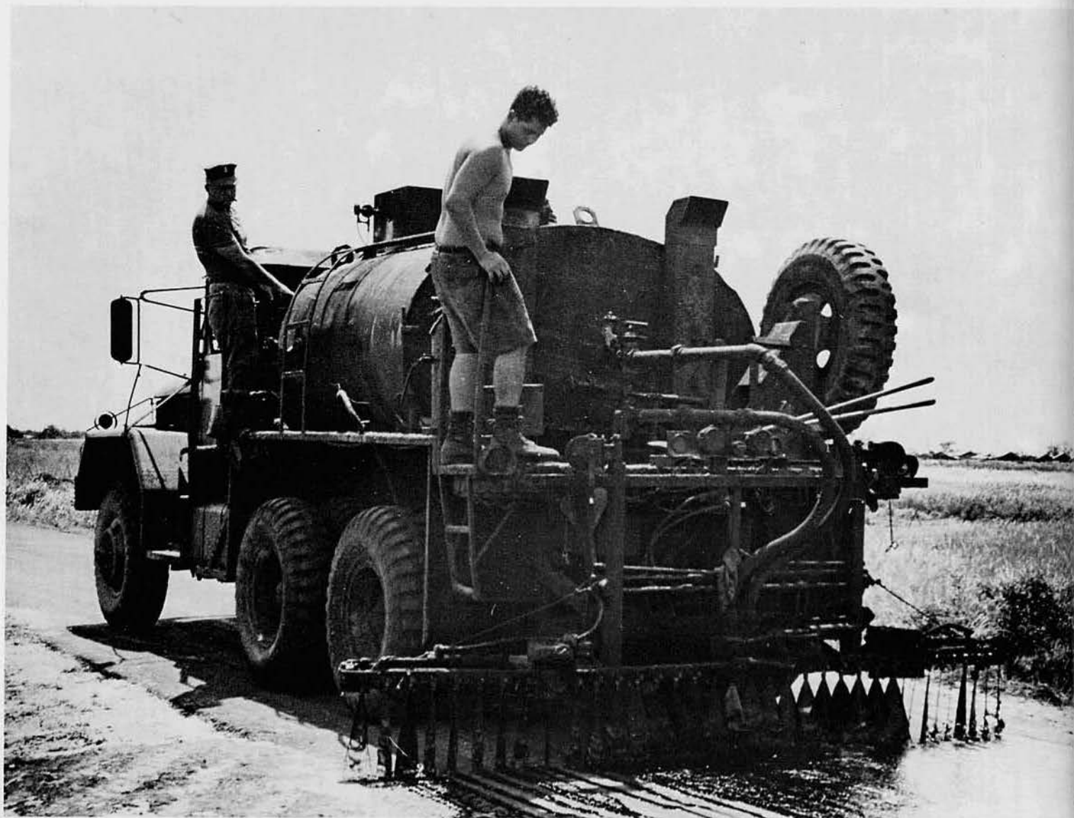
BELOW: Asphalt distributor paving the Can Gio road.
