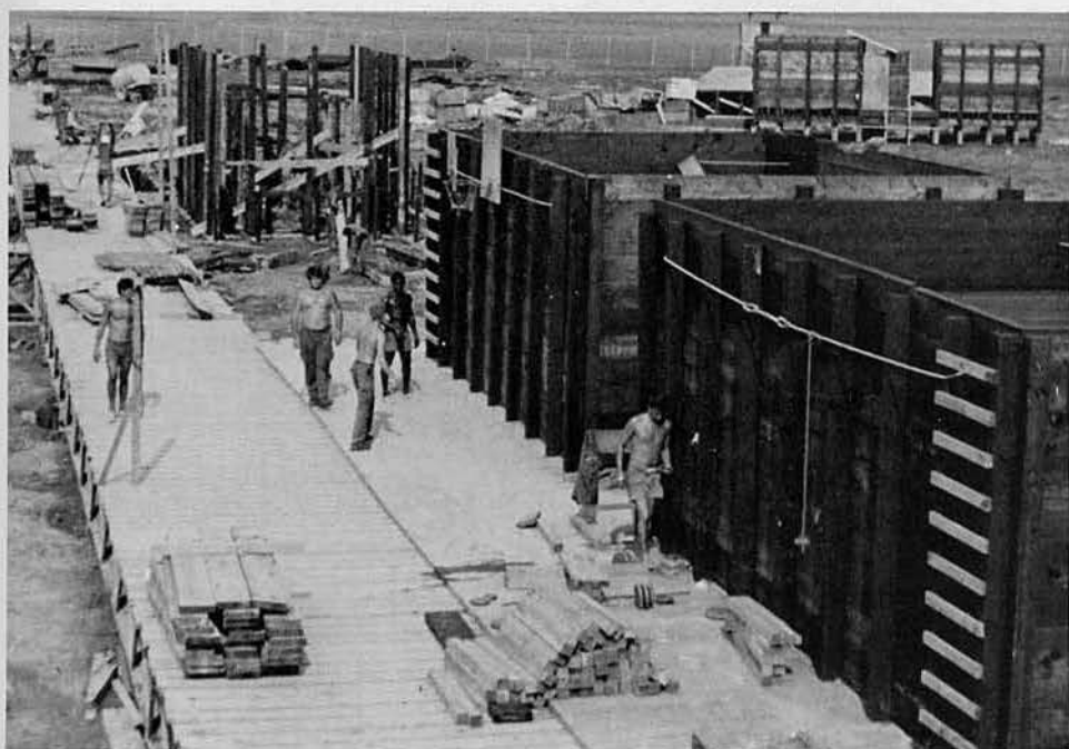
The 22 men of Detail Xray constructed an advance tactical support base at Phuoc Xuyen. The base, approximately 150 yards by 225 yards, was inundated with 3' of water during the monsoon season. Thus, it was necessary to construct the entire facility on stilts. A communication facility, helicopter pad, ammunition storage bunker, personnel bunker, perimeter defense systems, and 6' elevated catwalks were constructed at the site. The officer-in-charge of the detail was BUC D. E. Barnes.
