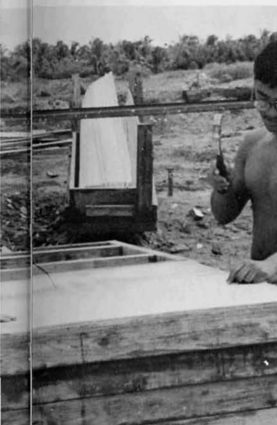
ABOVE: EA2 Bouska "floats" freshly poured cement.
