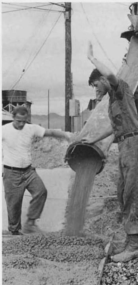
Pouring concrete for a command bunker.
