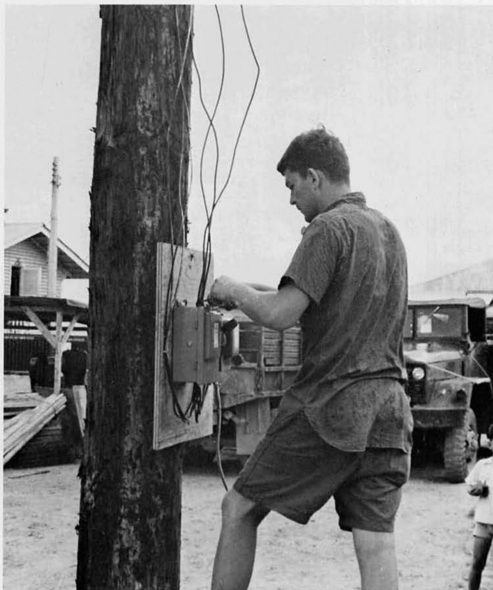
LEFT: SWCN Kahoiwai on watch. BELOW: CE3 Grenz installing a switch box for power distribution.
