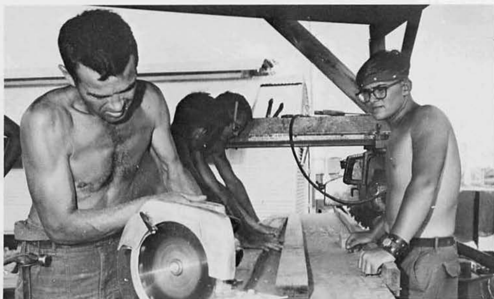
BELOW: BU2 Napier trims a board to be used in building frames.
