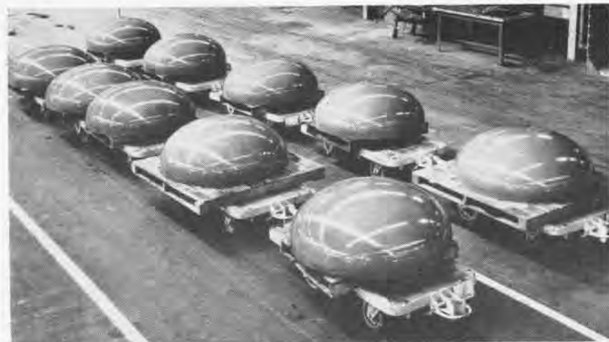
POLARIS rocket chamber end enclosures, explosively formed from flat blanks of high strength steel, stand ready for shipment at Aerojet-General's Ordnance Division, Chino Hills Laboratory. Uniformity of diameter, thickness is improved by process.
