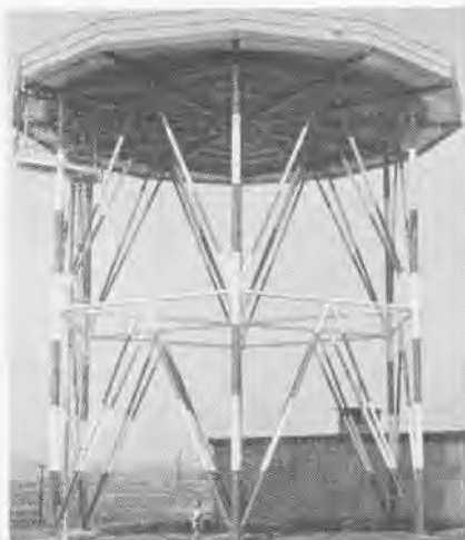
NEW RADAR antenna at NAS Miramar nears completion. To enter service next year, it will increase station's radar capability by 50 percent. FAA operated, it will give sharper image, won't pick up building reflections.
