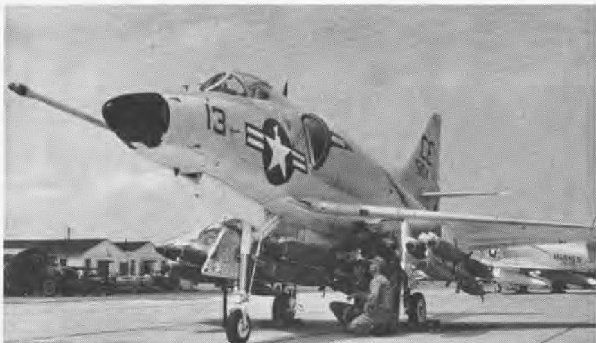
EXPERIMENTAL Multiple Bomb Rack , which has been evaluated at NATC Patuxent River, is displayed on an A4D of VMA-225 at Cherry Point. Three multiple racks may be suspended from A4D type aircraft. Each rack can carry six 500-lb. bombs or 12 250-lb. bombs.
