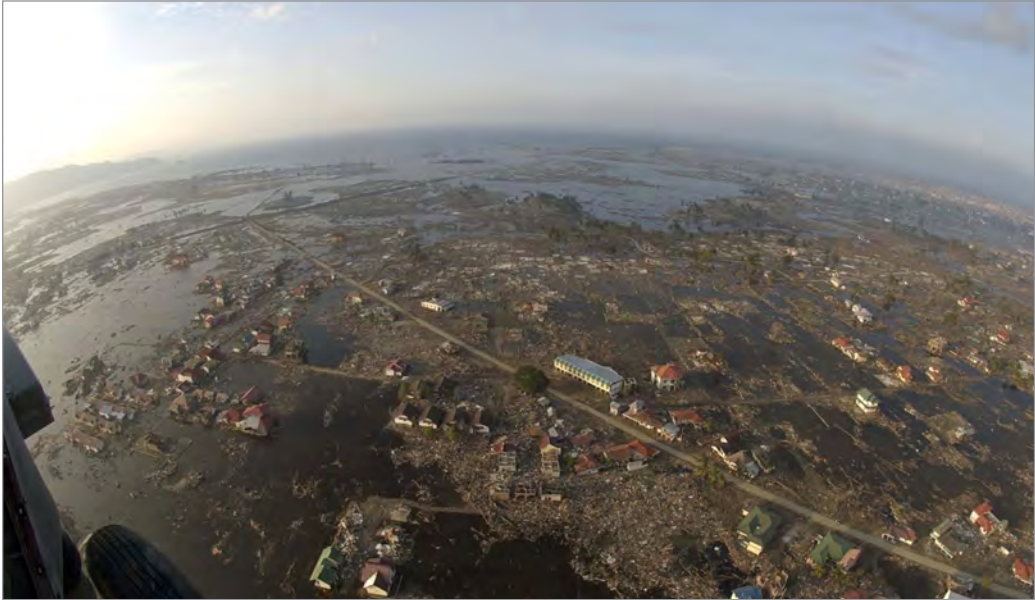
An aerial view of the devastation in Banda Aceh following the December 2004 earthquake and tsunami. (Photographer's Mate Third Class Jeremie M. Yoder, USN; NARA, DN-SD-06-12137)
