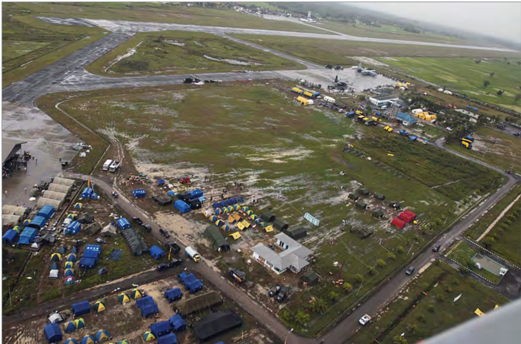
An aerial view of Banda Aceh Airport on the island of Sumatra, Indonesia. Note that there was very little dry land near the taxiways to store relief supplies and erect tents for military personnel and aid workers. (Photographer's Mate Airman Patrick M. Bonafede, USN; NARA, DN-SD-06-12028)
