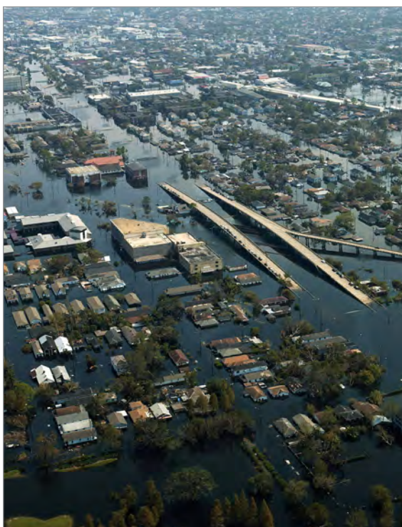
An aerial view of the devastating flooding caused by breakage of the levee separating the city of New Orleans from the Mississippi River and Lake Pontchartrain during Hurricane Katrina. (Photographer's Mate Second Class Michael B. Watkins, USN; NARA, DN-SD-06-02467)
