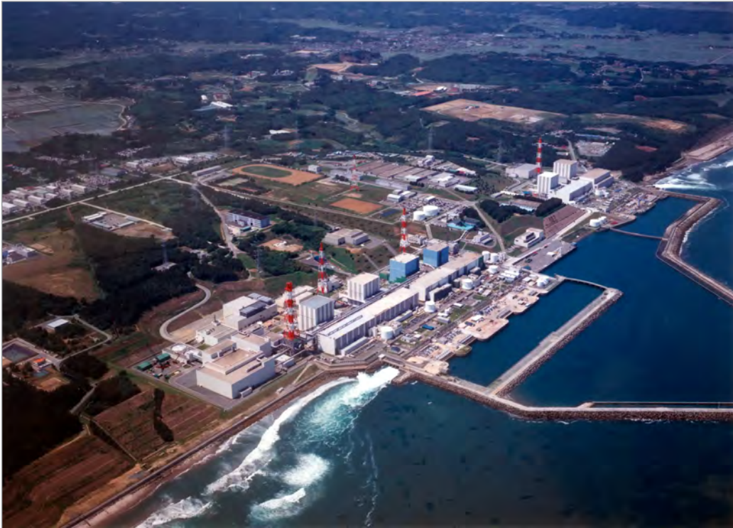
Aerial view of the Fukushima Daiichi Nuclear Power Plant taken before the disaster in 2011. The tallest six buildings contain the nuclear reactors in numerical order beginning with Unit 1 ( foreground, left ) and ending with Unit 6 ( background, right ). (International Atomic Energy Agency [IAEA], 8388174045)
