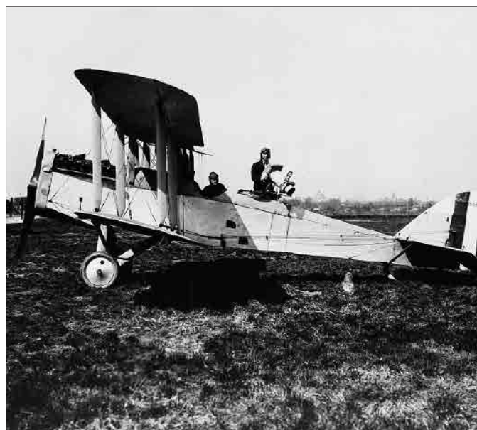
An aerial camera fitted to the gun mount of a DH-4 biplane.
