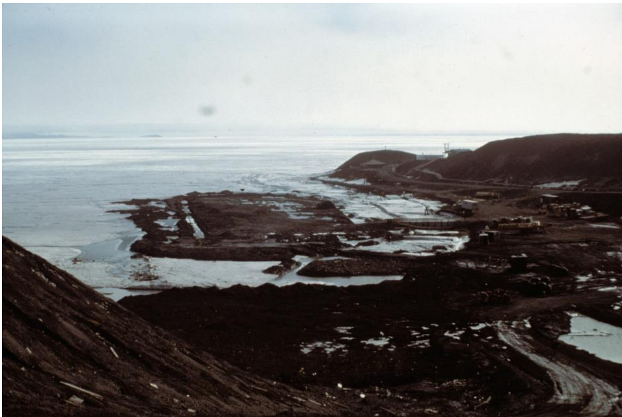
The ice pier with explosive charges set along the white line near the outer edge of the pier. The pontoon bridge is seen between the pier and the land at the right.
