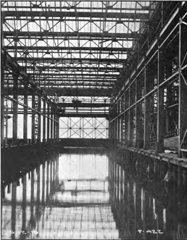
Interior view of wet slip, Squantum destroyer plant.
