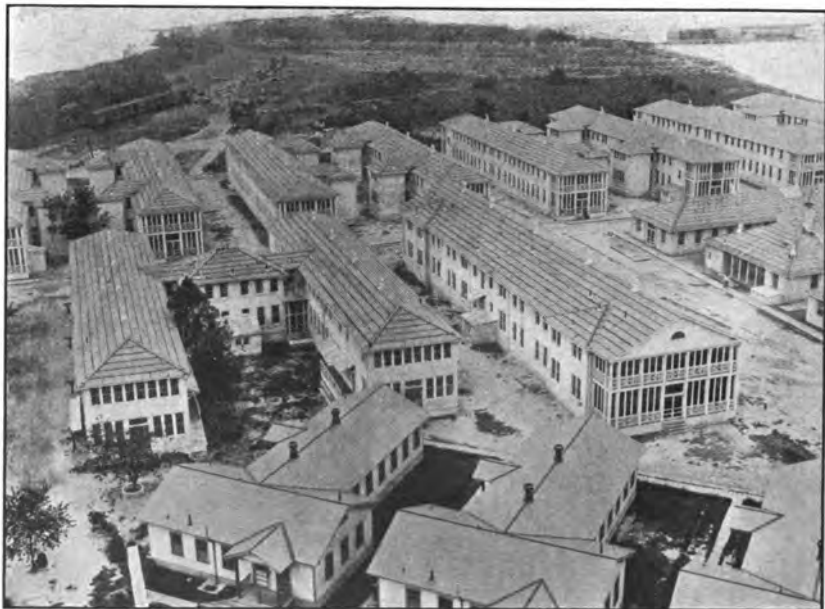
Emergency buildings, Naval Hospital, Norfolk, Va.
