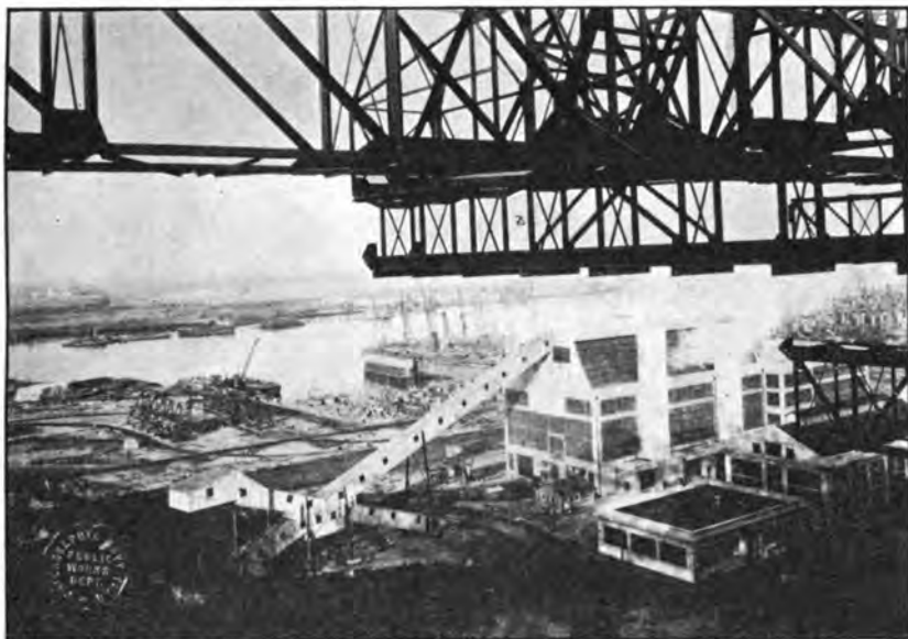
Power plant, Navy Yard, Philadelphia, Pa. View showing coal-handling plant (left), taken from crane runway of shipbuilding slip.
