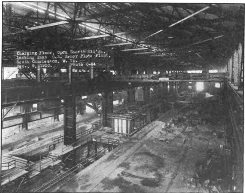
Charging floor of open-hearth building, Armor Plant, Charleston, W. Va.
