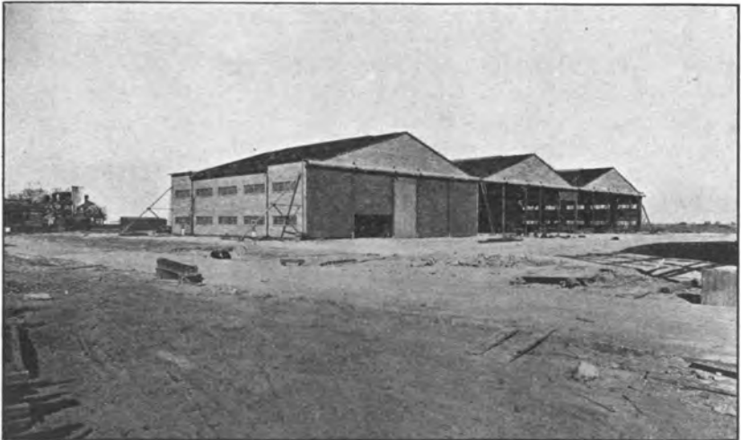
Seaplane hangars, Hampton Roads, Va. ; straight-truss, rolling-door type.
