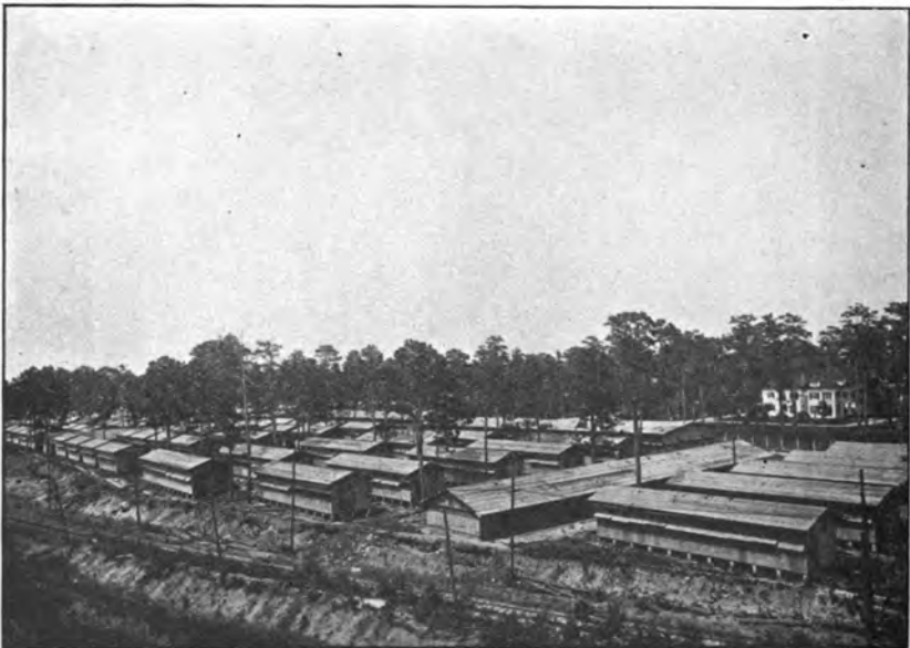
General view, Naval Training Camp, Charleston, S. C.
