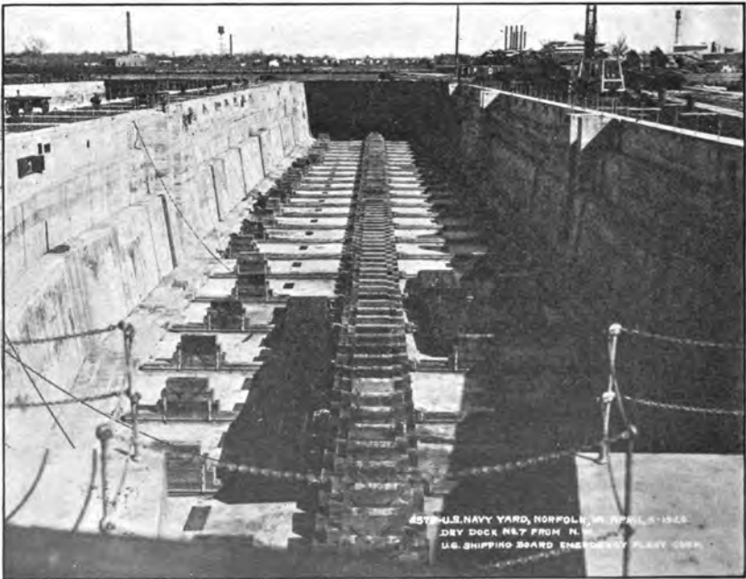
Dry Dock No. 7, Navy Yard, Norfolk, Va. Looking toward caisson.
