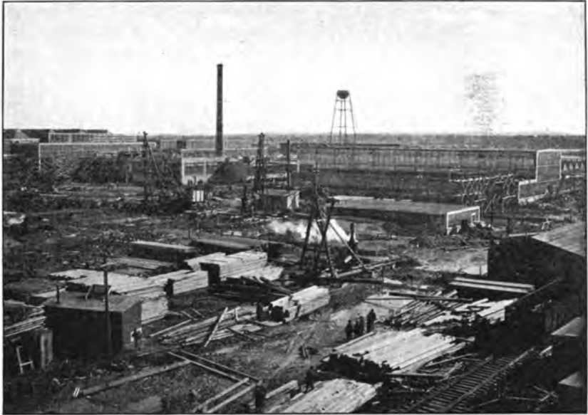
Squantum destroyer plant. General view during construction.
