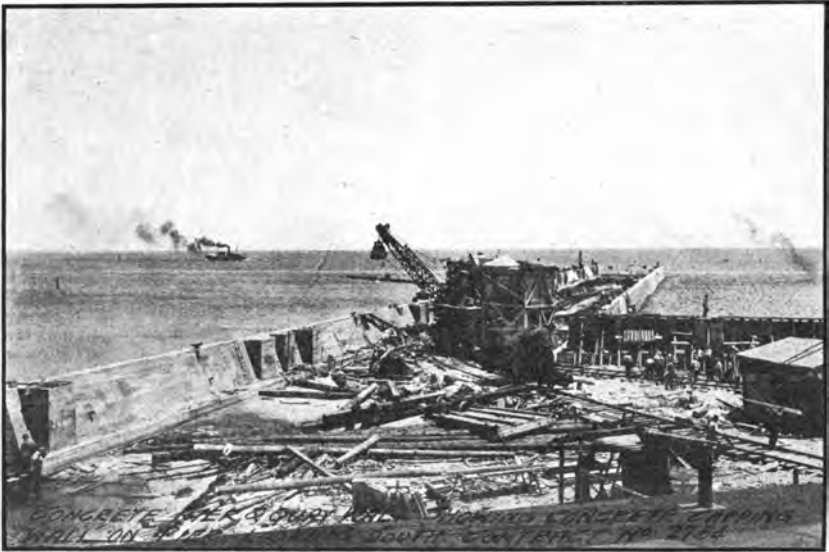
Concrete retaining wall for pier, Naval Air Station, Pensacola, Fla.
