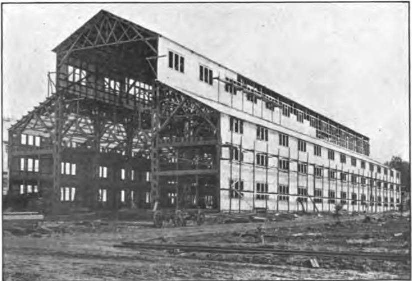
Boat-storage building (timber), Navy Yard, Mare Island, Calif.
