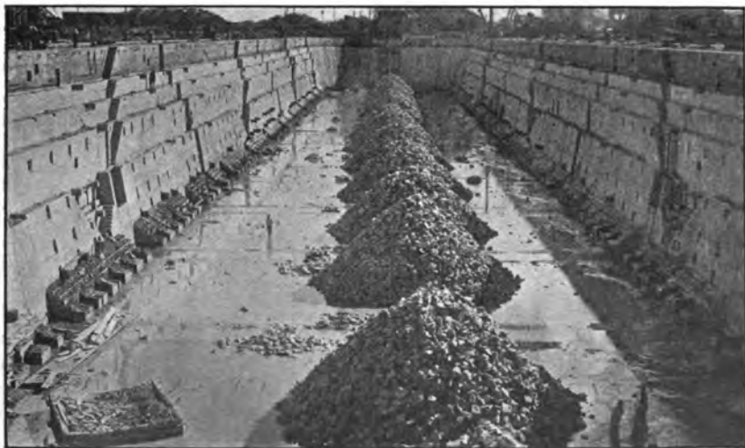
Dry Dock No. 1, Naval Station, Pearl Harbor, Hawaii. Interior view after first pumping, showing rock ballast before completion of floor.
