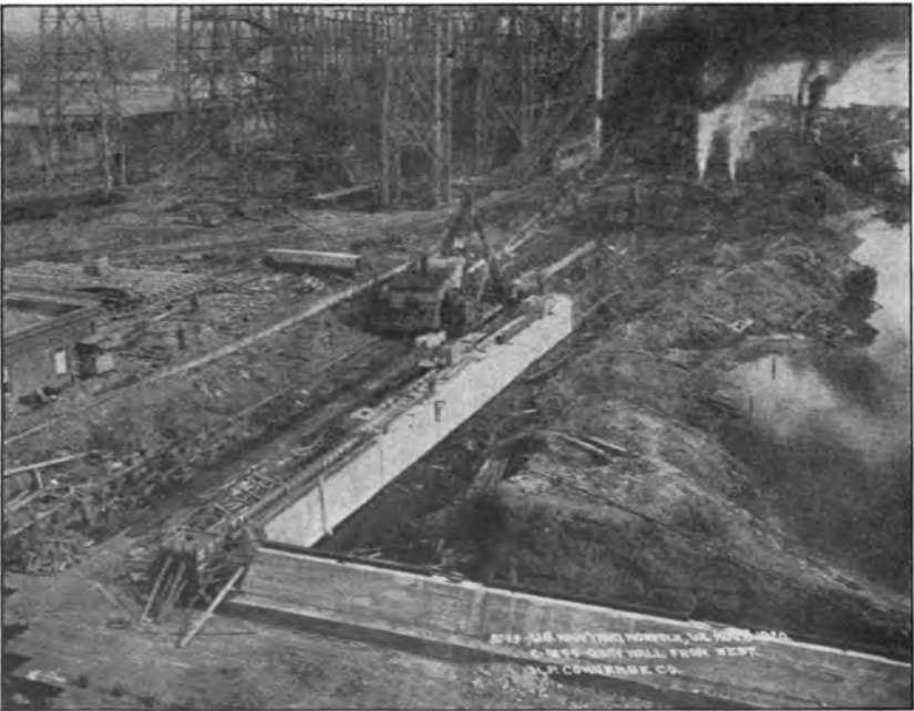
Construction of concrete retaining wall, Navy Yard, Norfolk, Va.
