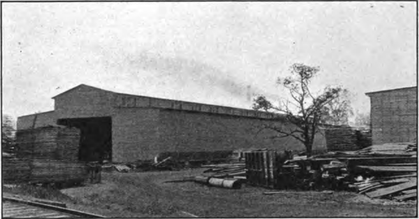
Lumber-storage building, Navy Yard, Portsmouth, N. H.
