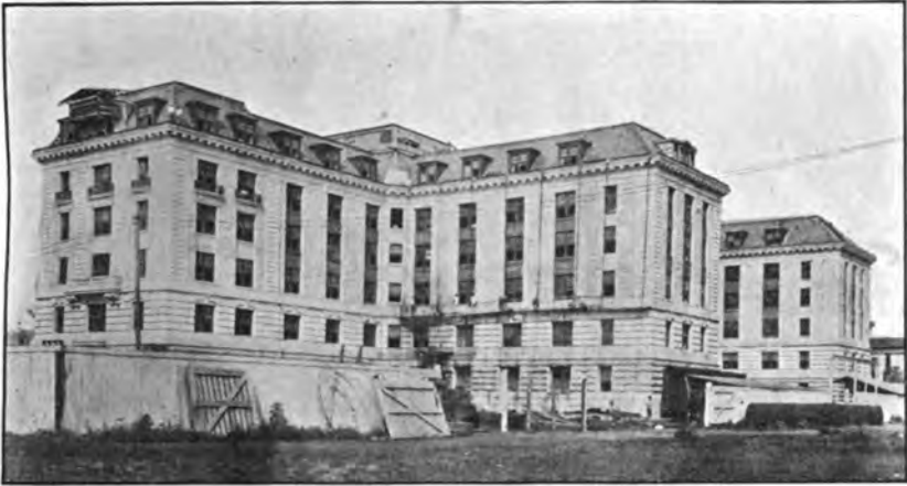
Bancroft Hall extension, east wing, Naval Academy, Annapolis, Md.
