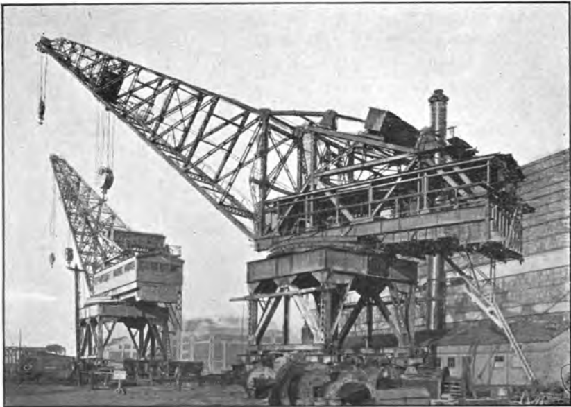
Locomotive cranes (50-ton) for Dry Dock No. 3, Navy Yard, Philadelphia, Pa.
