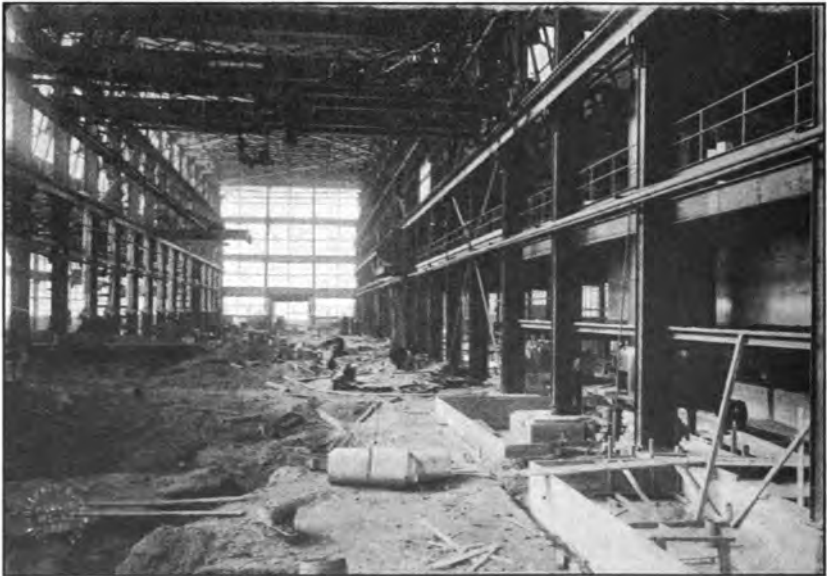
Foundry, Navy Yard, Philadelphia, Pa. Interior view.
