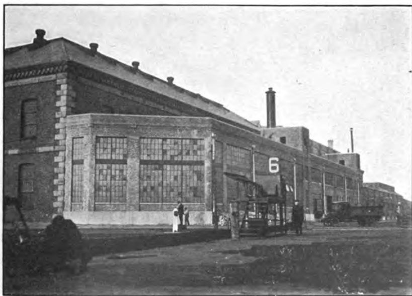
Foundry, Navy Yard, Boston, Mass. Second extension.
