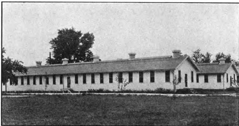
Ward buildings, Naval Hospital, New Orleans, La.
