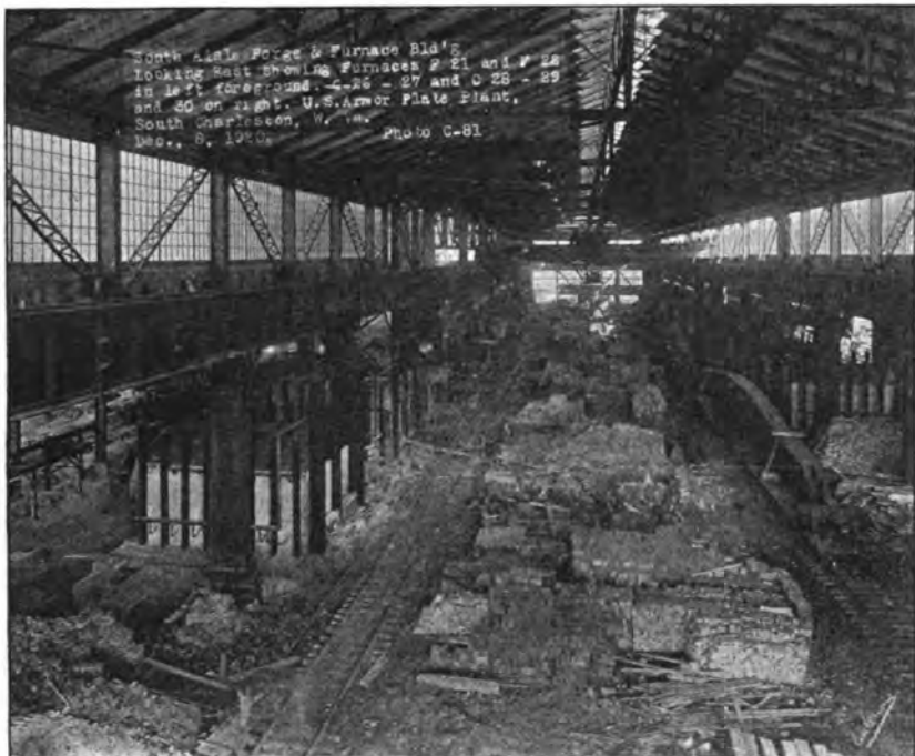
South aisle of forge and furnace building, Armor Plant, Charleston, W. Va.
