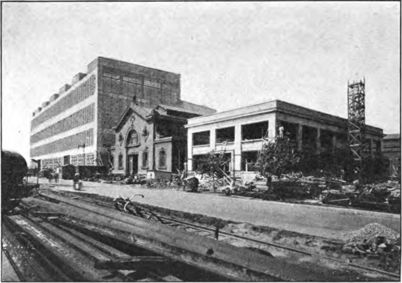
Machine shop (center) and "extension" (left), Navy Yard, Philadelphia, Pa.
