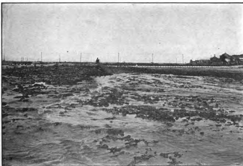
Filling behind bulkhead, Naval Operating Base, Hampton Roads, Va.
