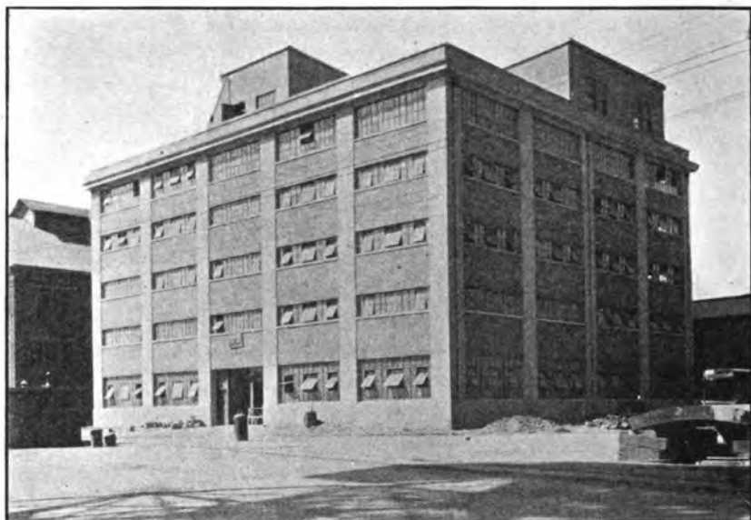
Electrical storehouse, Navy Yard, Mare Island, Calif.
