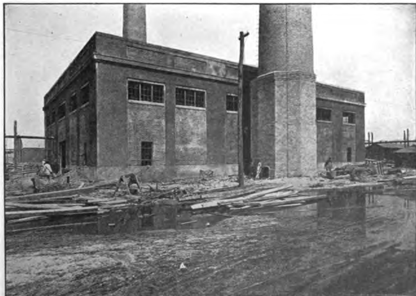
Boiler plant, East Camp, Hampton Roads, Va.
