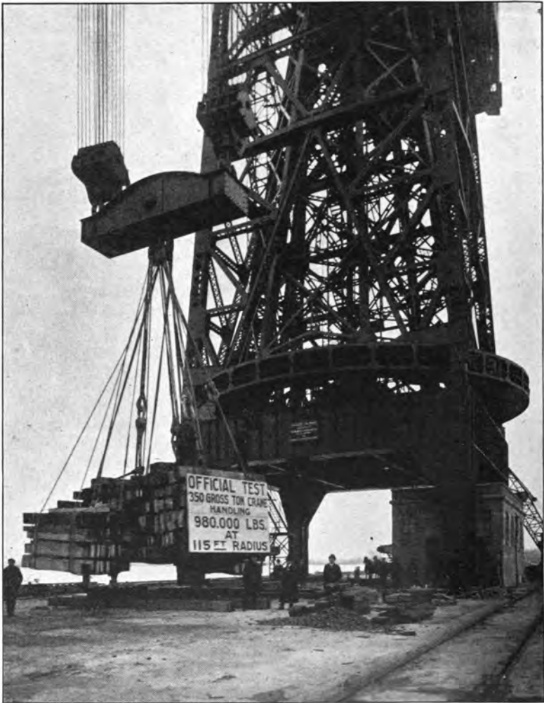
Official test of 350-ton fitting-out crane, Navy Yard, Philadelphia, Pa.
