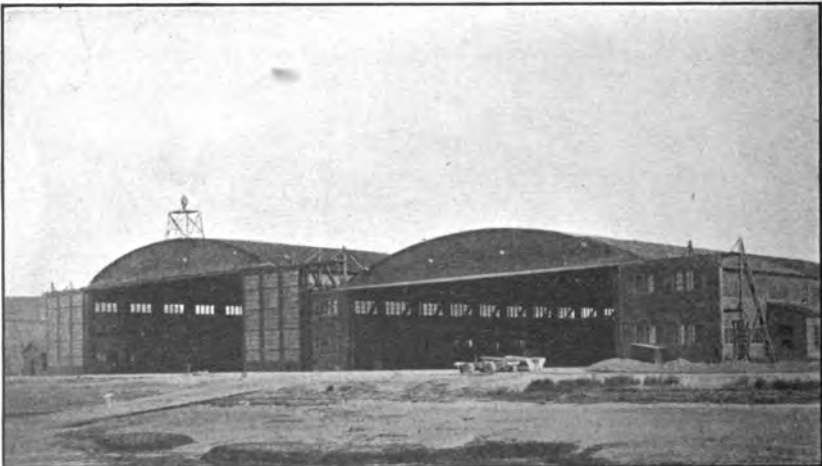
Seaplane hangars, Cape May, N. J.; curve-truss, sliding-door type.
