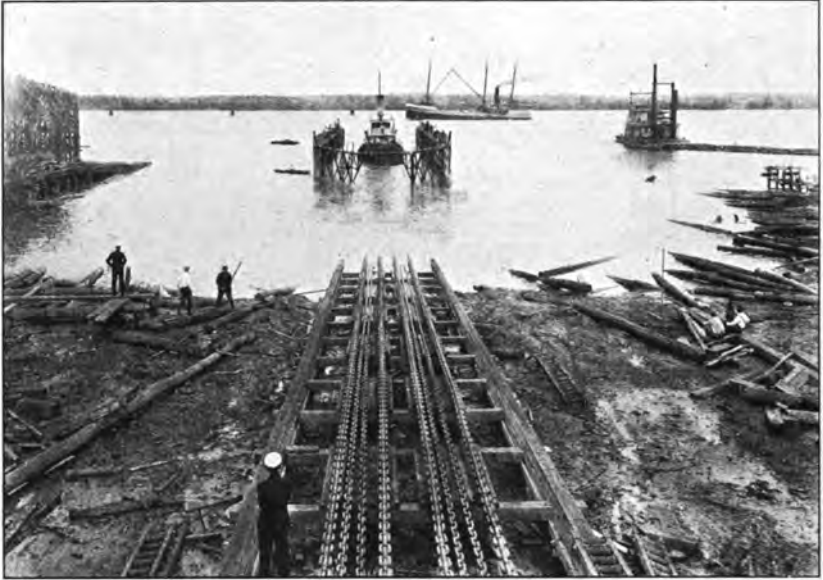
Marine railway, Navy Yard, Charleston, S. C. Cradle submerged.
