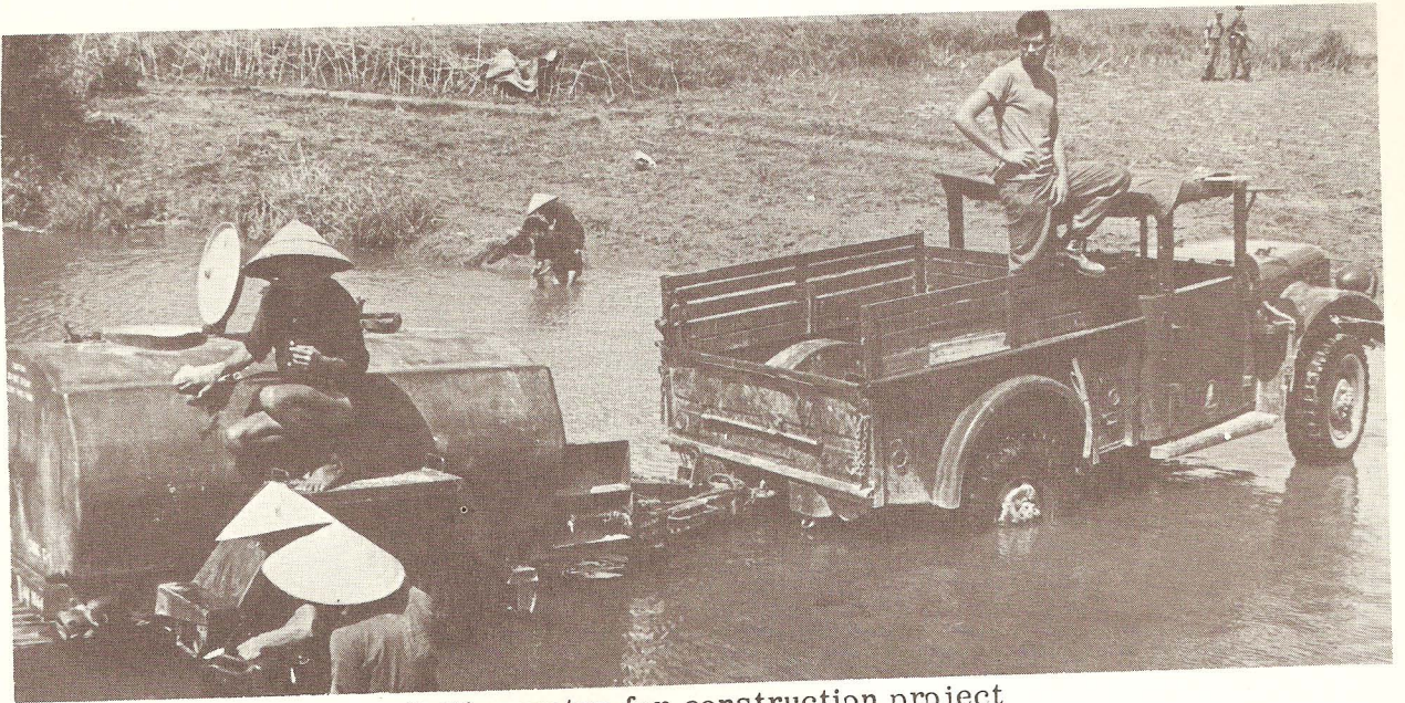
Getting water for construction project
