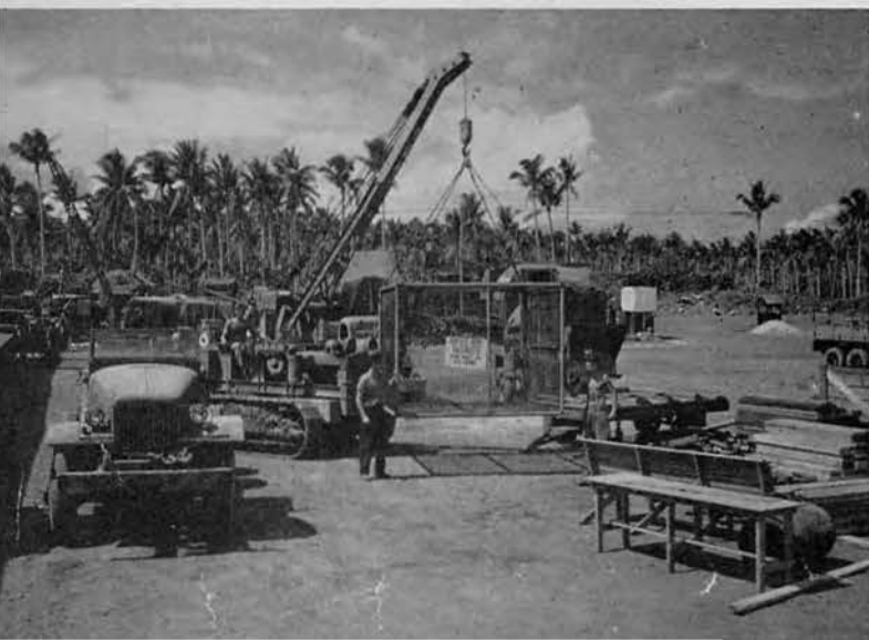
Lower left: The area in front of the maintenance building at Samar. The sign on the monkey cage says, "Enter here all disgruntled Seabees who want to go home."
