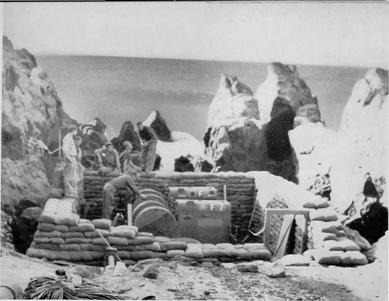
The beach pumps that pumped sea-water to the 95th Water Purification Stills; sand bagging before bomb proof roof was added. One of the 95th Water Stills—Destefano, J. W. Taylor, Kolb, W. W. Young.
