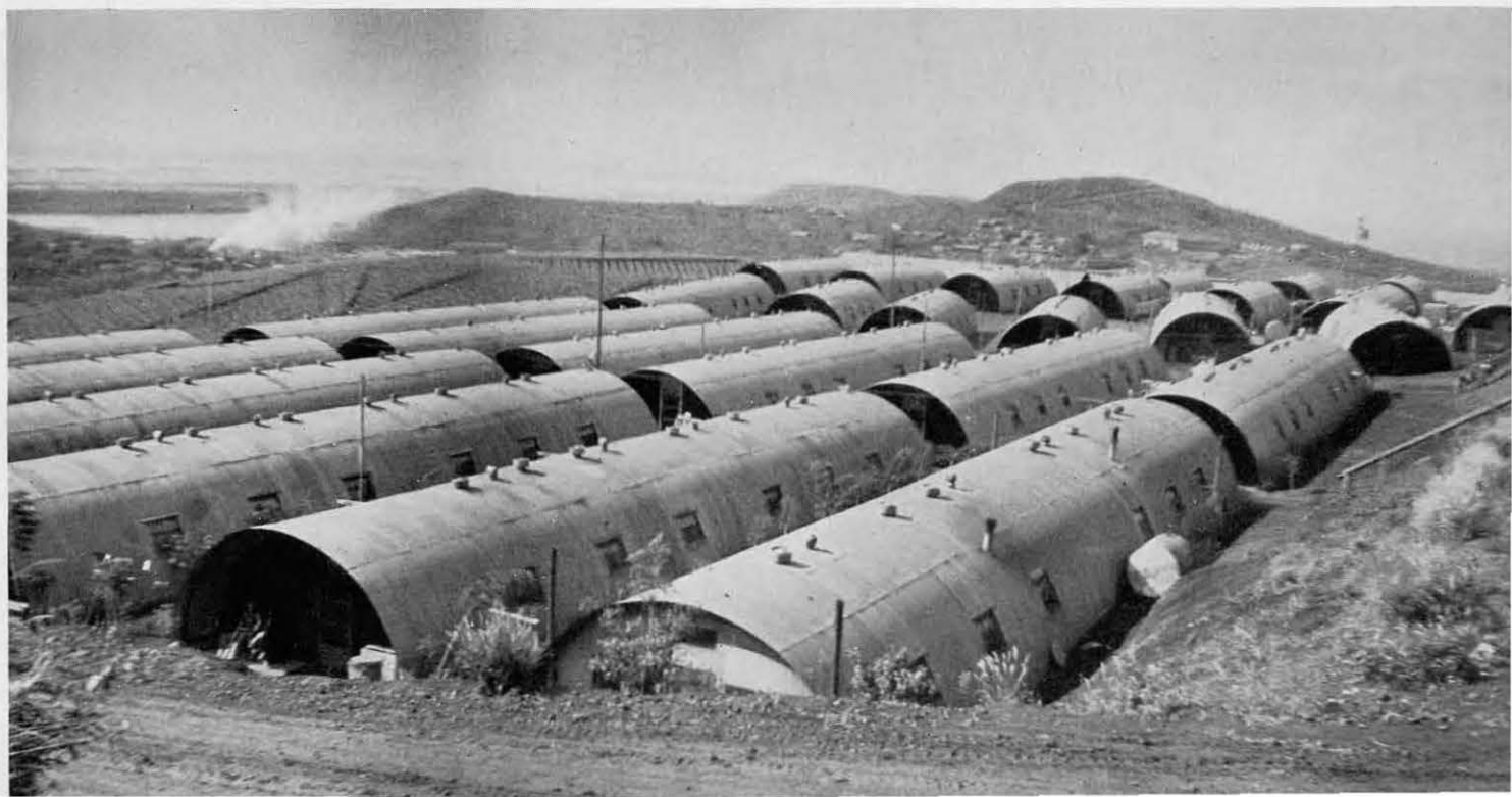
The upper part of the 95th area at Red Hill.
