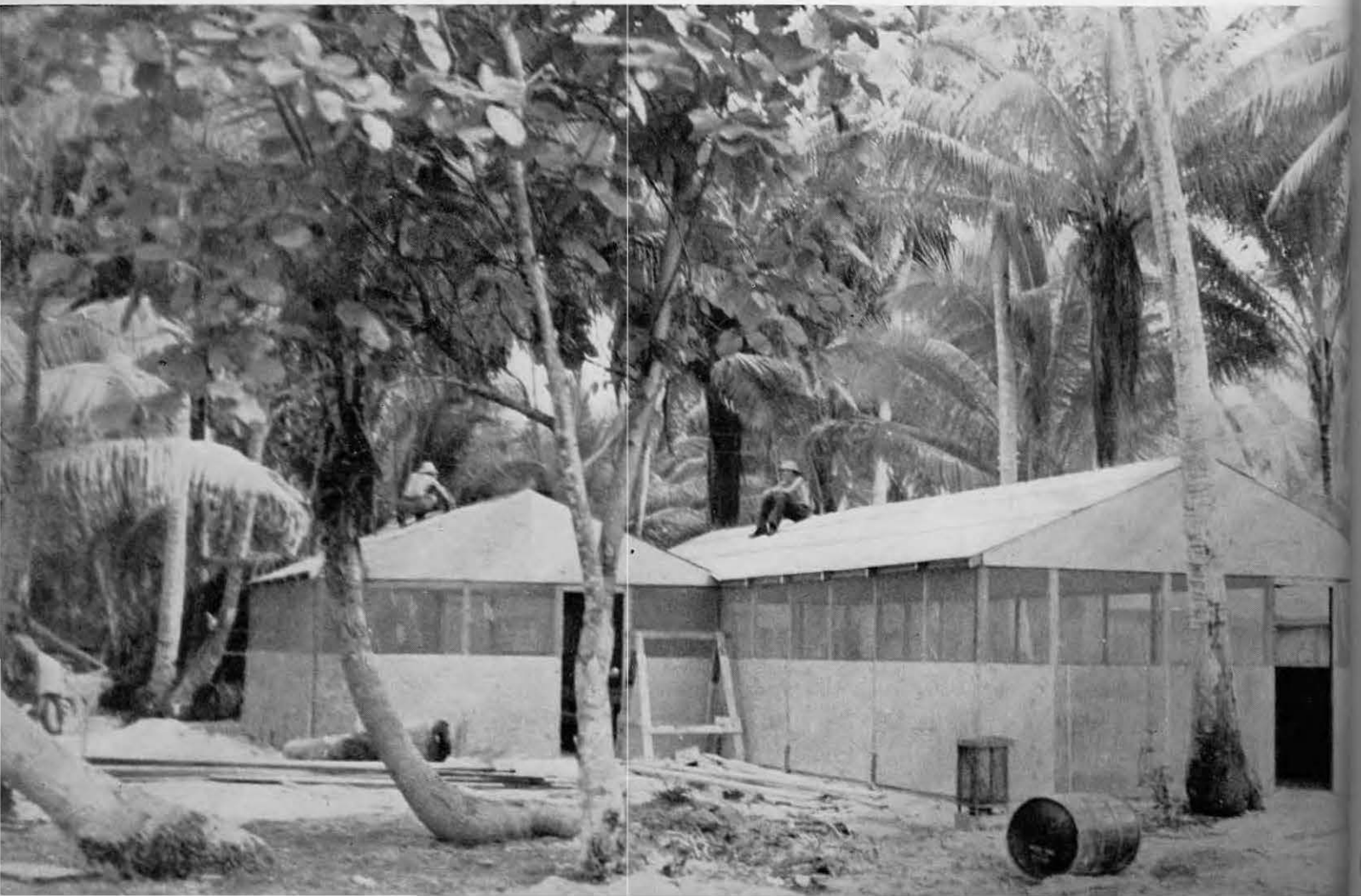
95th CHOW HALL—side view (incomplete).
