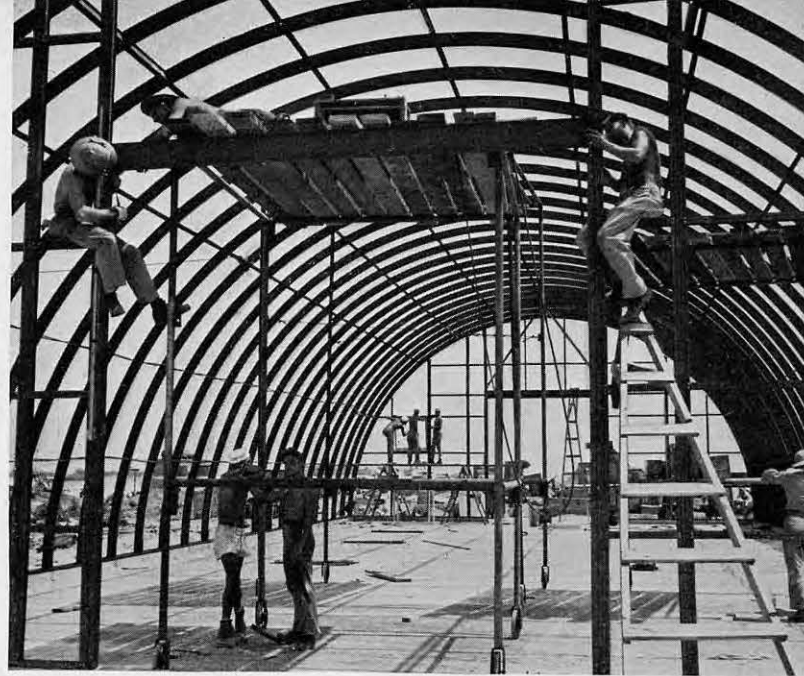
Framework of one of 19-40 x 200 foot storage huts.
