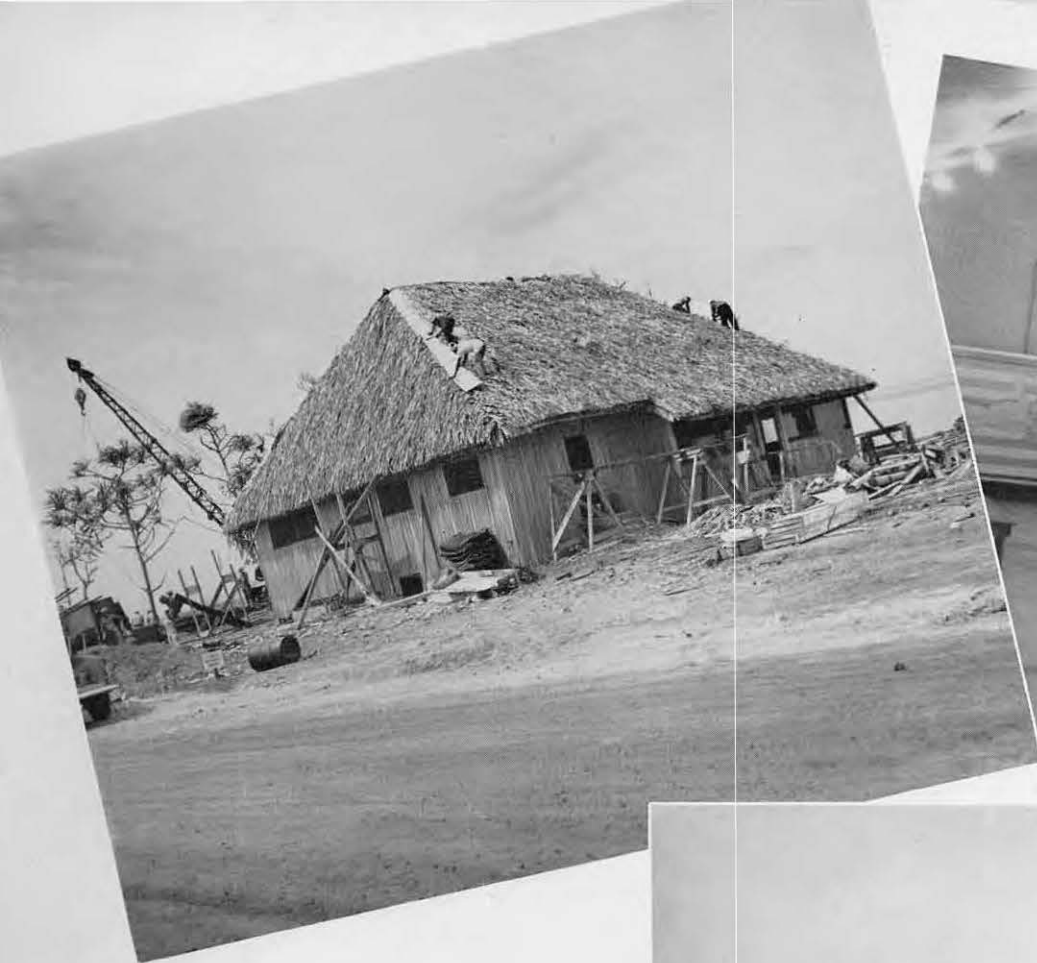
Construction of the Island Commanders house; natives thatching roof.
