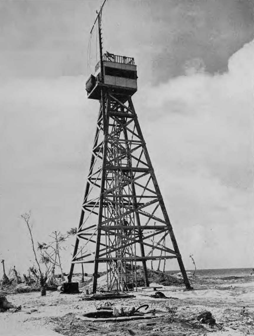
Timber signal tower, 80 feet high, Ivan Island.
