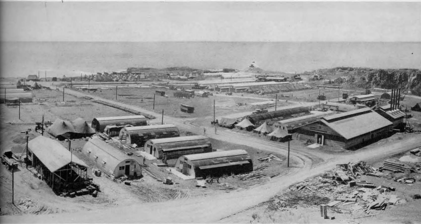
Hospital under construction.
