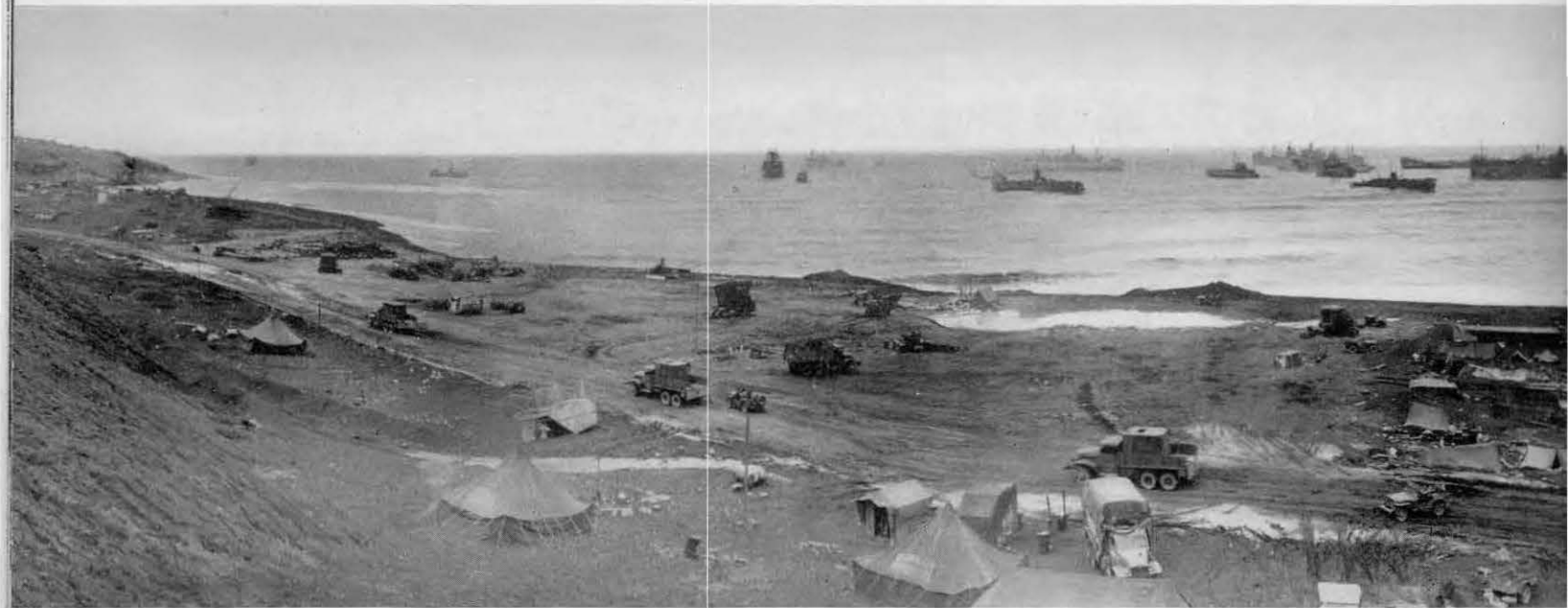
Panorama of Brown Beach, stabilized and graded by the 95th.
