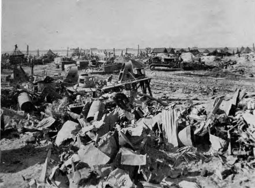
'Dozers starting to clear an area for the 95th camp.
