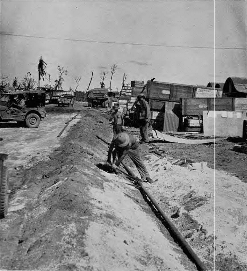
Laying water pipe line.
