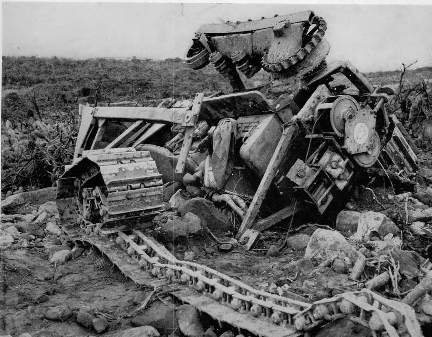
Wreck of a D-8 'Dozer. It was while operating this dozer April 25 that Francisco (Poncho) Jaramillo was killed as the blade struck a buried enemy land mine.
