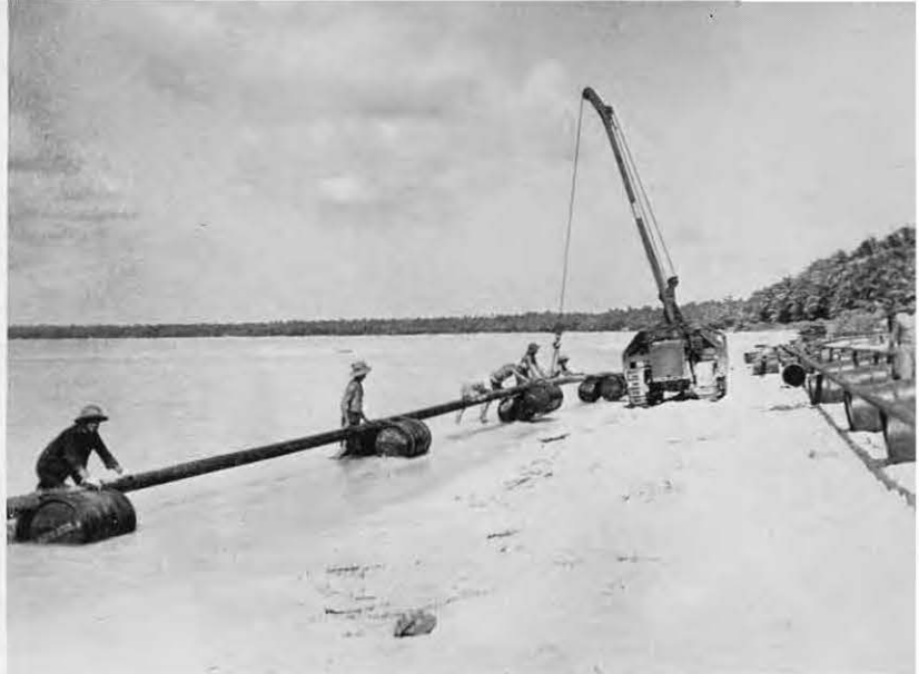
Launching Pipe Line from Tanker buoy to tank farm, January 18, 1944.
