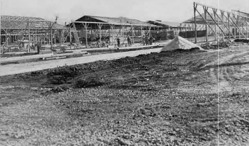
Part of huge Manana job—storage warehouses (750,000 square feet of covered storage).
