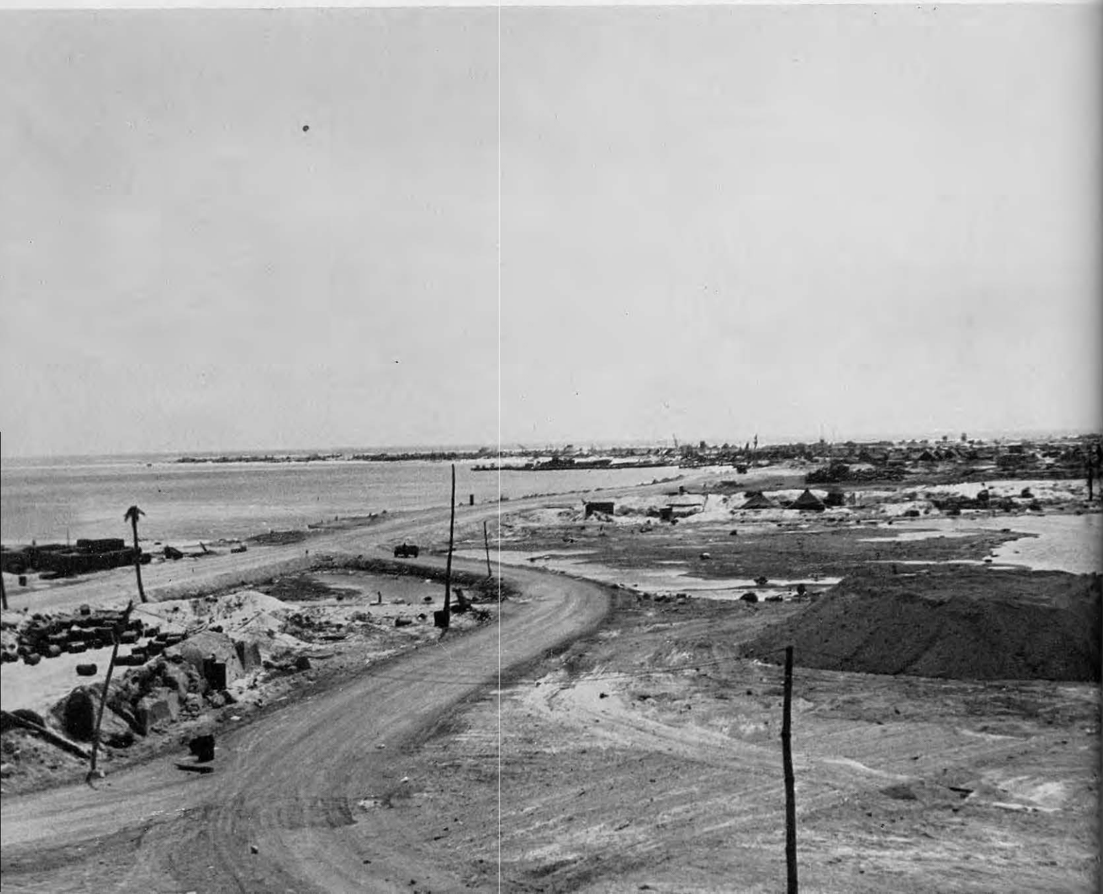
The island of Roi in the distance; Namur in the foreground, connected by the Jap built coral causeway.
