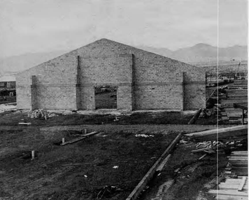
Fire wall in one of the Manana Storage Warehouses.
