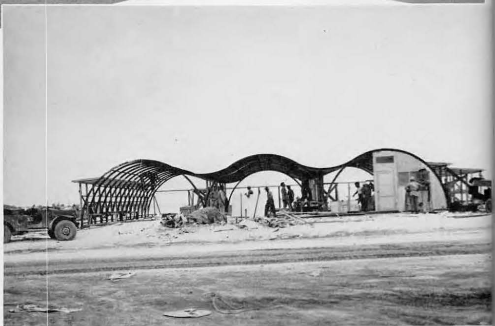
Structural framework of Fleet Officers Clubhouse.
