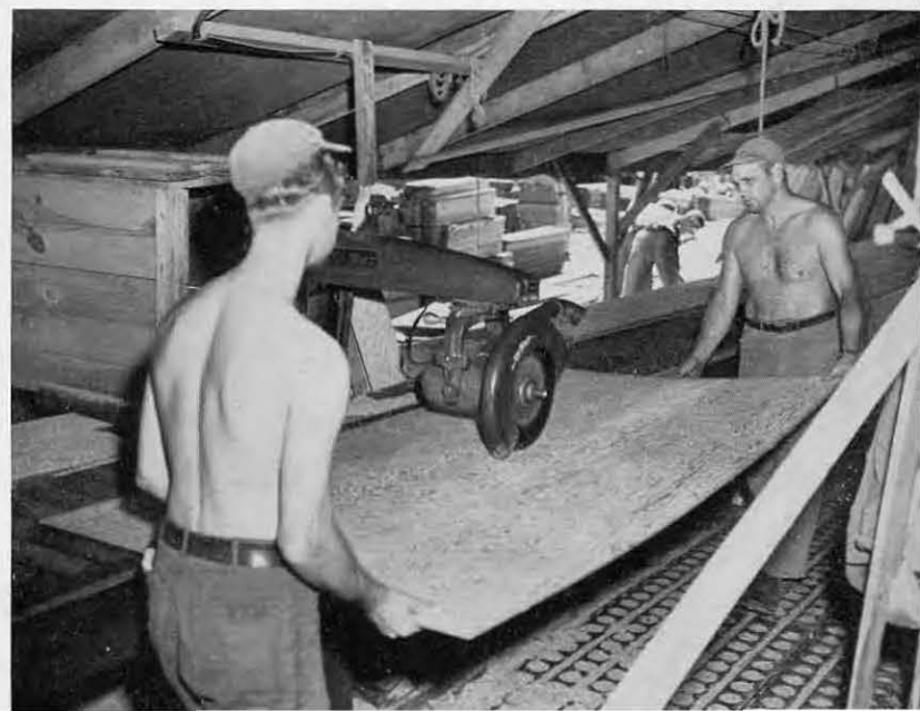
Hendrickson and Kuder at work in the Carpenter Shop.
