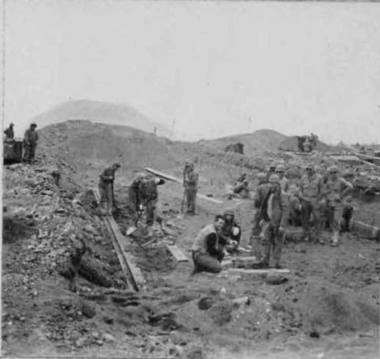
OUR FIRST JOB ON IWO — a torpedo storage dump. This steel and concrete "house" for the deadly projectiles was buried almost to the roof in
