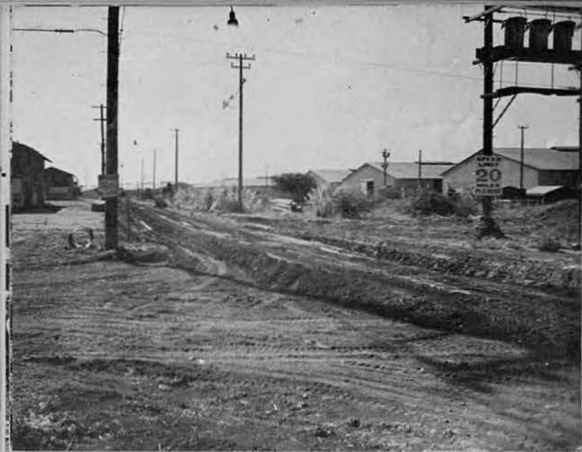
Paving laid by 90th men in the CHA 1-3 Naval Housing areas added a pleasing modern village appearance. Here reside hundreds of civilian workers employed at the nearby Pearl Harbor Navy Yard. In addition to the paving, the 90th Seabees did the highway culvert job shown in
