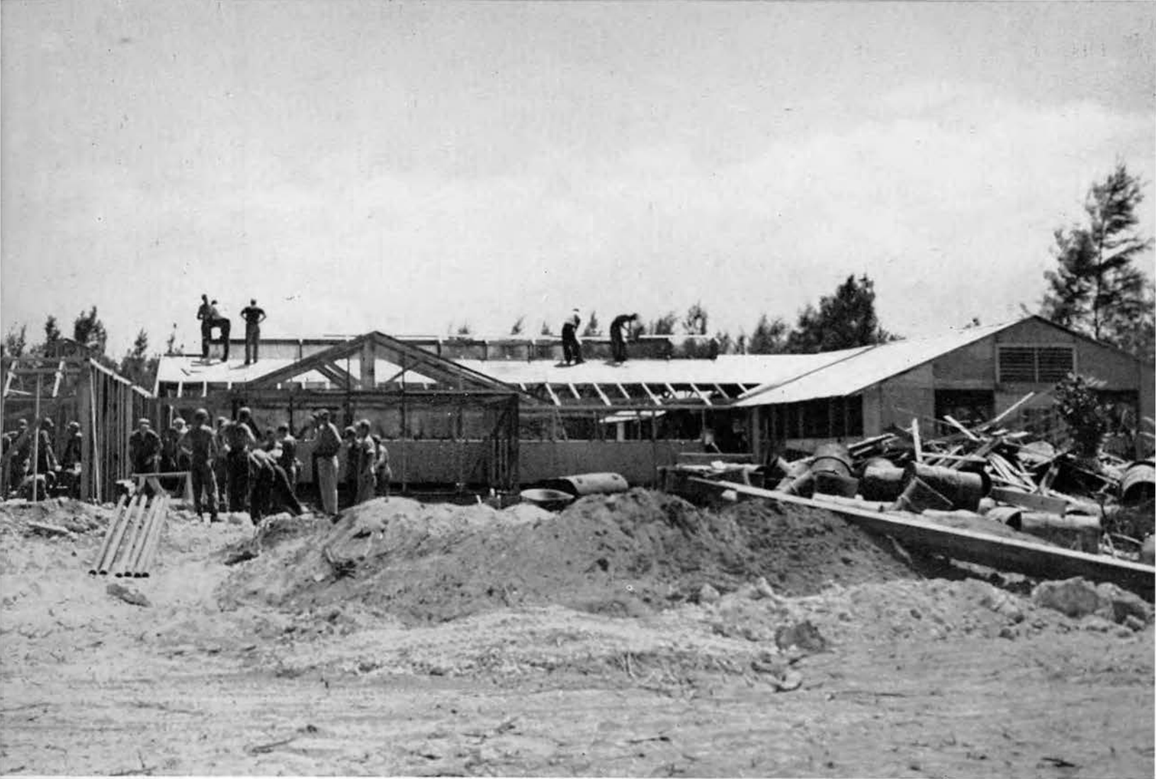
CONSTRUCTION AND MORE CONSTRUCTION. THE DITCHER WAS EMPLOYED BUT WITH LITTLE SUCCESS, BECAUSE THE SOIL WAS OF A SANDY NATURE.
