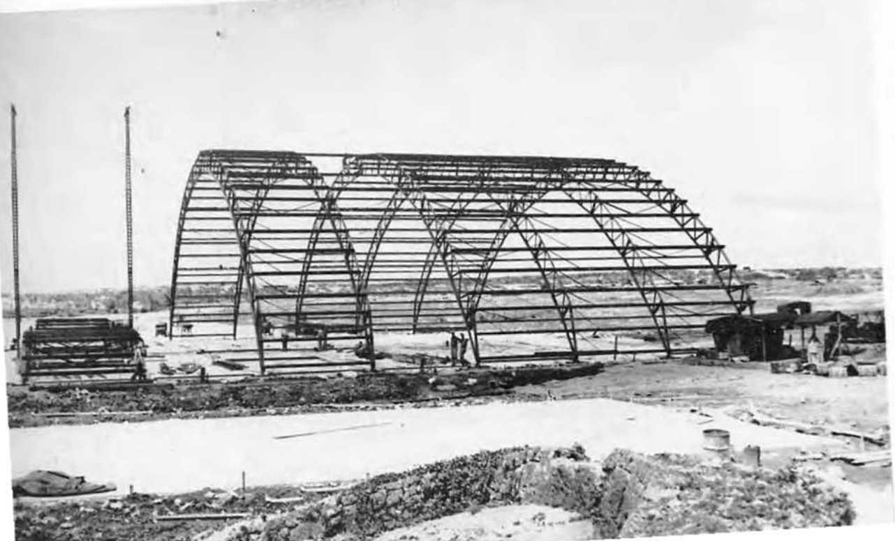
AFTER SECTIONS ARE IN POSITION SEABEES APPLY SCREWS TO SECURE THEM.
