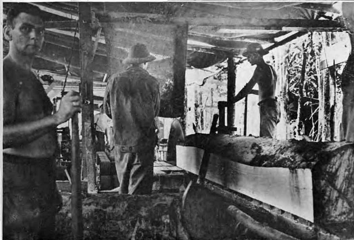
MESSEHALLS, DOCKS, HOSPITALS AND TENT DECKS... THE 82ND'S SAWMILL WAS THE CHIEF SOURCE OF LUMBER SUPPLY FOR THE TREASURY ISLAND GROUP. DAILY PRODUCTION TOTALED ABOUT 8,500 FINISHED BOARD FEET OF LUMBER. THE SAWMILL CREW HAD TO BE ON THE ALERT FOR SHRAPNEL LODGED IN THE TREES.
