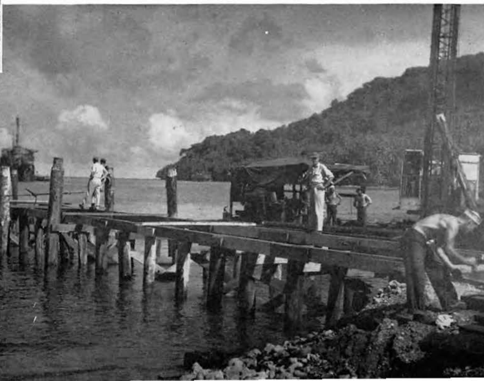
PIER CONSTRUCTION, MONO ISLAND
