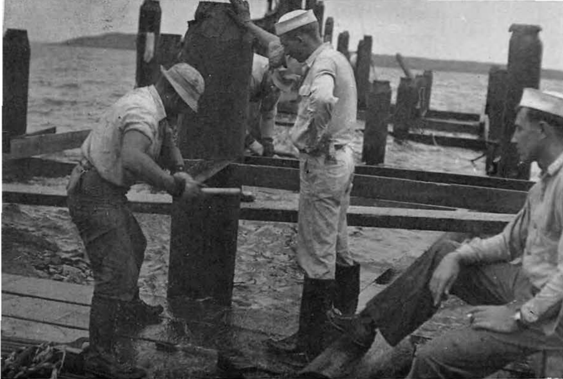
PILES RECEIVE FINISHING TOUCHES
