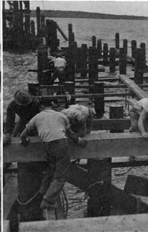
THERE, IT'S IN PLACE.
