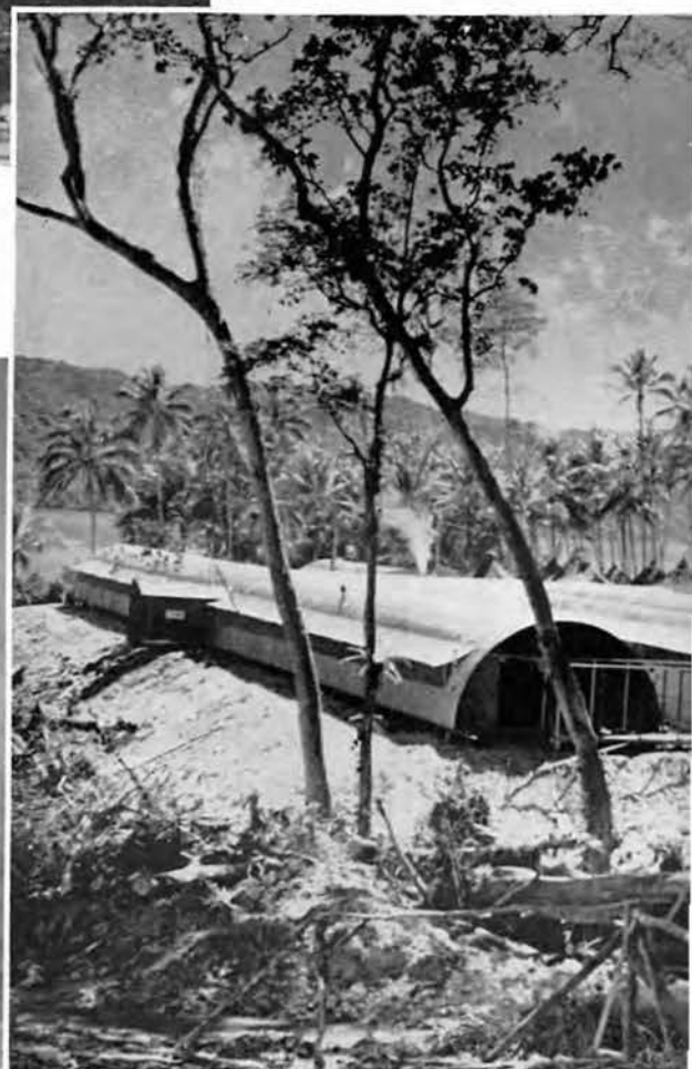
WE CONSTRUCTED FLE
