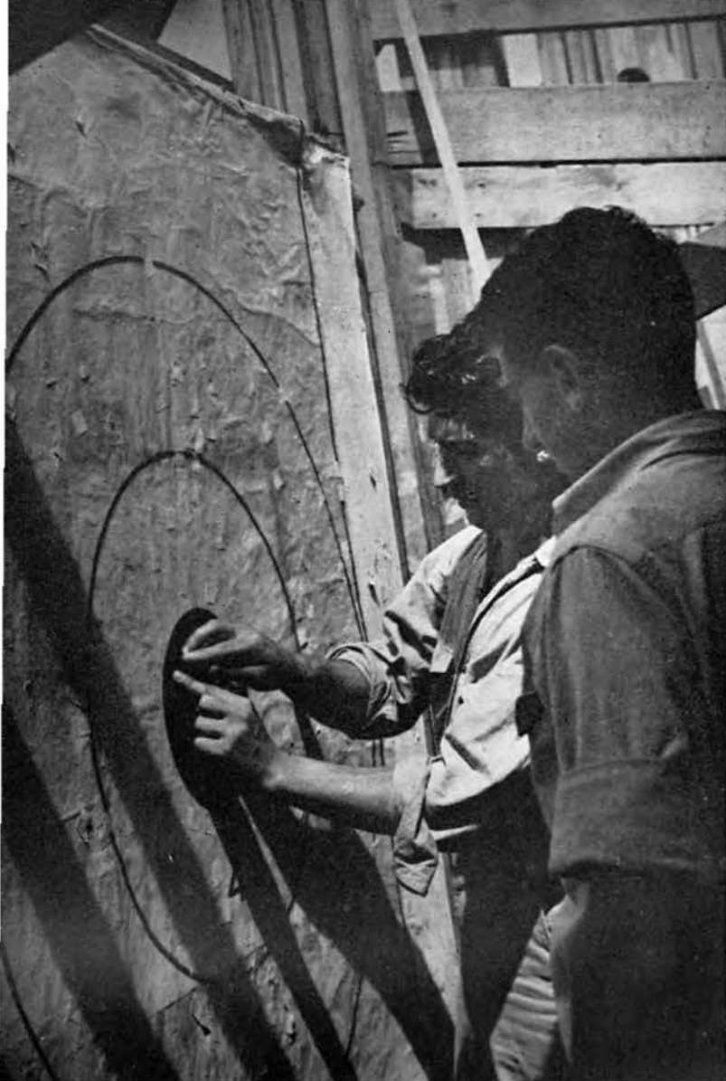
SEABEES REPAIR TARGET AT THE 82ND. RIFLE RANGE.
