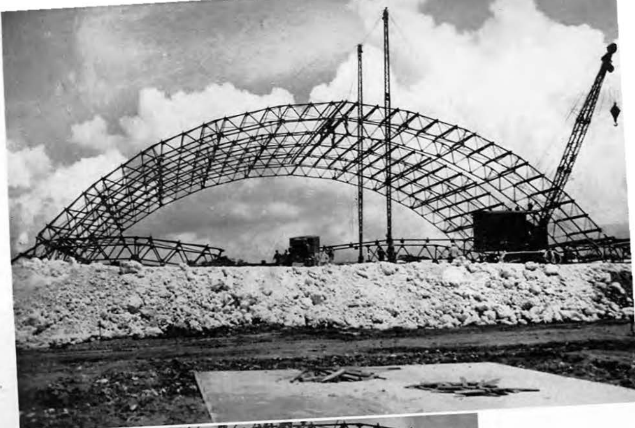
THE CRANE IS USED TO LIFT EACH SECTION INTO POSITION.
