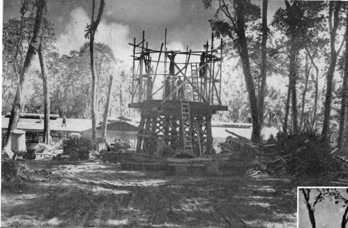
CONSTRUCTION OF WOODEN WATER TANK
