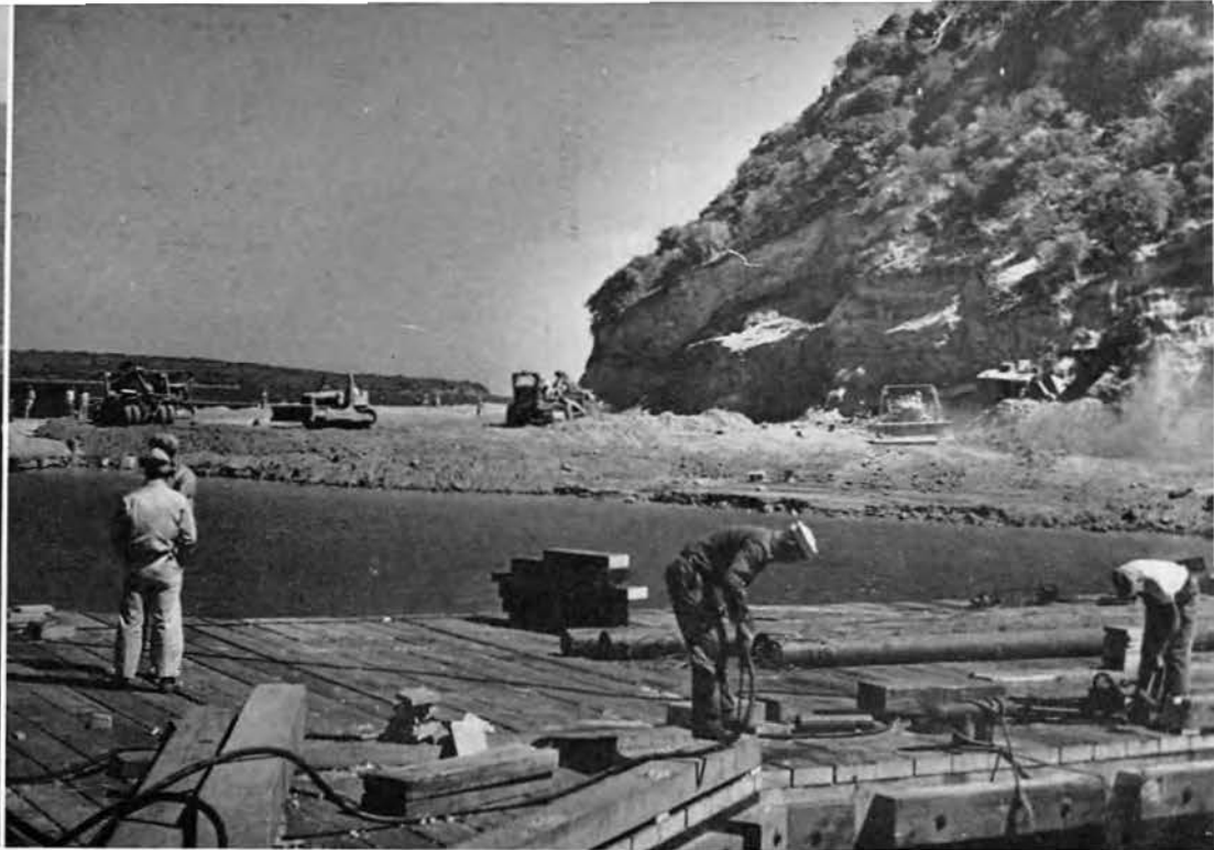
BY HAND AND ELECTRIC DRILL THE BOLTS SINK INTO THE TOUGH WOOD.
