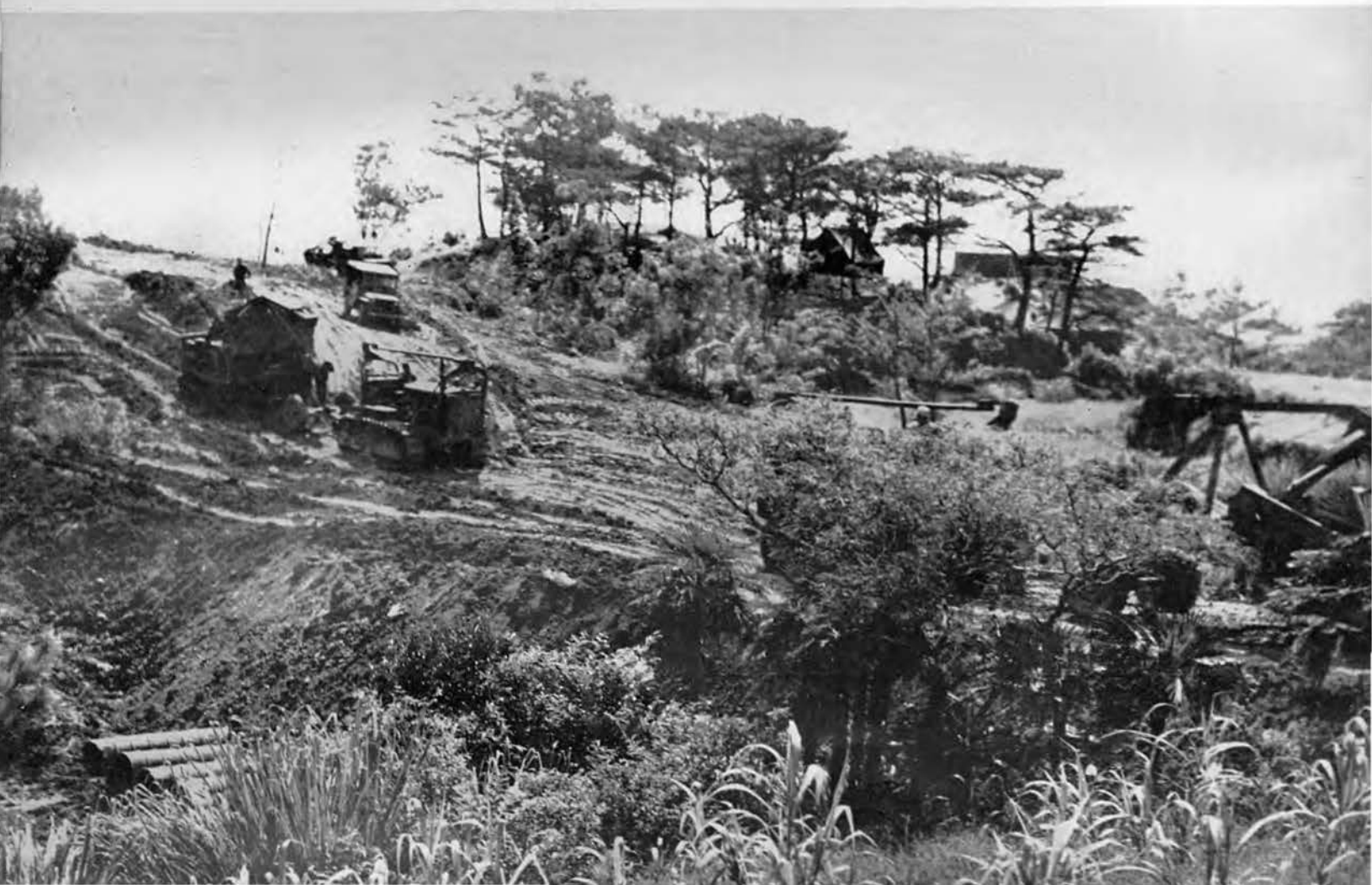
SUCCESSFUL DRAINAGE IS ACQUIRED BY EMPLOYMENT OF EMPTY FUEL DRUMS
