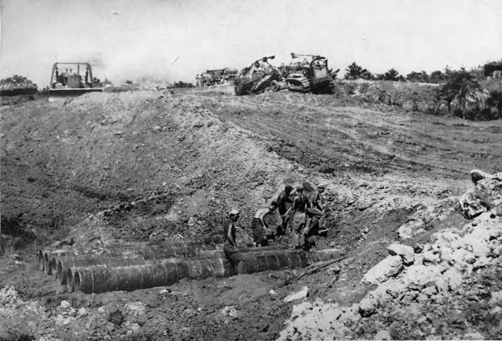
SUCCESSFUL DRAINAGE IS ACQUIRED BY EMPLOYMENT OF EMPTY FUEL DRUMS
