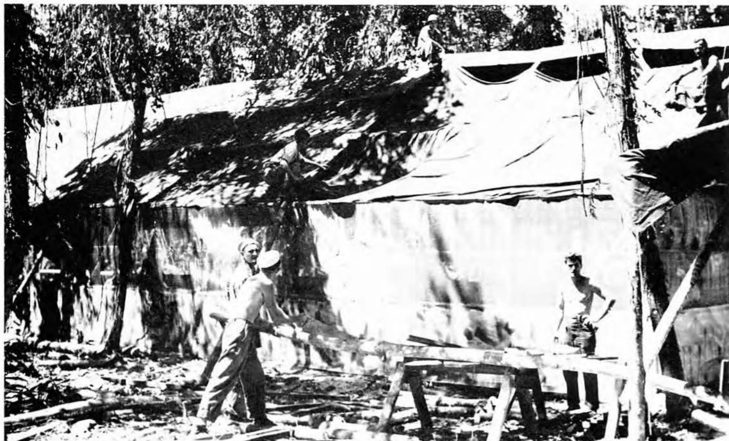
77th Mess Hall Going Up
