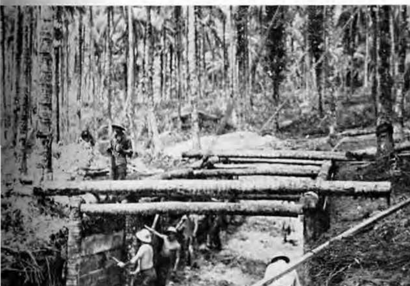
Framing underground surgery
