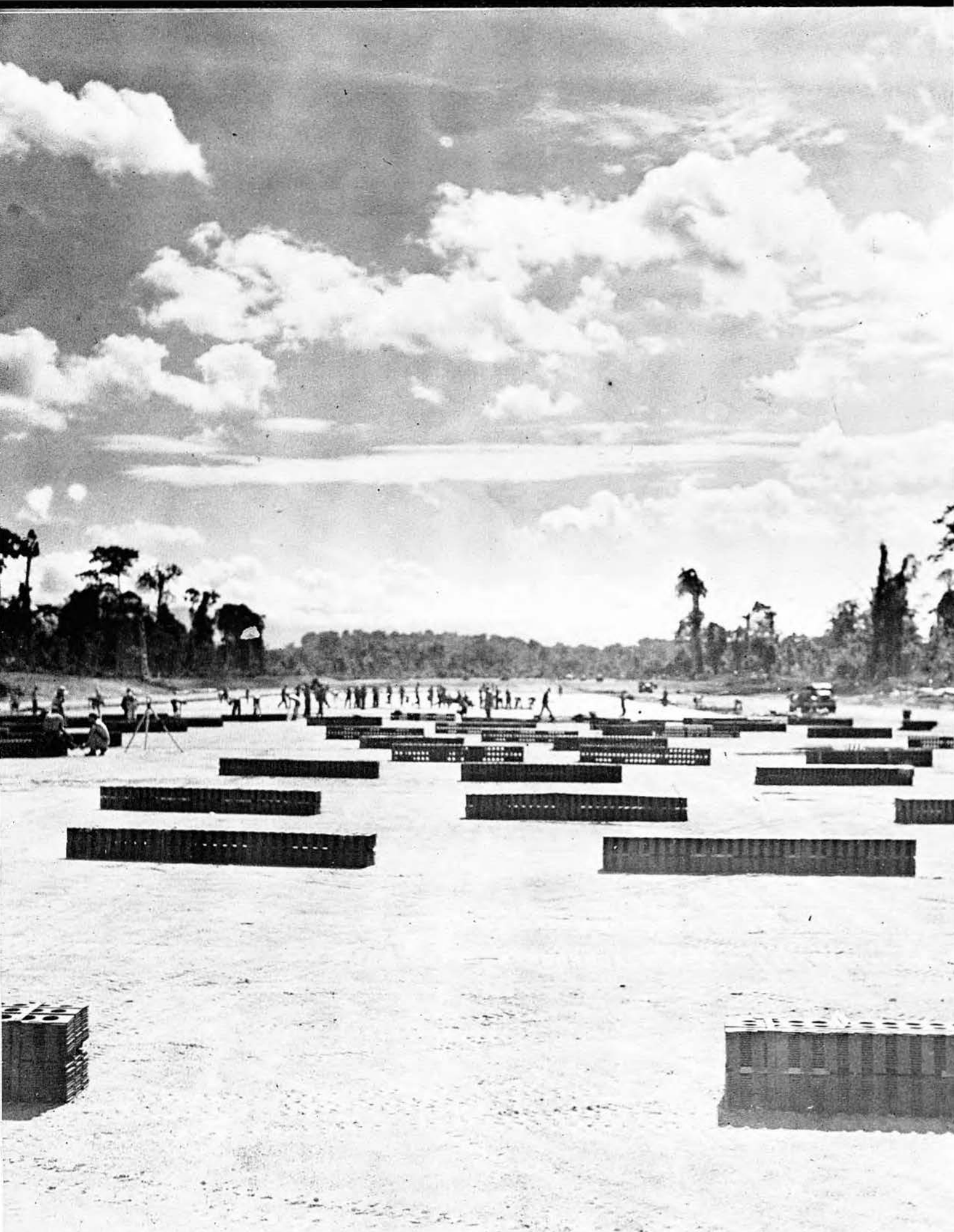
Spreading a Carpet of Steel
