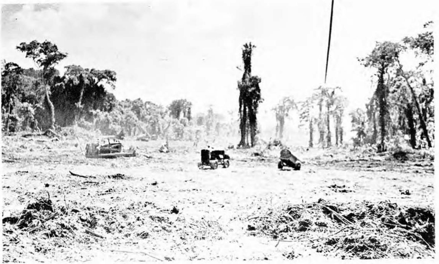
Start of Clearing
