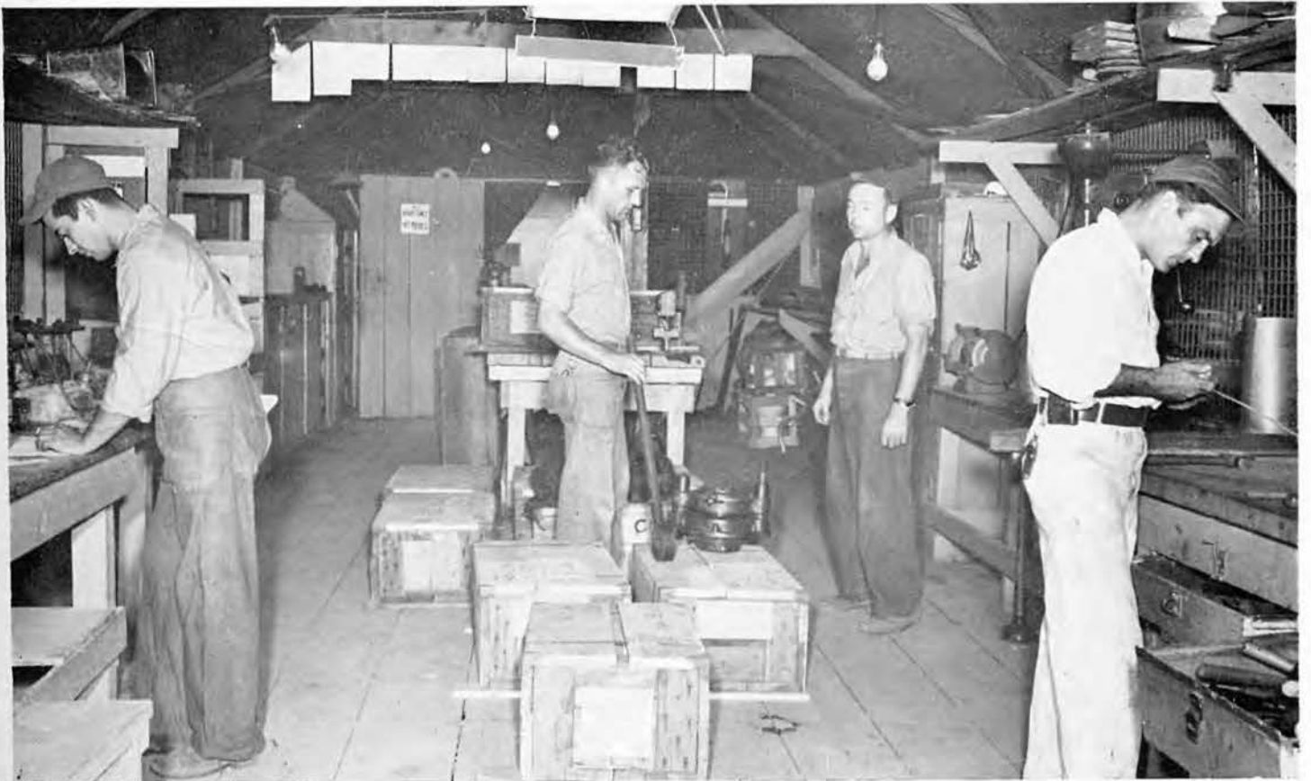
Our Plumbing and Metal Shop
