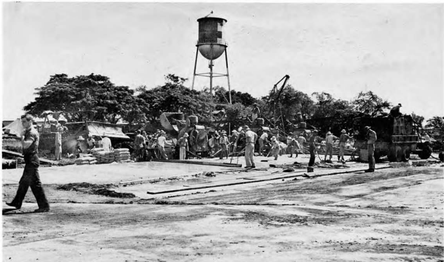
Cement Deck Going Down
