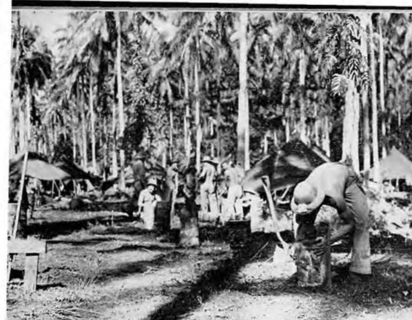
Setting foundation blocks for hospital
