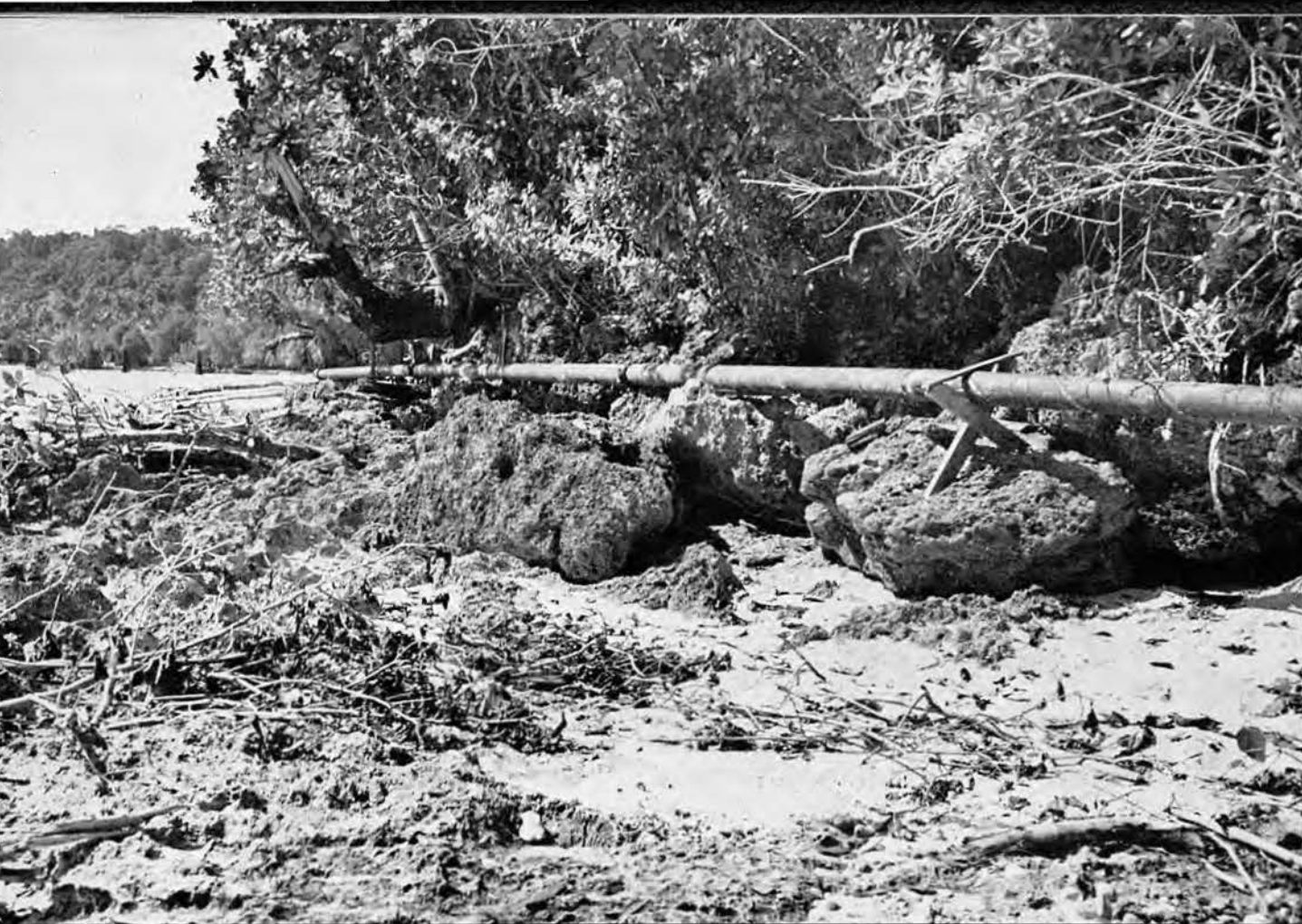
Pipeline Along Shore
