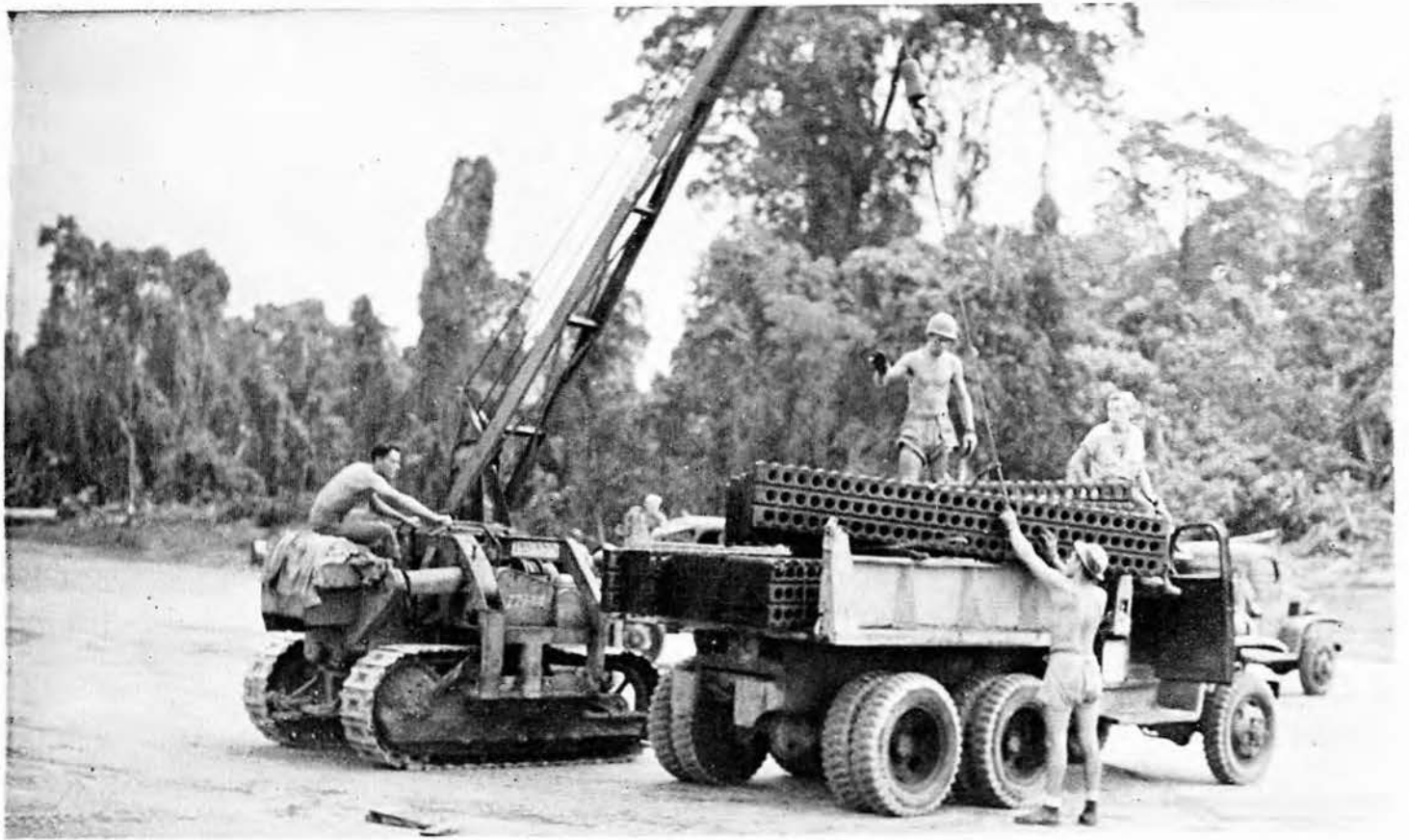
Unloading Pierced Planking
