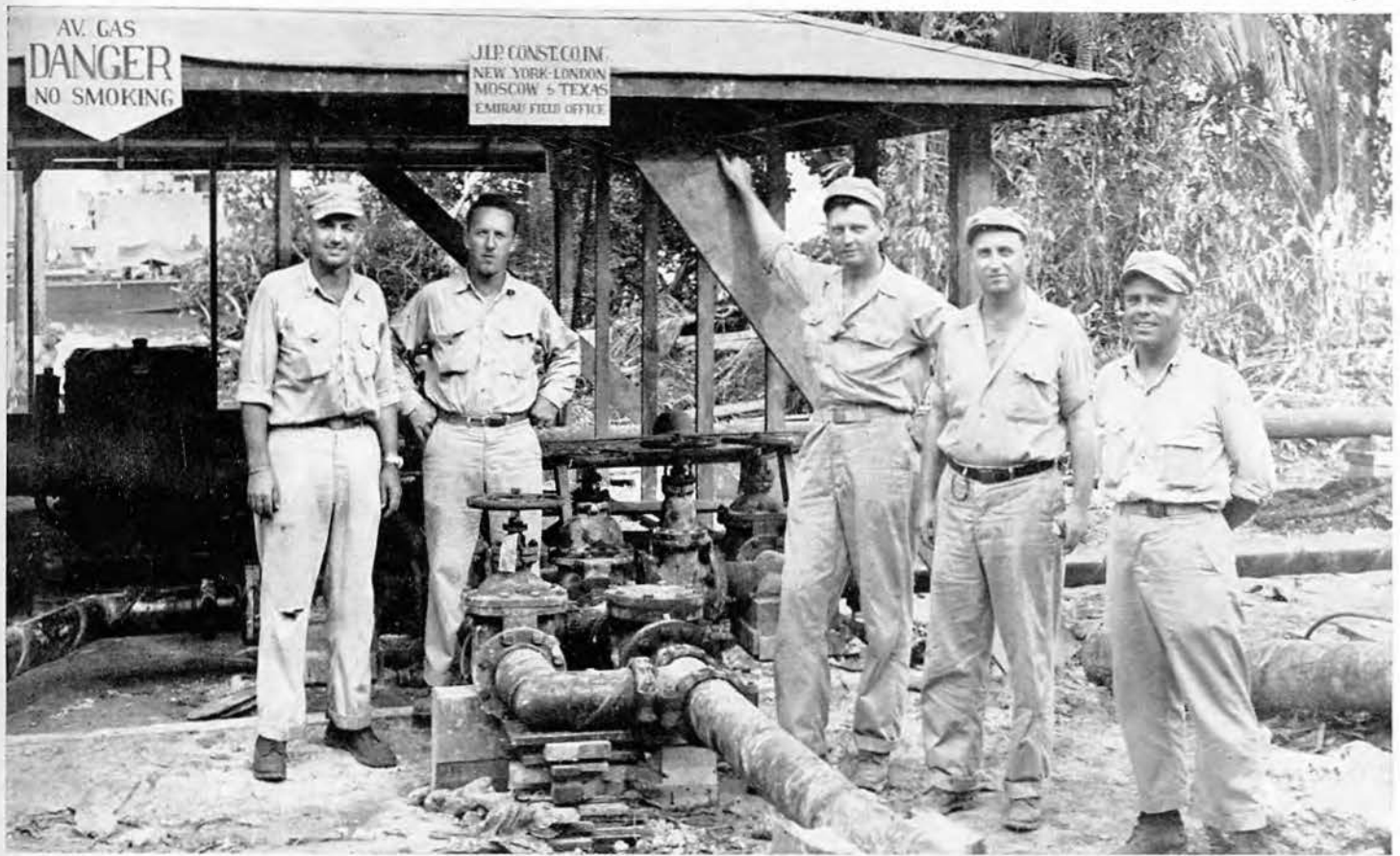
Hamburg Bay Pump Station
