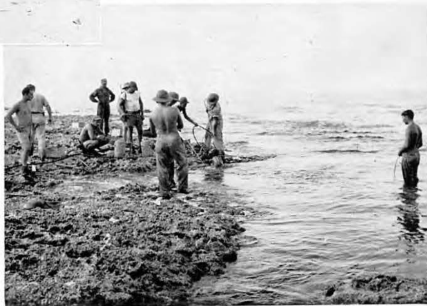
Setting Dynamite Under Water-Pilots' Pool
