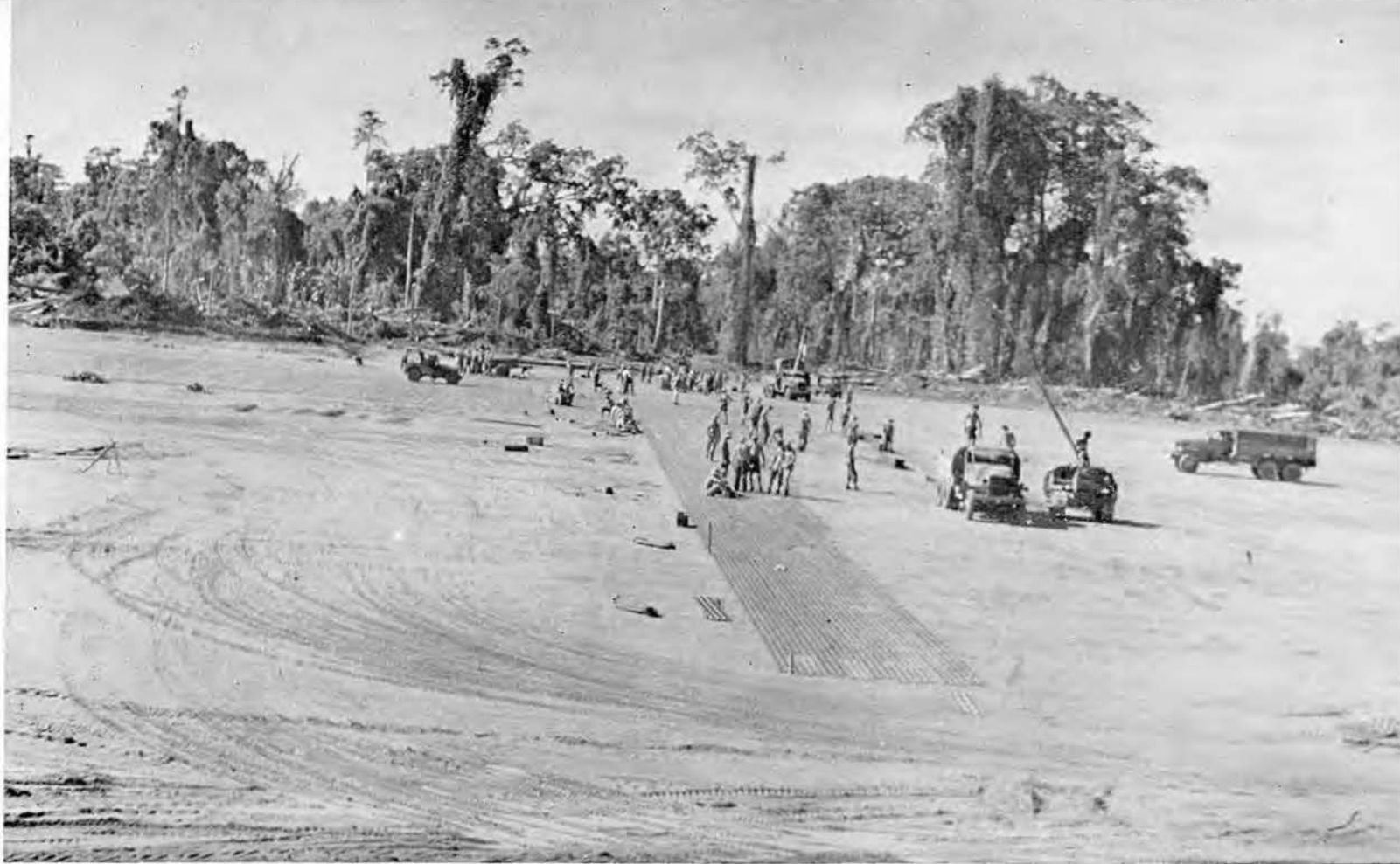
Apron Under Construction
