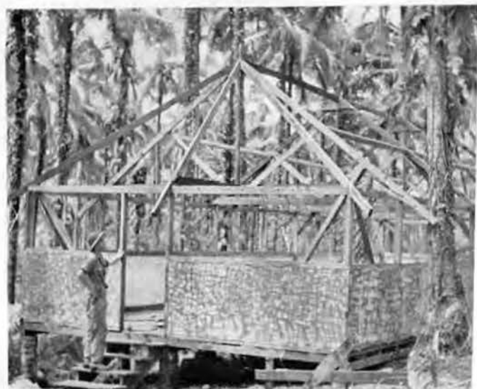
Ready for tarpaulins
