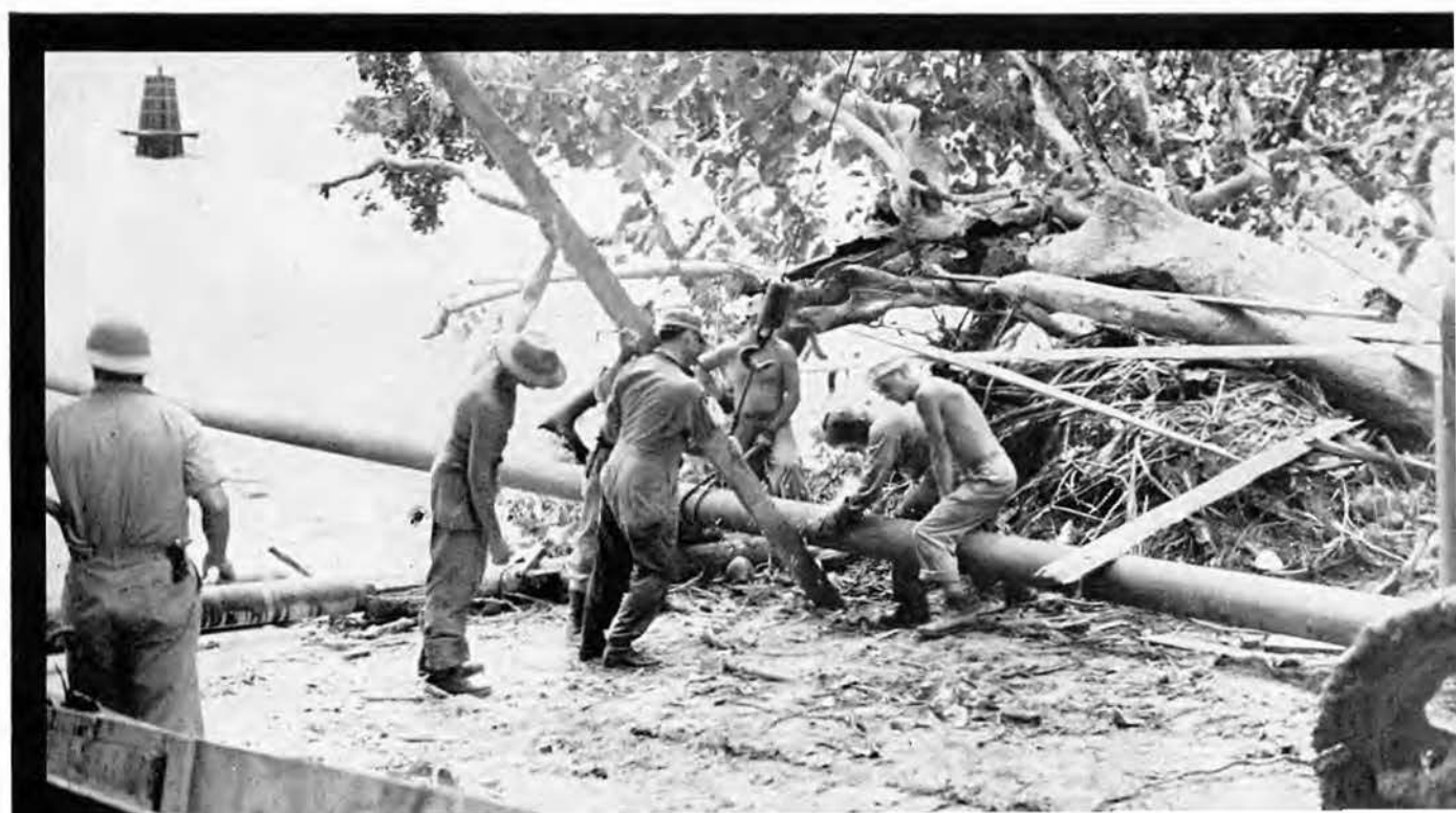
Welding Sea Line
