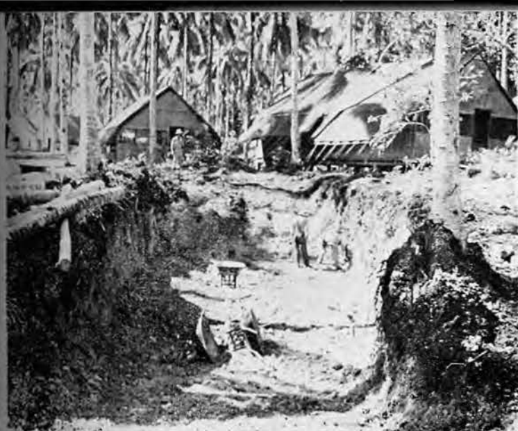
Excavation for underground surgery
