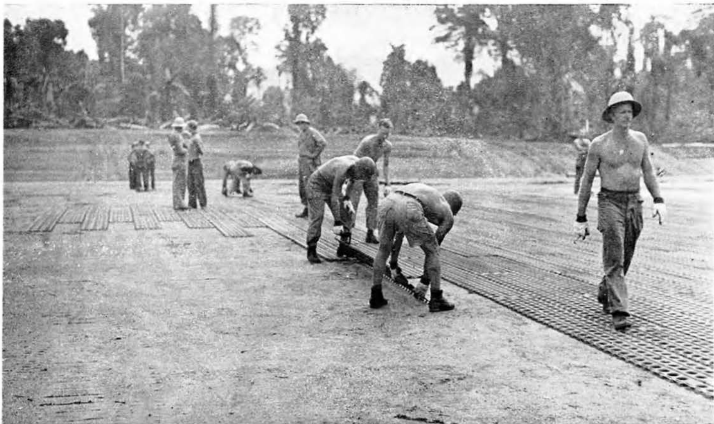
Laying Pierced Planking
