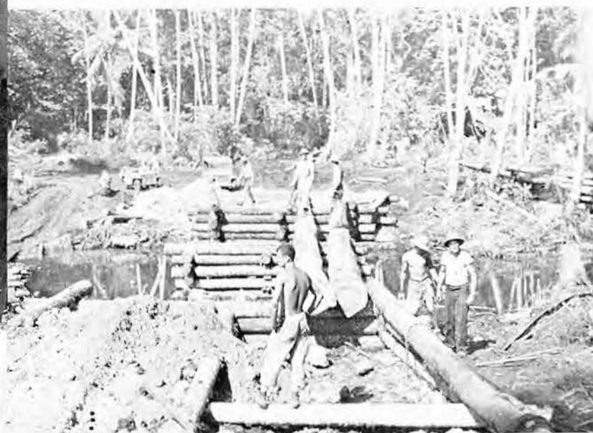
At left, reading from top to bottom: Temporary bridge—Biporo River. Beginning second bridge. Below, left: Open to traffic; right: Sawmill on Juno River.
