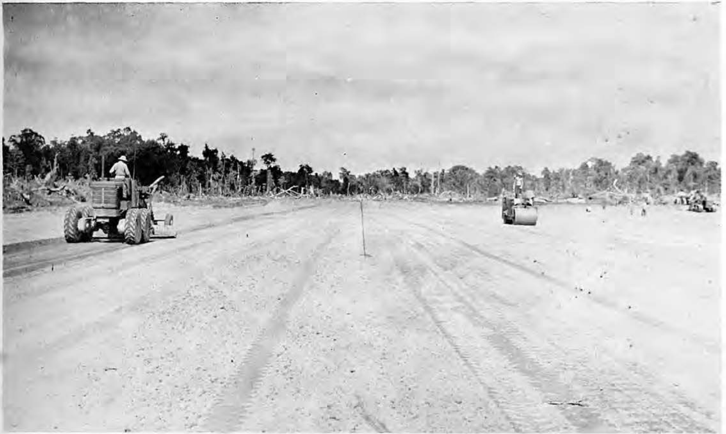
Rolling and Grading Extension
