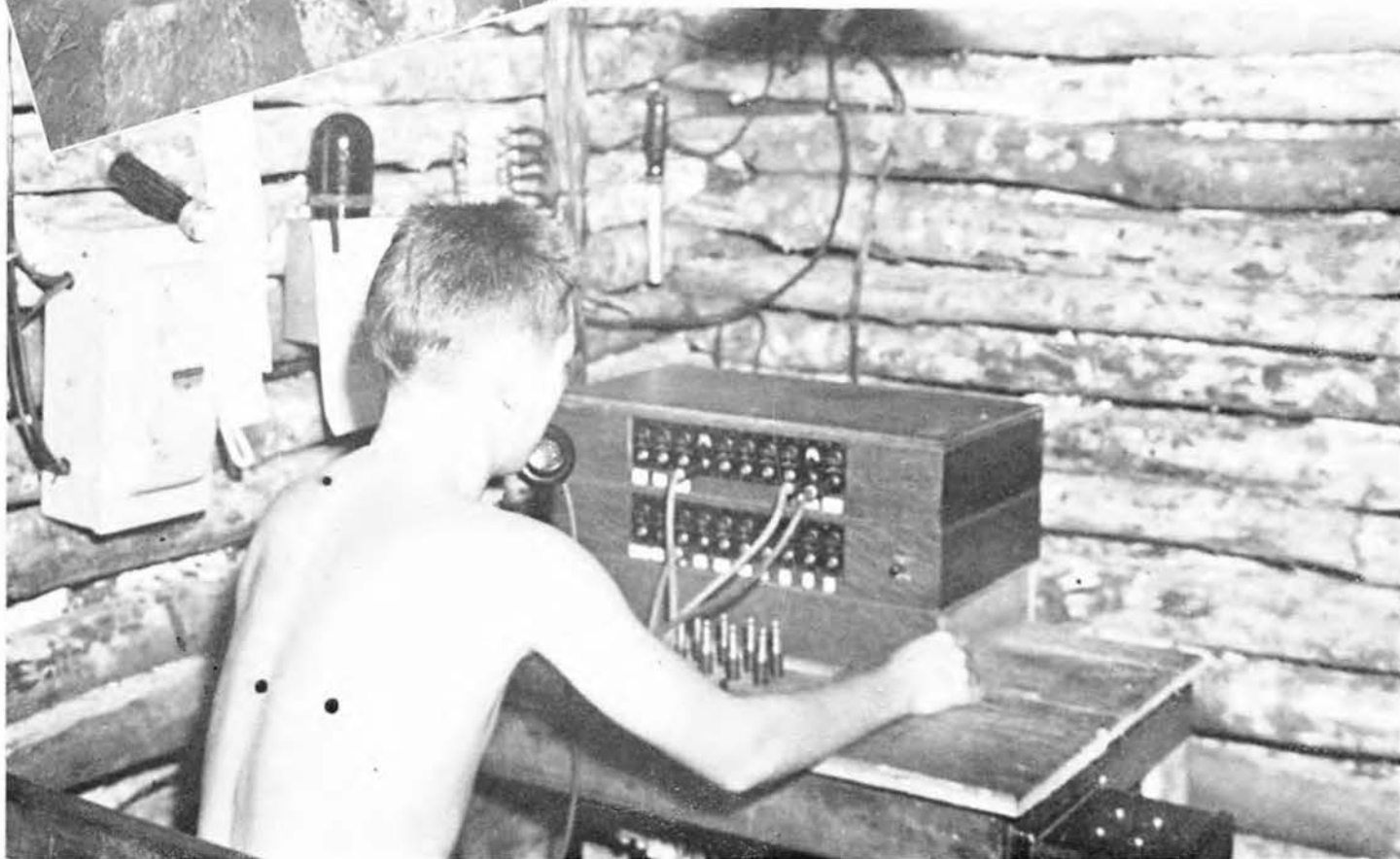
Underground Communication Center—Switchboard Built by 77th
