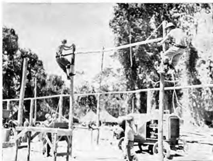
Framing 77th Machine Shop
