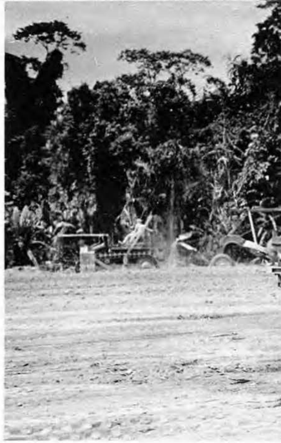
Compacting the Volcanic Ash
