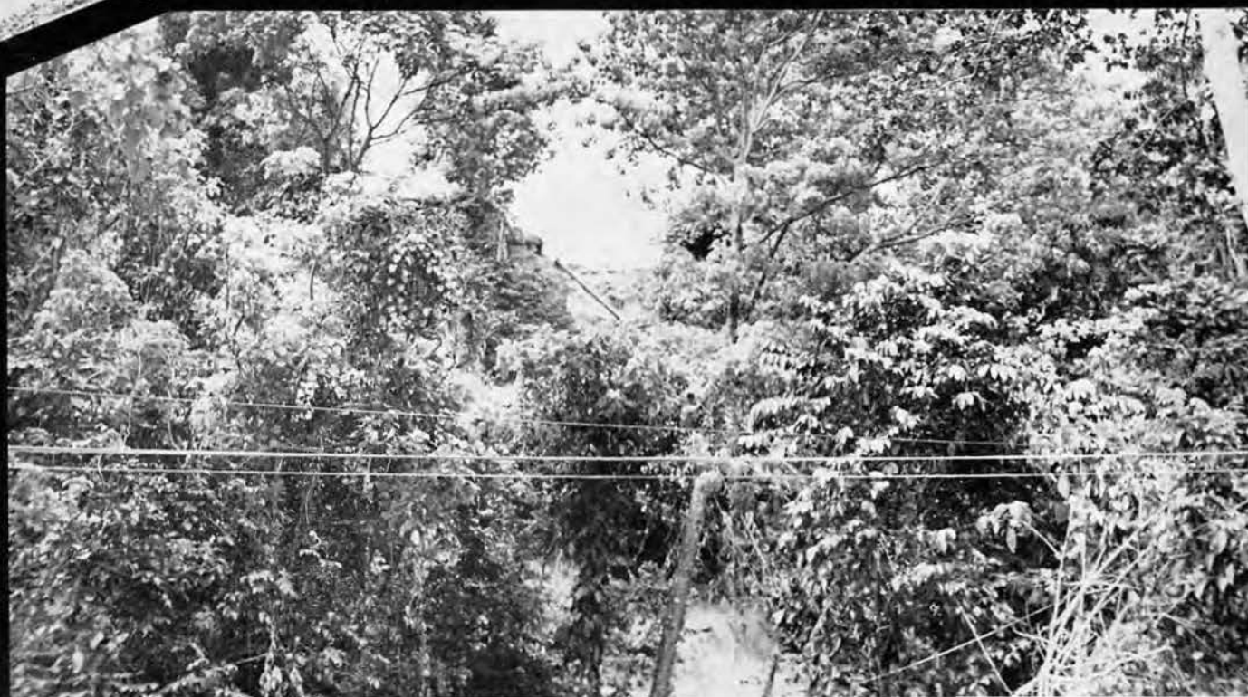
Pipeline Going Over Hill
