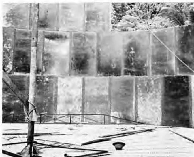
Tank Sections Going Up
