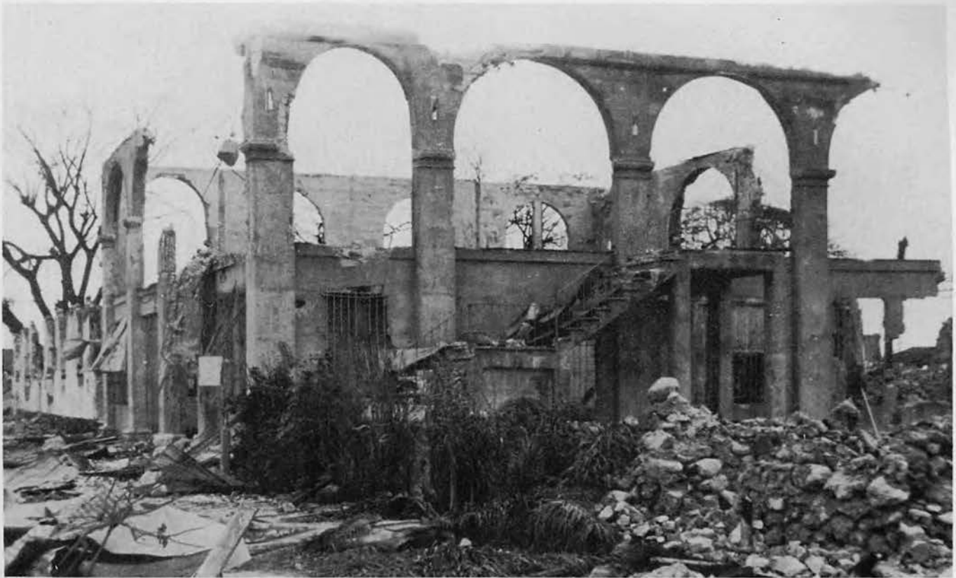
The ruins of Agana. This photograph of the former Court House and Bank of Guam, and the views immediately following, show the effects of the U.S. naval bombardment. This pre-invasion softening, which virtually leveled the city, took place in July, 1944.
