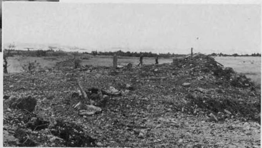
The smoke has cleared—the house has gone.
