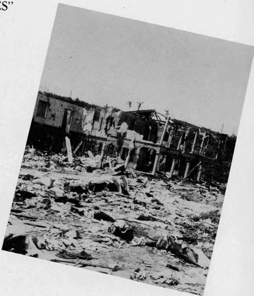
Principal building in the village of Agat.
