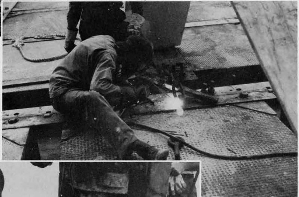
Right: Arc welding the chain in place.
