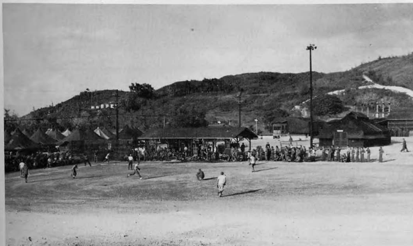
An action shot taken on the 76th Battalion's ball field. "C" Company Area and the Piti Power Plant can be seen in the background.
