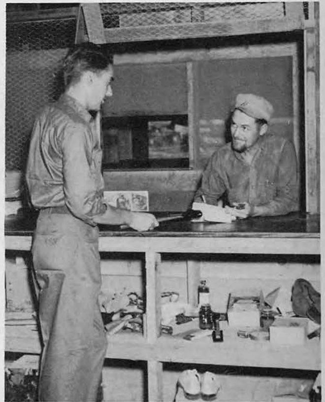
Issue of tools and small equipment for 1200 construction men was a job that required tact and ability. A. D. Sherrill issues one of the many tools at the warehouse. D. B. Joy is the Seabee signing the chit.
