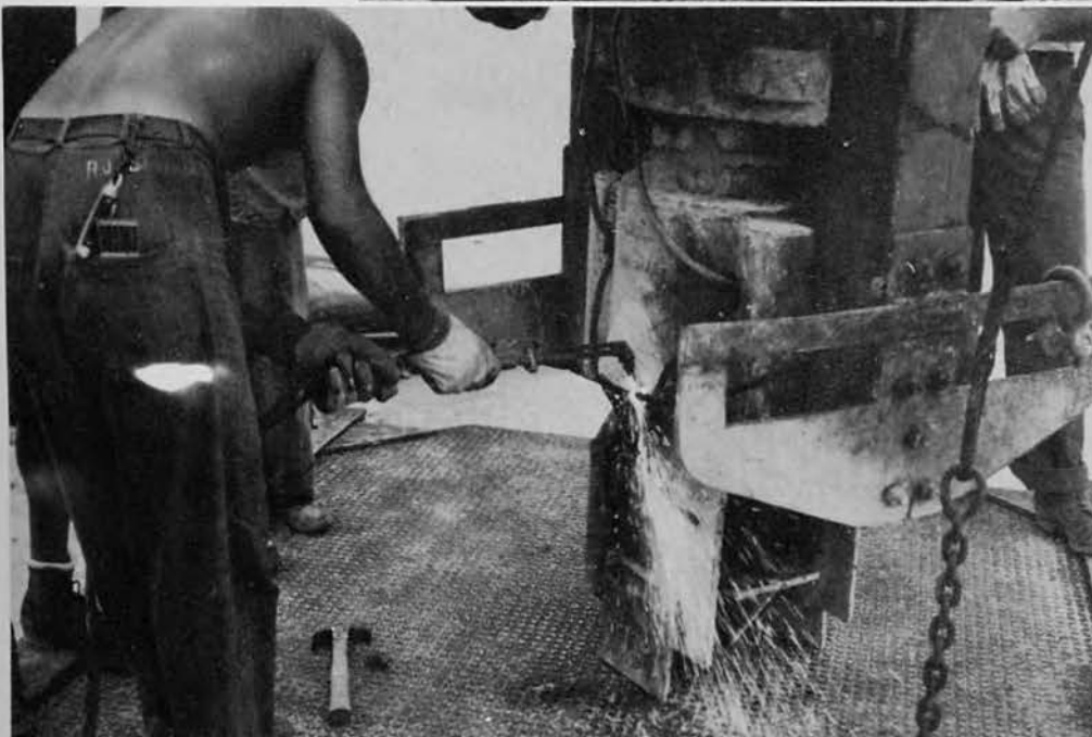
Left: Emergency repair on the pile-driver head-block.
