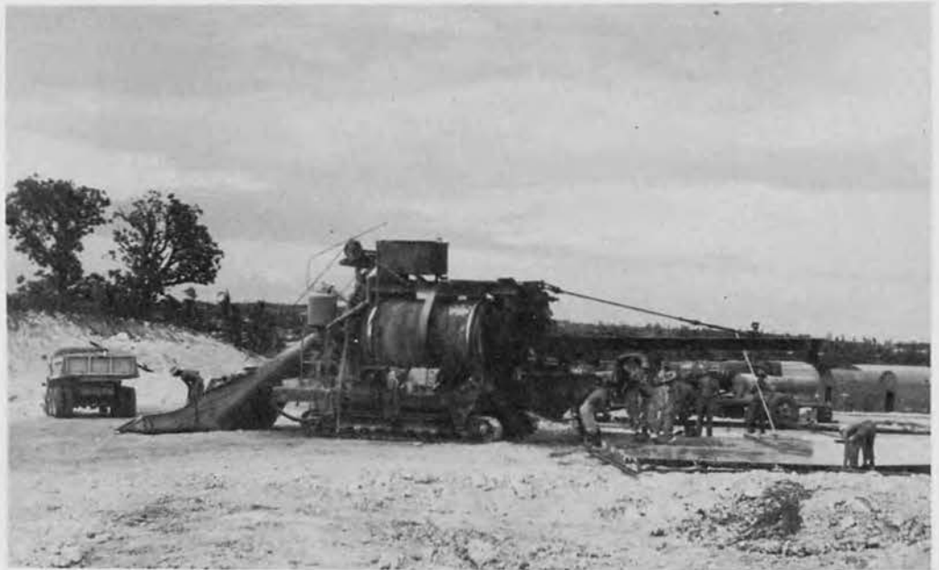
Pouring the decks for 40 by 100 storehouses with the big 27-E.
