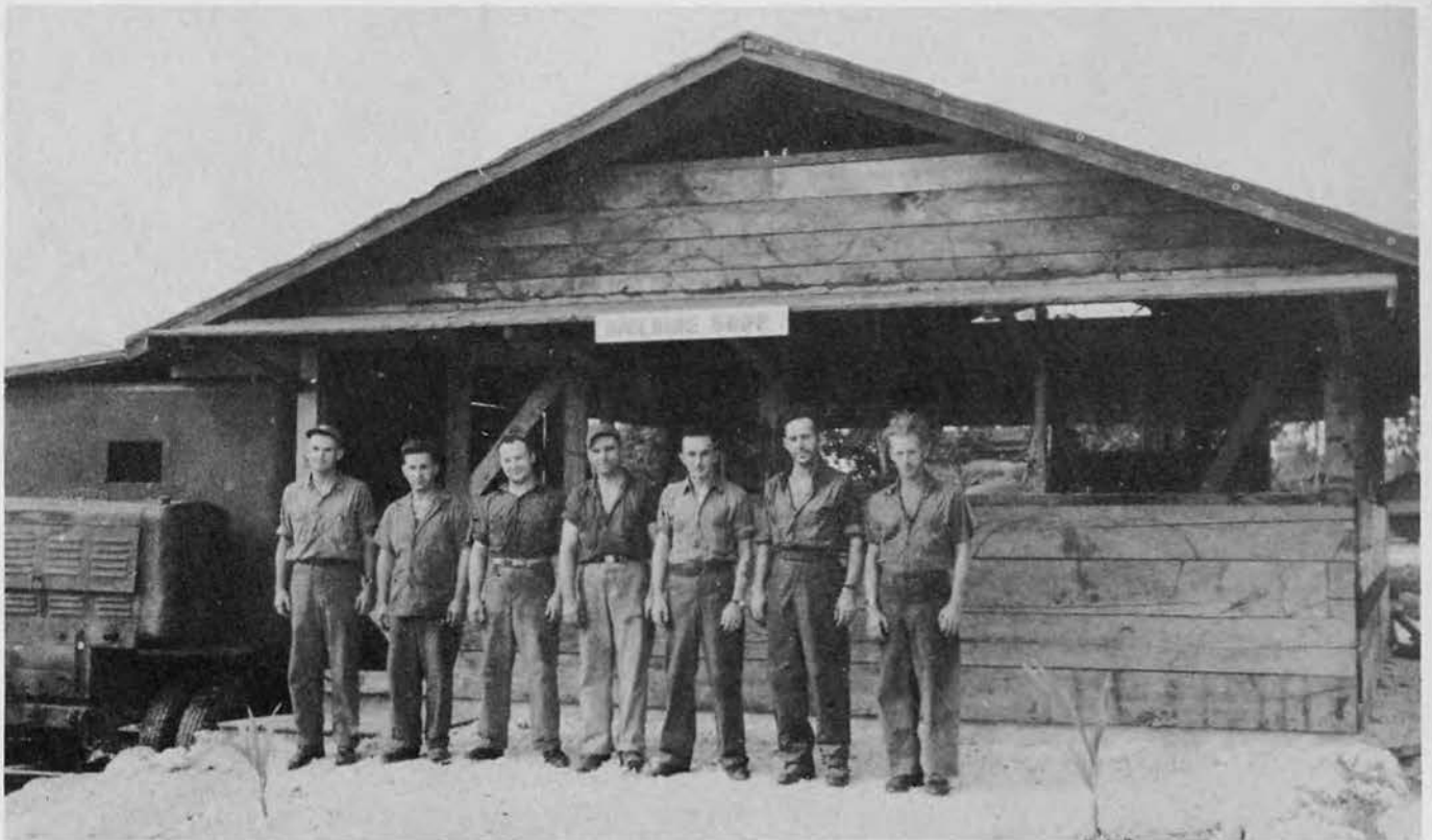
Exterior view of the battalion Machine Shop is shown in photo above. Left to right: Lt. (jg) H. C. Hepting, in charge of battalion shops. T. Lima, J. M. Barbier, C. Williamson, V. J. Zanelli, P. J. Gustis, and M. B. Kramer.
