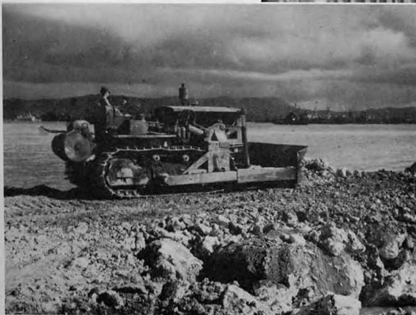
Left: Dozer builds a turn-around.
