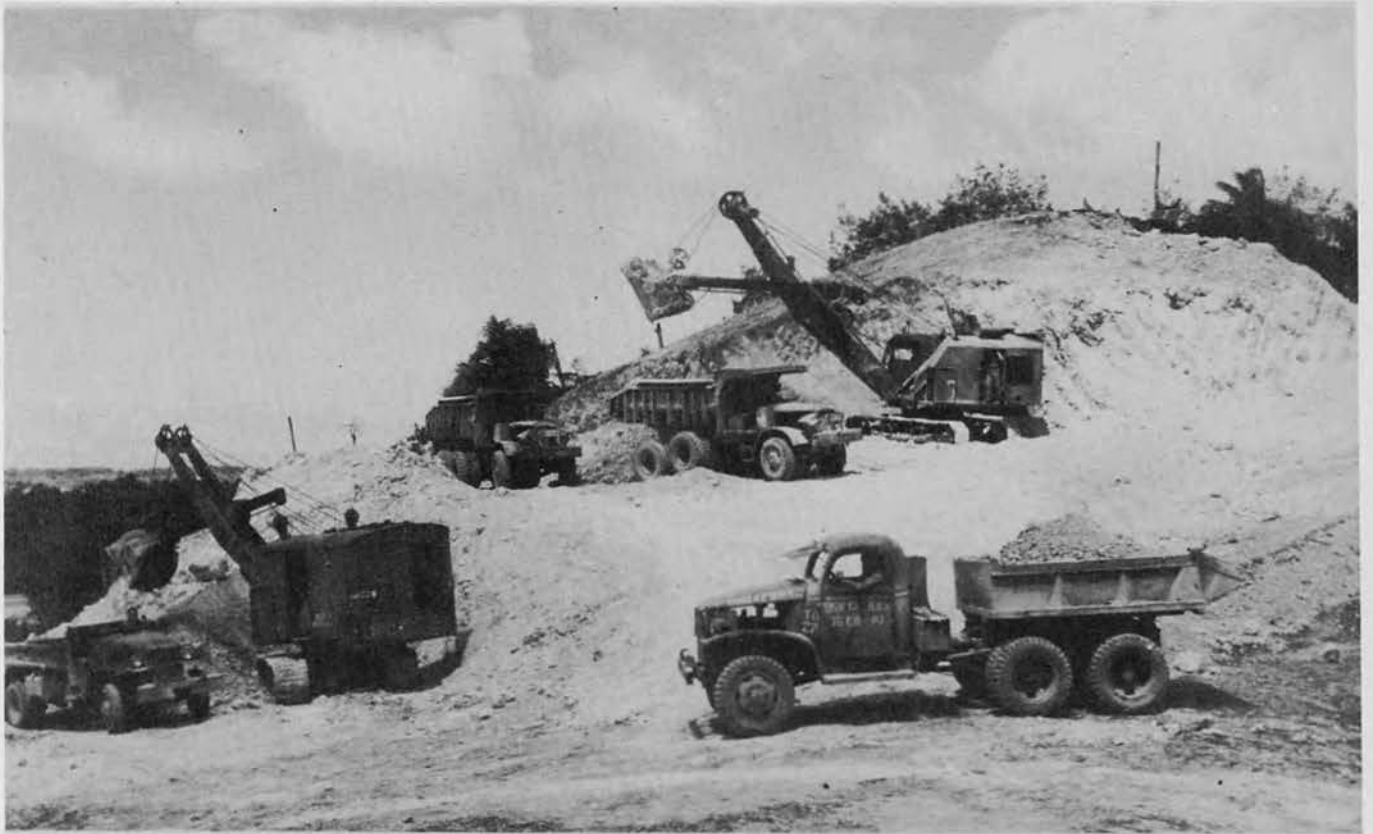
The Martinez coral pit. Two shovels turning out high-grade fill by the dipper full.
