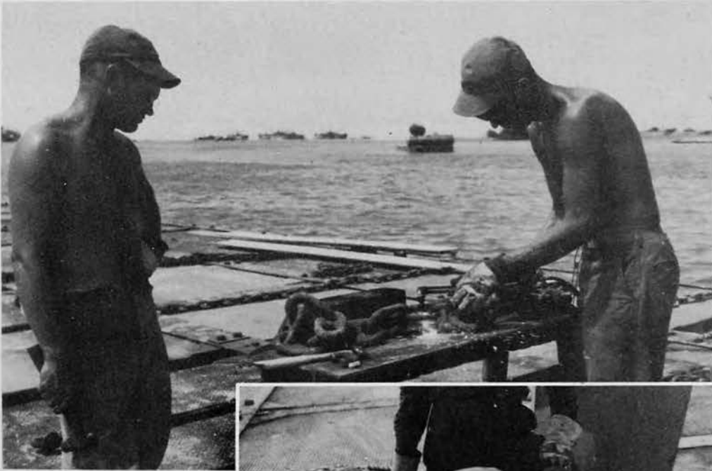
Left: T. N. Abbot and E. J. Broussard prepare flexible chain connection.
