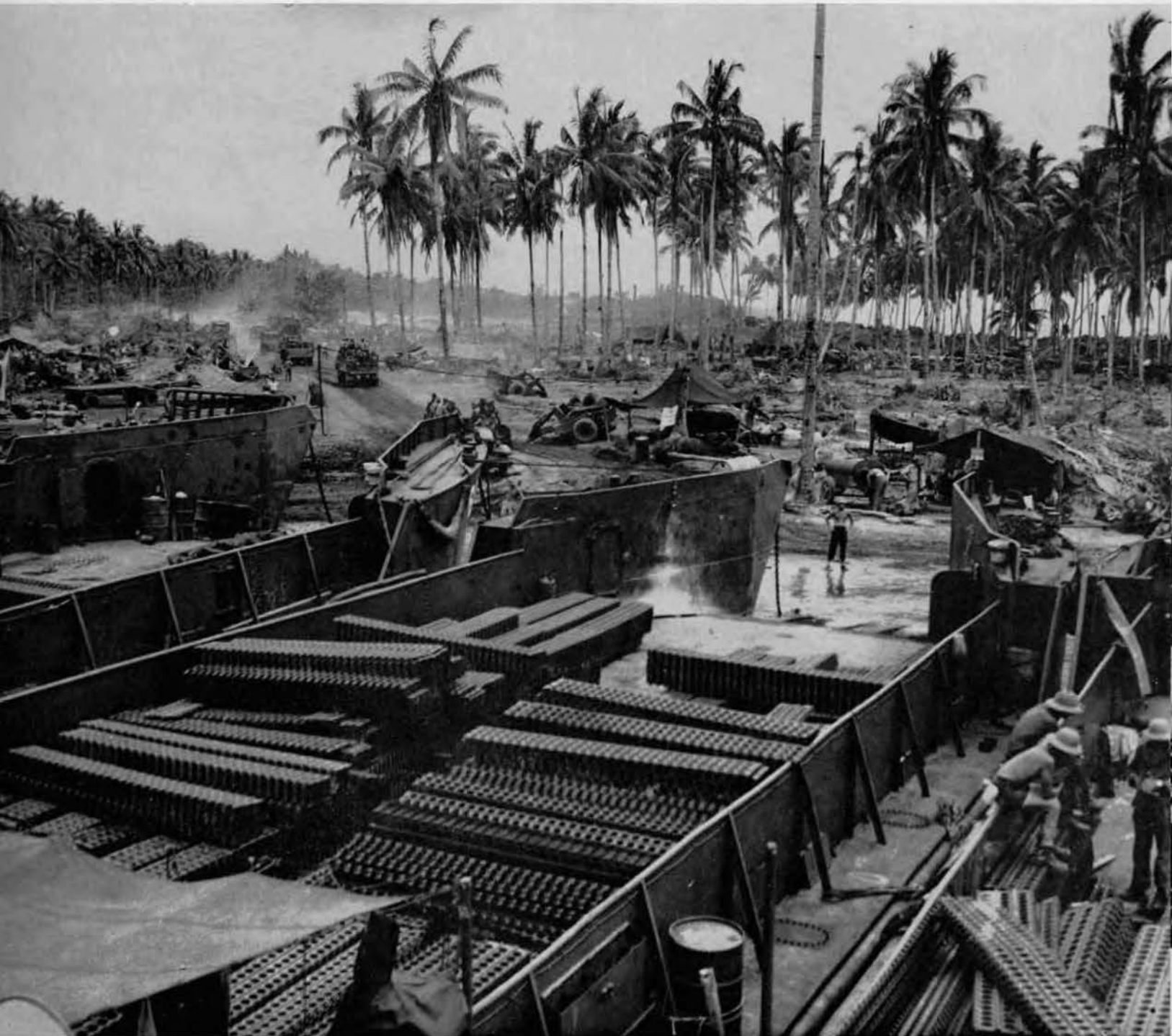
Seabees unload their supplies and equipment, to clear the jungles, roll the airport and put the metal strips together to form an airfield. The scene is in the Bougainville jungles.
