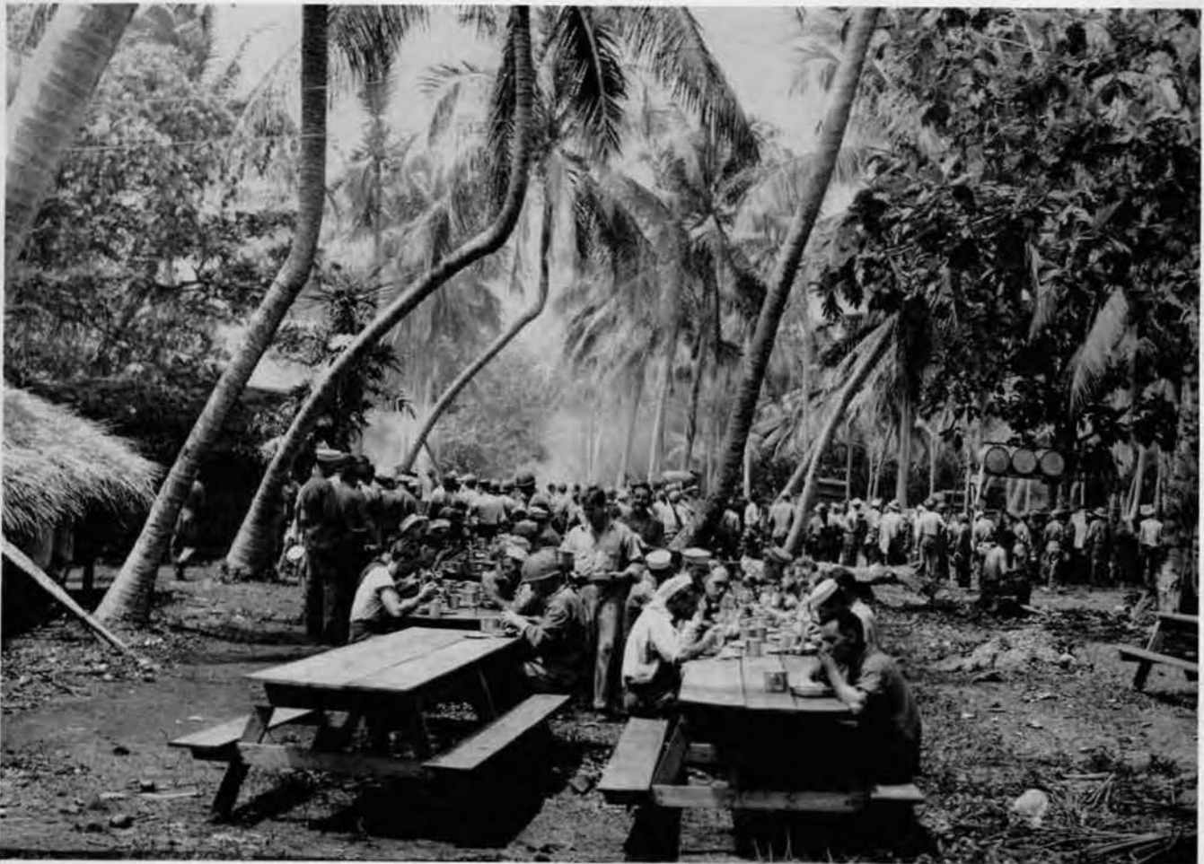
The first week following the landing at Espiritu Santo was much like the bustle of the first day, but gradually a semblance of order began to emerge. Messing facilities were established, and later mess halls were built.
