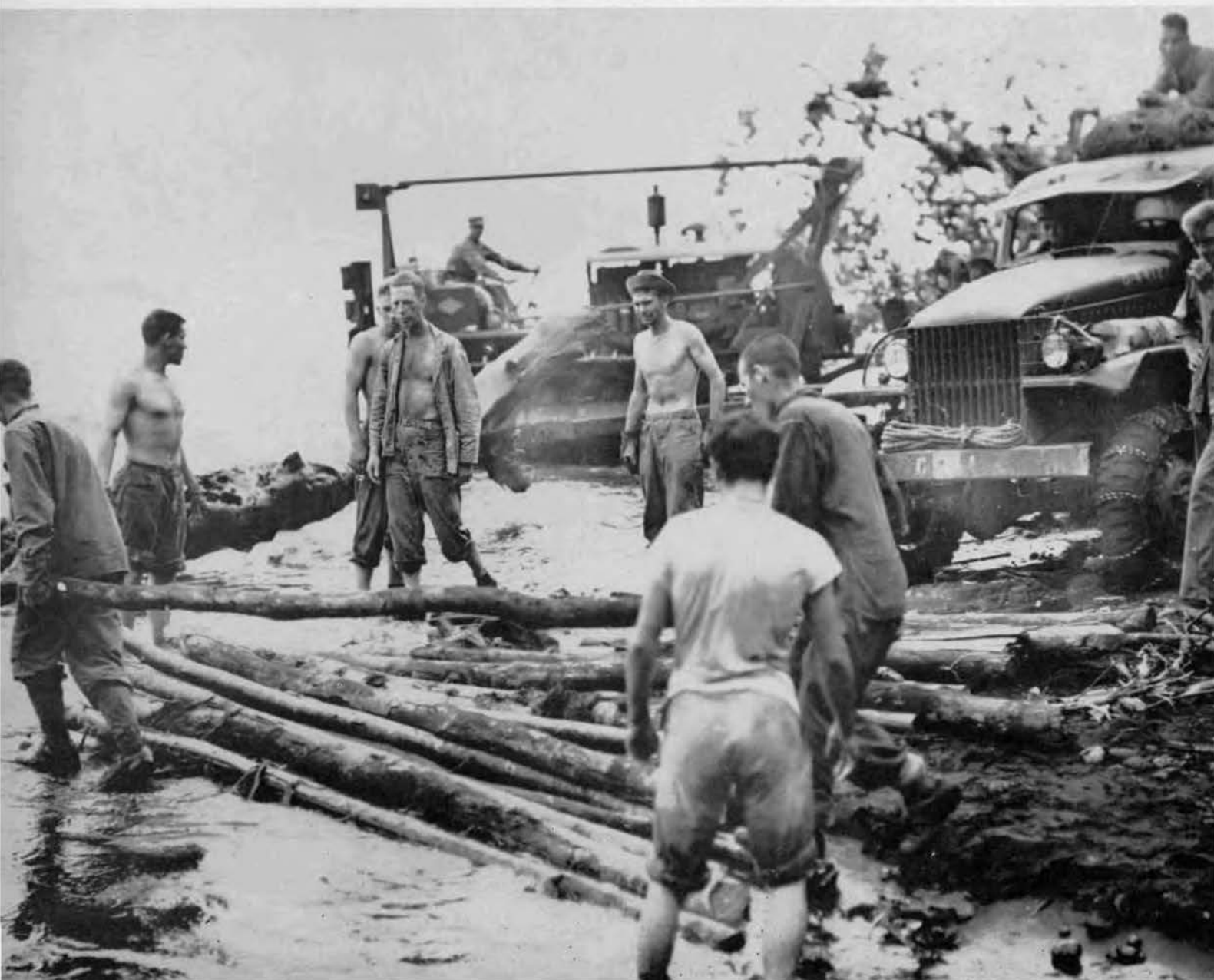
Trees and logs are put in place by Marines and Seabees for a bridge across a jungle stream on New Britain Island.
