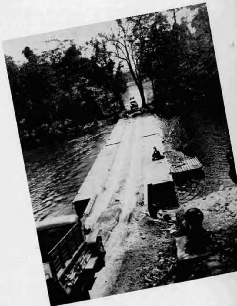
Steel runways connect two pontoons to form a hastily constructed span.
