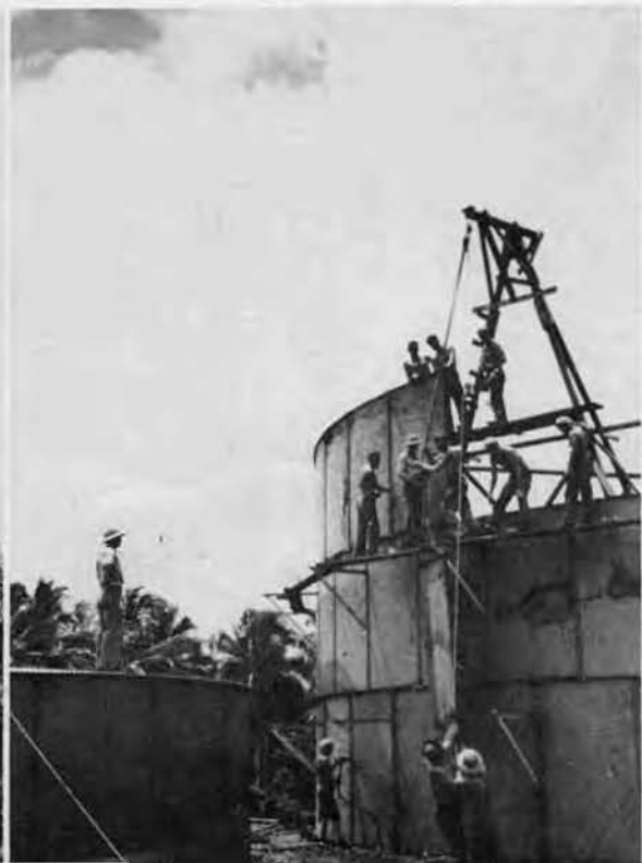
Up goes another sheet of steel as this piece on construction rapidly takes on the appearance of a tank.
