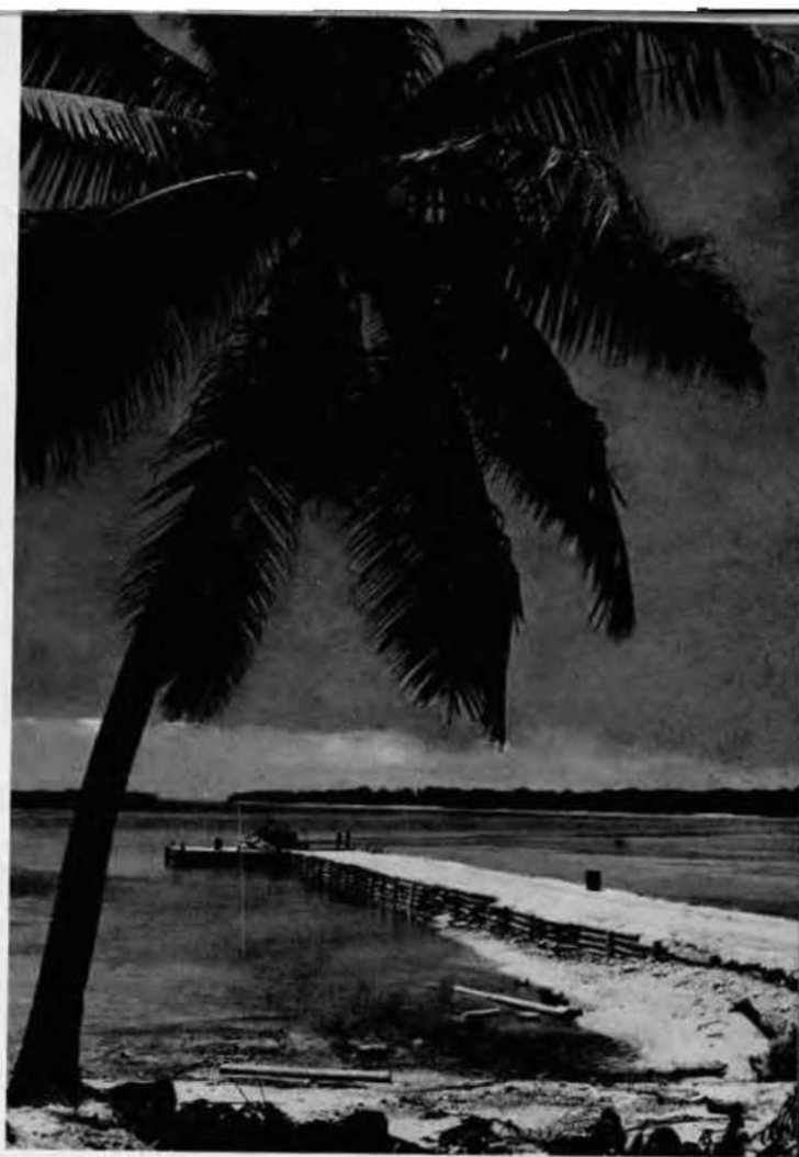
The palm stands like a sentry near the newly constructed pier. The shoreline soon gradually takes on the aspects of a civilized land.
