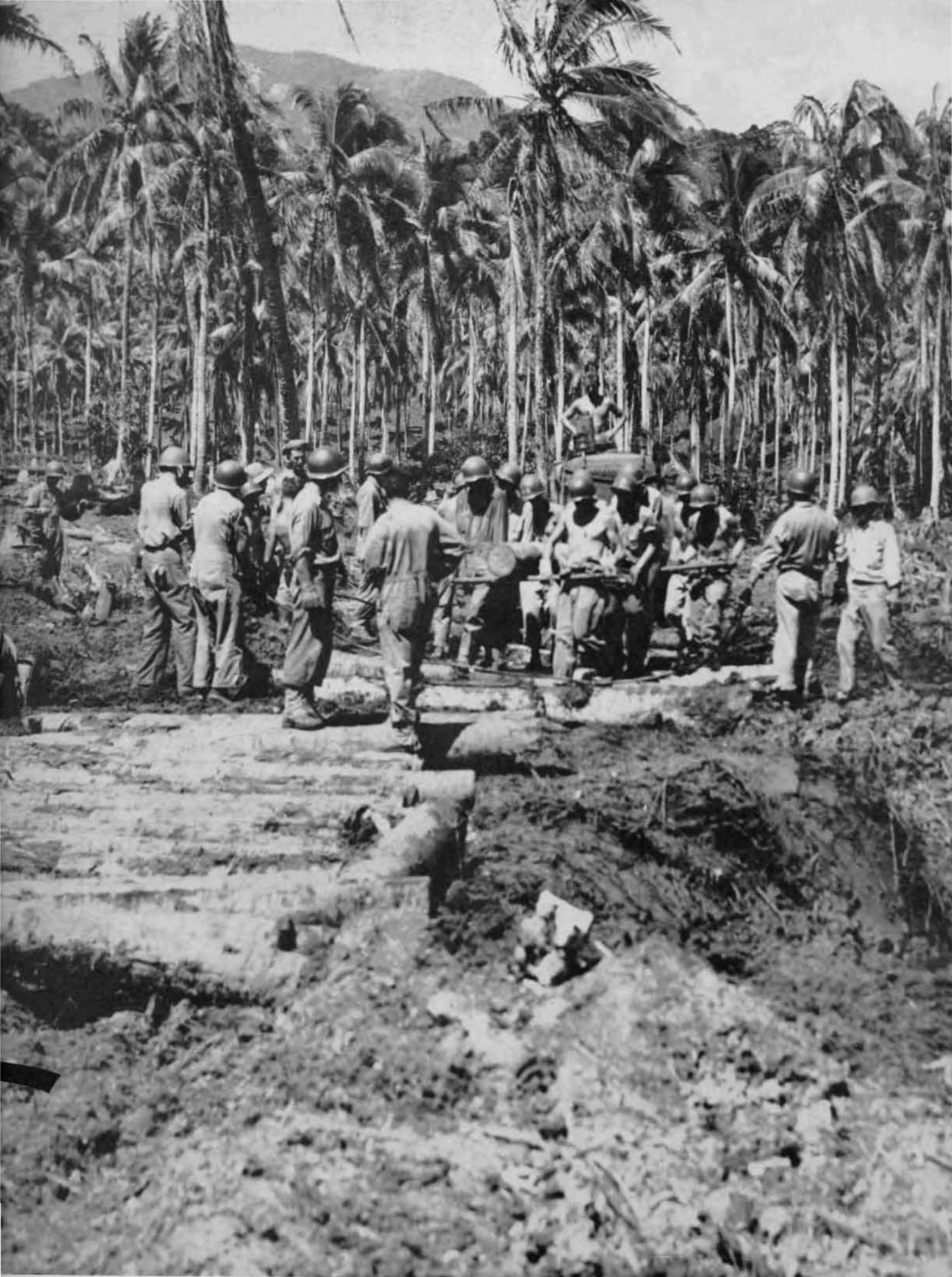
A log road is made through the jungle in the Philippines. U.S. Army photo.
