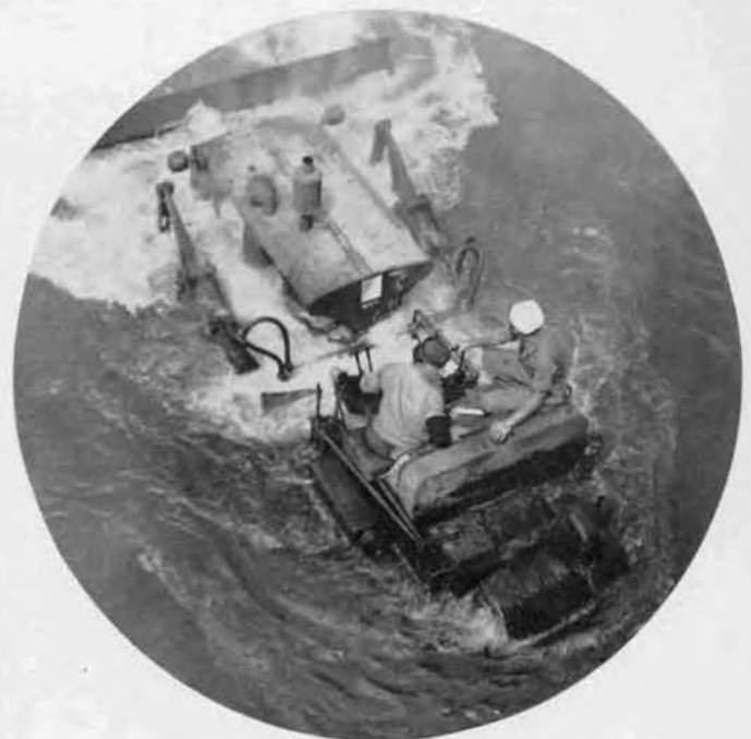
A Seabee tractor backs from shore to ramp over a submerged steel mat. The shot was taken at Port Hueneme, California.
