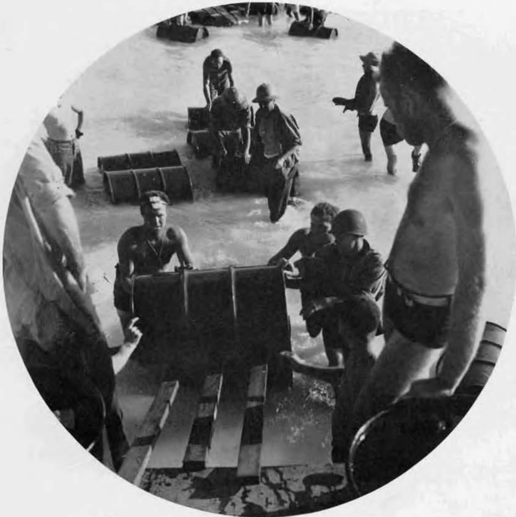
Seabees roll in the barrels. The drums are filled with aviation gasoline.
