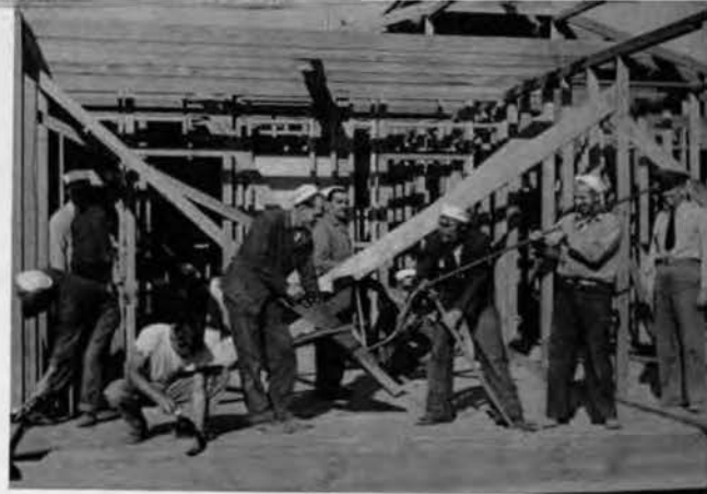
Seventh Battalion men construct new WAVE barracks.
