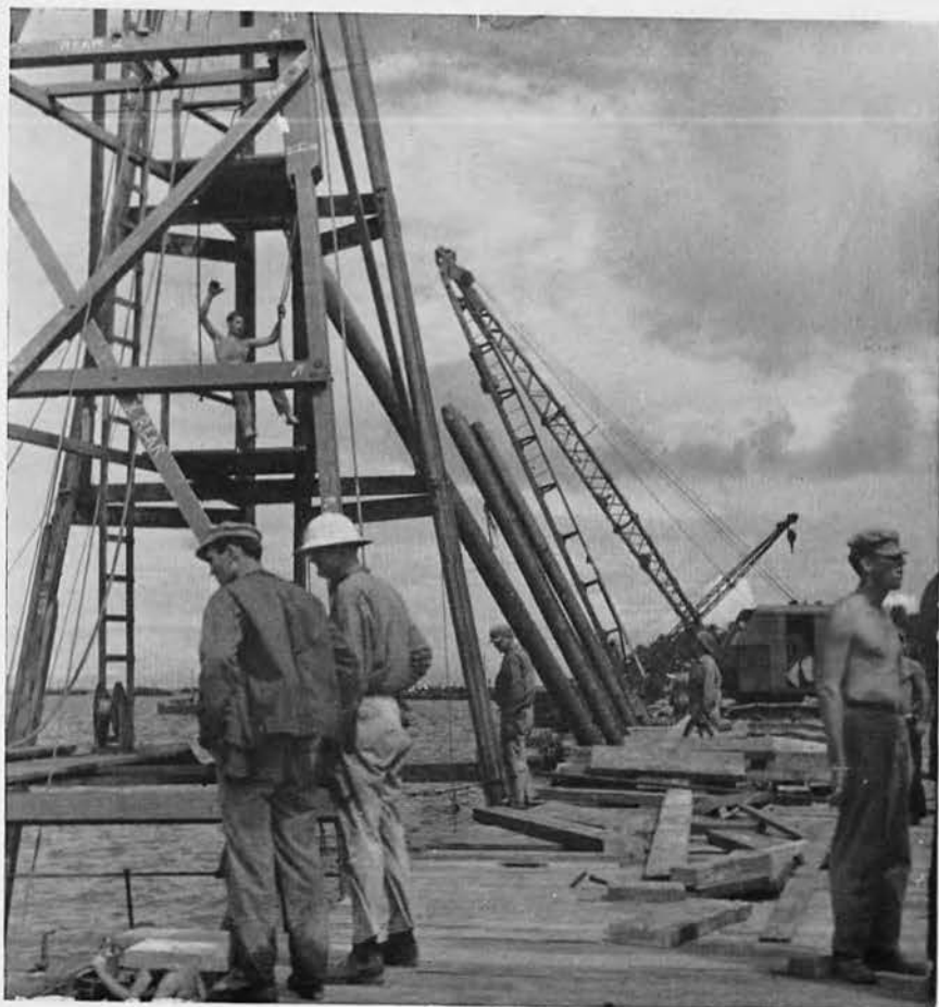
Pile driving operations nearing completion.
