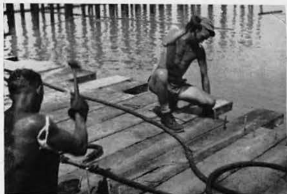
Placing the deck.
