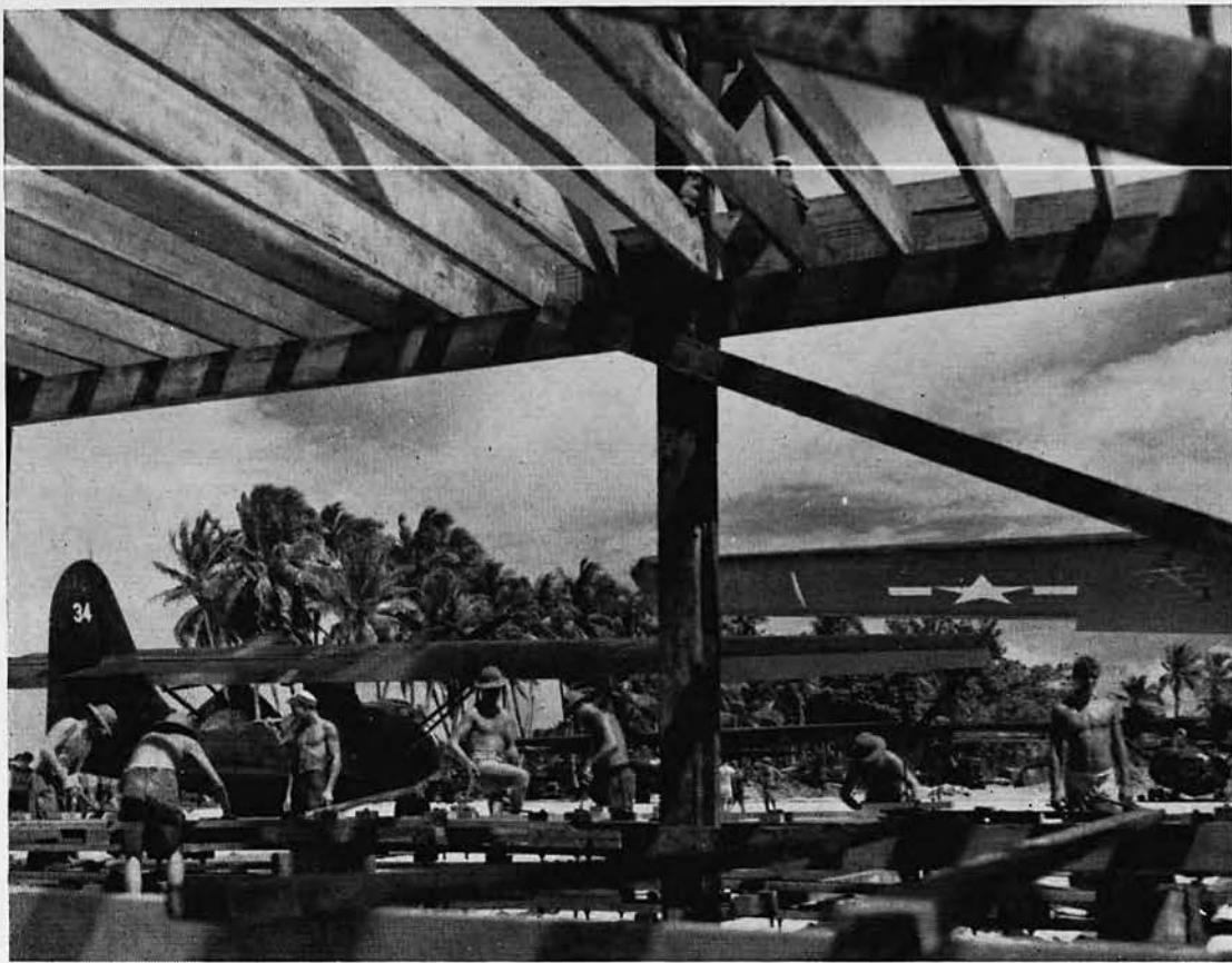
Laying deck for nose hangar.
