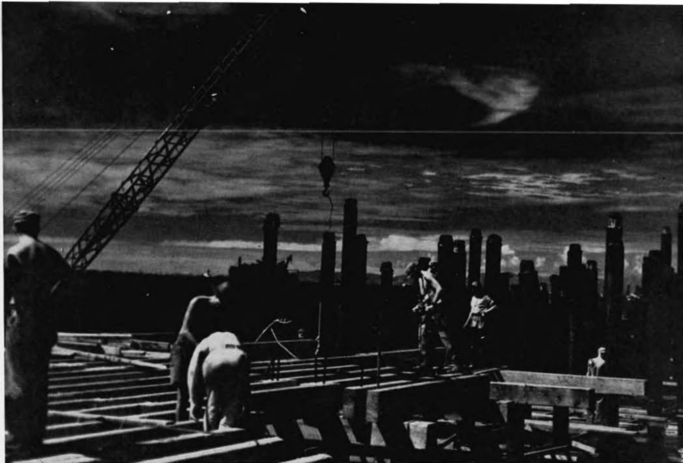
Placing stringers on pile bents.
