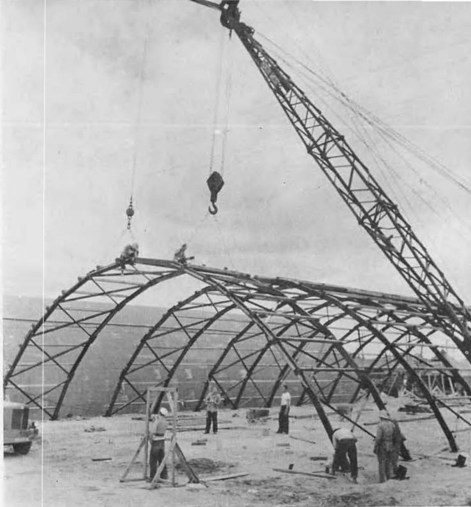
Placing trusses with crane.
