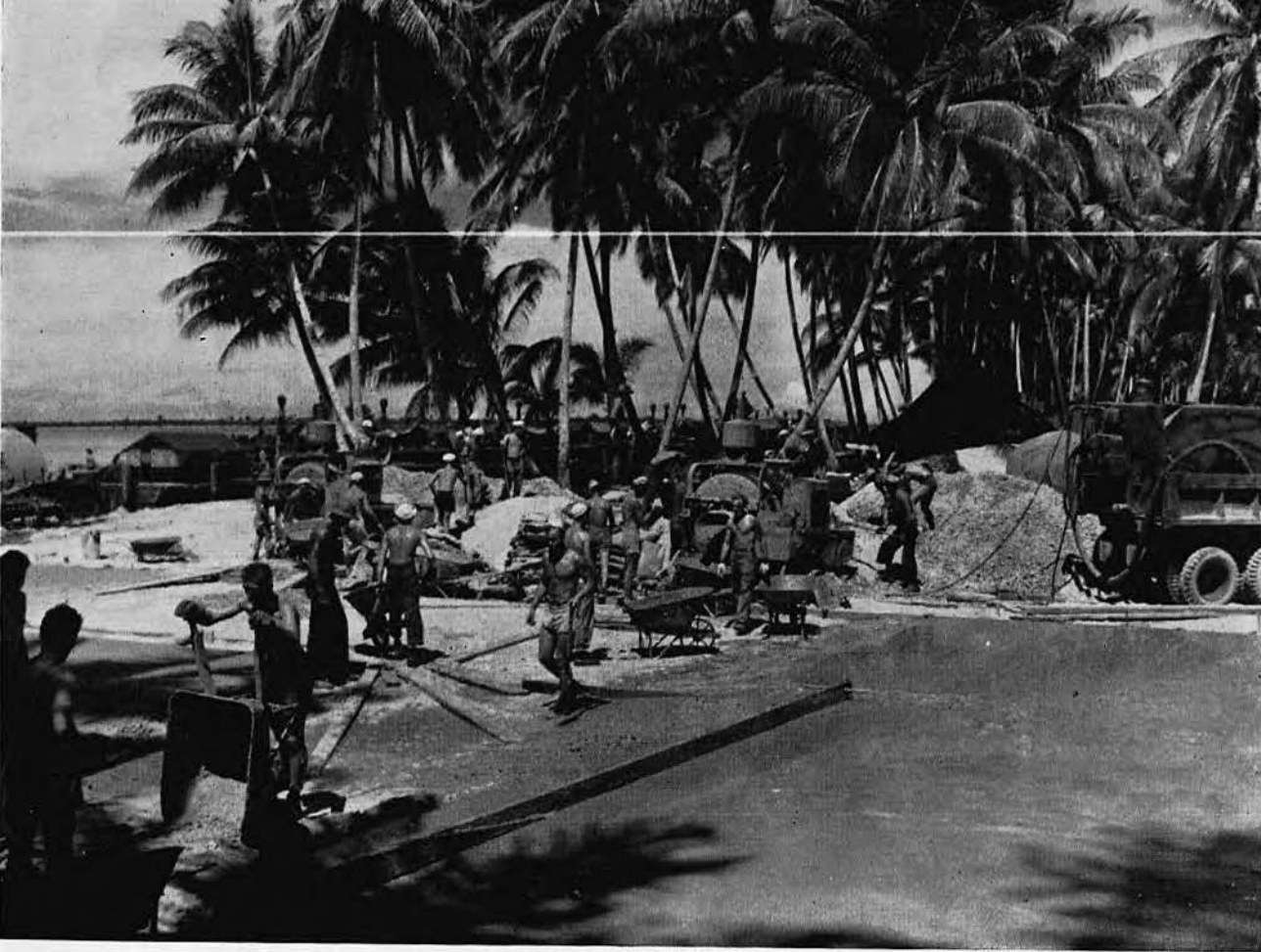
Pouring concrete floors for torpedo shop.
