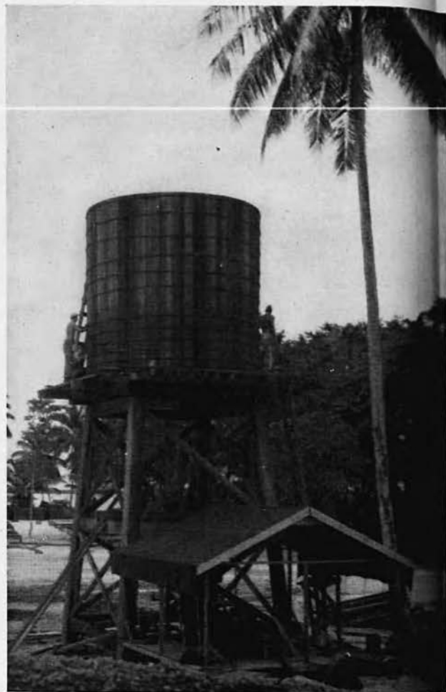
Pumping station and water tower.
