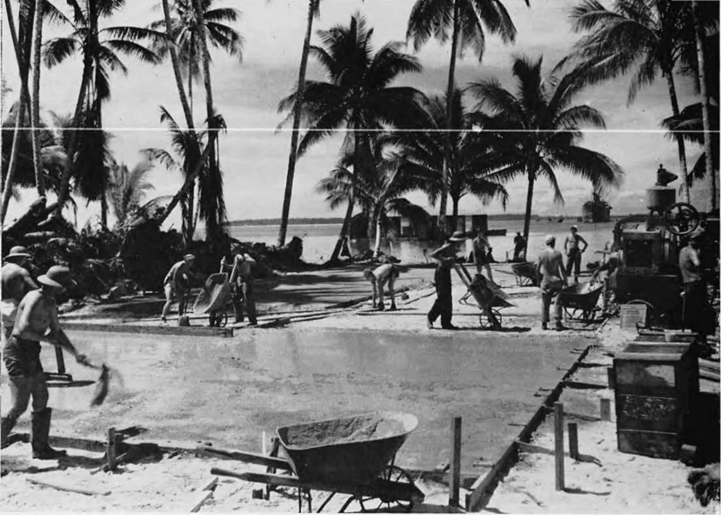
On foundations of concrete, many warehouses and shops rose beneath the palm trees.
