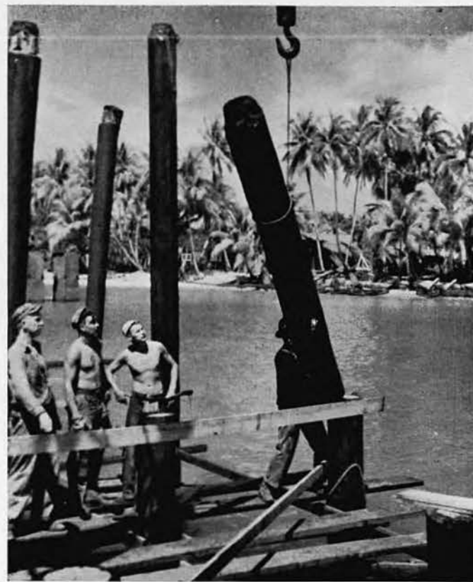
Cutting off piles to grade.
