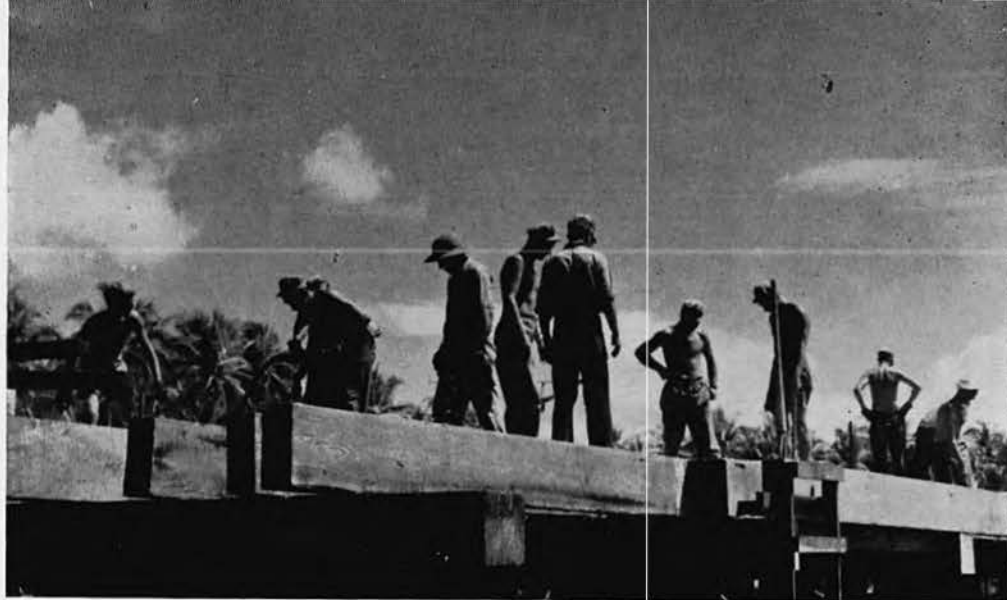
Skilled workmen spent long hours setting heavy timbers.
