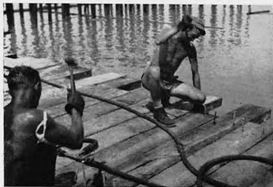
Placing the deck.
