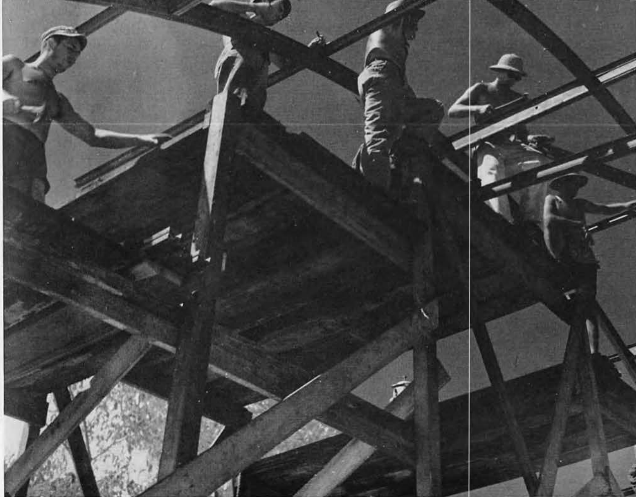
Framing a 40 by 100.
