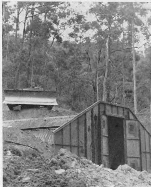
Work at the mine depot.
