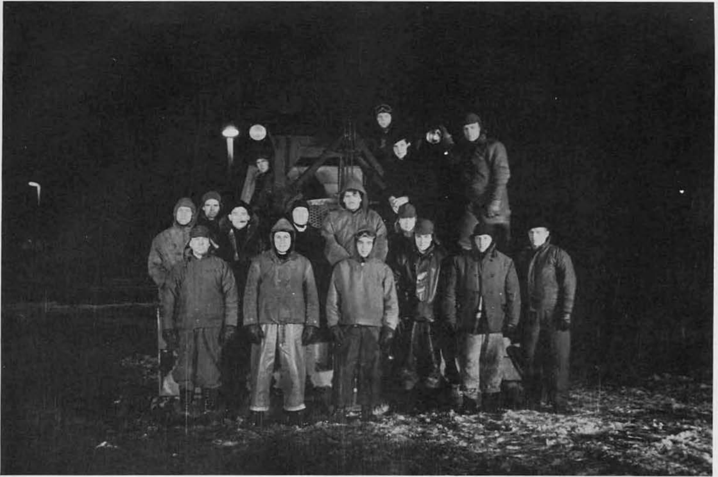
NIGHT ROAD MAINTENANCE
