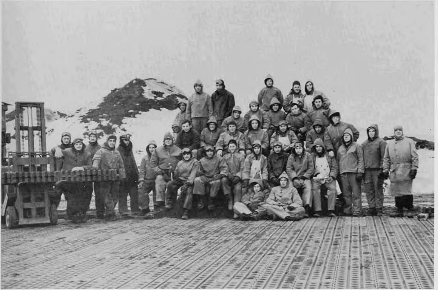
PIERCED PLANK LAYING CREW
