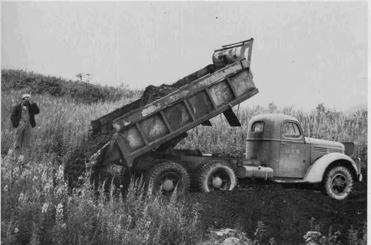
ROAD BUILDING, ISLAND "X"
