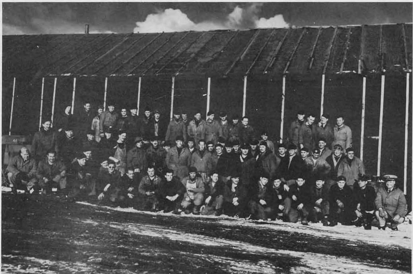
THEY KEPT 'EM ROLLING ON ISLAND "Y"
