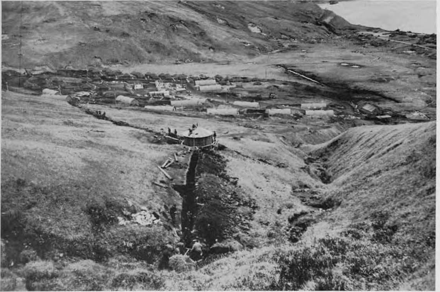
"POLLY CREEK WATER SUPPLY SYSTEM" ISLAND "Z"
