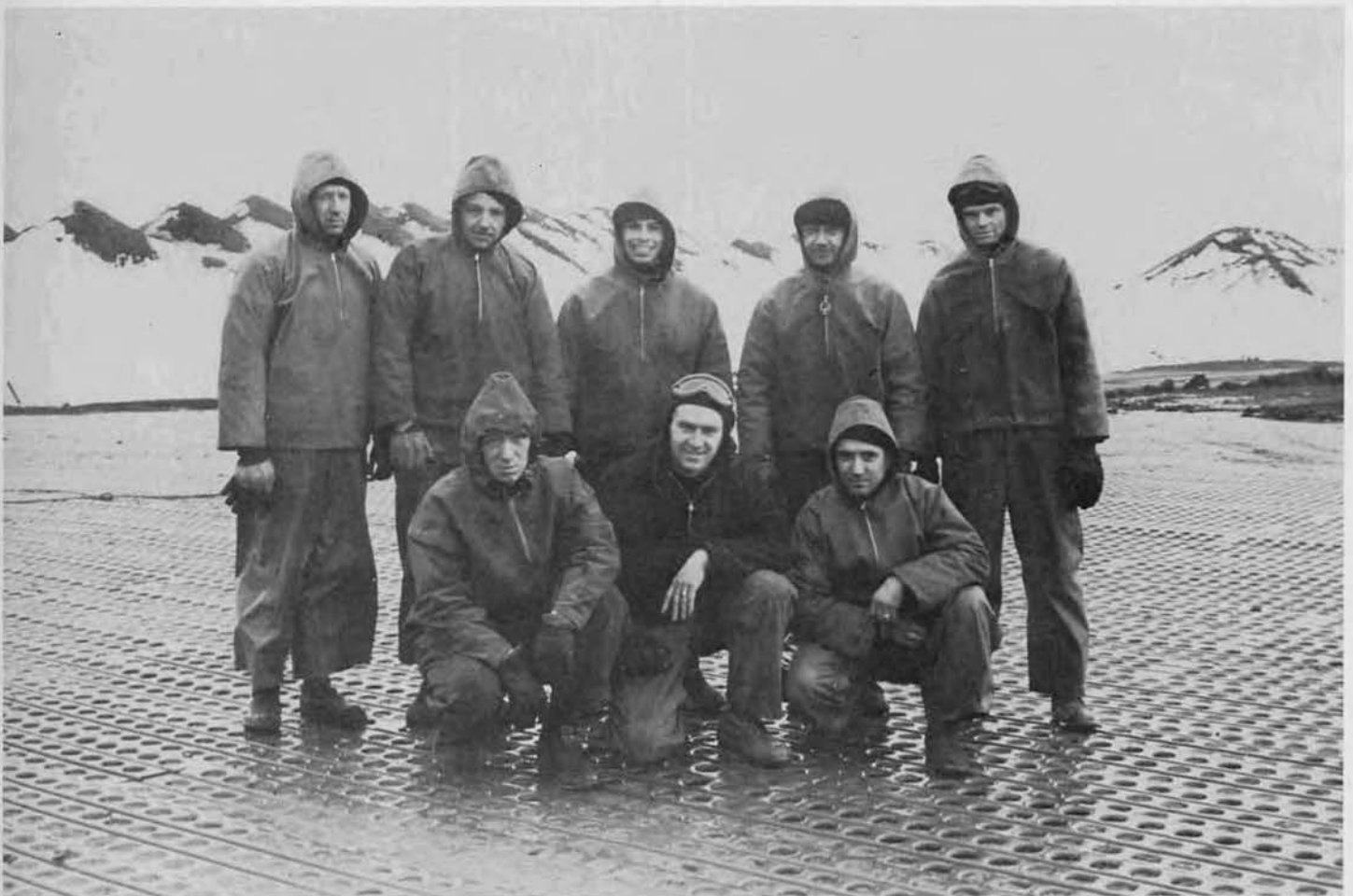
DAY ELECTRICAL CREW
