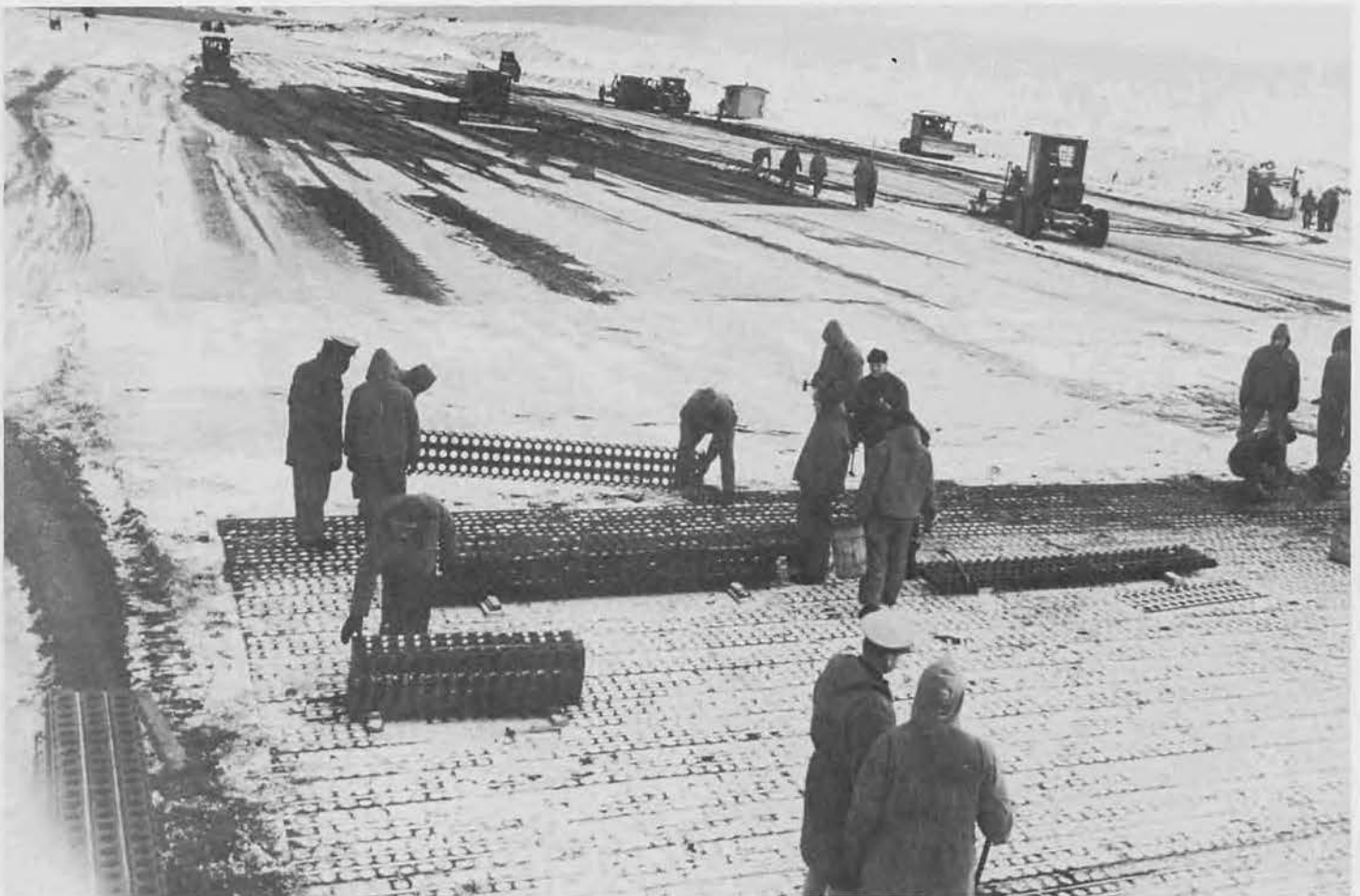
LAY THAT PLANKING DOWN, BOYS!
