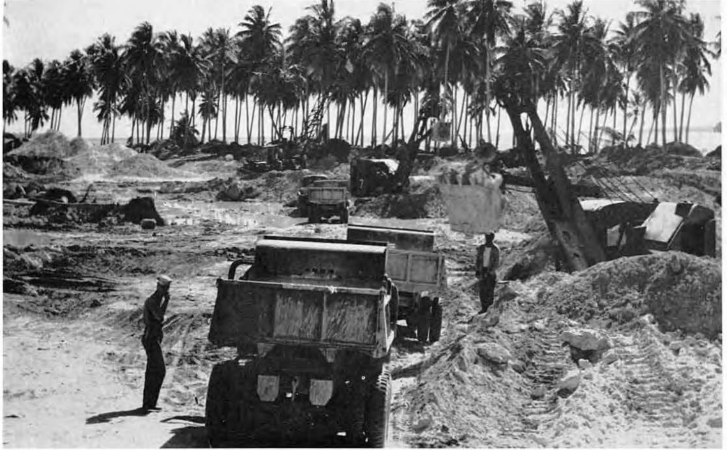
This is the Bougainville airstrip, in preparation.
