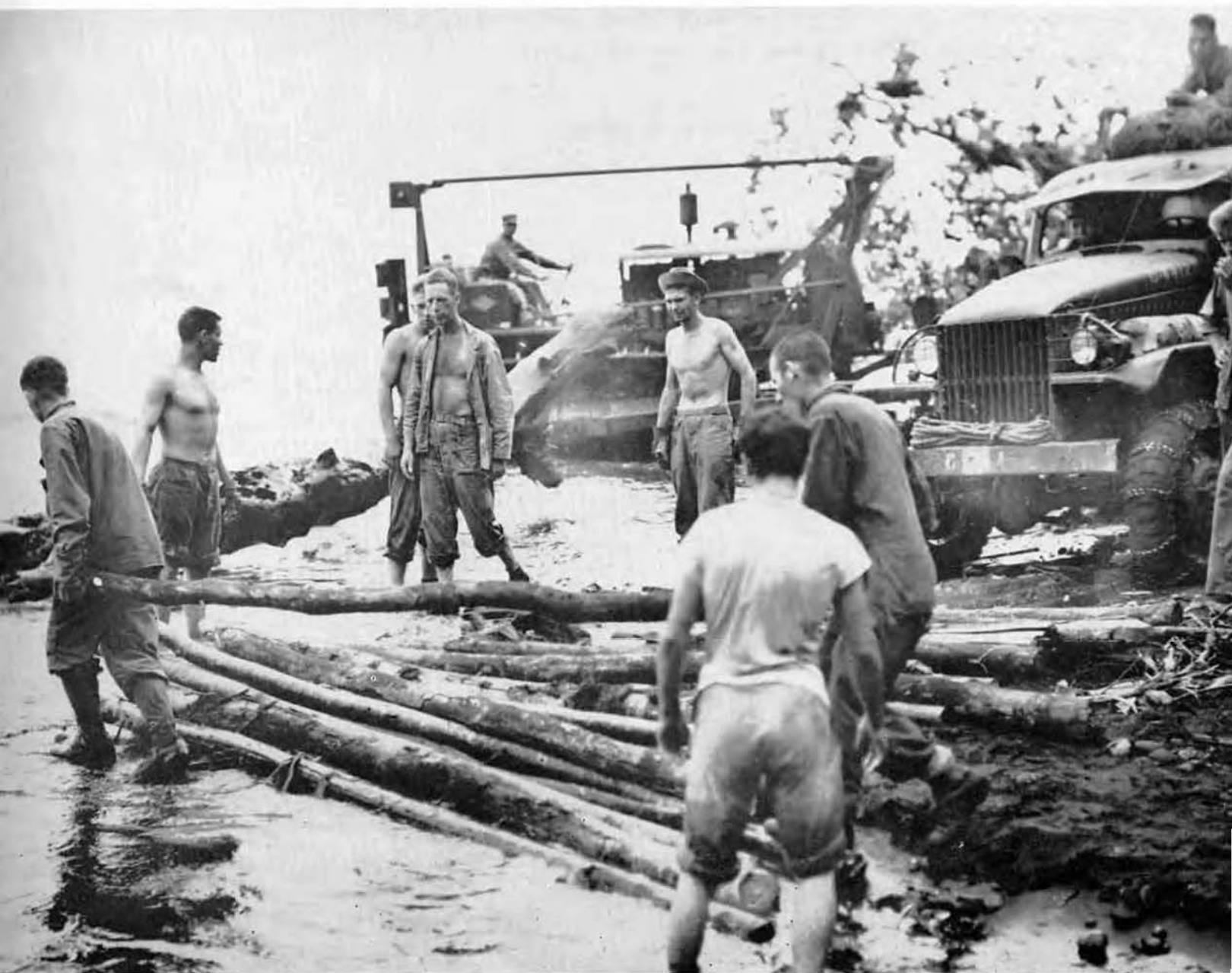
Trees and logs are put in place by Marines and Seabees for a bridge across a jungle stream on New Britain Island.
