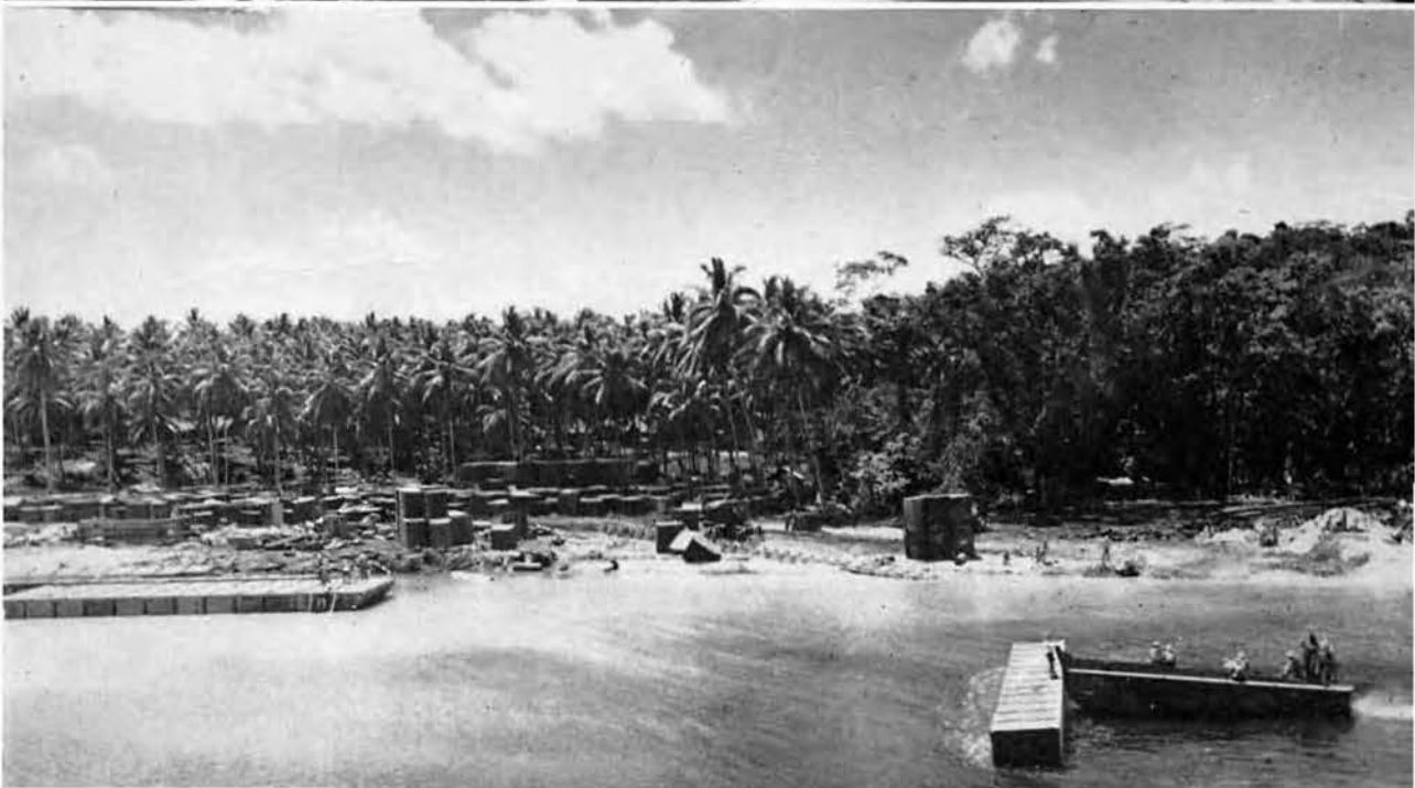
Getting part of dock in place, Banika
