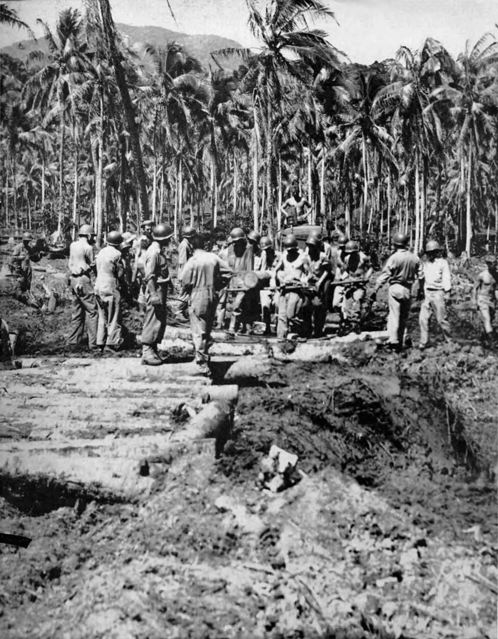
A log road is made through the jungle mud on Rendova Island. Coconut palms felled along the route served as a ready supply of road building material. Heavy artillery of the Marines was carried over this road to a point where it was in range of the Jap stronghold at Munda.
