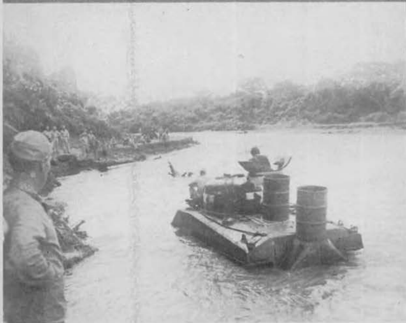
Those tanks we waterproofed
