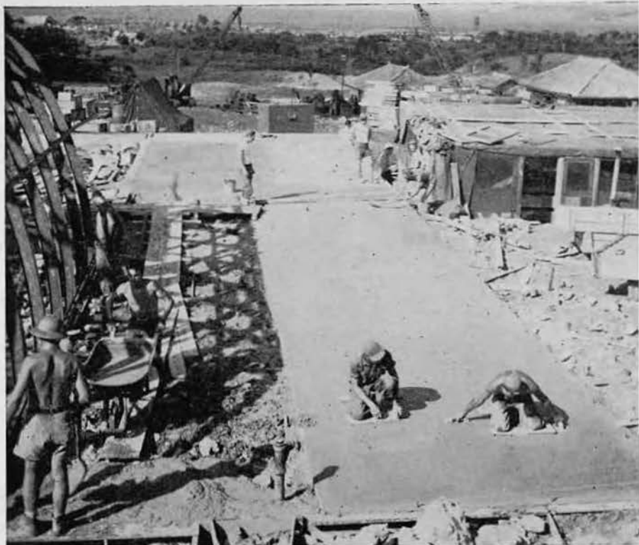
Finishing Concrete Slab for Reefers
