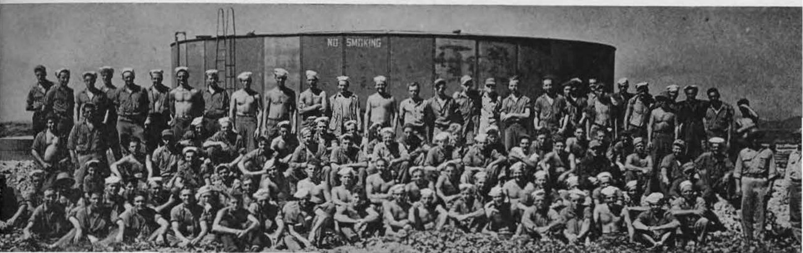
Tank Erection Crews
