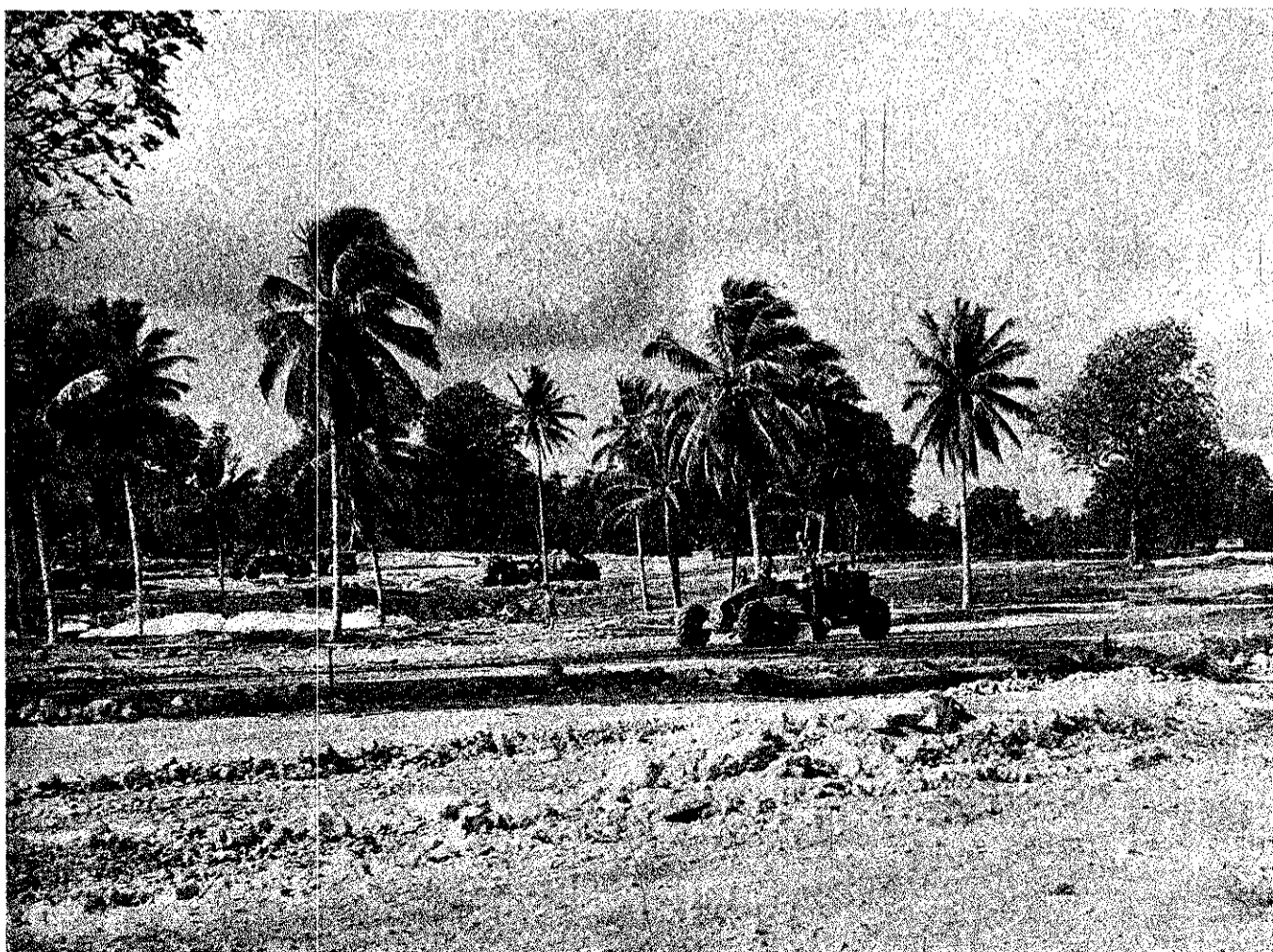
“CLEARING THE NEW AREA”
