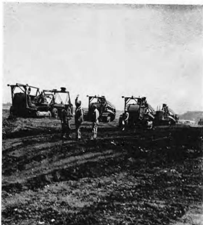
CARRYALLS STRIPPING BEFORE FILL
