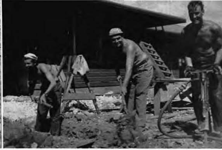
DIGGING THE DITCH
