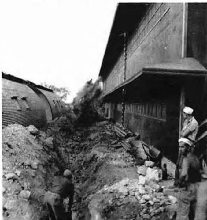
DITCH BLASTING, EWA
