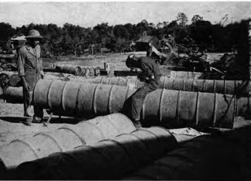
FUEL DRUMS, TO BE MADE INTO CULVERTS
