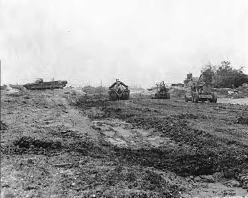
PURPLE BEACH ROAD UNDER CONSTRUCTION
