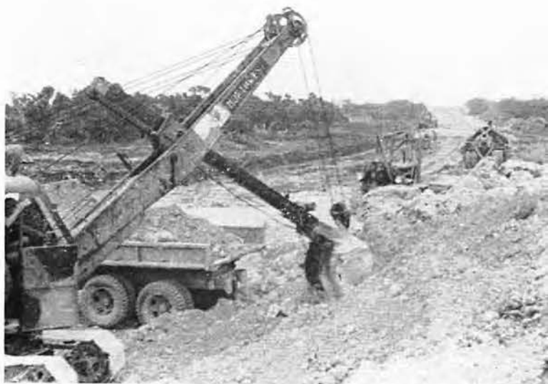
SHOVEL MAKING CUT FOR ROAD
