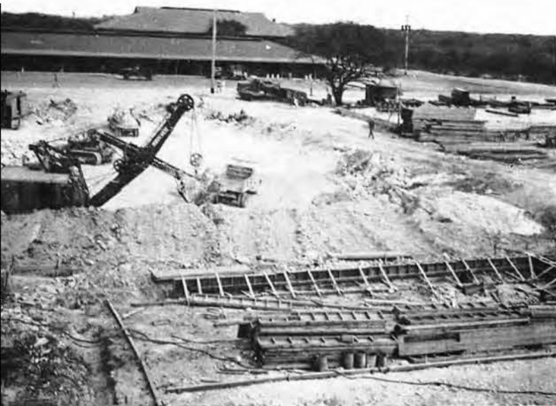
SWIMMING POOL EXCAVATION, EWA
