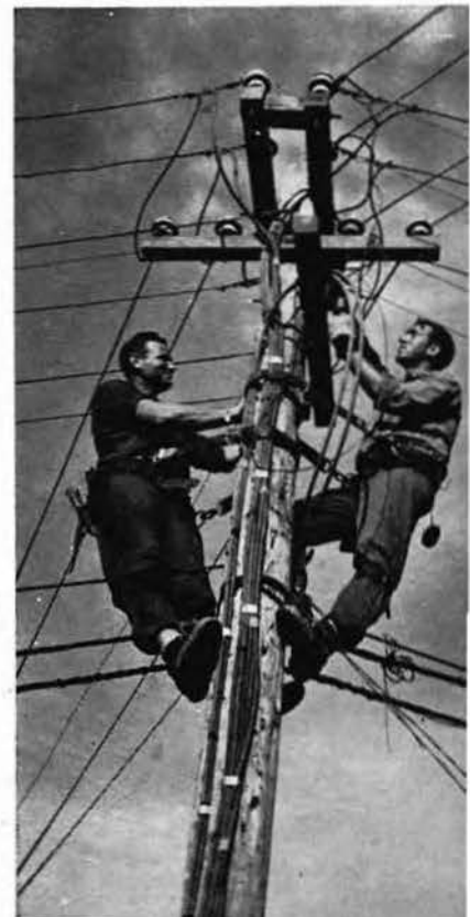
LINEMEN AT WORK
