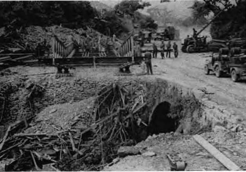
BAILEY BRIDGE UNDER CONSTRUCTION
