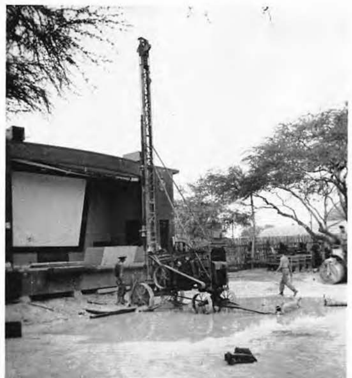
DRILLING DRYWELL, EWA
