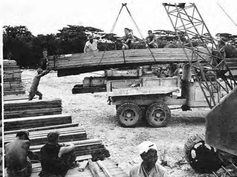
CREW UNLOADING LUMBER
