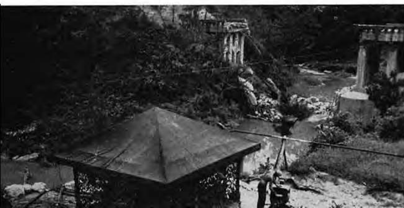
PUMP HOUSE ON BISHA GAWA
