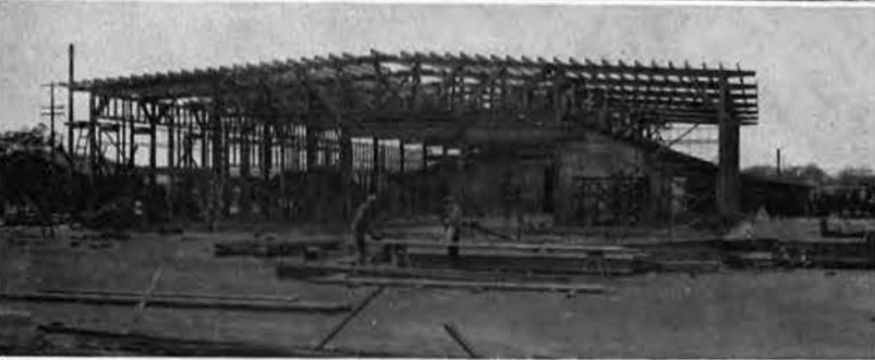
PUBLIC WORKS GARAGE ANNEX
