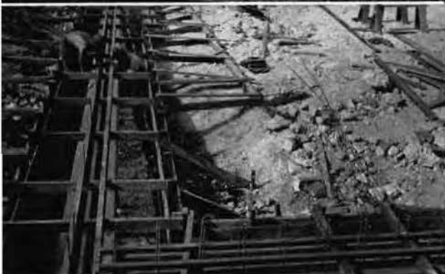
REINFORCING STEEL IN CONCRETE
