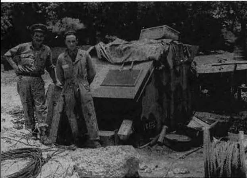
TWO MEN FIND USE FOR THE ARMORED DOZER CAB
