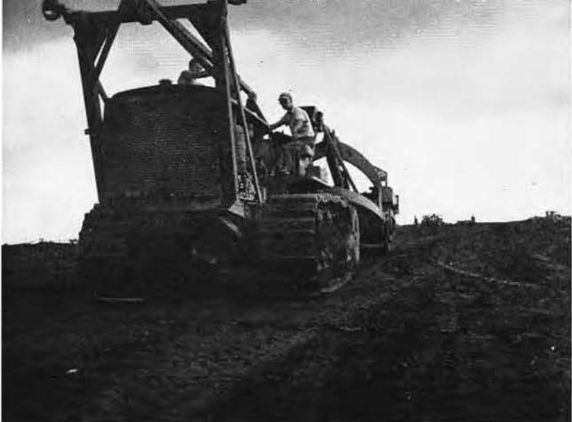
D-8 DOZER AND PAN STRIPPING
