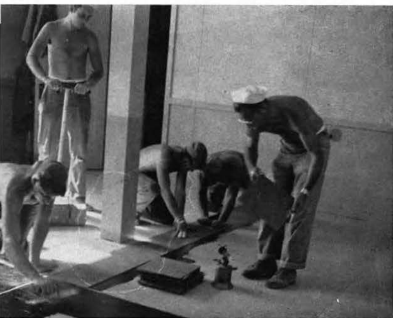
LAYING ASPHALT TILE
