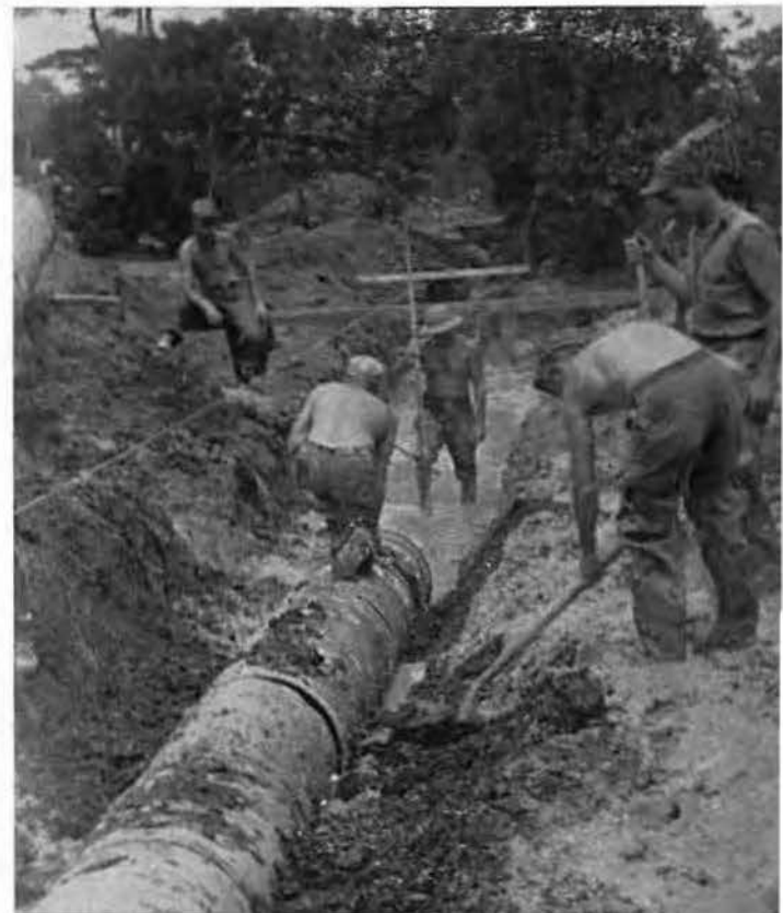
INSTALLING CULVERT FOR CAMP DRAINAGE
