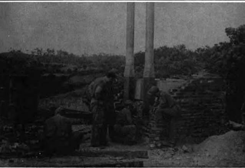
INSTALLING BAKING OVENS, OKINAWA
