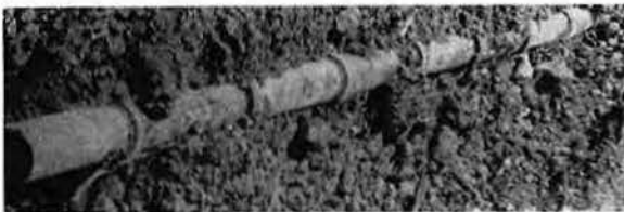
WELDING DRUMS INTO CULVERTS
