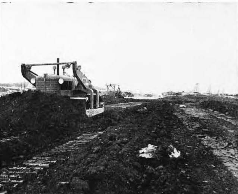
DOZER STRIPPING ON SUB-GRADE
