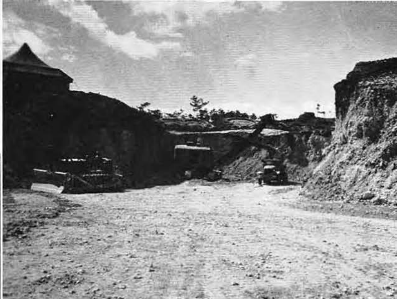
SHOVEL DIGGING CORAL FROM PIT
