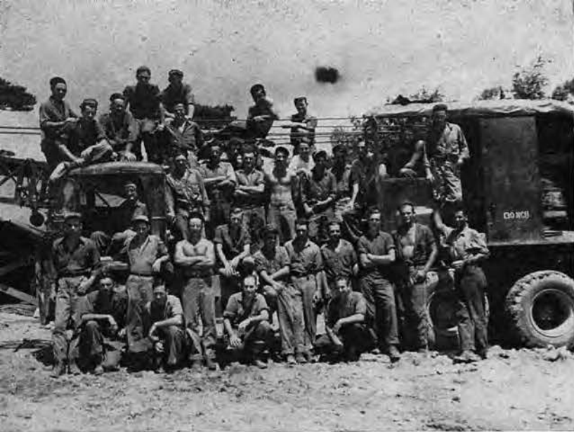
REPAIR AND RIGGING CREWS
