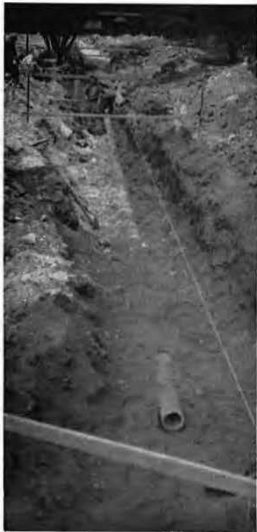
A LINE BEING LAID
