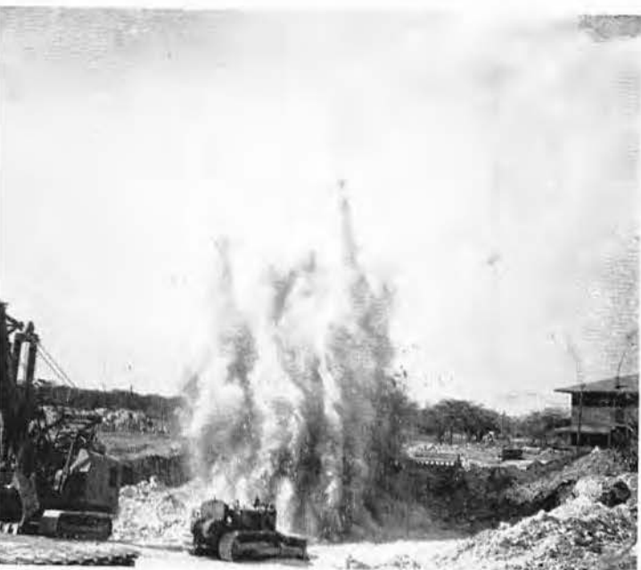
BLASTING FOR MCAS SWIMMING POOL
