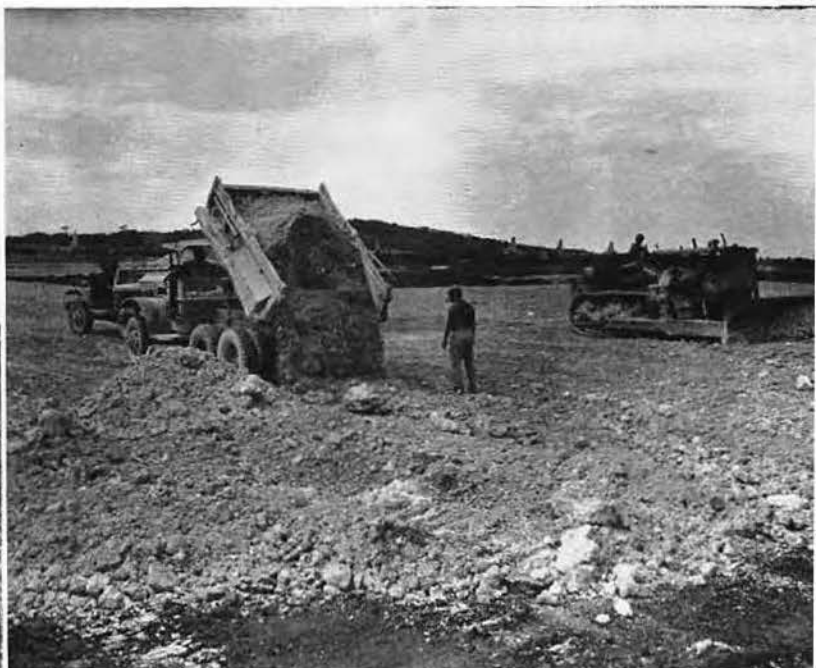
TRUCK DUMPING CORAL FOR SURFACE
