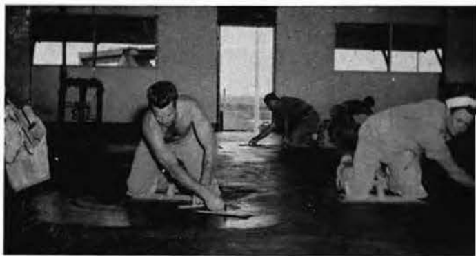
FINISHING CONCRETE
