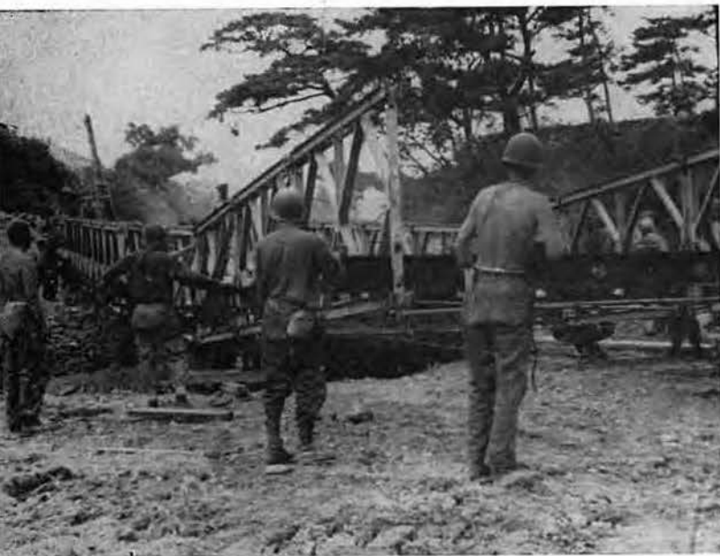
SAME NEAR COMPLETION, BISHA GAWA
