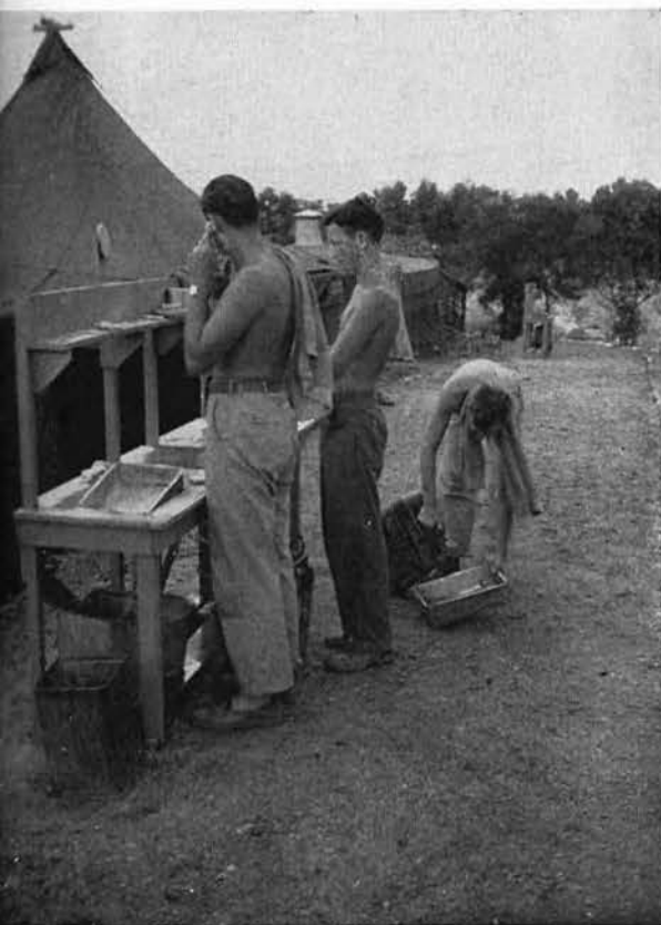
WE RIG UP WASH BASINS
