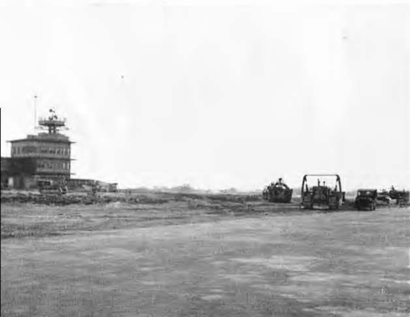
CONTROL TOWER AREA, EWA
