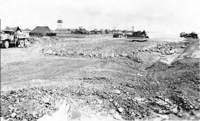
TAXIWAY UNDER CONSTRUCTION
