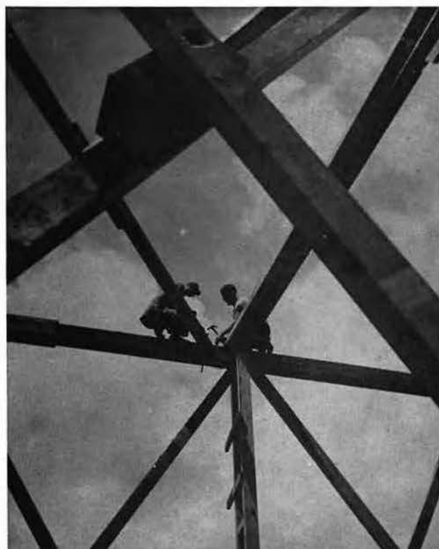
MEN WORKING ON CONTROL TOWER FRAME
