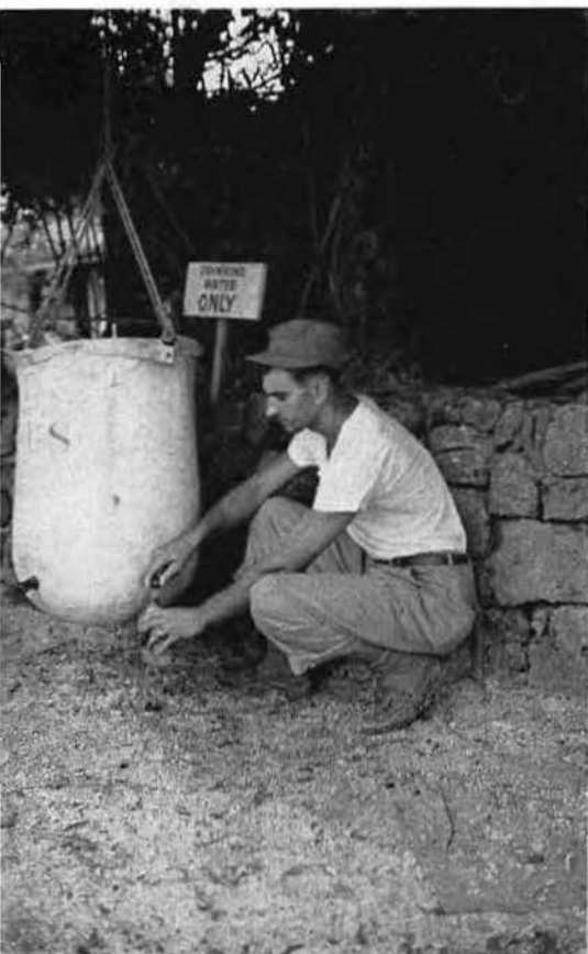
CANTEEN WATER POINT
