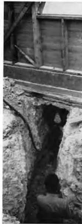
HARD DIGGING BEFORE INSTALLATION
