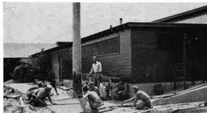
INSTALLING RAMP AND WALK, EWA
