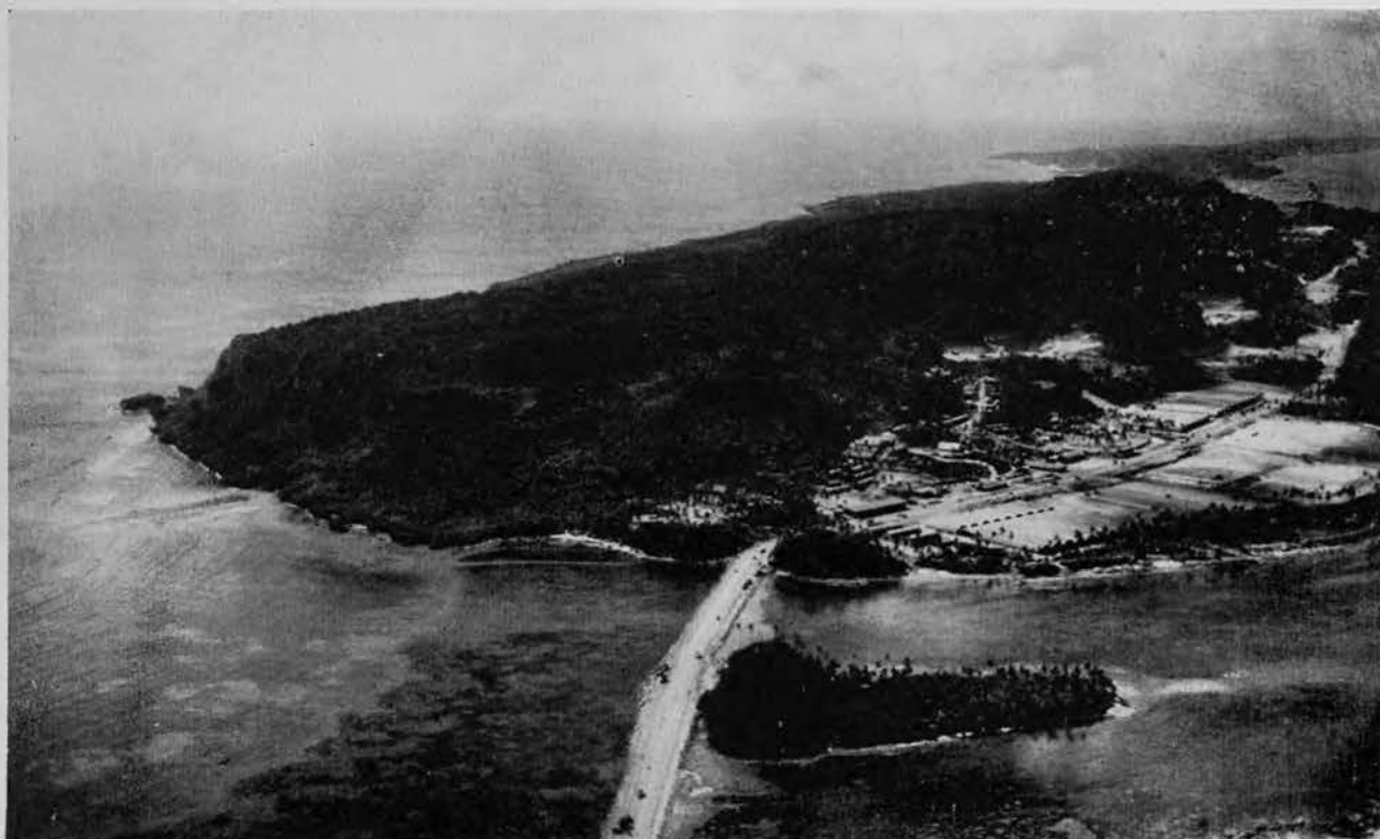
AERIAL VIEWS OF 123RD AREA ON CALICOAN
