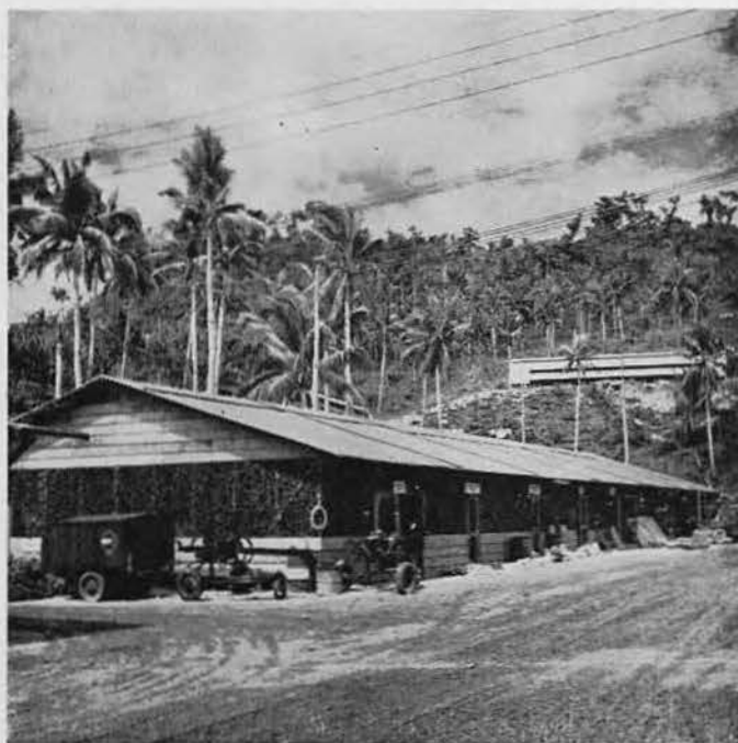
PNEUMATIC TOOL, ELECTRICAL, SHEET METAL AND PLUMBING
