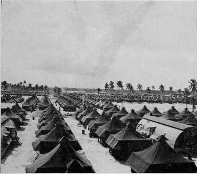
TENT CITY CONSTRUCTION AT RECEIVING AREA
