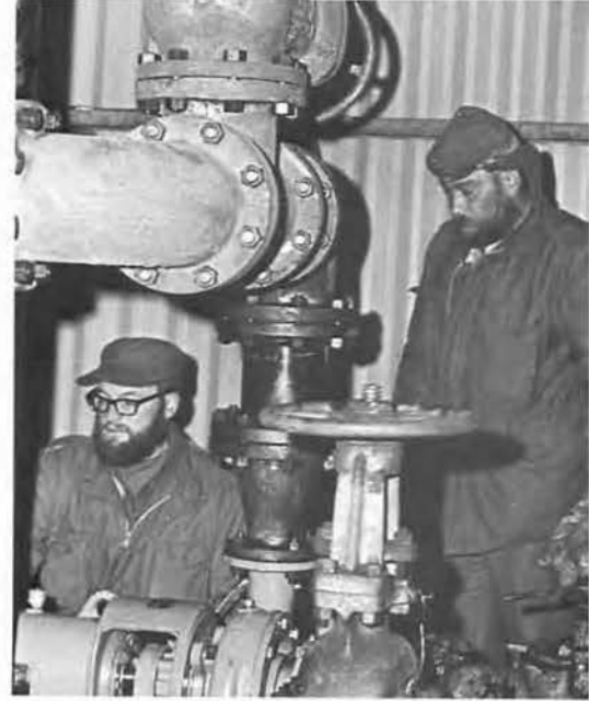
LTJG R. Oschner, left, and CE1 Frank Luck, right, are getting into a thing while inspecting new facilities at the pump house on Scott Point.
