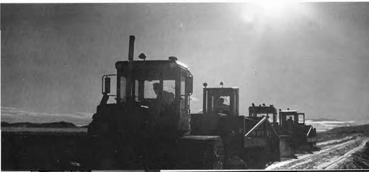
Surfacing snow roads with pulva-mixers
