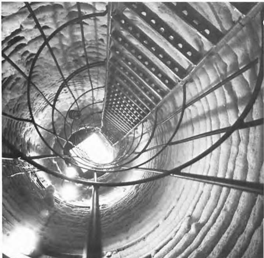
An emergency escape ladder ties the station with the surface in the event normal tunnels are blocked.
