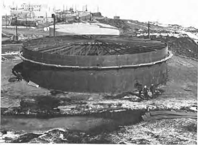
SW's of 201 put up this 500,000 gallon tank at McMurdo during the summer season.
