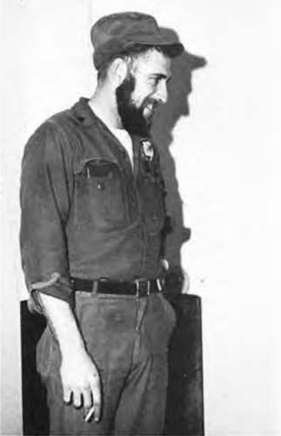
Supervising kept BU2 Olen Billen busy at M-46.
