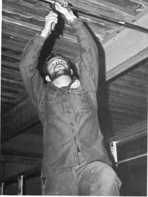
CECA Brian O'Donnell installs electrical piping.
