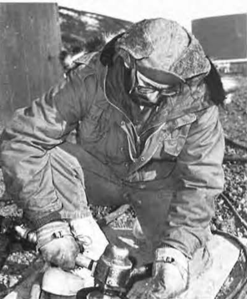
SW3 Ken Welch welds deck plating at the big tank.
