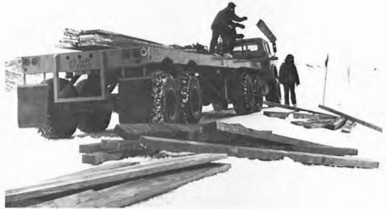
Off-loading lumber for road repairs
