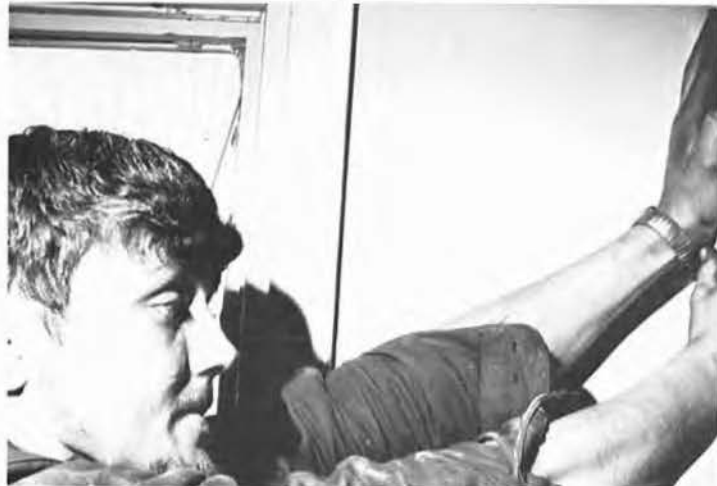
UT3 Steve Mettling IS holding up the wall.
