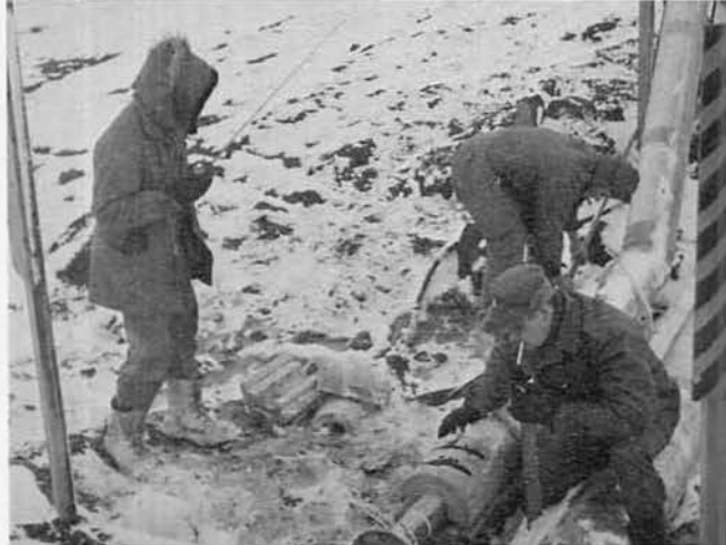
UTC James McFarren, "B" Co. Cdr. inspects installation of water line.
