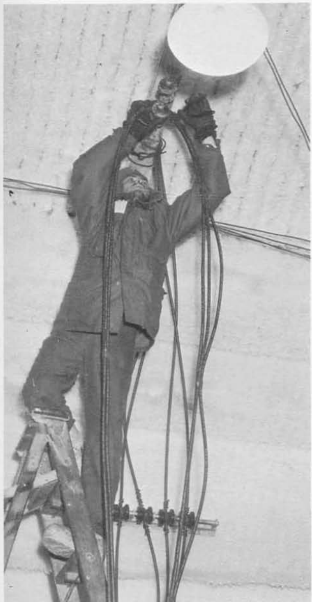
Paul Howard wires overhead light at Byrd Station.
