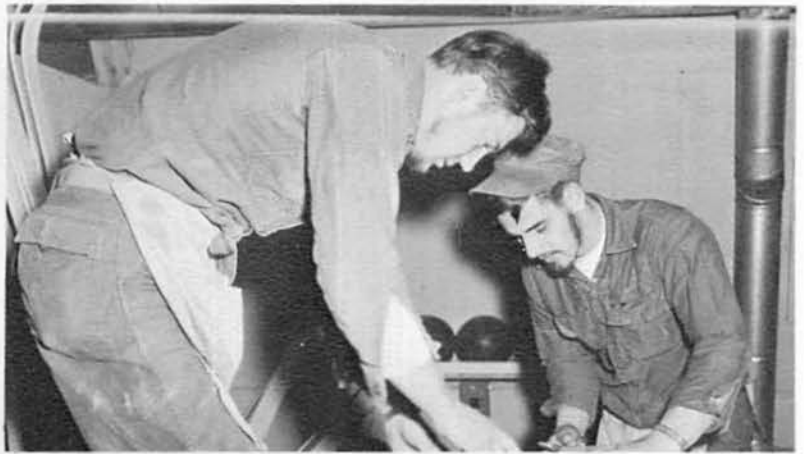
Cooper and Zdravec finish off the edges of the wallboard.
