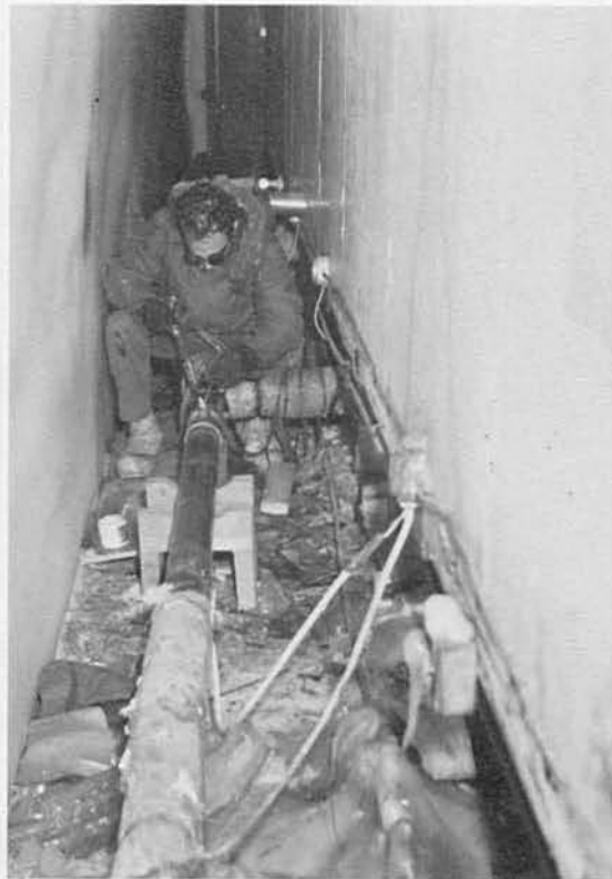
Donald Havens solders a sewer joint at Byrd Station.
