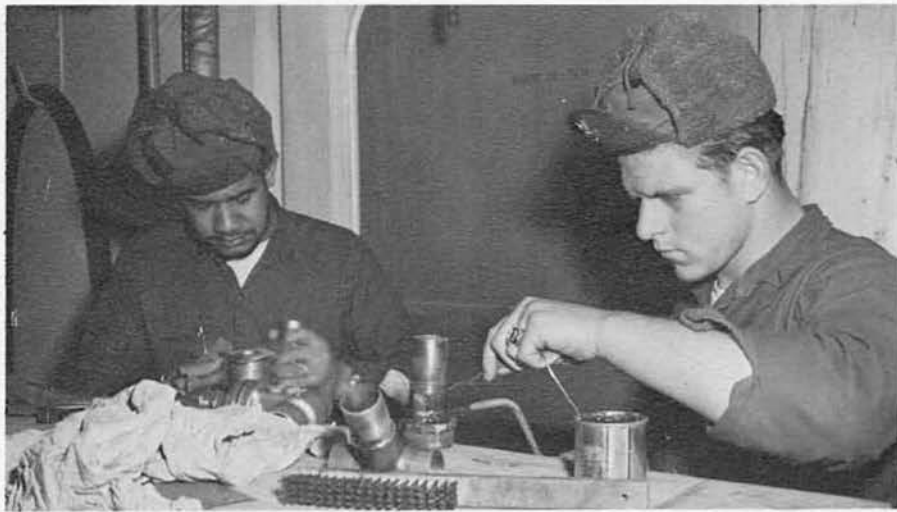
ABOVE - UTP2 Albert Beverly and UTP2 Arlan Gooden make repairs on a snow melter.
