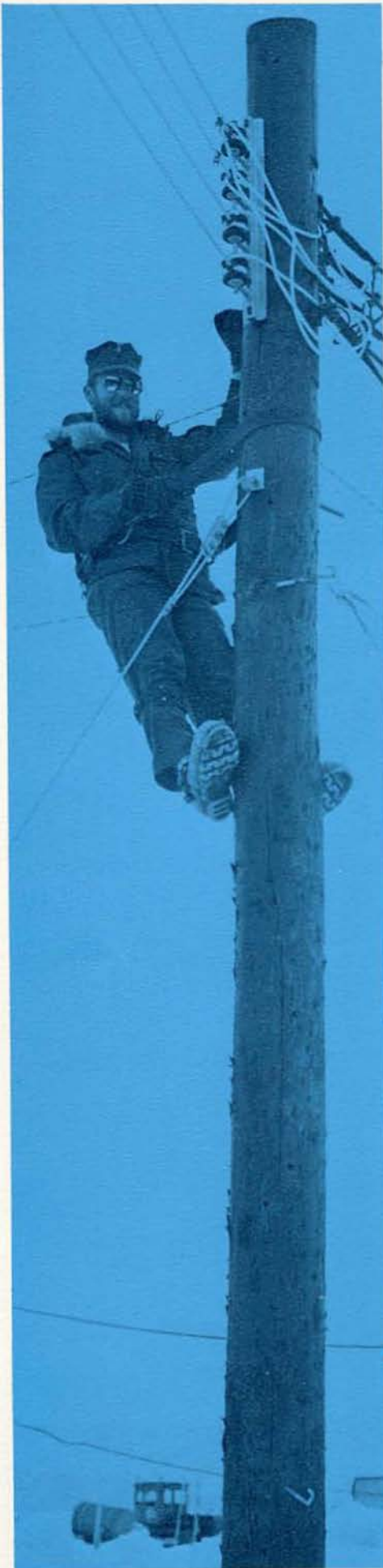
LEFT - EMS William G. White on another "south pole" at Williams Field. Ice and permafrost provide an effective barrier against underground lines, so most are strung on telephone poles.
