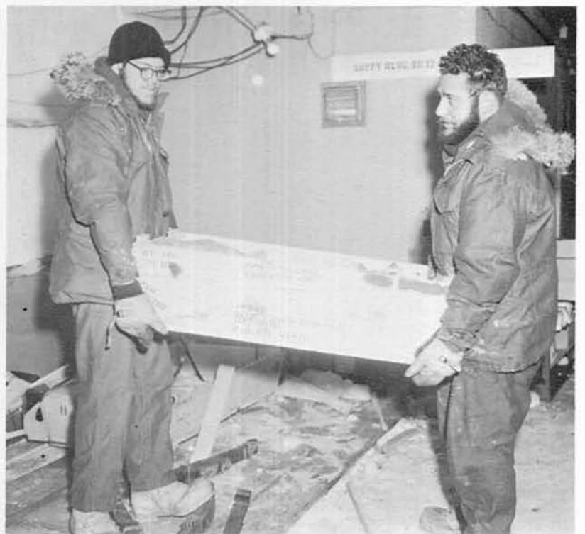
SKSN Ronnie Lee and SK2 George Breeding unload and store supplies in the supply tunnel.
