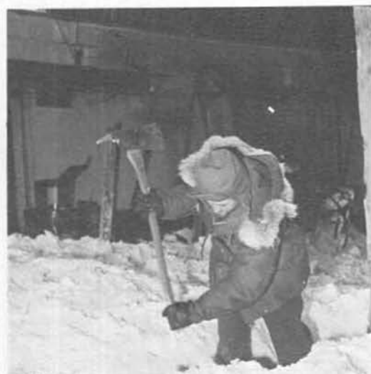
Paul Brooks digs for buried fuel line at South Pole Station.
