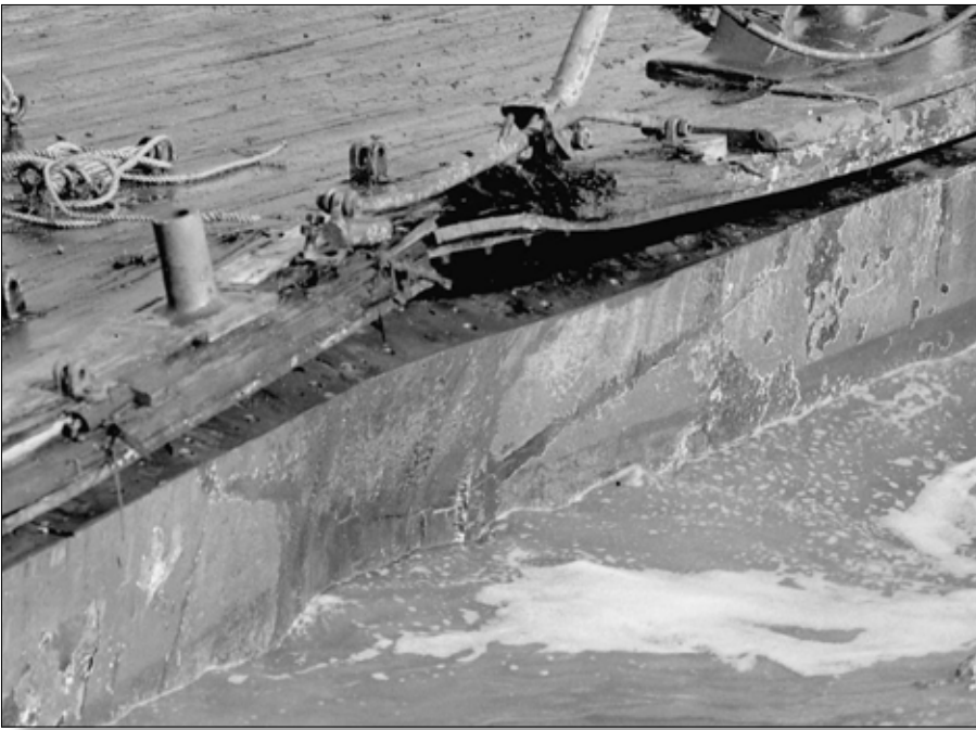
A closer photograph of the waterline test reveals that the damage was worse than first suspected. Although the water's depth at the Middle Ground was only one foot deeper than the monitor's draft, salvage crews four days later discovered Puritan had sank seven feet into the mud. (Courtesy the Library of Virginia)
