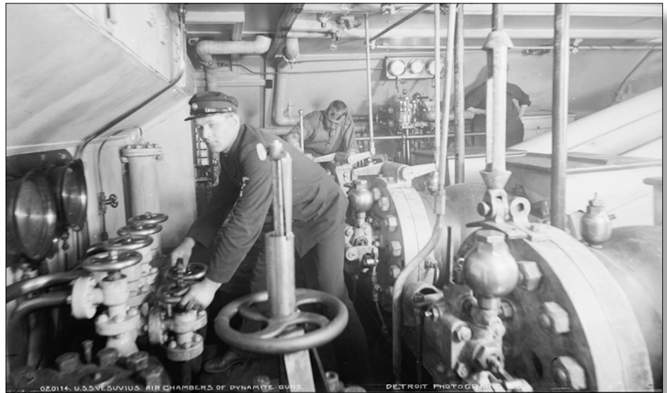
A Navy Machinist adjusts the air pressure flowing from air compressors into air storage tanks, where pressure as high as 1,000 pounds per square inch was maintained in order to shoot the 10.5-inch-wide projectiles (below). A witness to one of Edmund Zalinski's early tests recalled, "an engineer turned a crank up by the breech, there was a sudden hiss as of steam escaping from a locomotive, and the next instant, with a screech like a monster sky rocket, the projectile went sailing into space." (Detroit Photographic Co. Collection, Library of Congress)
