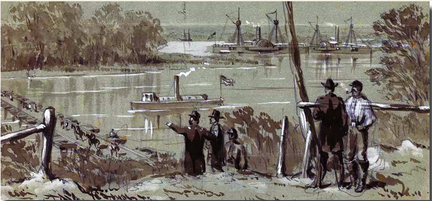
Alfred Waud drew this pen and ink sketch of Deep Bottom (named because of the unusual thirty-five foot depth in the river), where Fourmile Creek meets the James River. Located about twenty miles upstream from City Point, Butler's troops built a pontoon bridge across the river to establish communication and a supply line with Grant's forces located farther north. Shown here are troops from the 10th Corps's 2nd Division marching north across the bridge and their leader, Major General Robert Foster, overseeing the move. Two "double-ender" gunboats, USS Mendota and Mackinaw, stand by at Fourmile Creek with their guns facing north, ready to assist. No information is available on the man on the bridge who decided to ignore all the activity and go fishing. (Library of Congress image)
