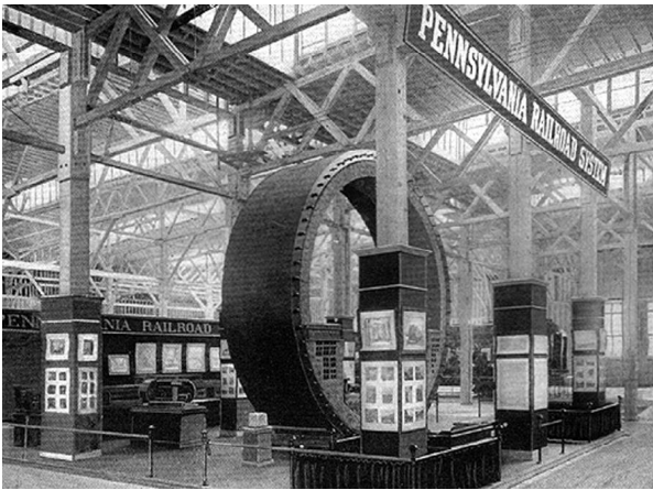
The mighty Pennsylvania Railroad, one of the largest transportation companies in the world, vainly displayed its corporate power at the Machinery and Transportation Building. Central to the exhibit was a sample of the steel ring to be used in the company's future tunnel project underneath the Hudson River. (Photo from the Official Blue Book of the Jamestown Ter-Centennial Exposition)
