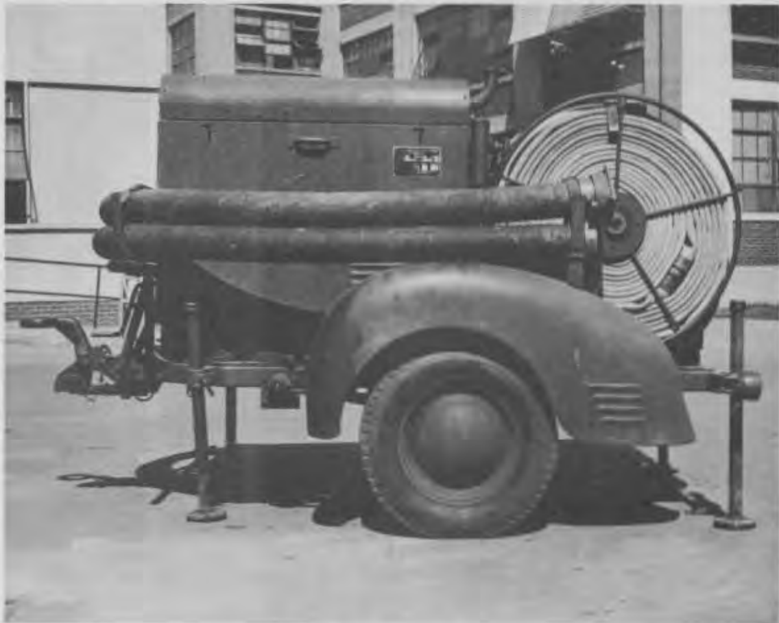
TRAILER FIRE PUMP (2H93)
