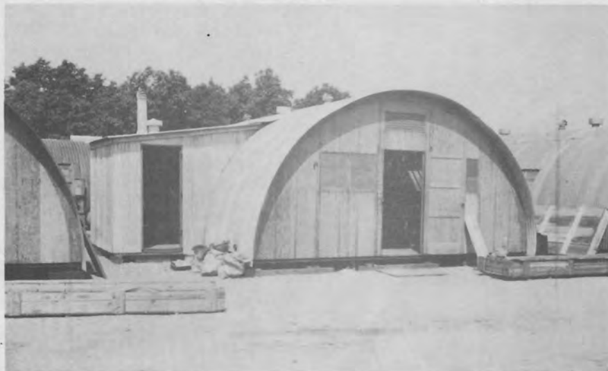
LEAN-TO ON SURGERY HUT
